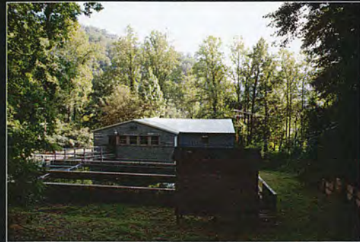
D. Rear Yard And Concrete Water Tanks, View North
