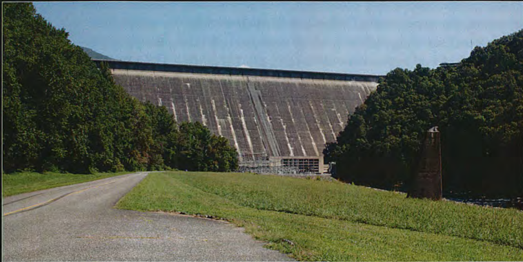
A. View of Fontana Dam, Looking Northeast
