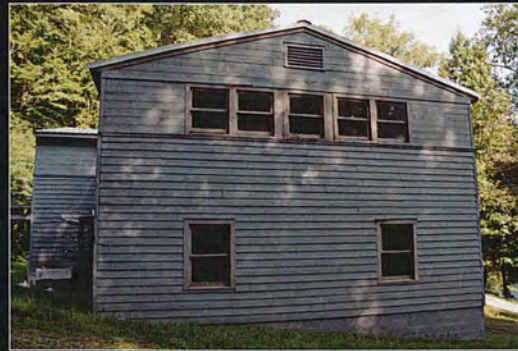
F. East Elevation, View West
