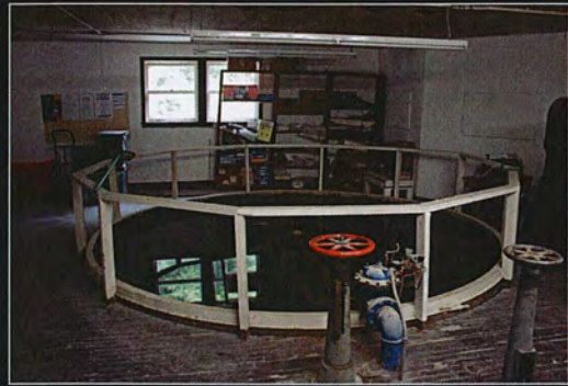
D. Top of Water Tank on Second Story, View East
