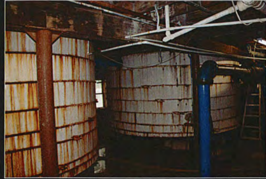
B. Original Redwood Water Tanks, View East
