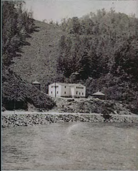
C. Exterior View, View Southwest
