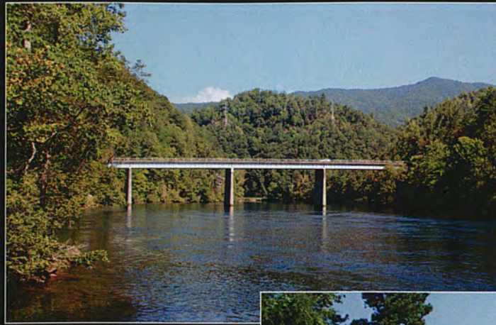
A. Bridge, View West Elevation from Project Site
