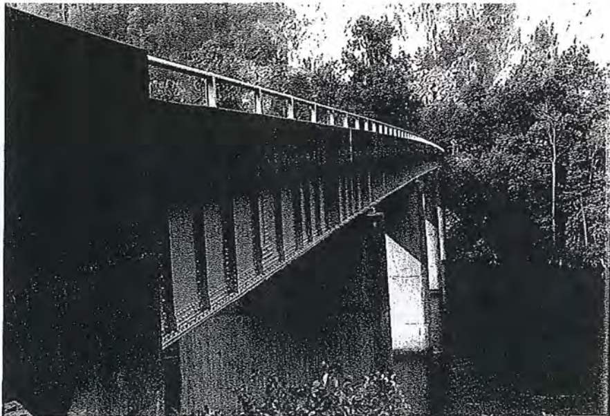
207:15. Upstream (east) elevation.
