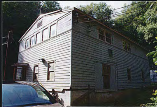
E. West Elevation, View Southeast
