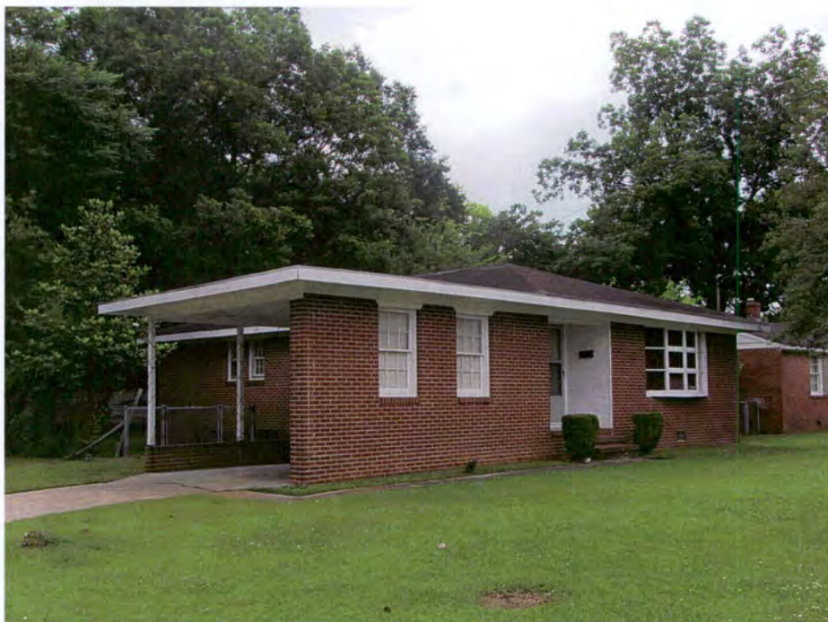
Figure 74. 104 South Alabama Avenue, Goldsboro, Looking Southeast (TRC June 2012).
