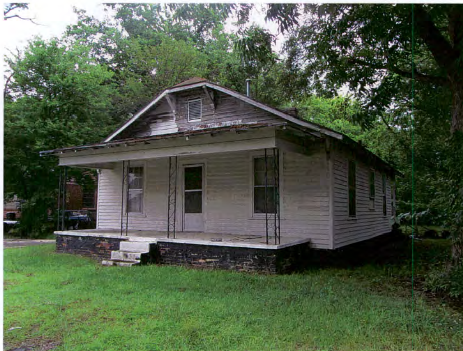
Figure 73. 108 South Alabama Avenue, Goldsboro, Looking Northeast (TRC June 2012).
