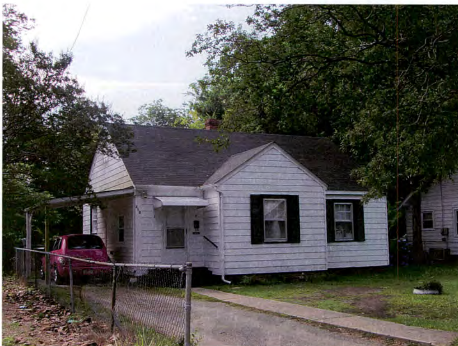
Figure 18. 312 North Carolina Street, Goldsboro, Looking Southeast (TRC June 2012).
