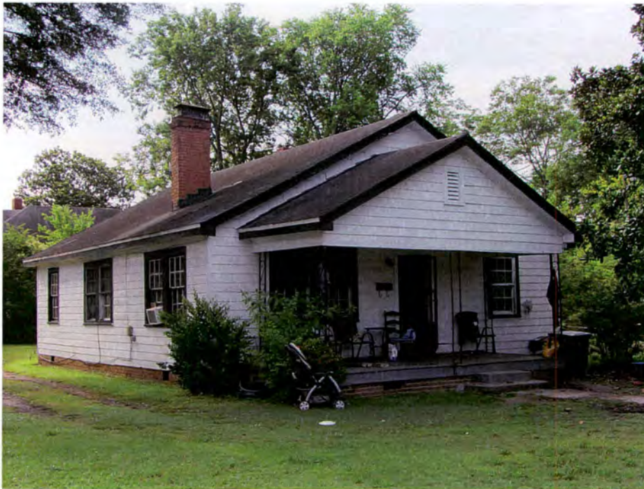
Figure 17. 316 North Carolina Street, Goldsboro, Looking Southeast (TRC June 2012).
