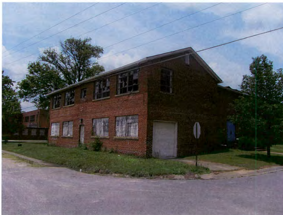
Figure 90. 400 West Elm Street, Goldsboro, Looking Northwest (TRC June 2012).
