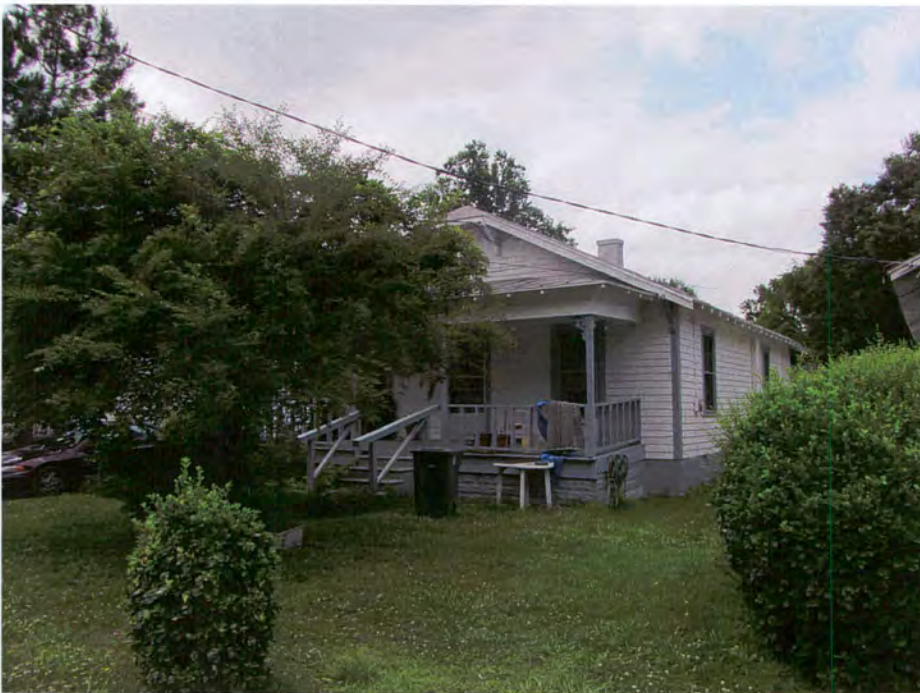
Figure 60. 702 West Walnut Street, Goldsboro, Looking South (TRC June 2012).
