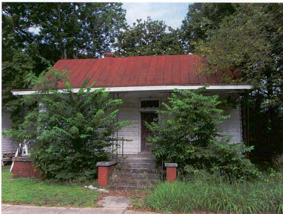
Figure 26. 313 North Carolina Street, Goldsboro, Looking West (TRC June 2012).
