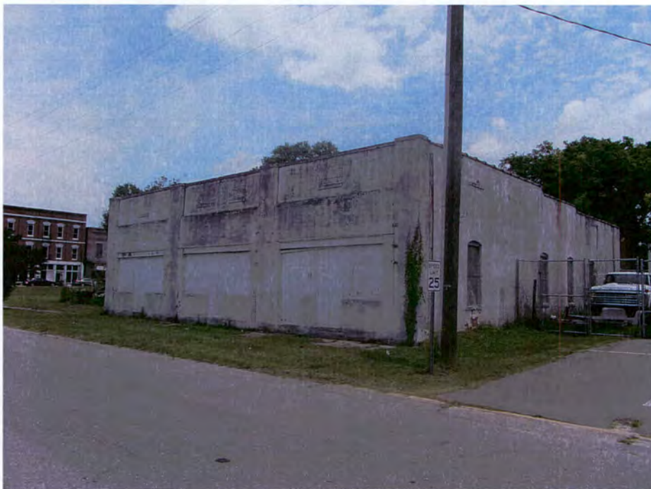
Figure 34. 110-120 South Carolina Street, Goldsboro, Looking Northeast (TRC June 2012).
