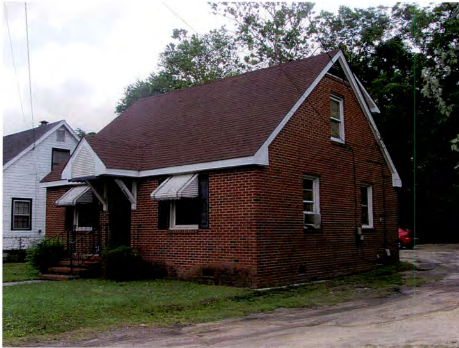
Figure 75. 104 North Alabama Avenue, Goldsboro, Looking Northeast (TRC June 2012).
