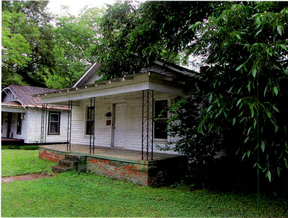
Figure 71. 120 South Alabama Avenue, Goldsboro, Looking Northeast (TRC June 2012).
