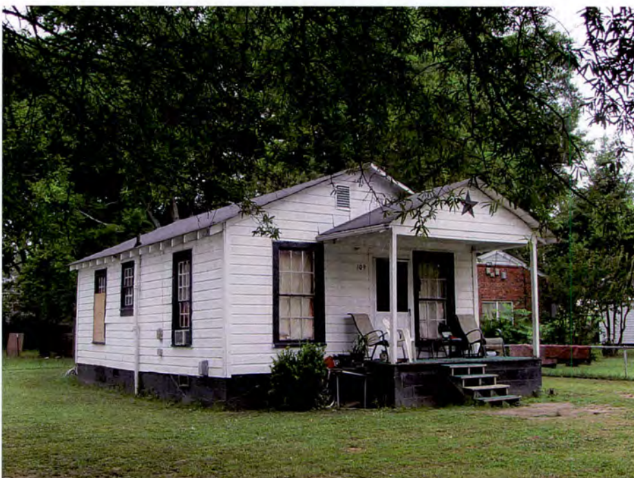
Figure 82. 109 South Alabama Avenue, Goldsboro, Looking Northwest (TRC June 2012).
