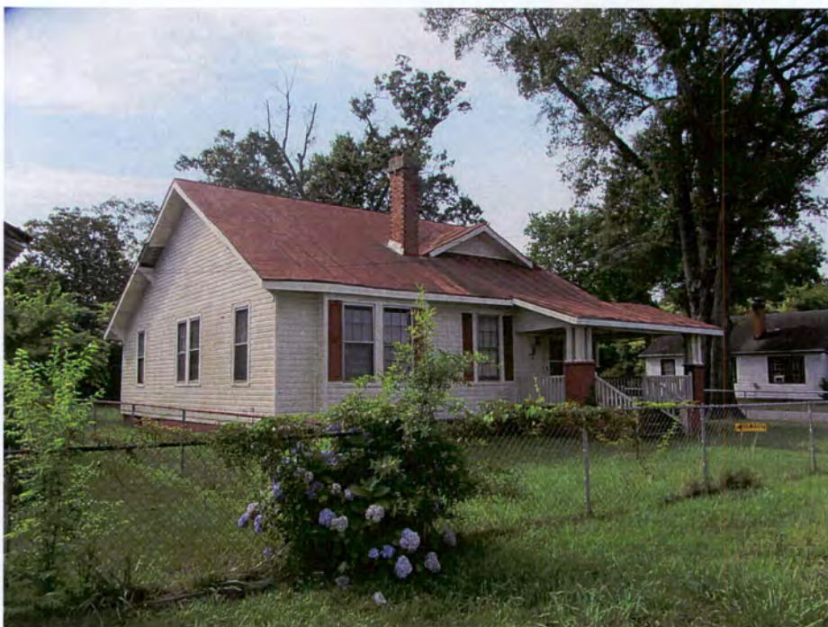
Figure 16. 400 North Carolina Street, Goldsboro, Looking Southeast (TRC June 2012).
