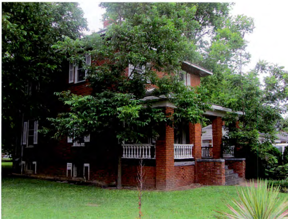
Figure 81. 115 South Alabama Avenue, Goldsboro, Looking Northwest (TRC June 2012).
