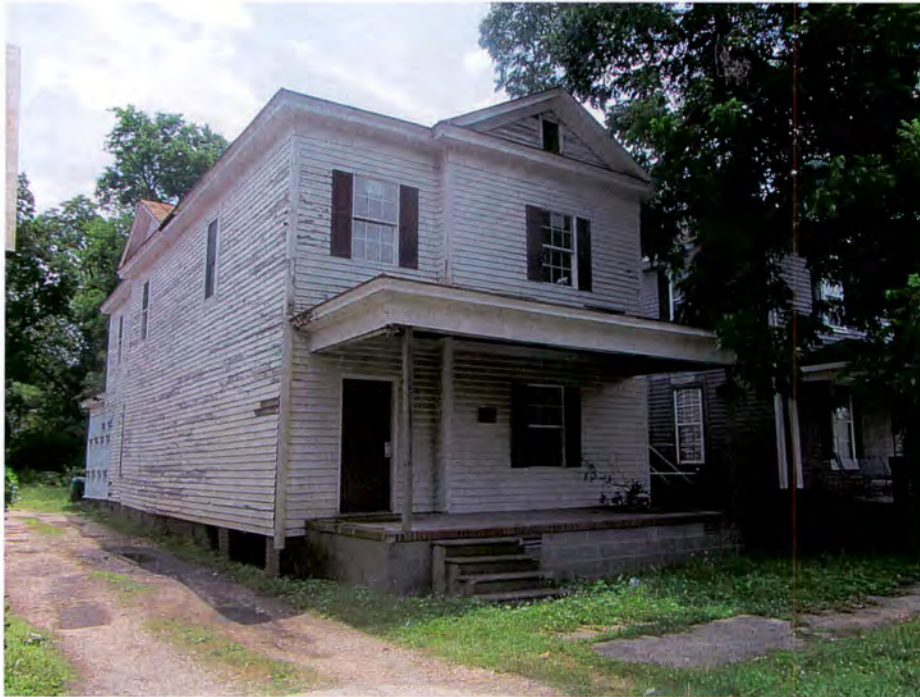
Figure 29. 206 North Carolina Street, Goldsboro, Looking Southeast (TRC June 2012).
