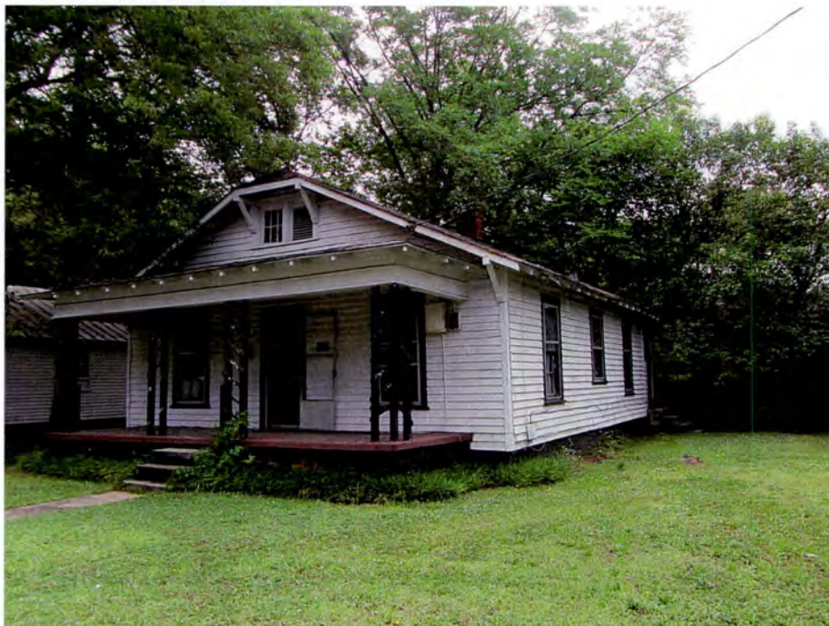
Figure 72. 118 South Alabama Avenue, Goldsboro, Looking Northeast (TRC June 2012).
