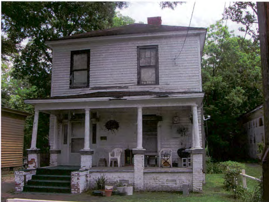
Figure 36. 204 South Carolina Street, Goldsboro, Looking East (TRC June 2012).
