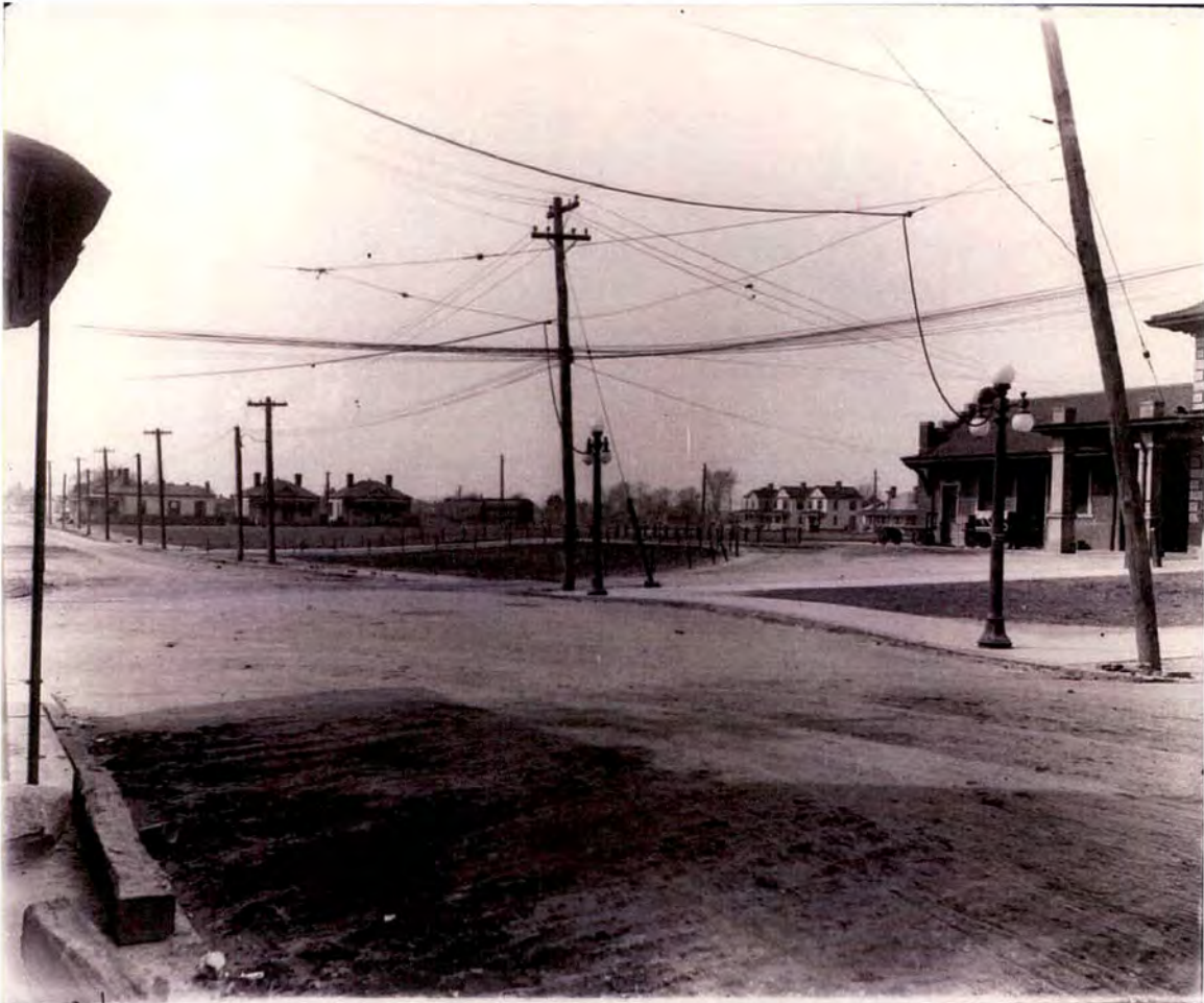
Figure 8. West End of West Walnut Street at Goldsboro Union Station, ca. 1915. Houses Immediately to the Left of the Railroad Station are on South Georgia Street (Still Extant), and to the Left of These are Two Houses (Still Extant) on West Chestnut Street. (Source: Wayne County Public Library, www.wcpl.org/genealogy/photographcategories.asp )
