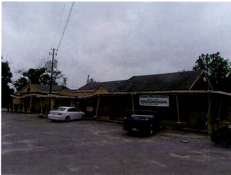
Figure 85. 706 South George Street, Goldsboro, Looking Northeast (TRC June 2012).
