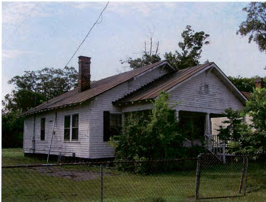
Figure 15. 402 North Carolina Street, Goldsboro, Looking Southeast (TRC June 2012).
