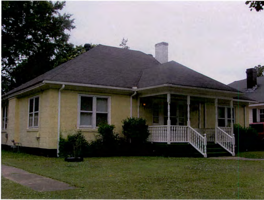
Figure 83. 105 South Alabama Avenue, Goldsboro, Looking Northwest (TRC June 2012).
