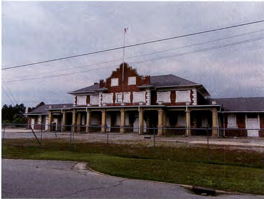
Figure 10. Goldsboro Union Station following NCDOT Stabilization, East Façade, Facing West (TRC 2012).
