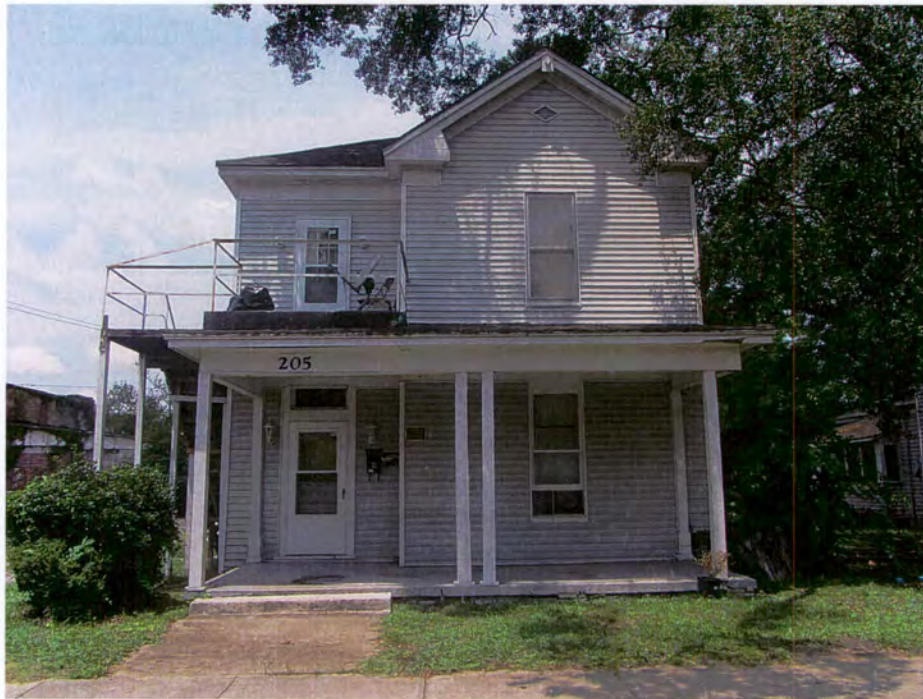
Figure 33. 205 North Carolina Street, Goldsboro, Looking West (TRC June 2012).
