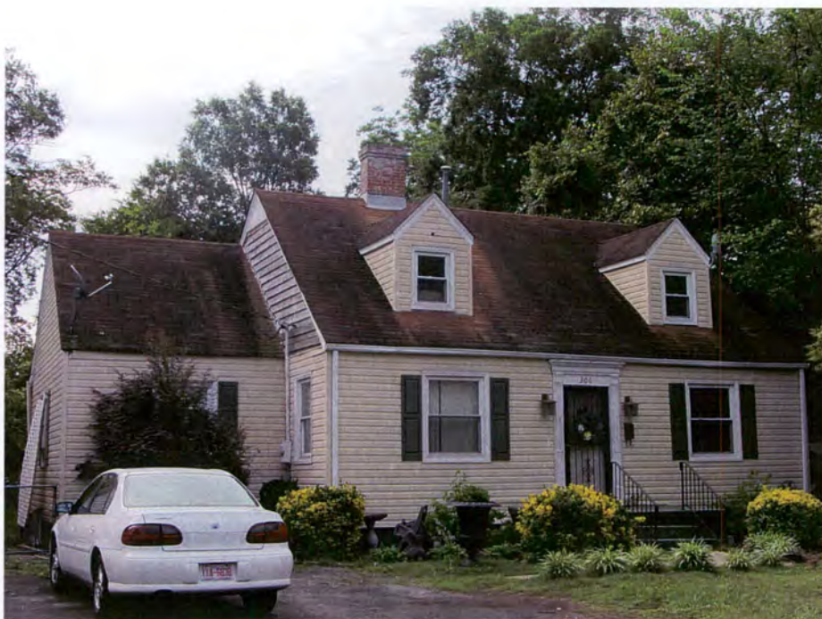
Figure 20. 306 North Carolina Street, Goldsboro, Looking Southeast (TRC June 2012).
