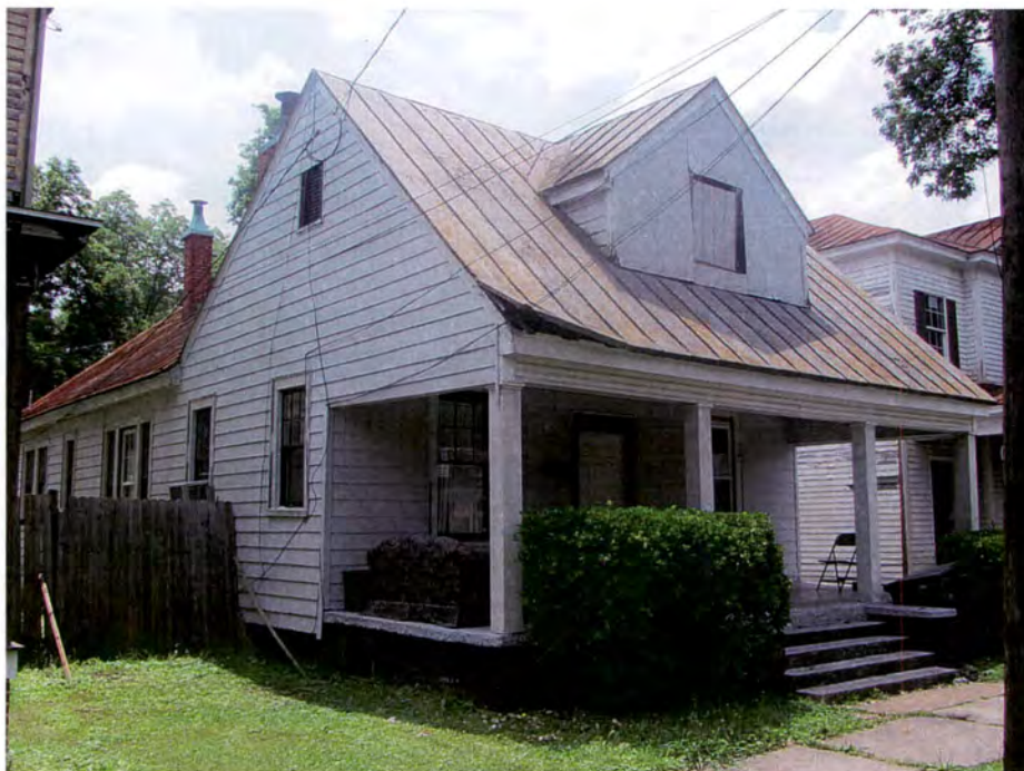
Figure 28. 210 North Carolina Street, Goldsboro, Looking Southeast (TRC June 2012).
