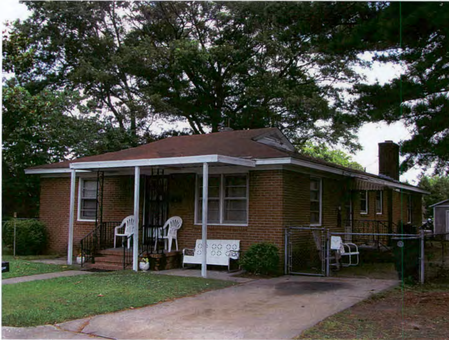
Figure 59. 707 West Walnut Street, Goldsboro, Looking Northwest (TRC June 2012).
