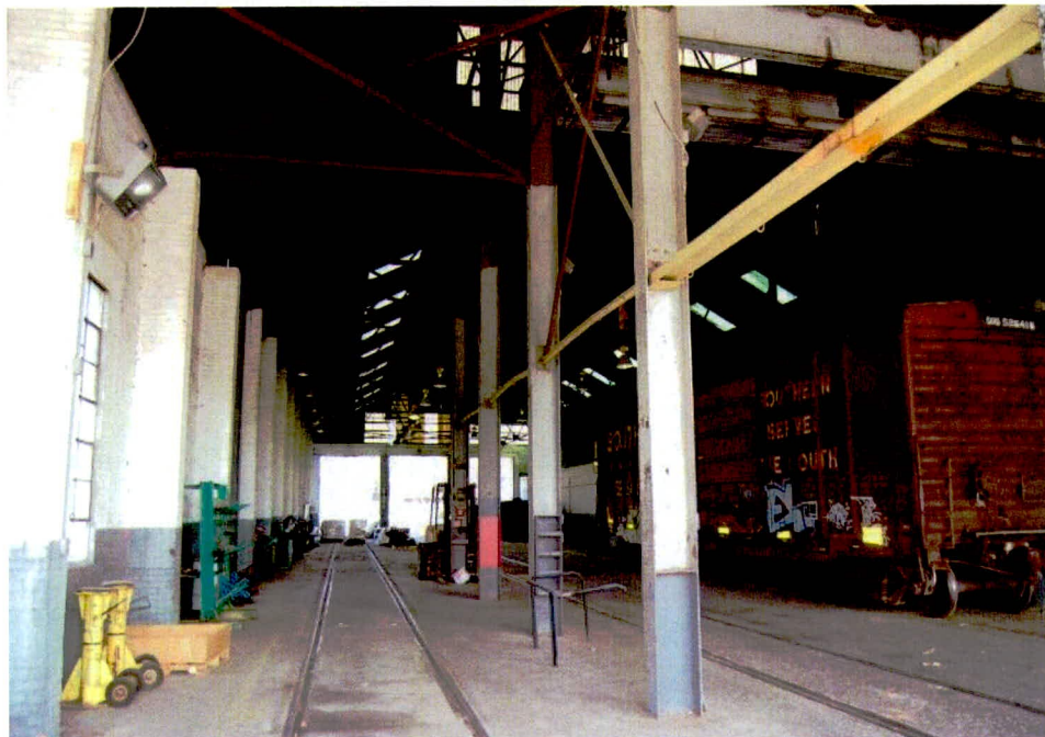
Plate 4. Pinoca Yard, Car Shop Interior, Looking North.
