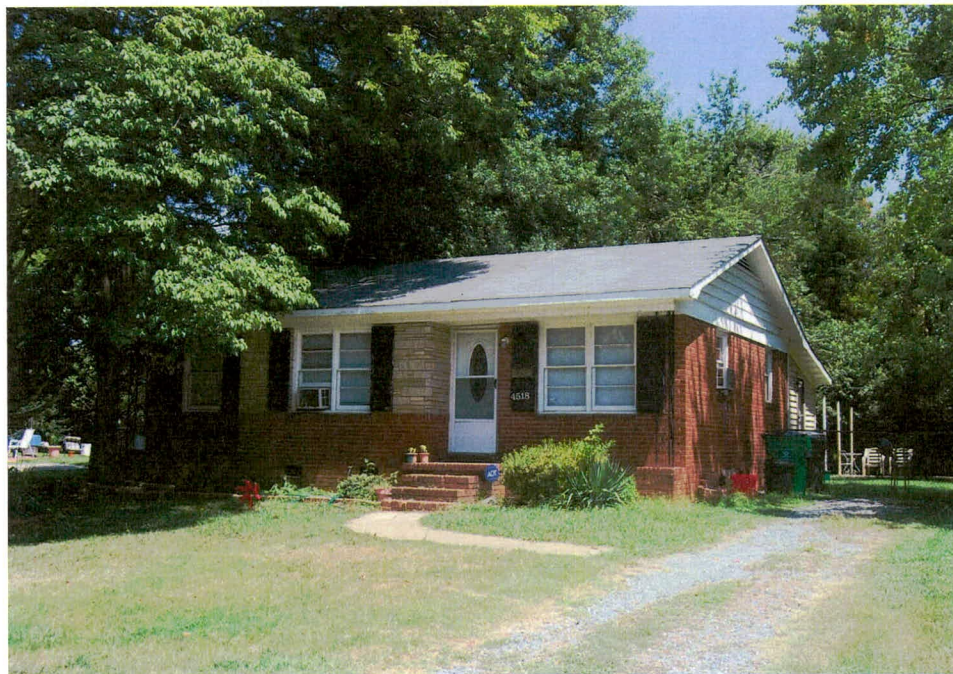
Plate 17. Brookfield, 4518 Ridgeley Drive (Within APE), Looking North.
