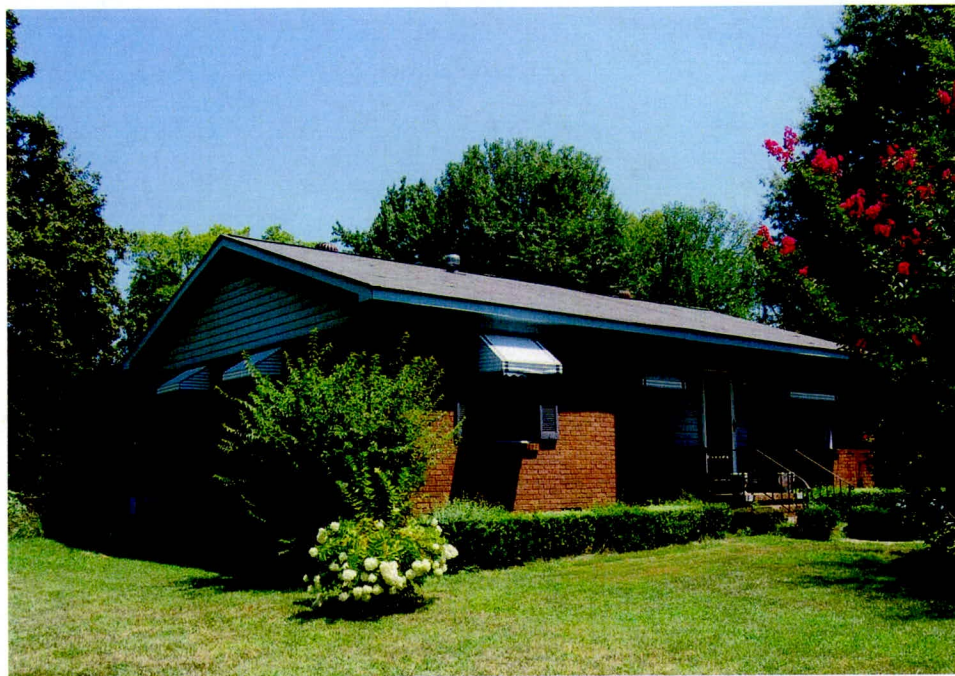
Plate 18. Brookfield, 4522 Ridgeley Drive (Within APE), Looking North.
