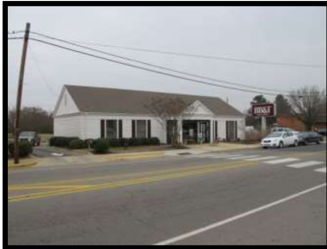
Figure 28: B – View of BB&T Bank Looking Southeast.
