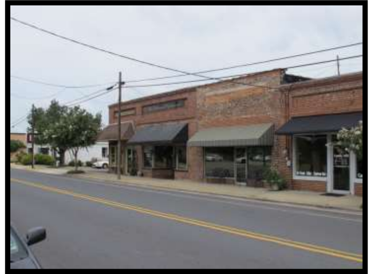
065 to 069 – 116 to 122 Main St. – 1920 – LE0269 Commercial Buildings
