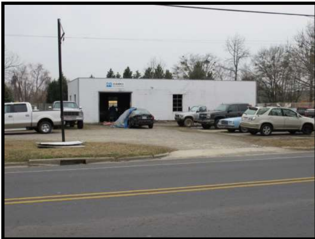
Figure 40: C – View of Garage Looking Northwest.
