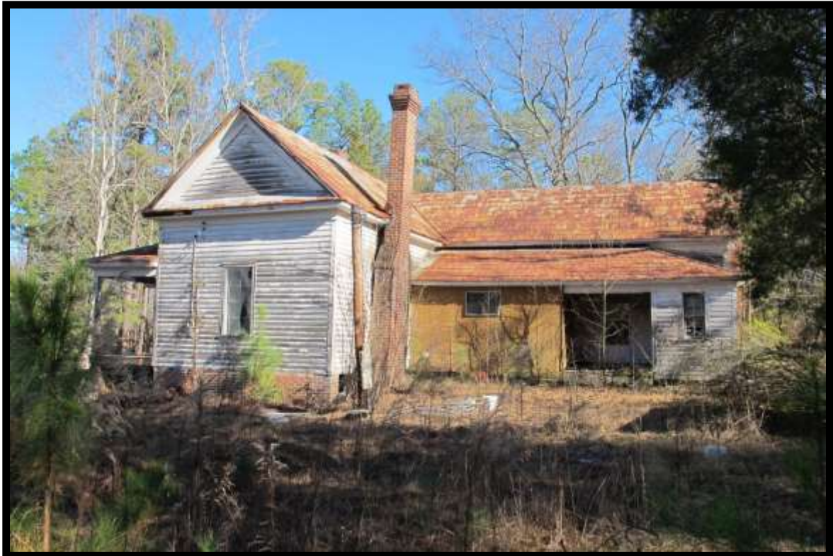
Figure 7: No. 44 View of Sloan House Looking East.
