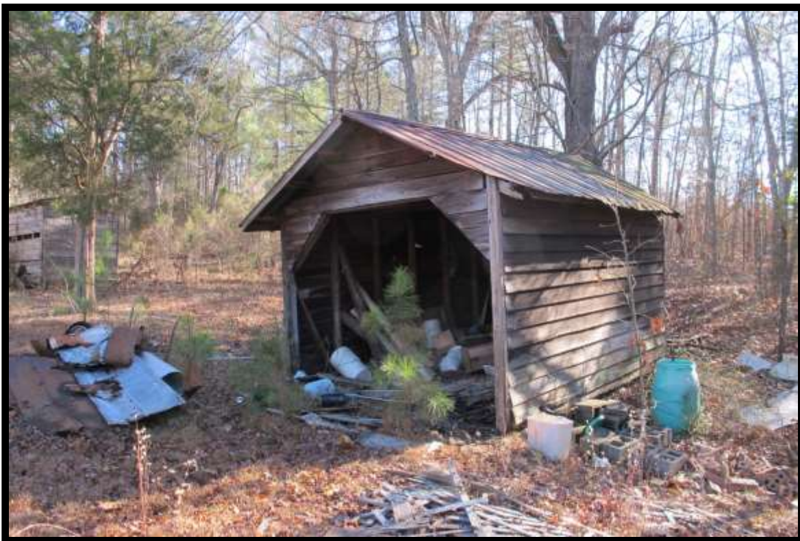
Figure 14: No. 44 View of Shed Looking Southeast.
