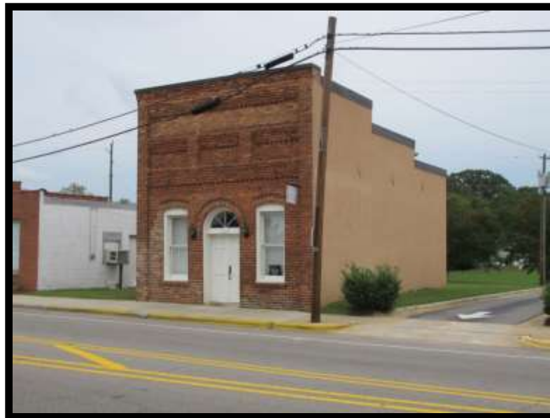
Figure 27: No. 65 View of Bank of Broadway Looking Northeast.
