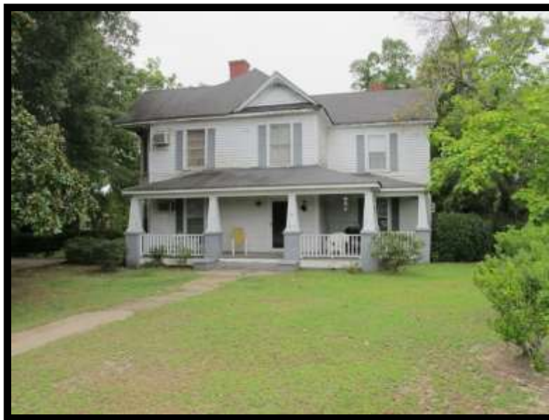
Figure 41: No. 80 View of Preston Morris House Looking Southwest.
