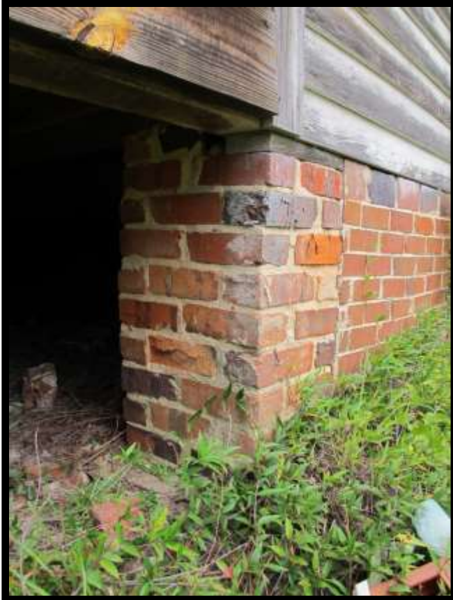
Figure 10: No. 44 Detail of Brick Piers and Brick Infill.
