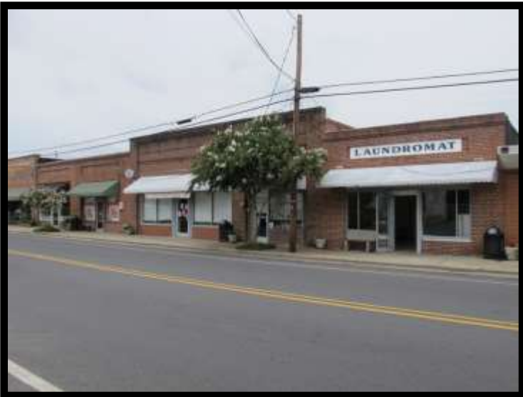
069 to 073 – 122 to 128 Main St. – 1920 – LE0269 Commercial Buildings
