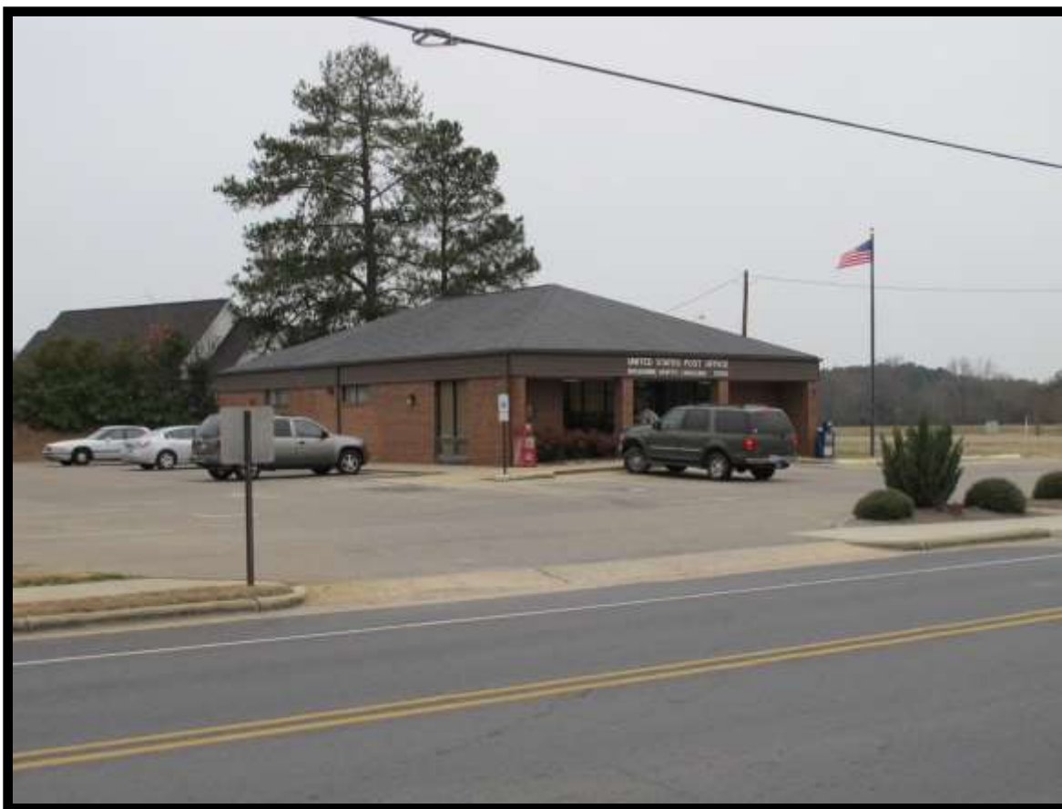
Figure 36: A – View of the U.S. Post Office Looking Northwest.
