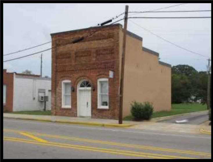
065 – 104 Main St. – 1920 – LE0267 Bank of Broadway
