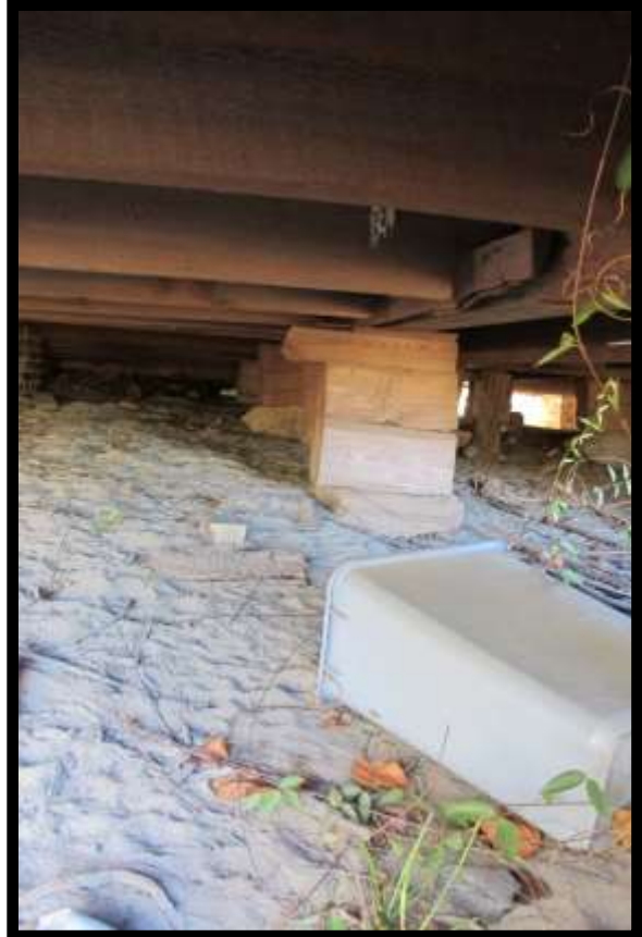
Figure 11: No. 44 Detail of Wooden Block Piers.
