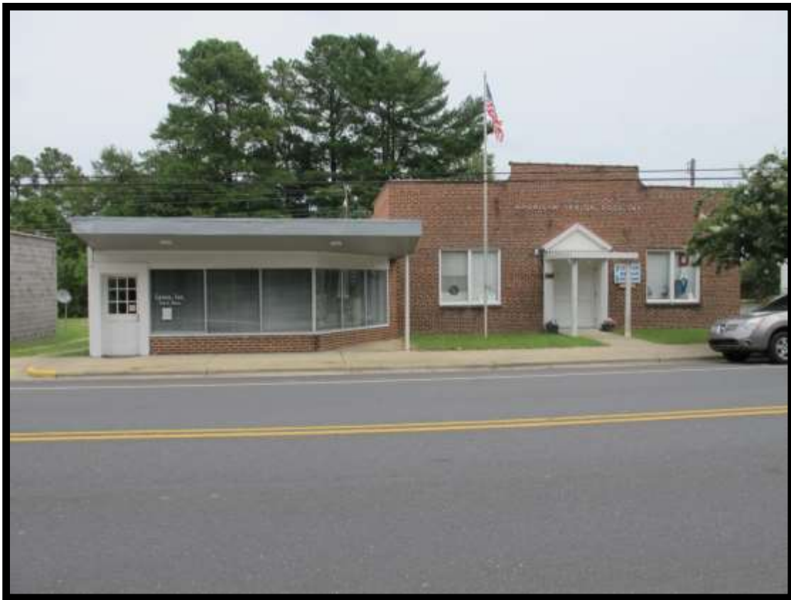
Figure 35: Nos. 83 and 84 View of the Broadway Appliance Company (left) and American Legion Post (right) Looking East.
