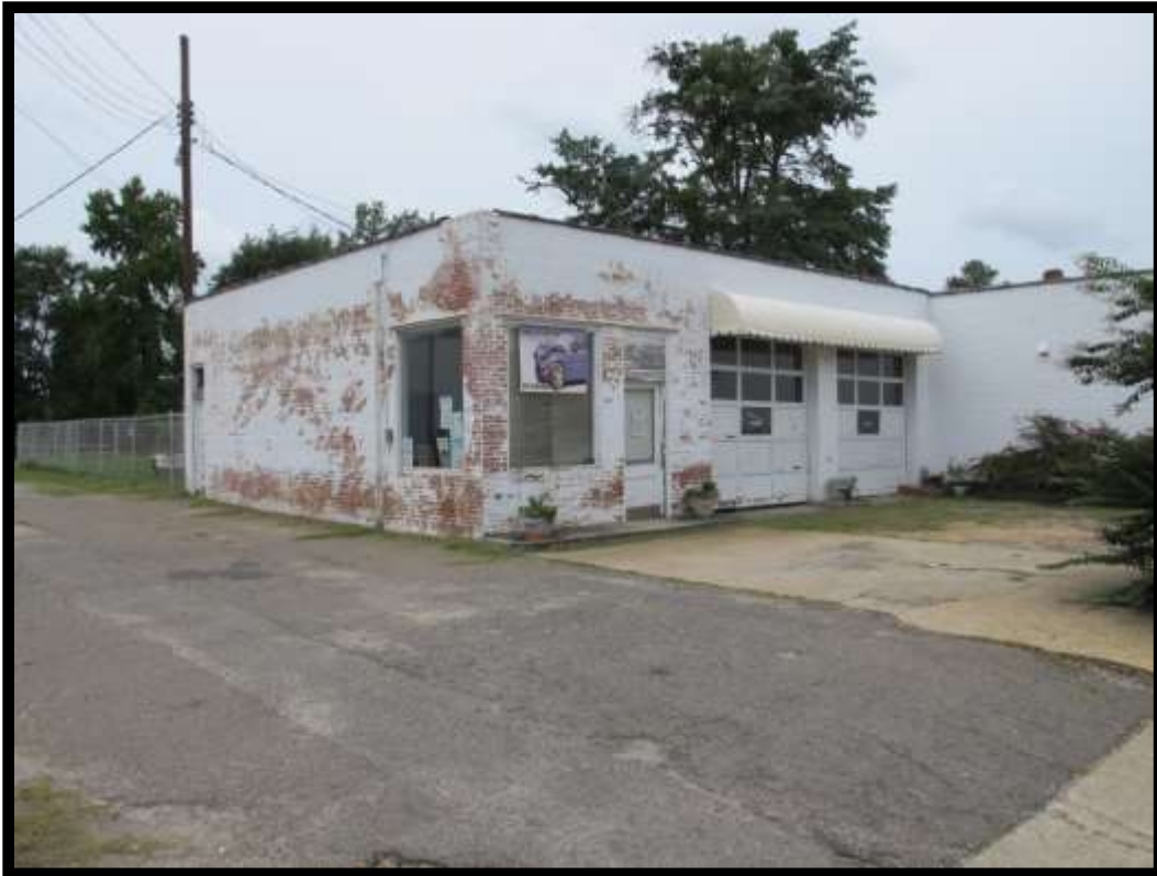
Figure 39: No. 79 View of Garage/Service Station Looking Northwest.
