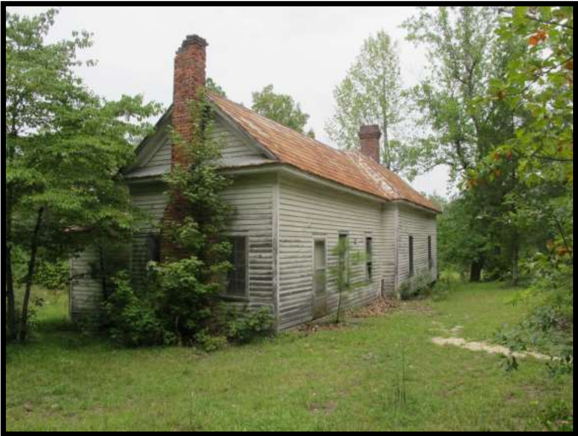
Figure 8: No. 44 View of Sloan House Looking Northwest.
