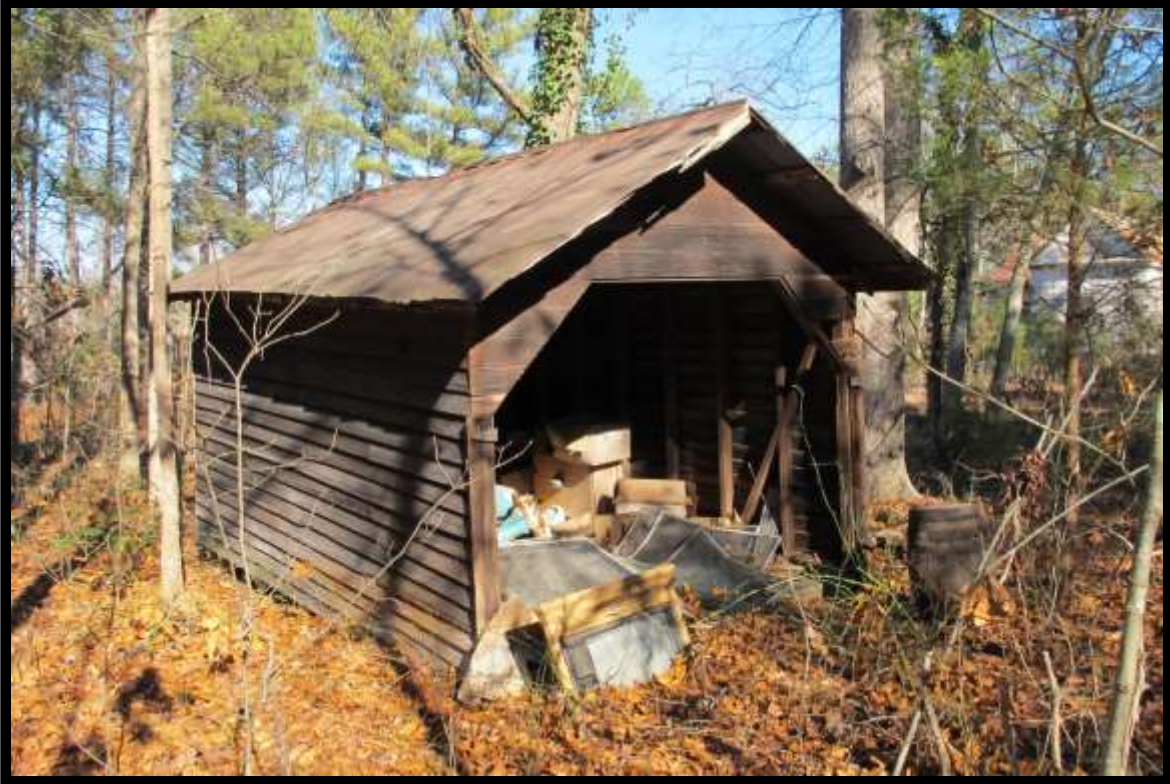
Figure 15: No. 44 View of Shed Looking Northeast.
