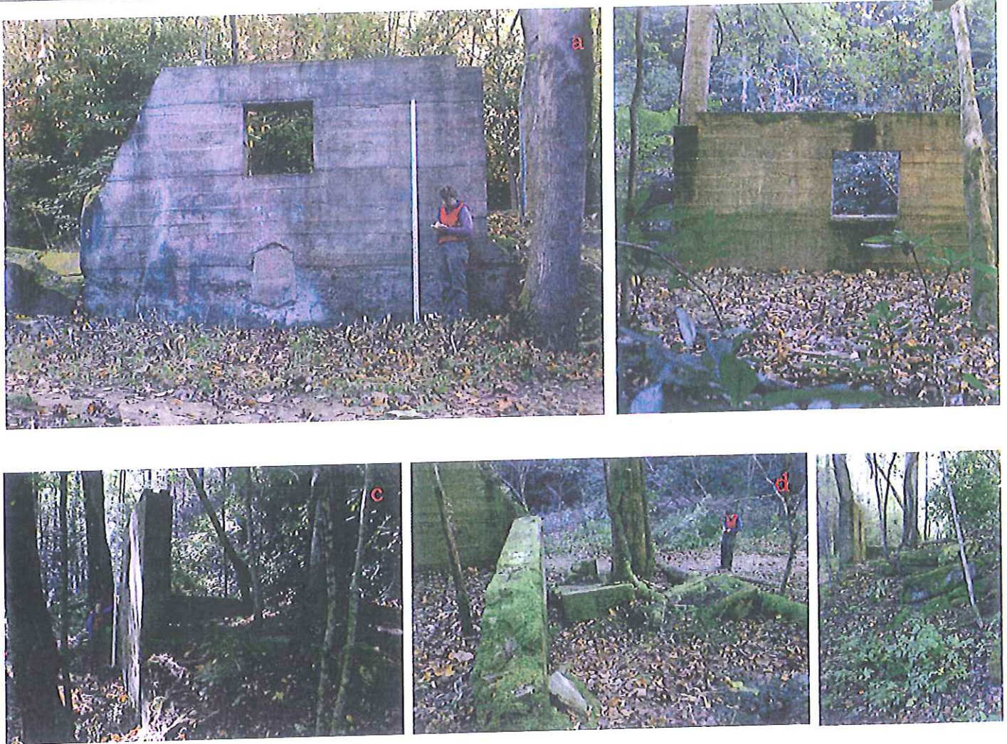
Figure 11a-e. Overview photographs of Power House No. 1 at MC 207: a) south wall, view to northwest; b) south and west walls, view to west; c) south and west walls, view to west; d) west wall remnant and rubble, view to the south; e) concrete rubble
