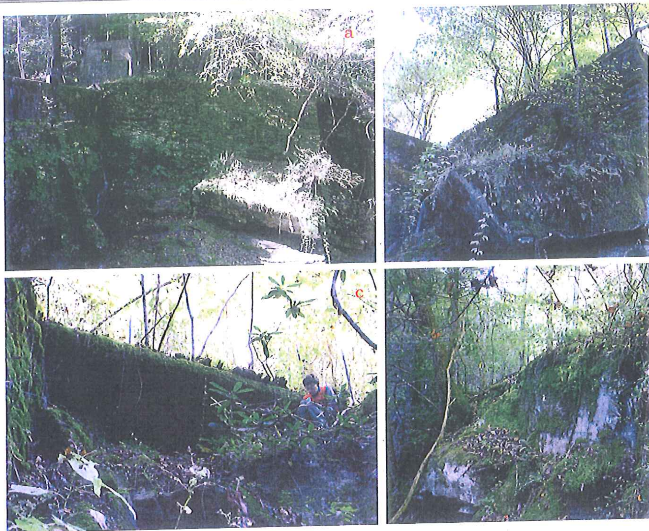
Figure 13a-d. Overview photographs of various features at MC 207: a) stone retaining wall/artificial platform, view to north; b) concrete retaining wall, view to west; c) log platform, view to northwest; d) concrete retaining wall, view to west.
