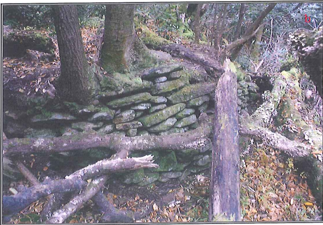
Figure 25. Photographs of stone cribbing at MC 208: a) view to southeast; b) view to southwest.
