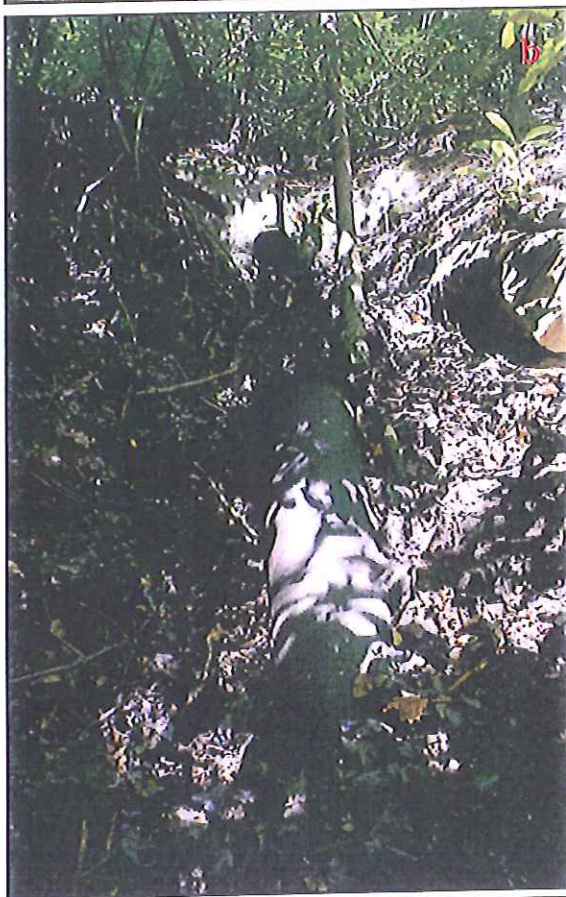
Figure 12. Concrete retaining wall (a) and cast iron pipe (b) on slope above Power House No. 1.
