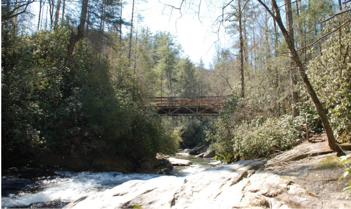
Photo 1. Bullpen Bridge, north side. (looking south downstream)
