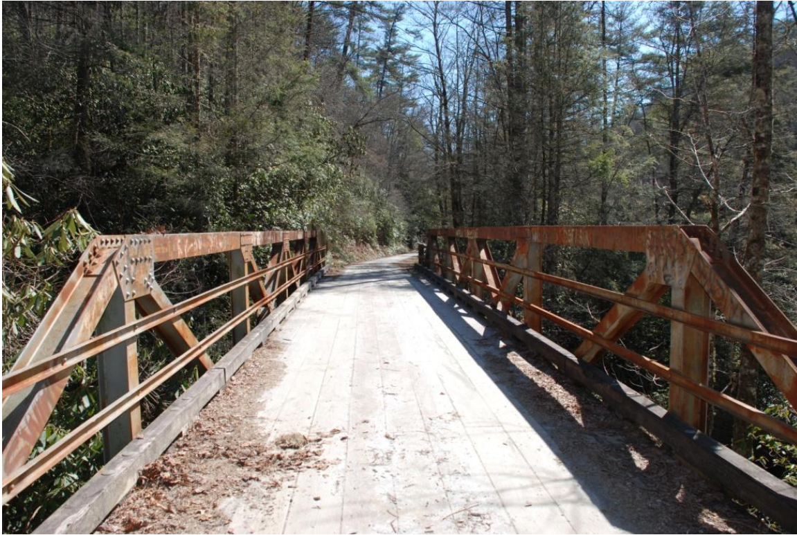
Photo 4. View looking east across the bridge.
