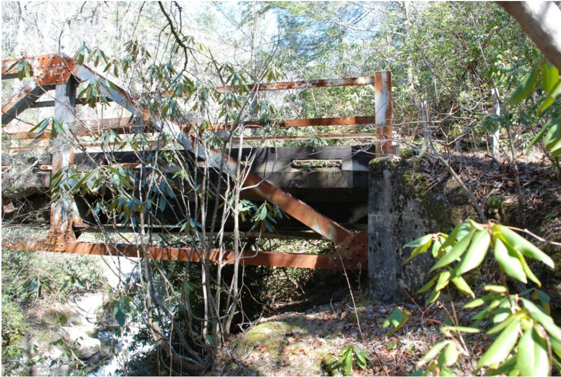
Photo 9. Eastern end looking north at the south side of the bridge.
