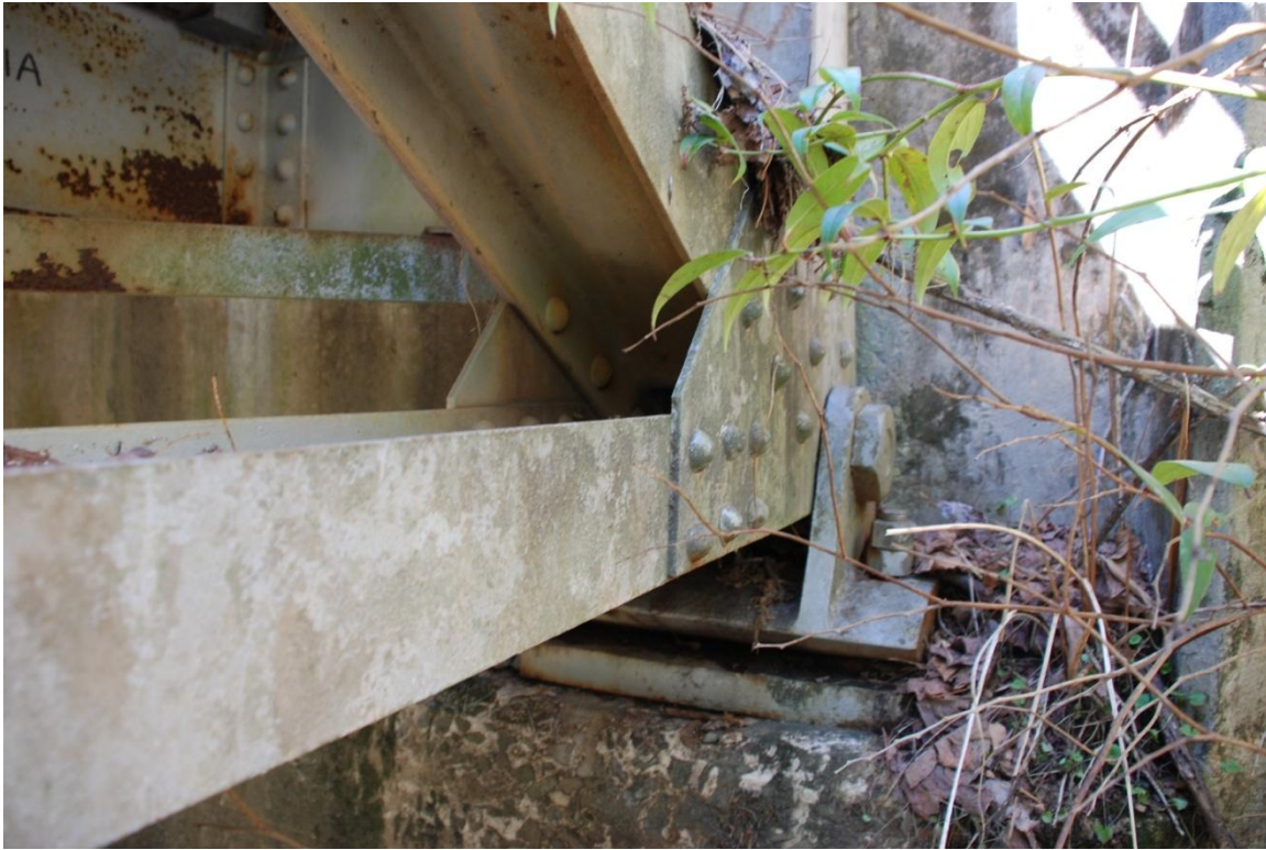
Photo 16. Rocker connection at base, NL1.
