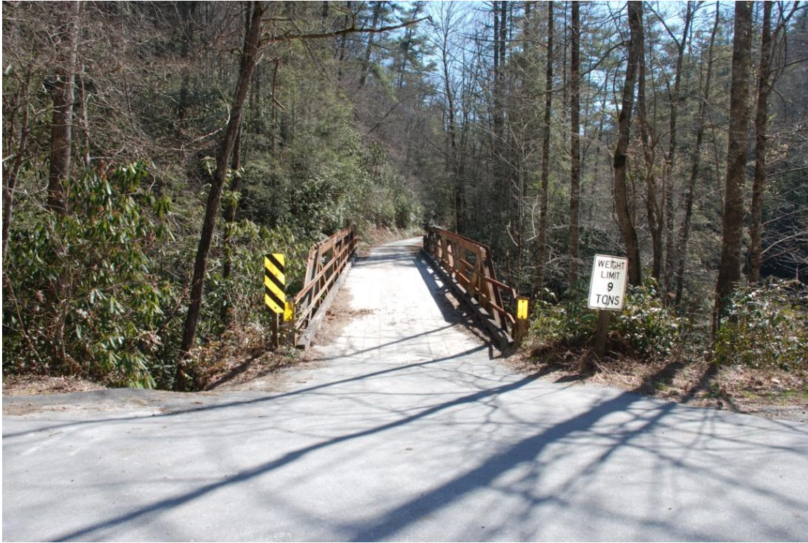
Photo 3. View looking east across the bridge.
