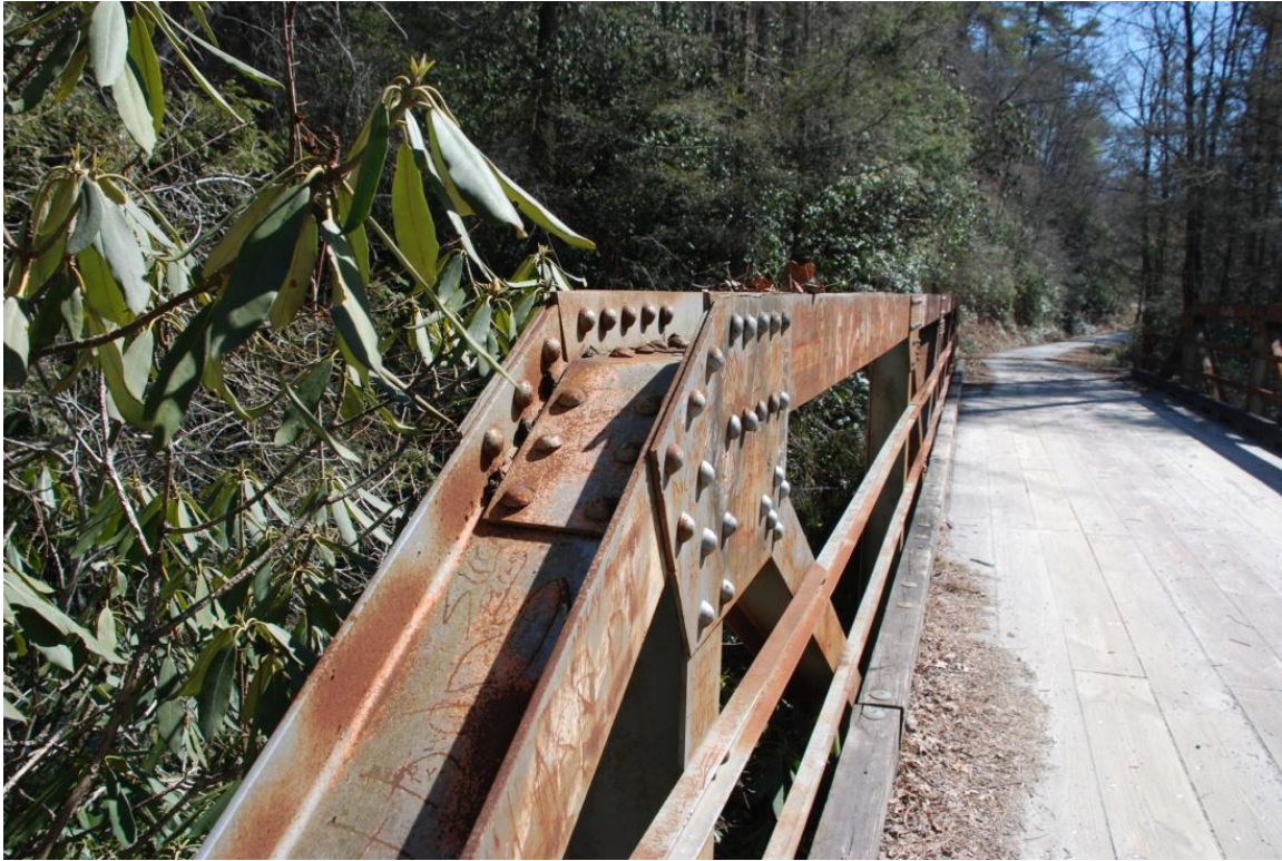
Photo 5. Detail at top rail at connection NU1.
