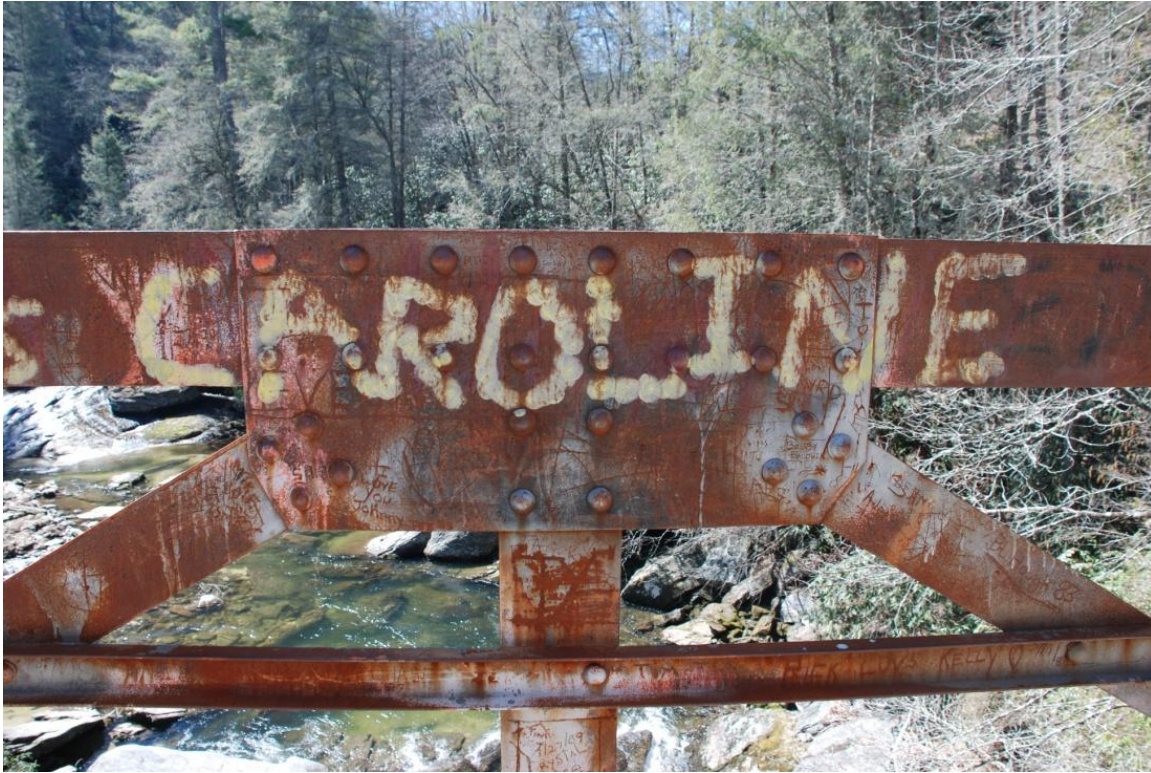
Photo 7. Detail at top rail, connection SU3.
