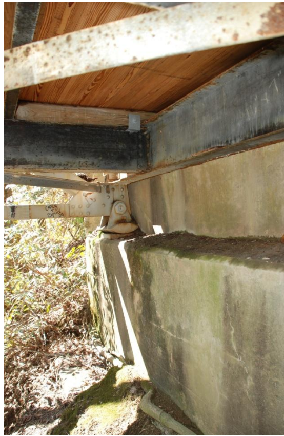
Photo 18. Base connection, SL1.
