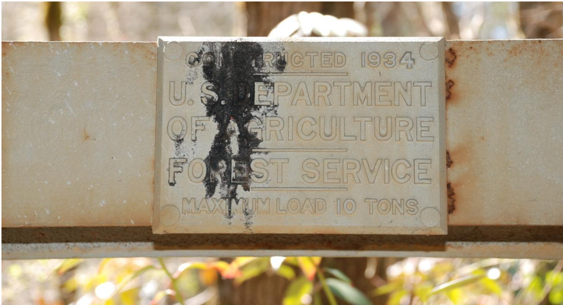
Photo 19. Plaque on lower cord, south side between connection SL1 and SL2.
