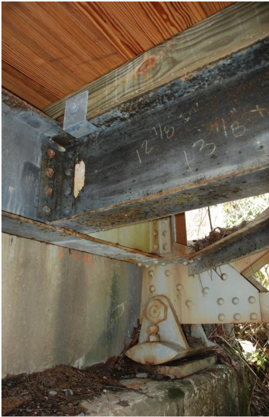
Photo 17. Base connection, NL1.
