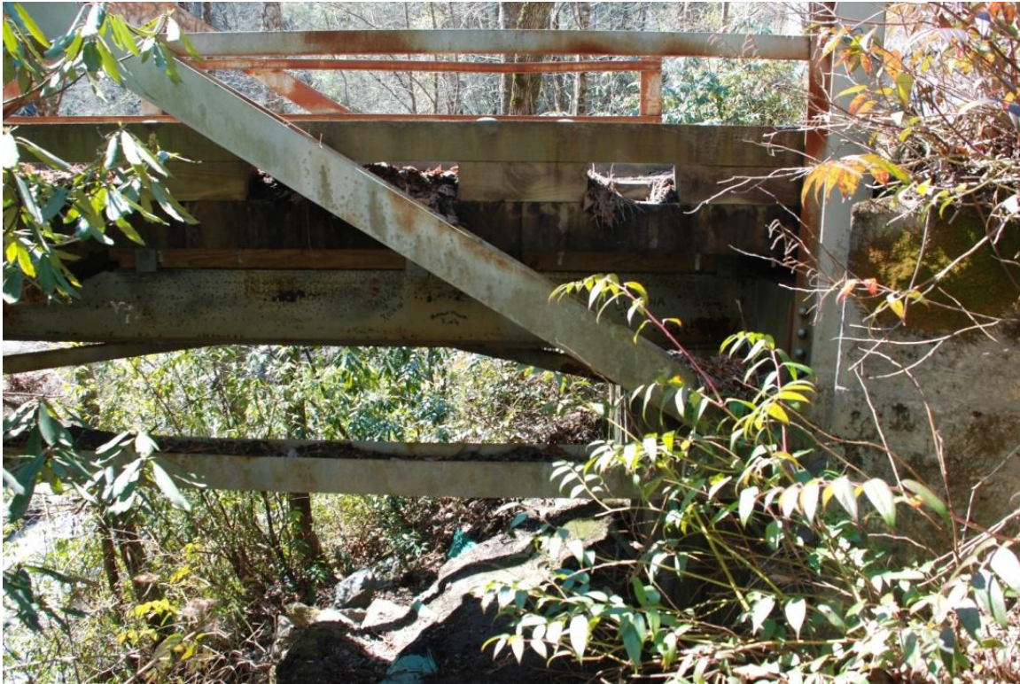
Photo 14. Western end of the bridge, looking south at the north side.
