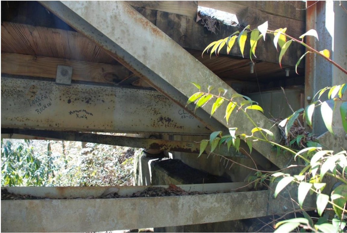
Photo 15. Western end of the bridge, looking south at the north side.
