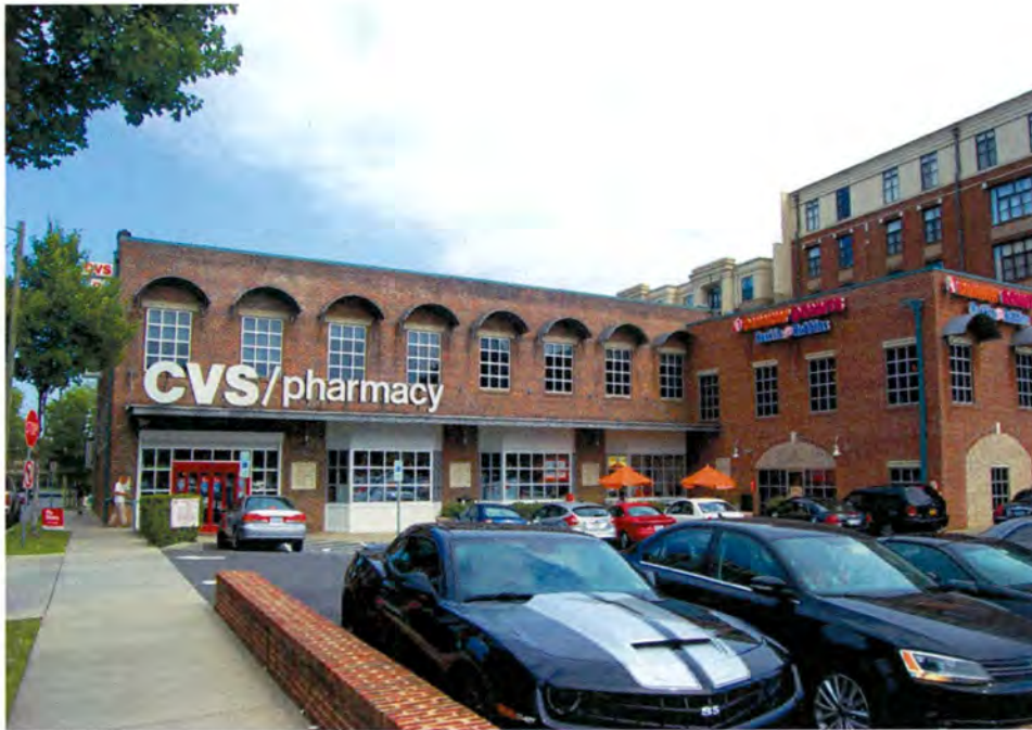
Plate 9. Warehouse. Looking West from North Graham Street.
