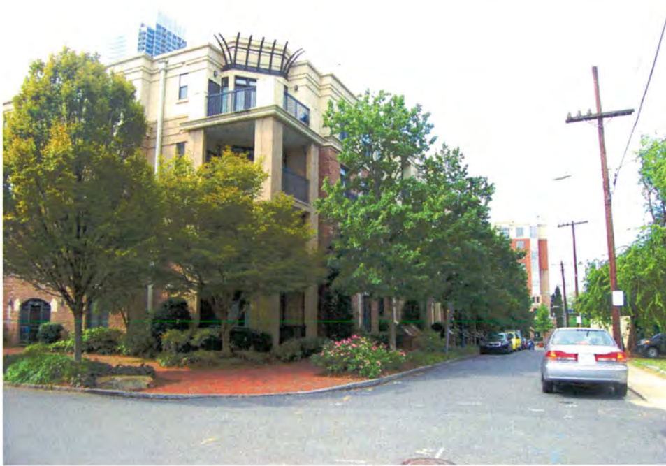
Plate 3. Fourth Ward Historic District. Modern Apartment Building at Southeast Corner of West Seventh and North Smith Streets, Looking South.
