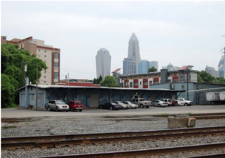
Plate 12. Seaboard Street Historic District, Interstate Mills Warehouse, Looking Southeast Towards Downtown.
