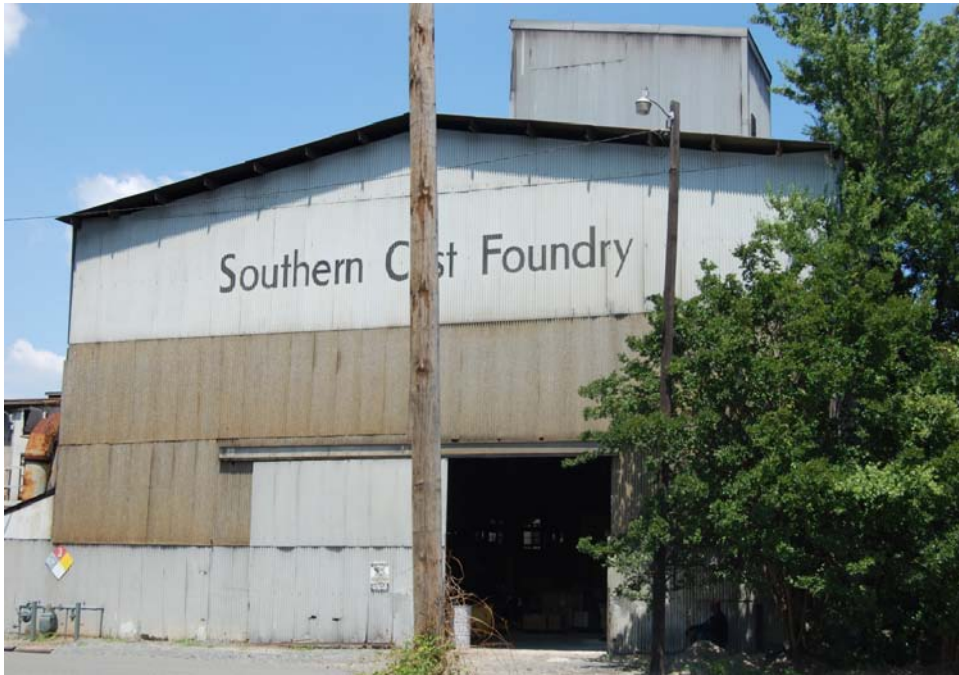
Plate 20. Soule Steel and Iron Works, 1940s Foundry, Looking Northwest.
