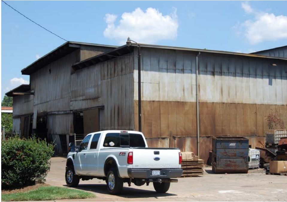
Plate 19. Soule Steel and Iron Works, 1940s Iron Shed, Looking North.
