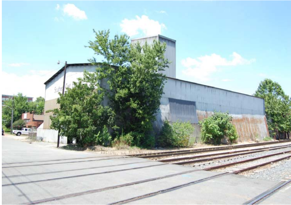
Plate 21. Soule Steel and Iron Works, 1940s Foundry, Looking West Across Rail Line.
