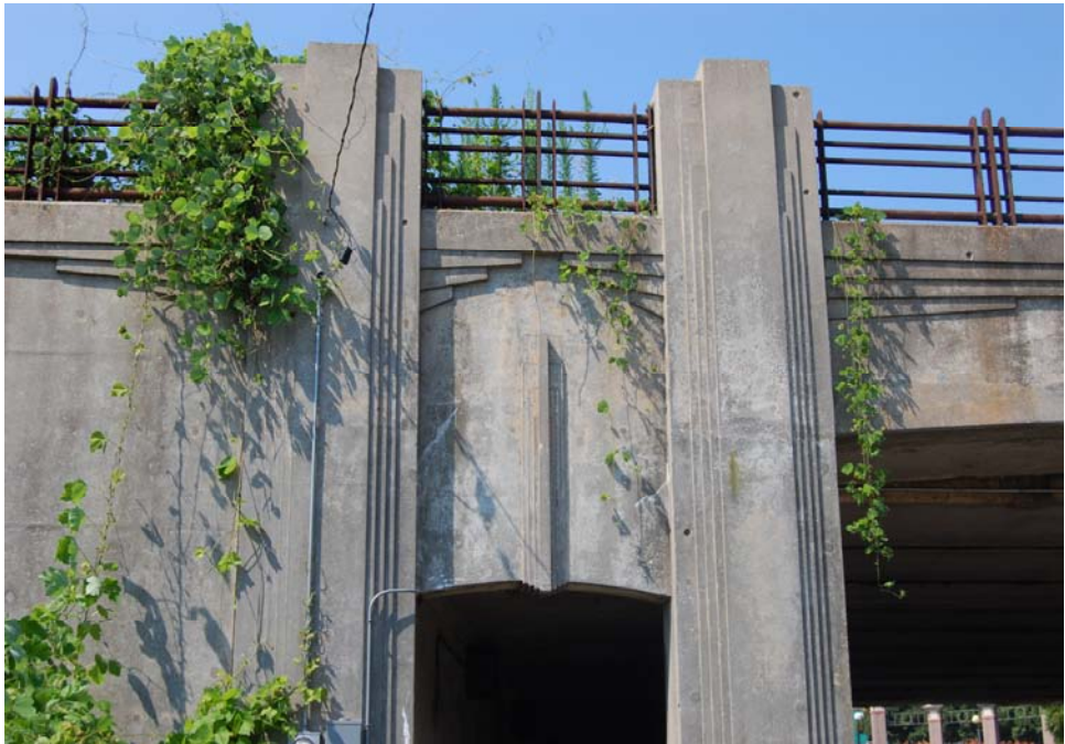
Plate 23. Seaboard Air Line Railway Bridge, Detail, Looking South.
