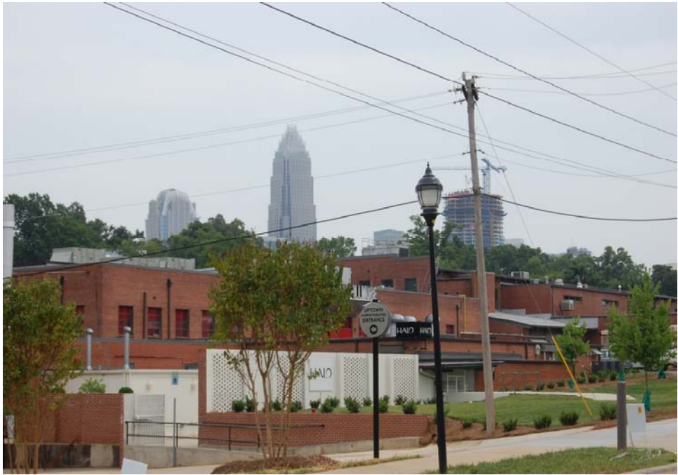
Plate 2. Southern Asbestos Company Mills, Looking South Along Hamilton Street.
