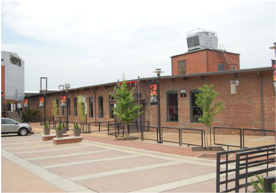
Plate 1. Southern Asbestos Company Mills, Looking Northwest.
