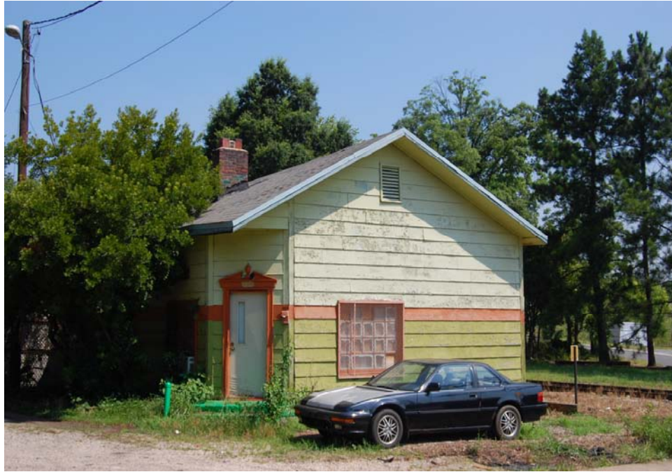
No. 12 Warehouse, 958 North Davidson Street, Looking Northwest.
