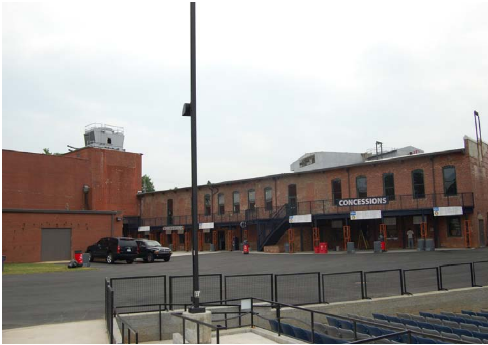
Plate 3. Southern Asbestos Company Mills, Looking Southwest.
