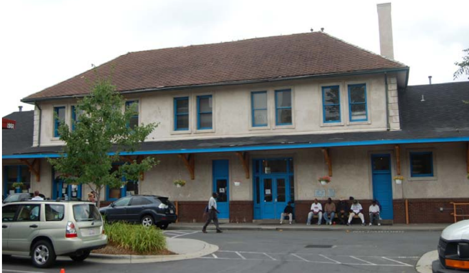
Plate 25. Seaboard Air Line Railway Passenger Station, South Elevation, Looking Northeast.
