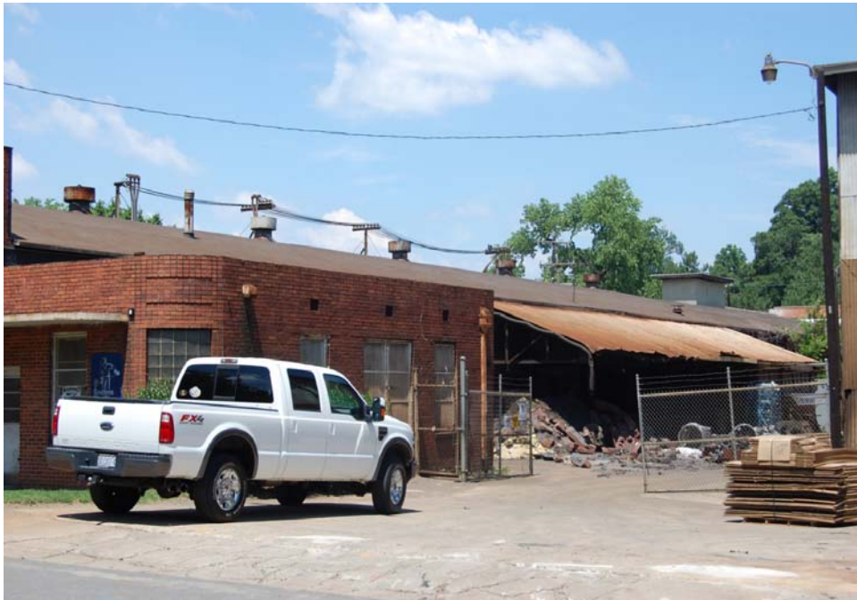
Plate 18. Soule Steel and Iron Works, Office and Original Foundry/Steel Fabrication Plant, Looking West.
