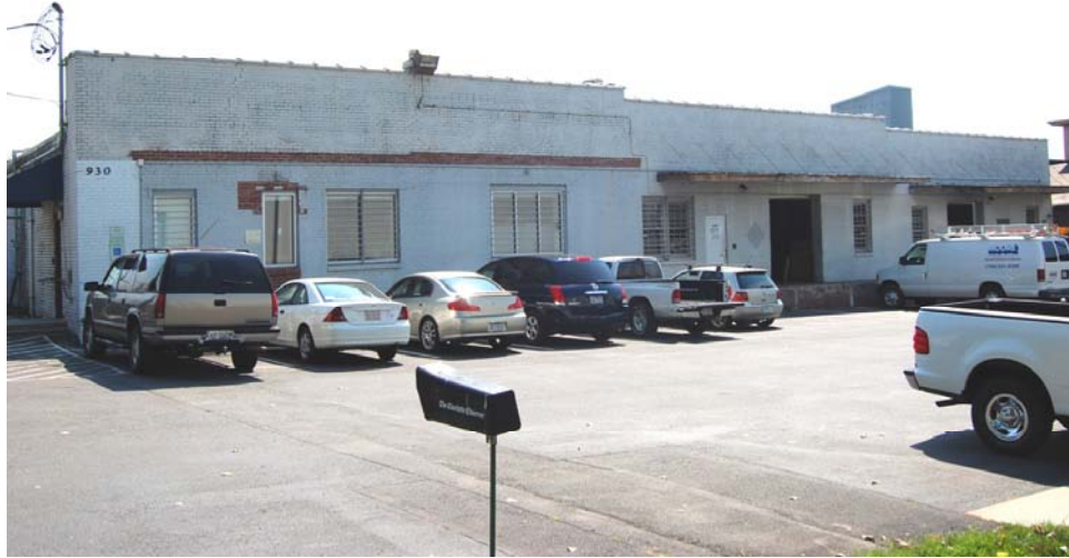
No. 4 Warehouse, 930 North Poplar Street, Looking North.
