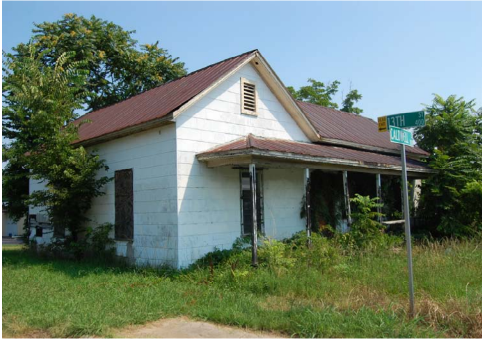
No. 10 House, 1001 North Caldwell Street, Looking Northwest.
