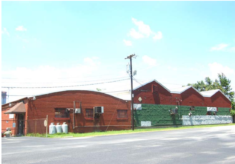
No. 6 Warehouse, 1001 North Church Street, Looking Southwest.
