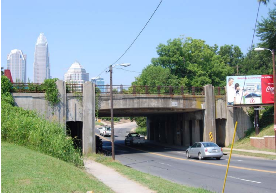
Plate 22. Seaboard Air Line Railway Bridge, Looking South.
