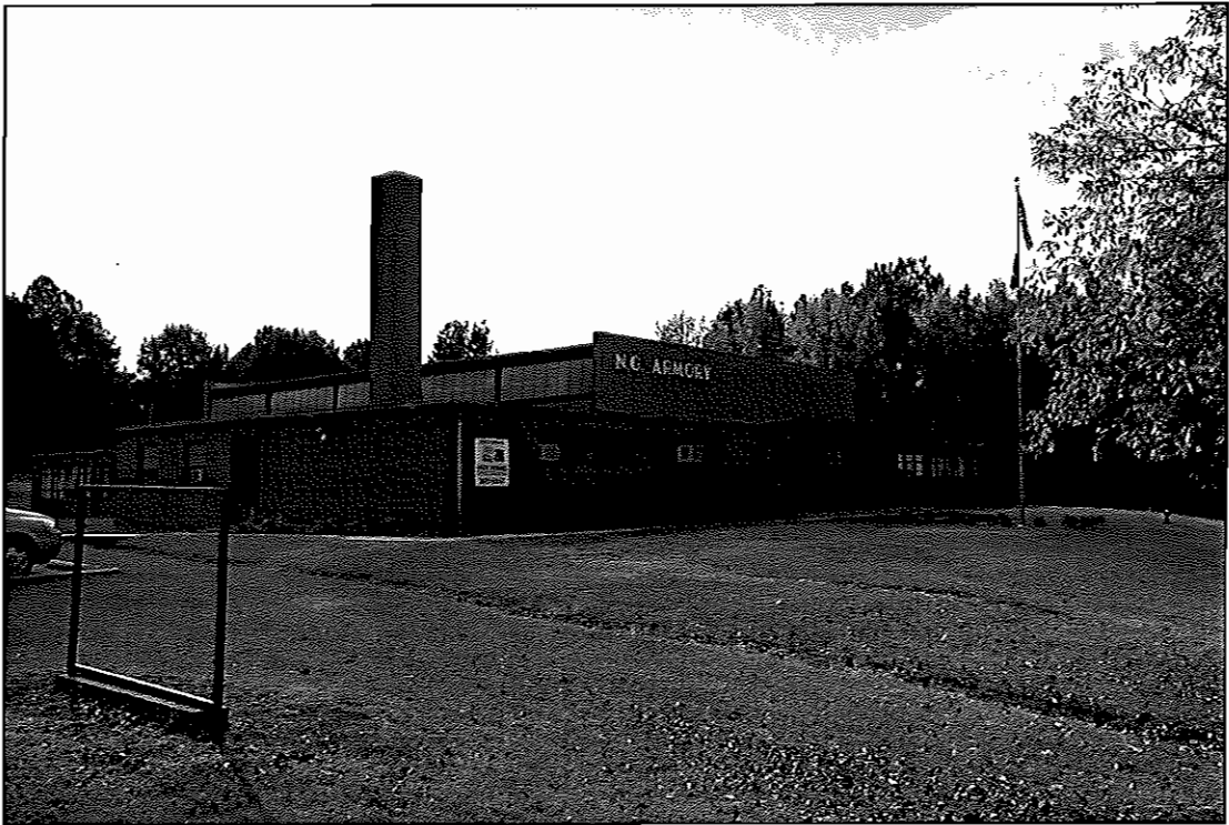
PLATE 18: Roxboro National Guard Armory
