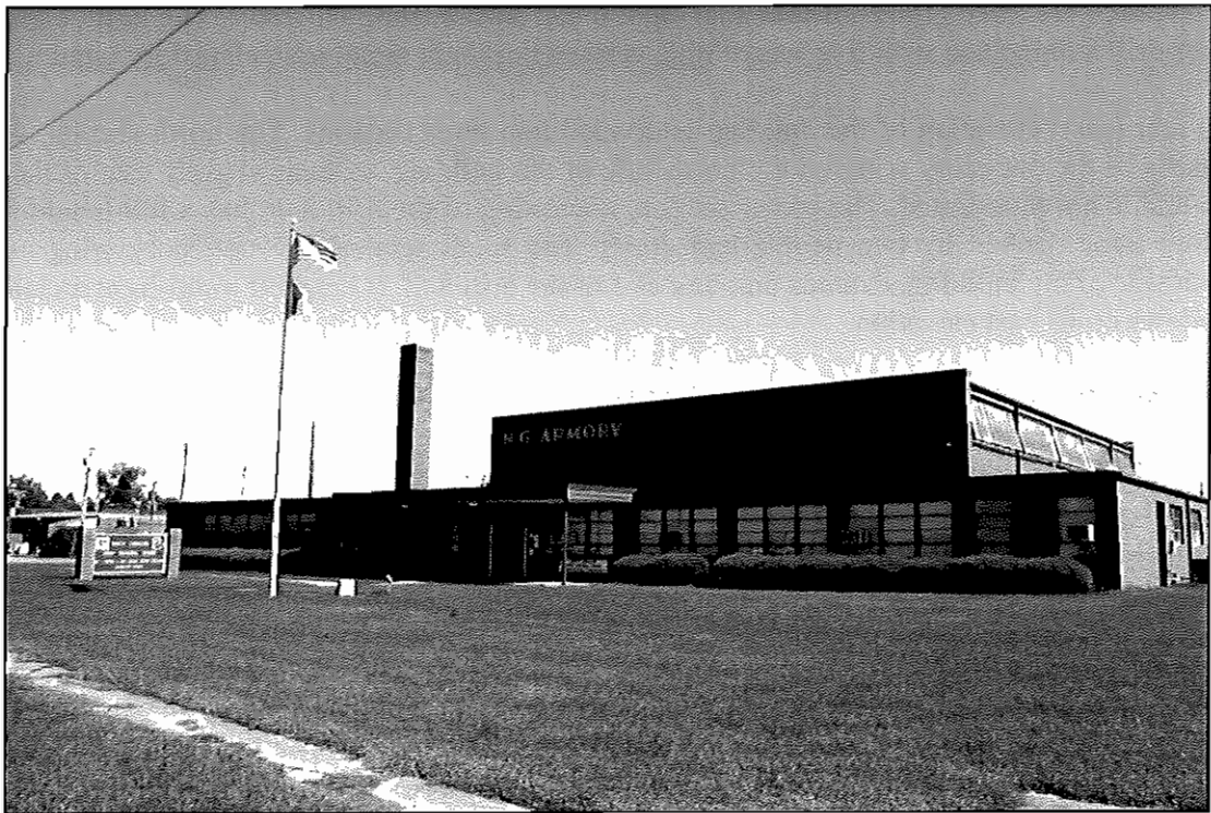
PLATE 4: Elizabeth City National Guard Armory
