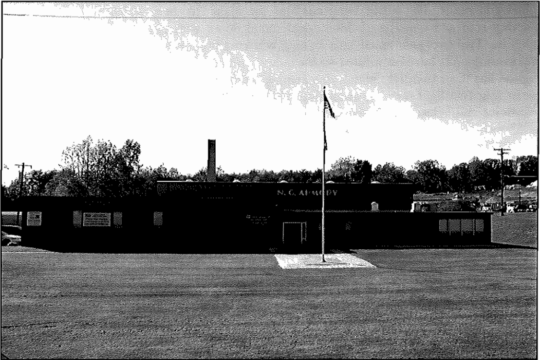
PLATE 6: Elkin National Guard Armory
