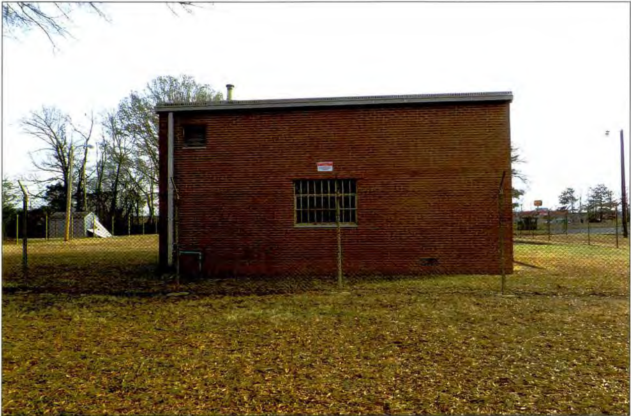
Figure 3.17 OMS building, west rear elevation.
