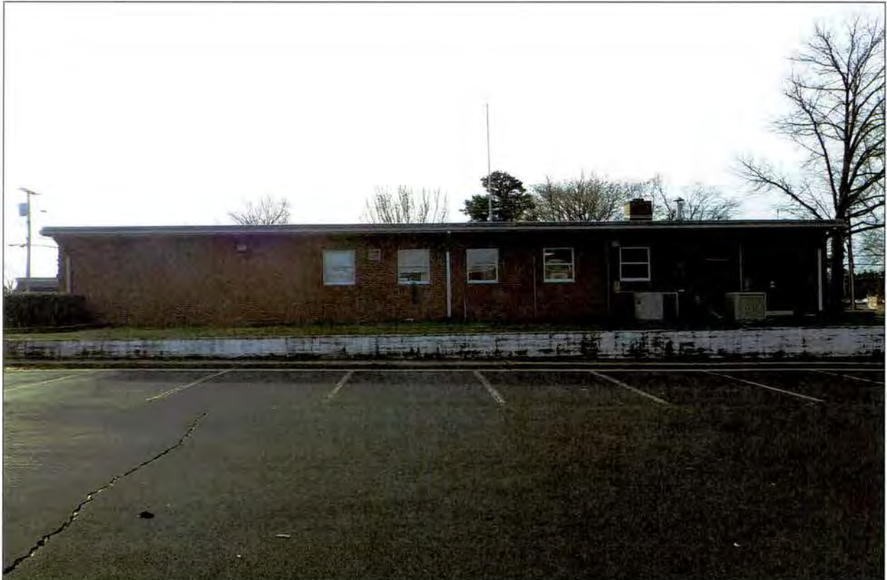
Figure 3.8 North rear elevation of the NC028/High Point ARC.
