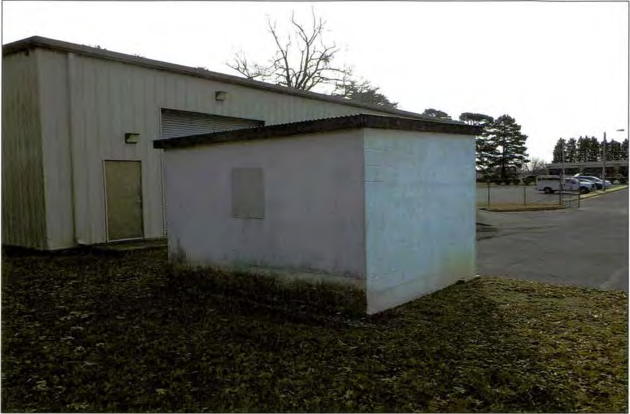
Figure 3.19 Flammable storage building, northwest oblique.
