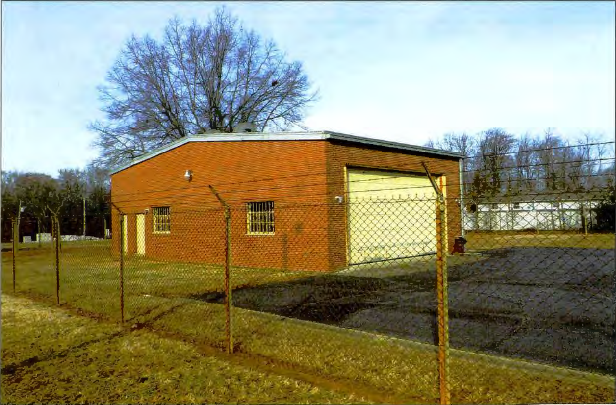
Figure 3.16 OMS building, southeast oblique.
