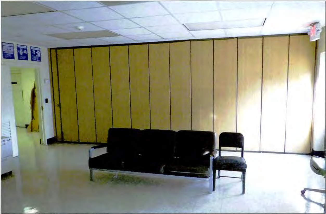
Figure 3.13 Accordion partition in the administration building of the NC028/High Point ARC.
