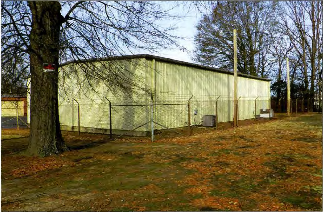
Figure 3.21 Metal classroom building, southeast oblique.
