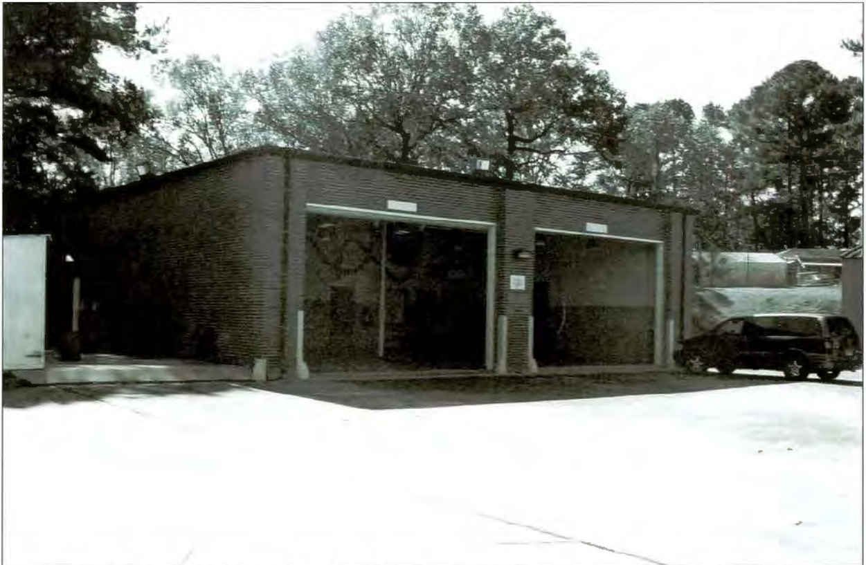
Figure 2.7 Typical OMS Building at the Lockhard ARC in Meridian, Mississippi, built in the late 1950s.
