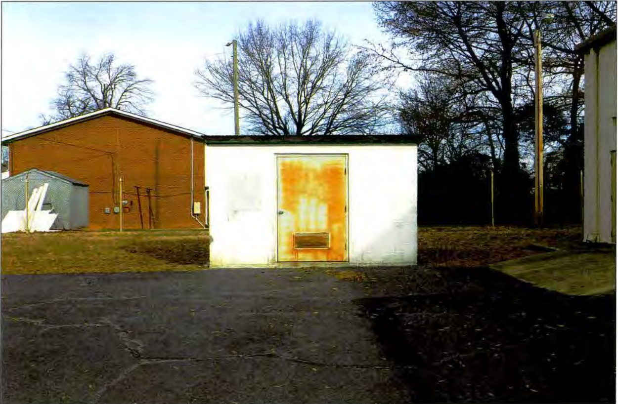
Figure 3.18 Flammable storage building, south front elevation.
