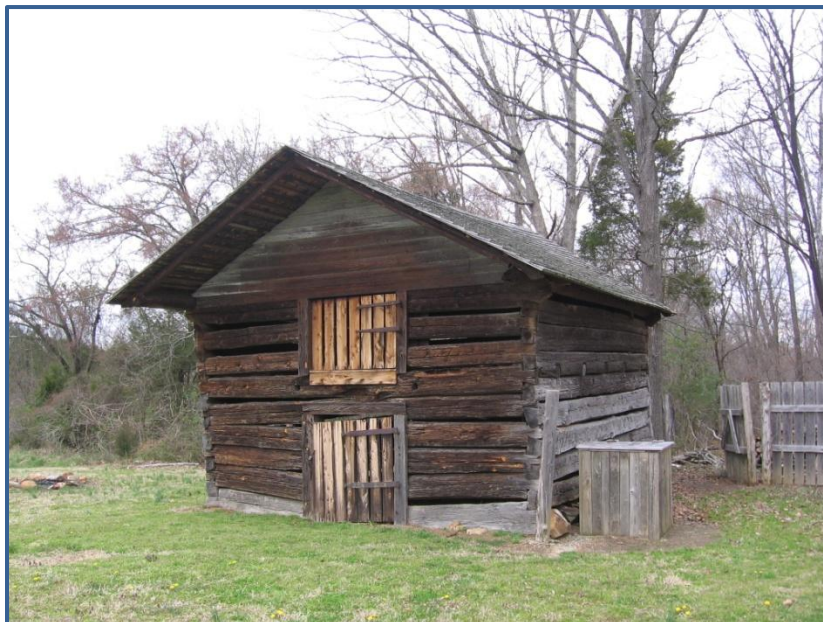
Figure 10. Polk Memorial – Crib. South and east elevations.
