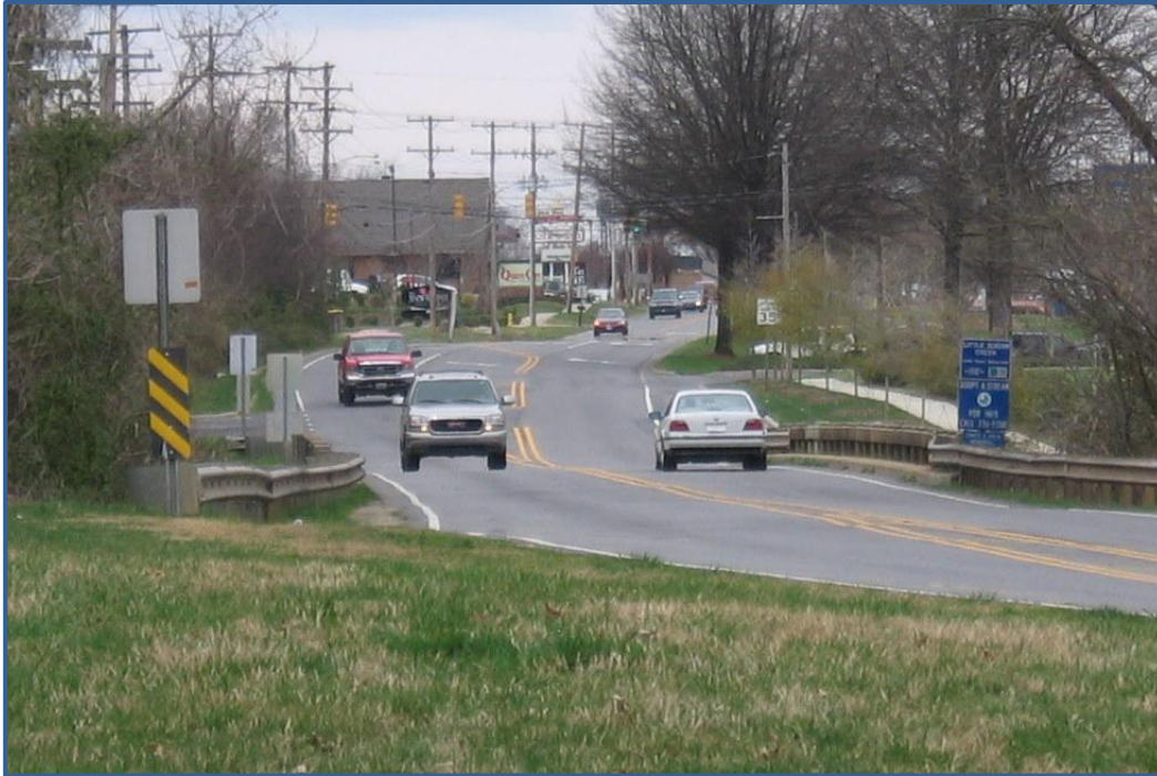
Property No. 3. Bridge No. 49. Looking north along South Polk Street.
