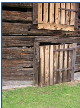
Figure 11. Polk Memorial – Crib. Detail of south elevation doorways.
