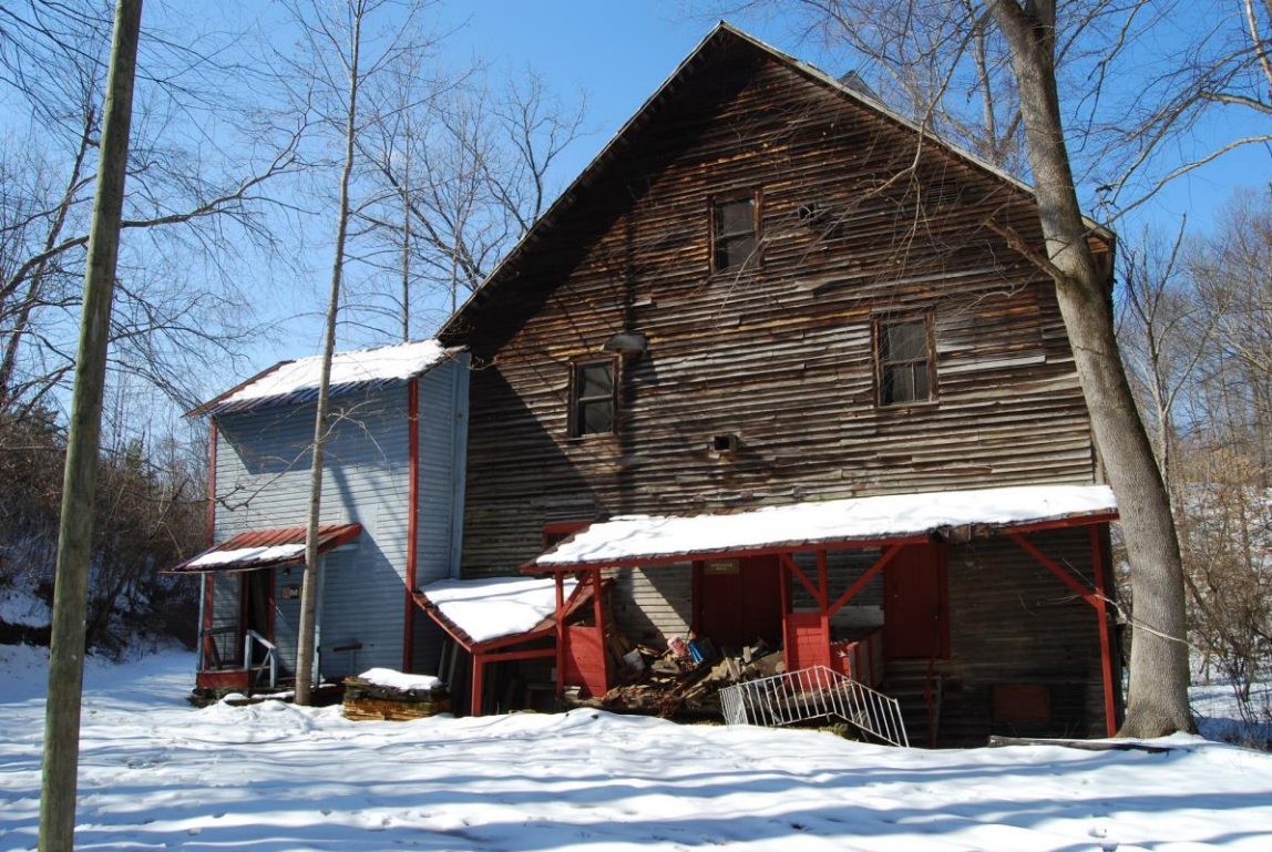
Worsham Mill southeast façade
