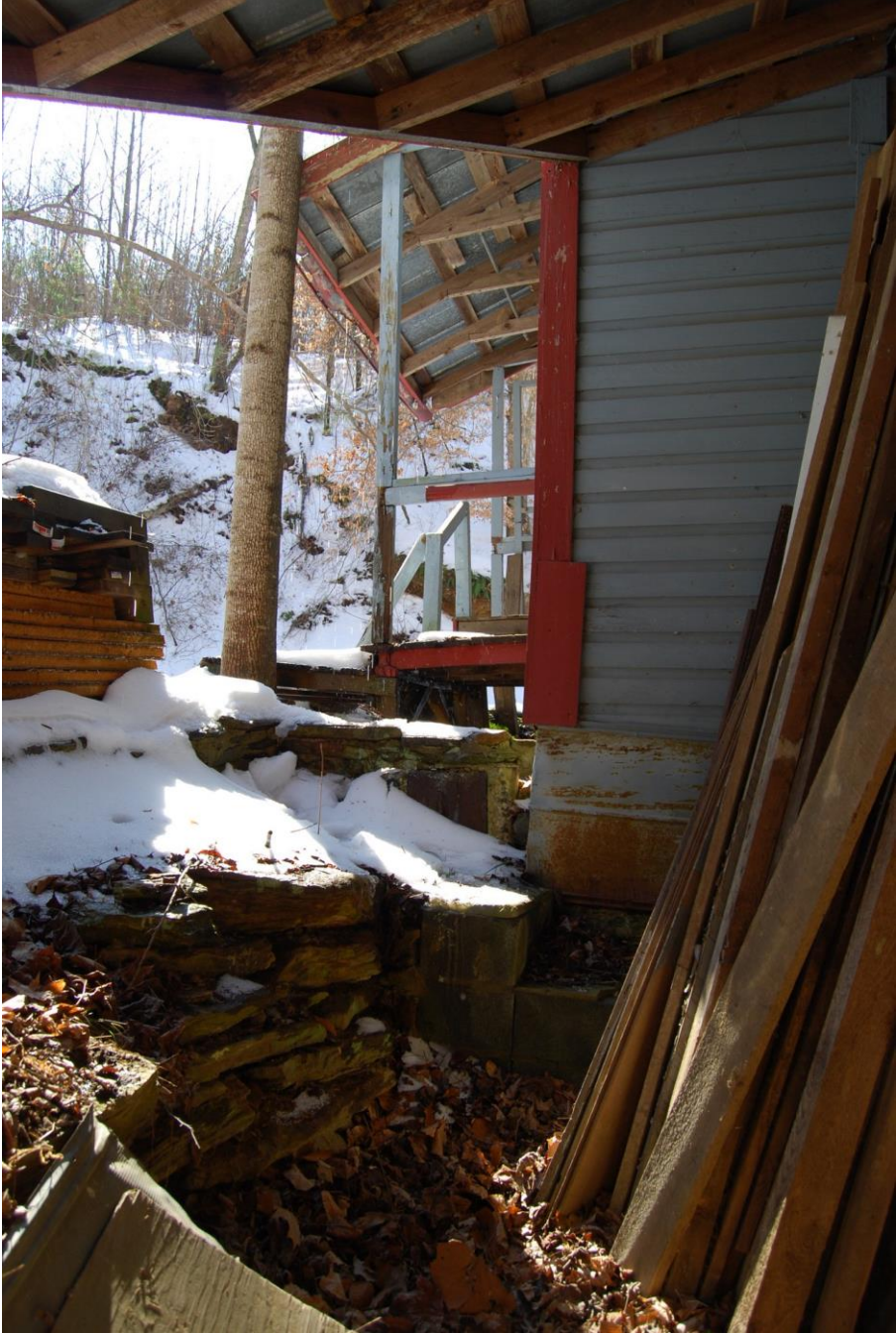
Detail of Foundation Materials
