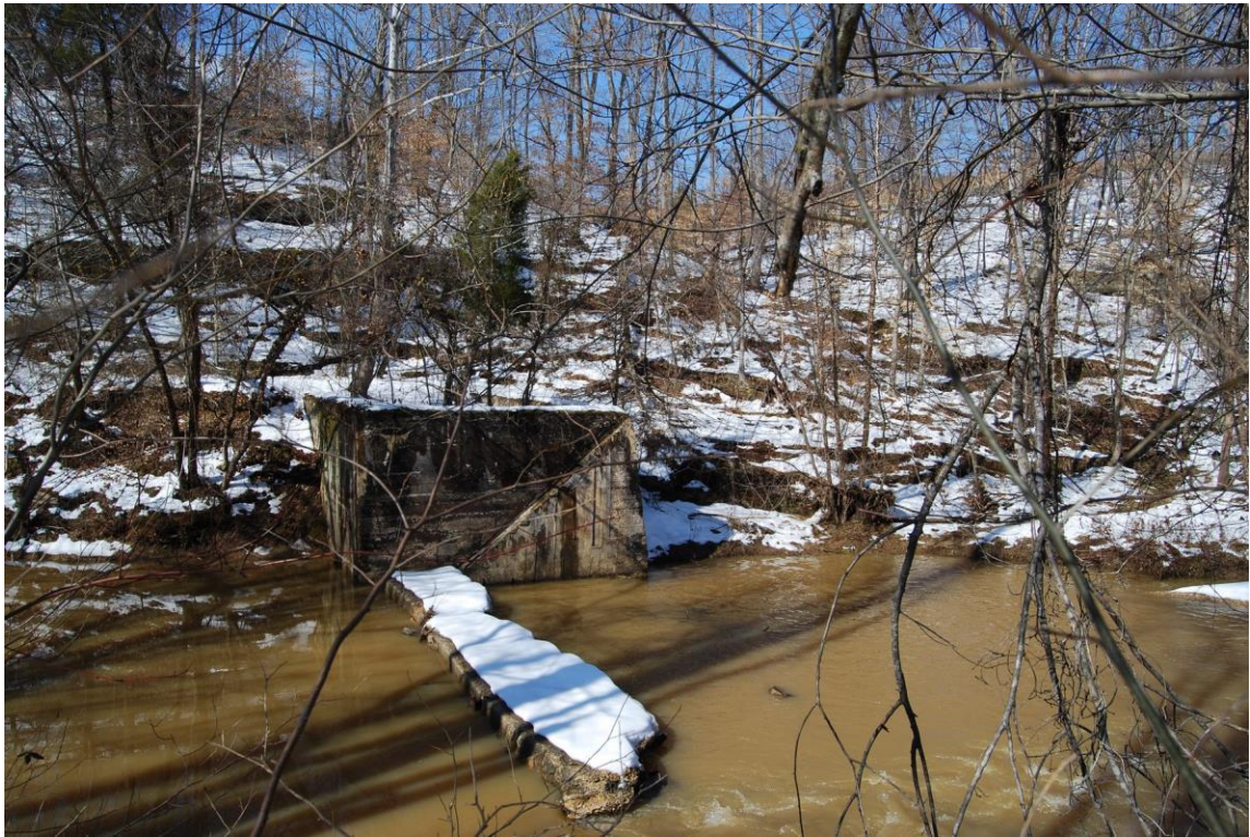
Dam Abutment on south side of Wolf Creek
