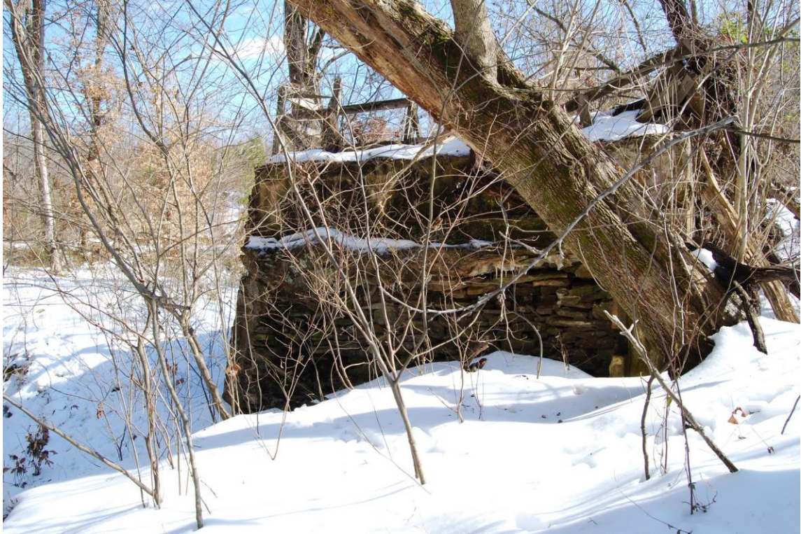
Dam Abutment on north side of Wolf Creek
