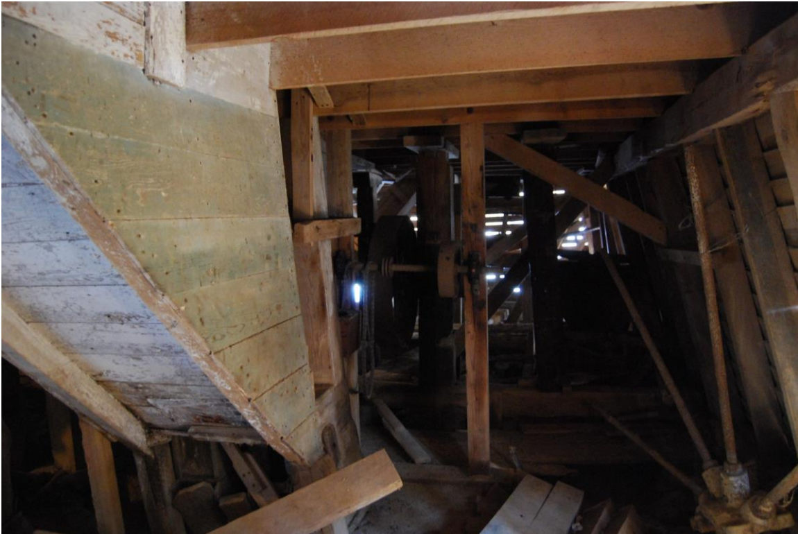
Timbers and Joists
