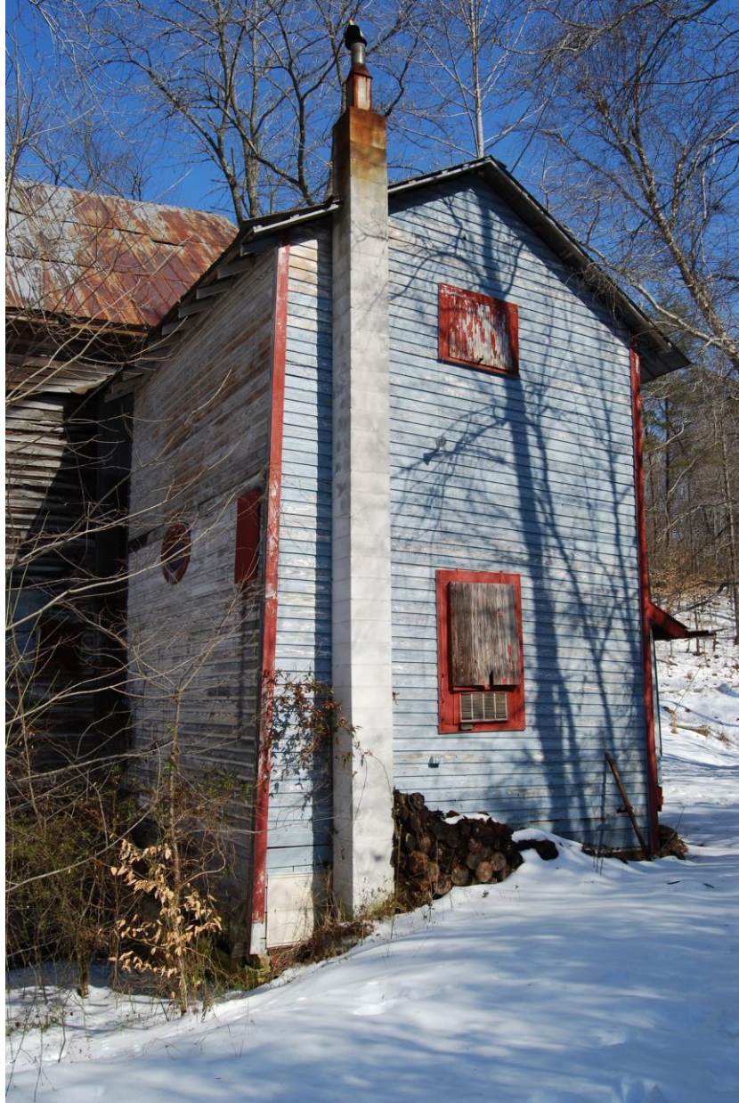
South (side) elevation of addition
