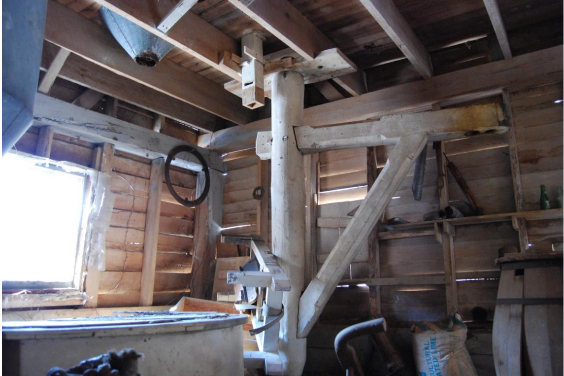
Swing arm hoist over grinding stone
