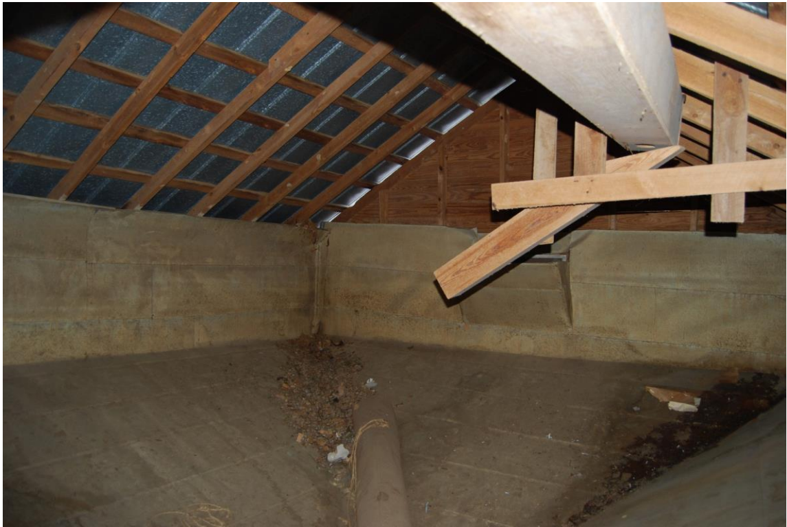
Grain bin (upper level of addition)
