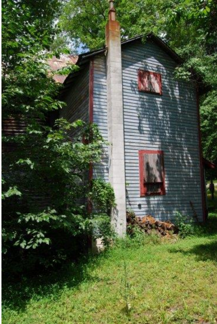
Southwest (side) elevation of addition
