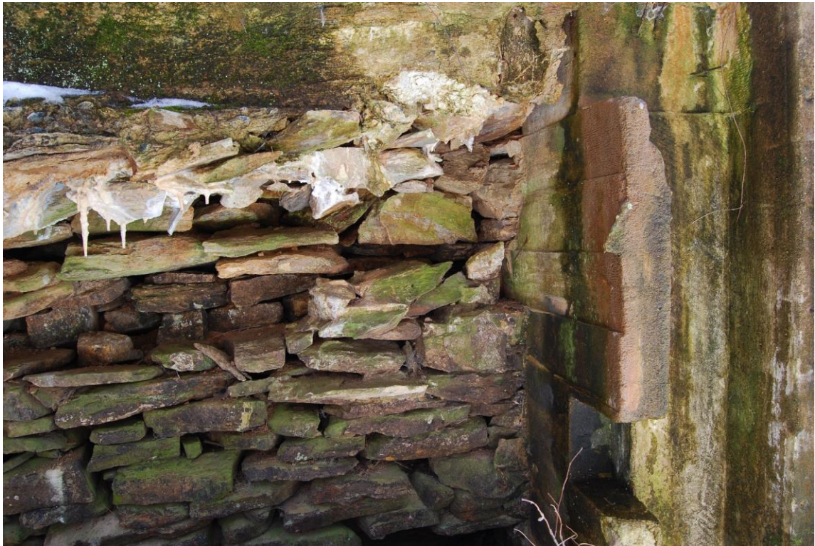
Detail of dam construction
