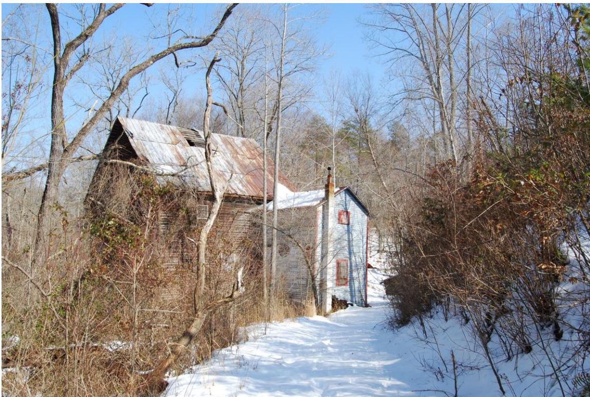
\frac{3}{4} View of Mill looking northeast
