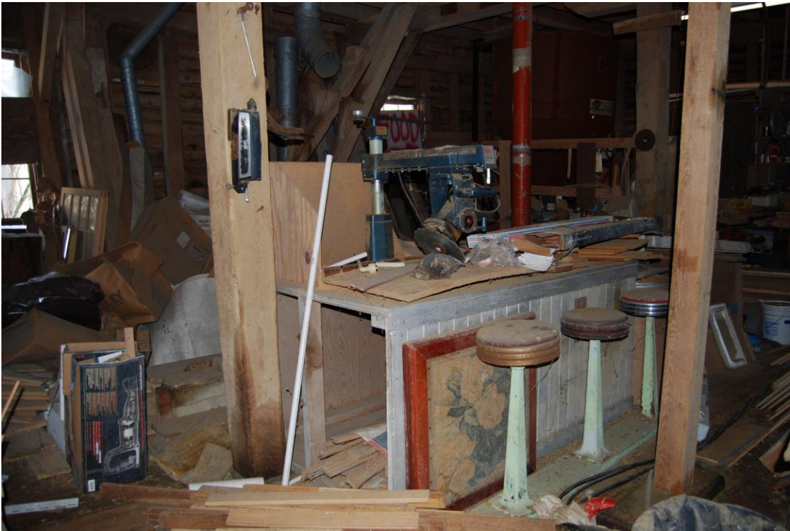
First floor showing some alterations
