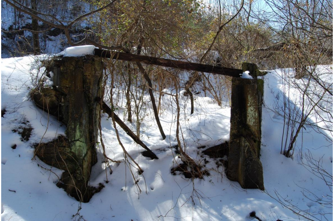
Headgate of millrace
