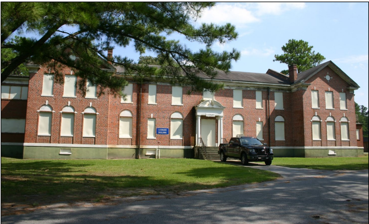
Figure 18: Leonard Building (ca. 1930), facade
