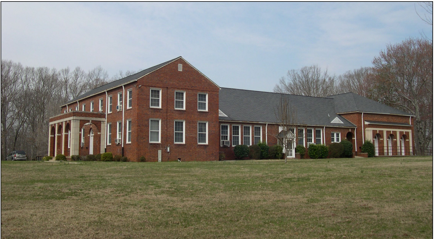
Figure 31 : Memorial Industrial School (orphanage), Winston-Salem, NC. Northup and O'Brien, ca. 1923 (photography courtesy Heather Fearnbach, 2008)
