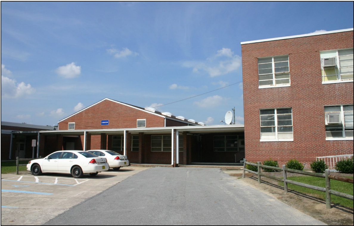
Figure 17: Gymnasium, rear extension of Mae D. Holmes Building
