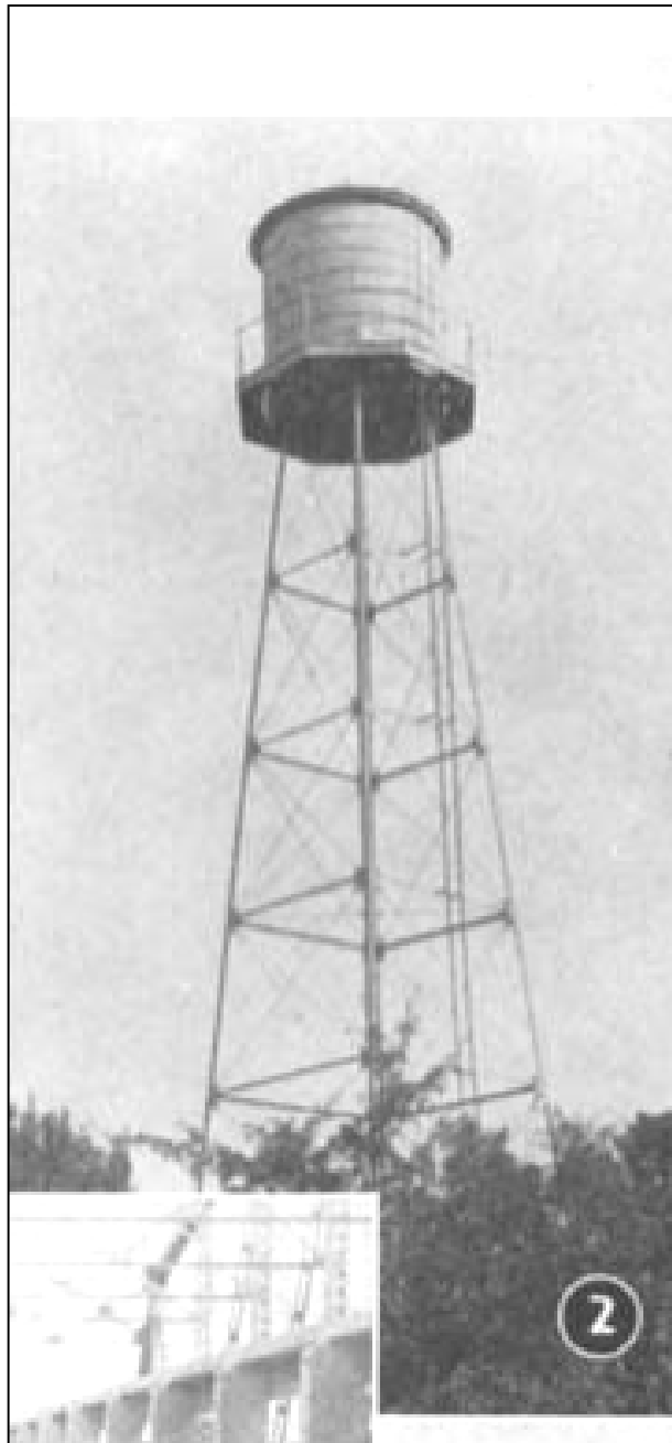
Figure 29 : Water tower built on Farm Colony complex ca. 1934-1935, from NC-FERA documents
