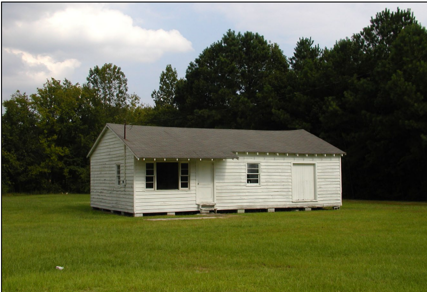
Property 21: Building "A" E. Side, facing 2857 Hull Road PIN 450601458836
