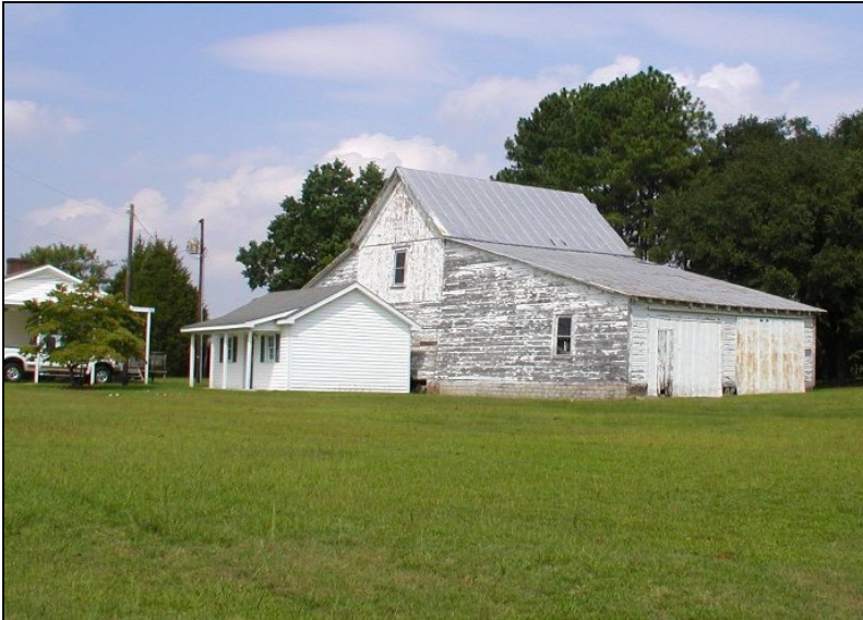
Property 6 : Barn SE corner Hillcrest Road And Vernon Avenue PIN 450512851652
