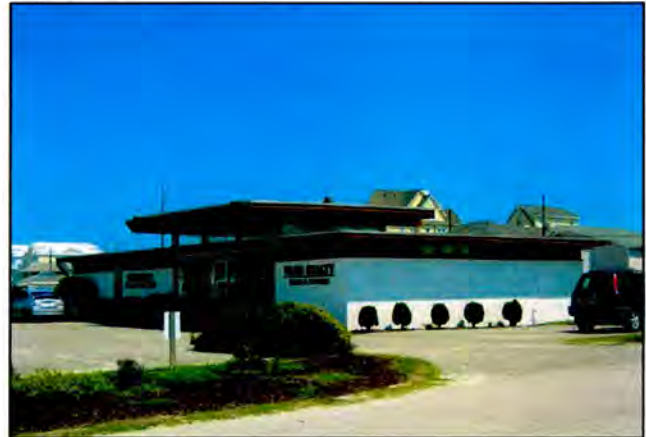
Ward Realty Corporation - view looking southeast
