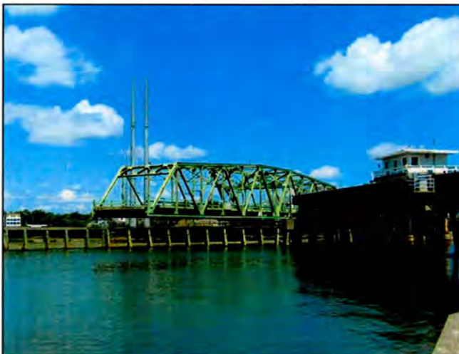
View of the main swing span while in the process of opening.
