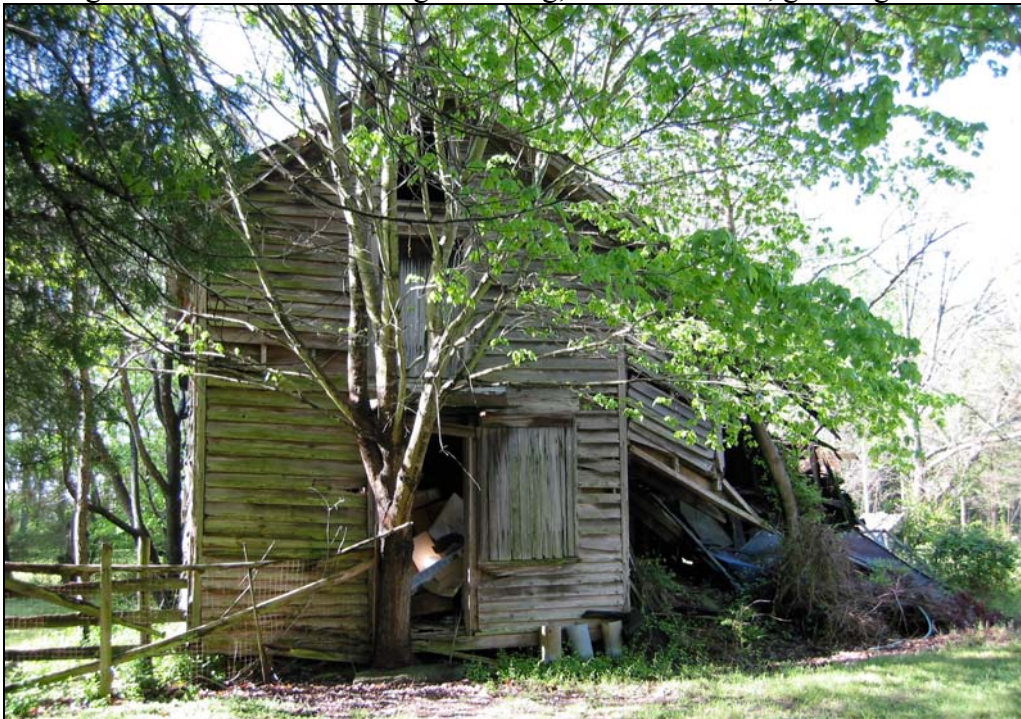
Figure 45: farm office/storage building, north elevation, g on Figure 23
