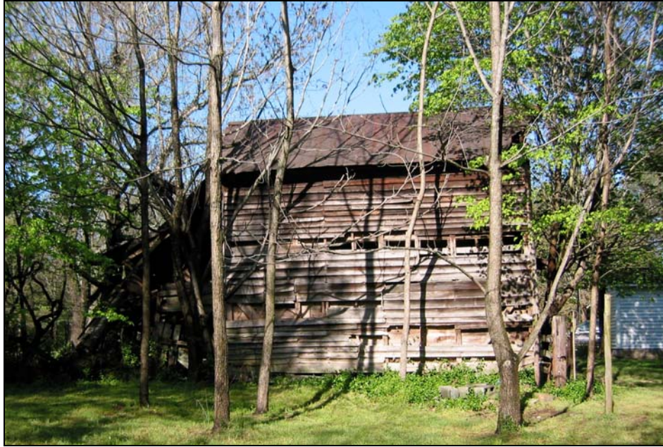
Figure 46: farm office, east elevation, g on Figure 23
