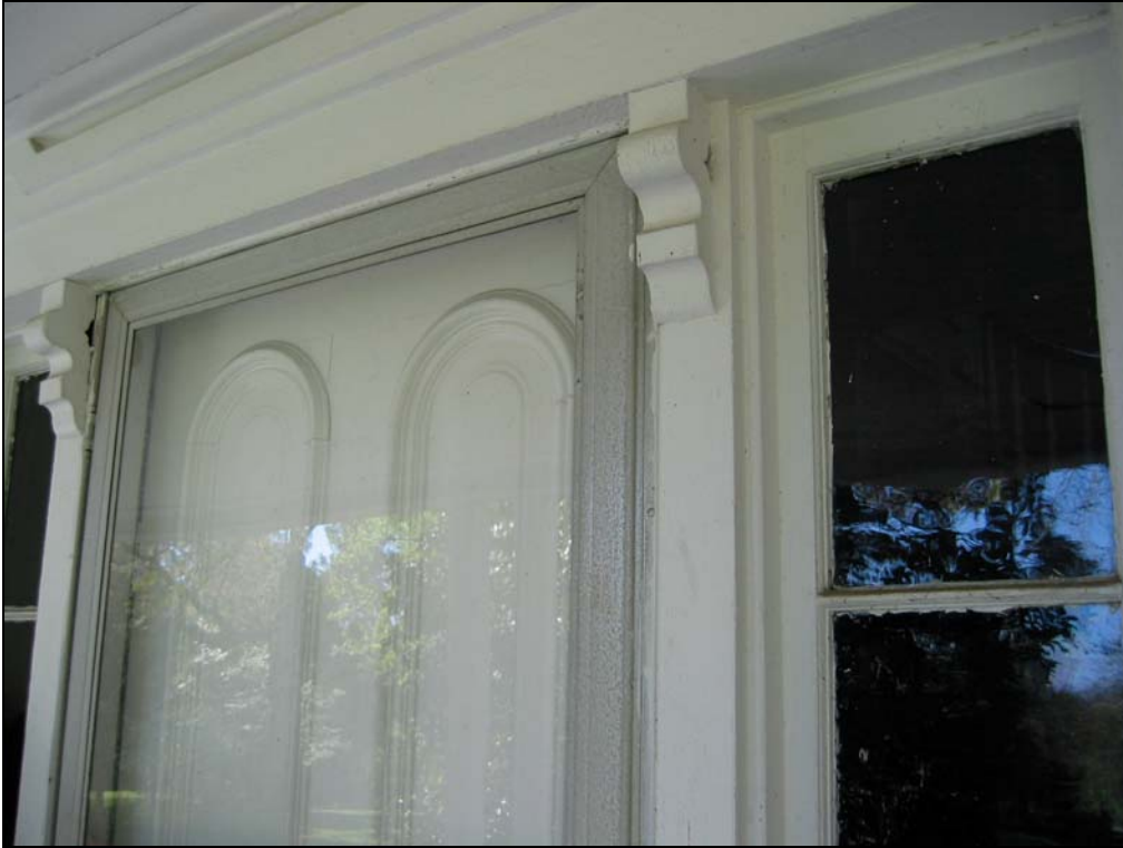
Figure 28: Caldwell House door detail
