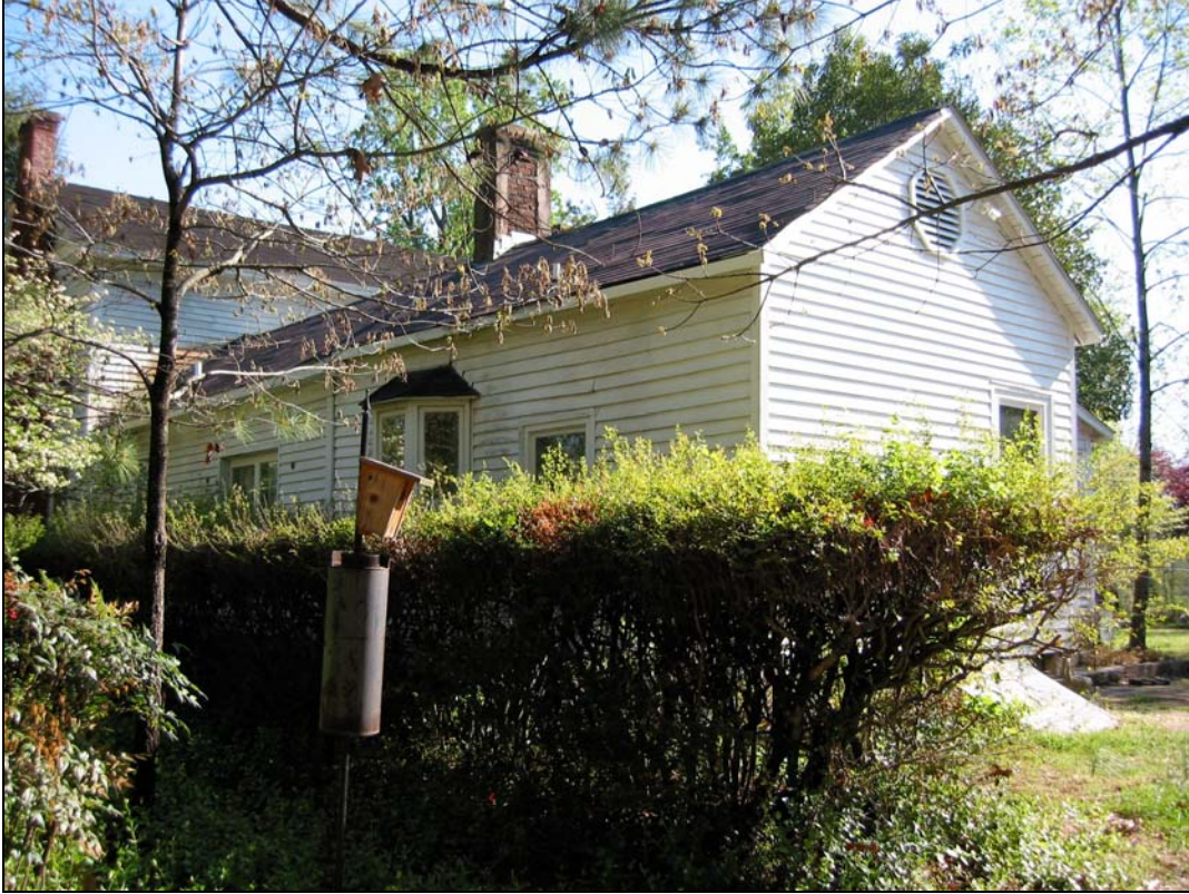
Figure 32: rear ell, southwest elevation
