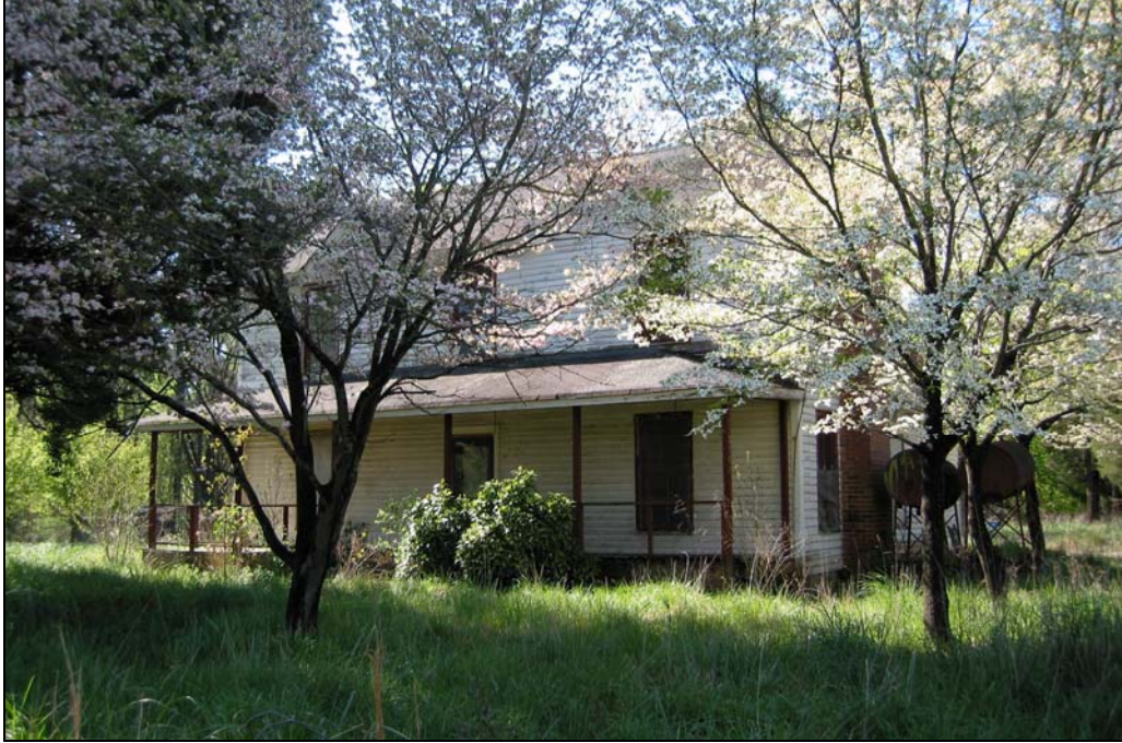
Figure 4: Mayes House, north elevation
