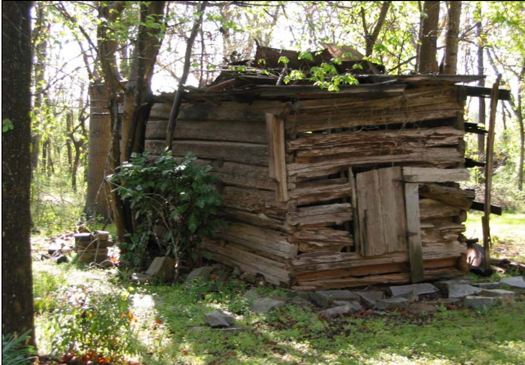
Figure 44: log animal barn, west elevation, d on Figure 23
