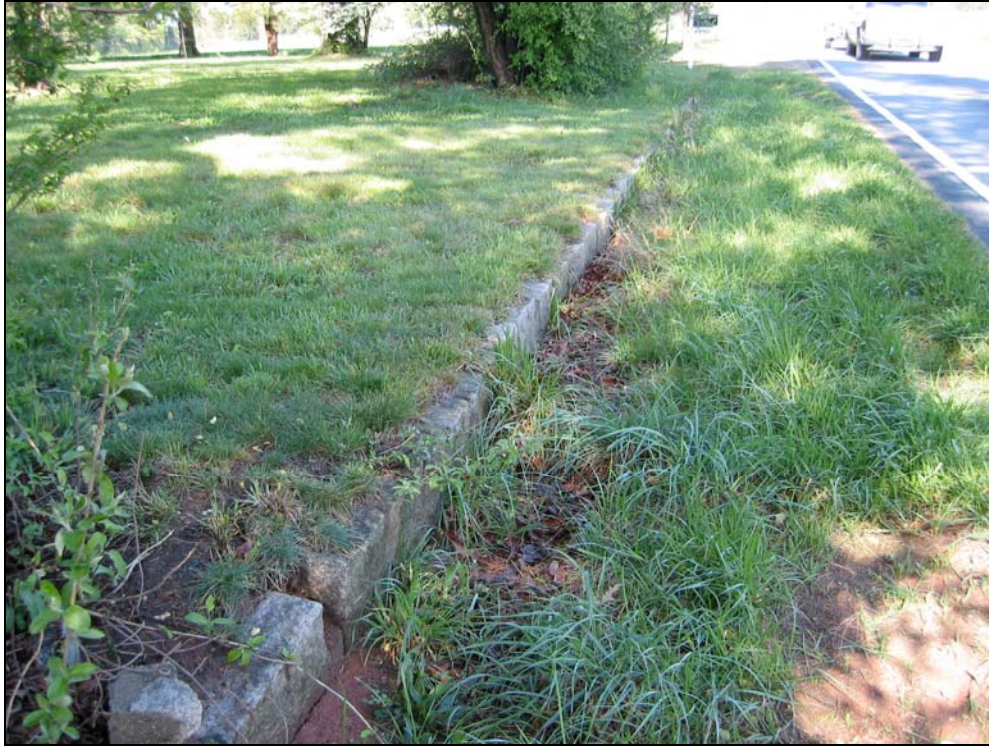
Figure 38: granite curbing between front yard and NC 73
