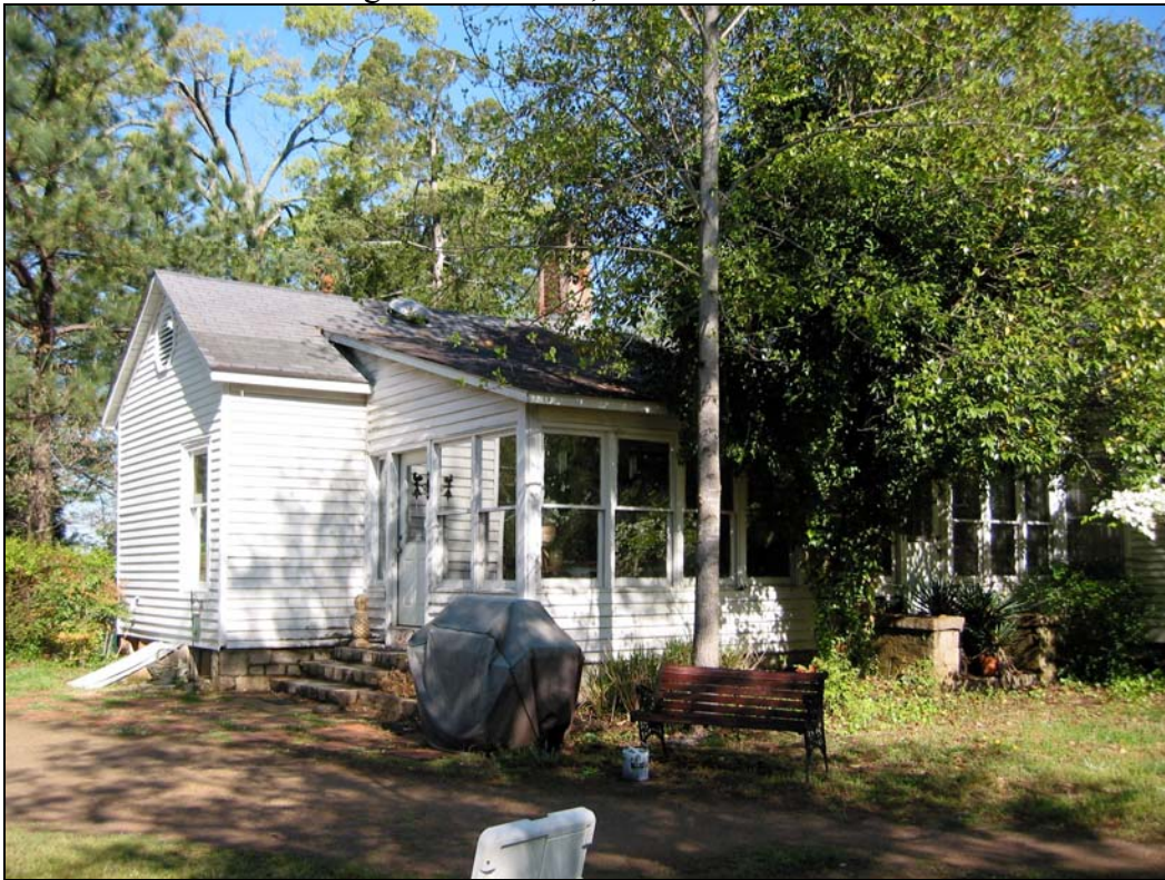
Figure 31: rear ell, southeast corner
