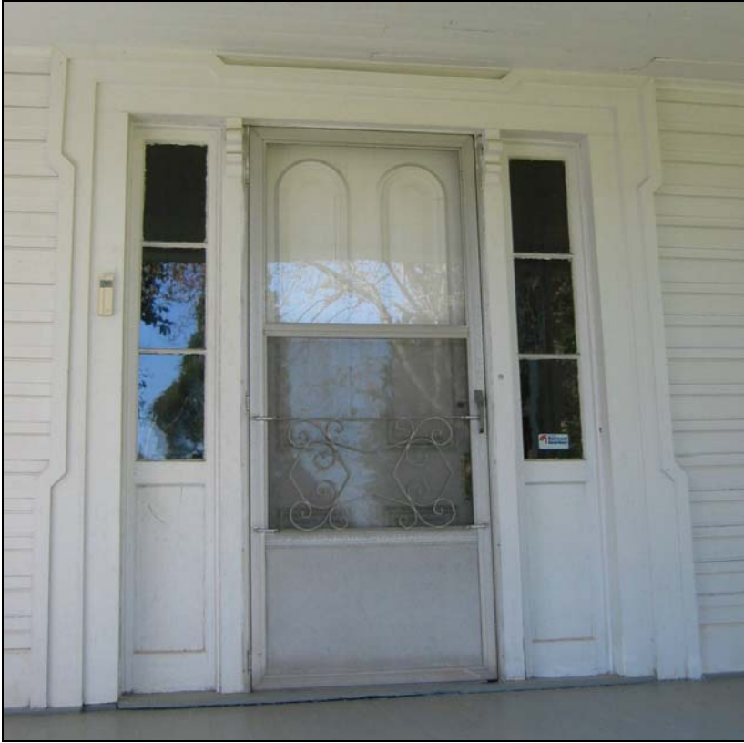
Figure 26: Caldwell House front door, north elevation
