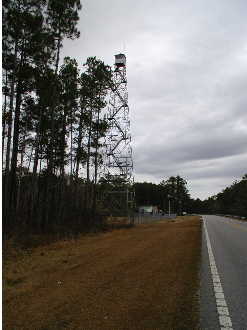
East Lake Fire Tower, view toward the east on US 64
