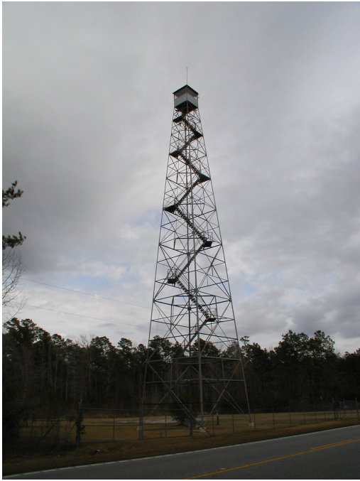
View to northeast
