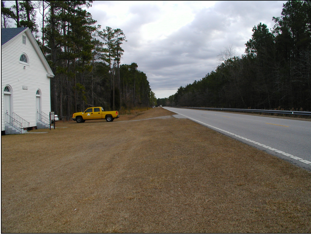
View of area looking east on US 64
