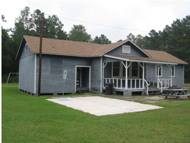
Property 16 East Lake Community Center DR 631 PIN 971800253027 16674 HWY 64
