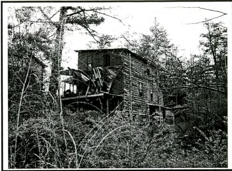
Figure 7 – Stepp's Mill, north elevation
