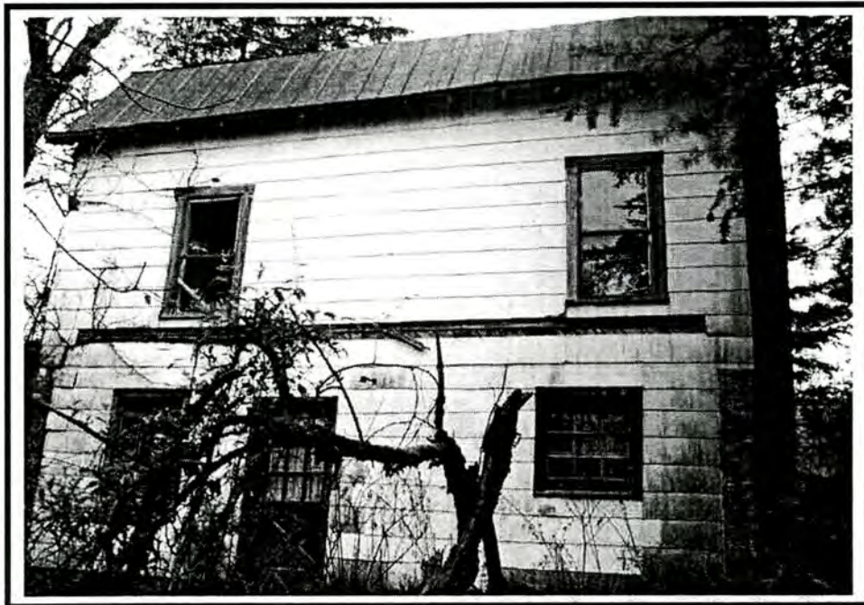
Figure 14 – Dwelling at Stepp's Mill, west elevation
