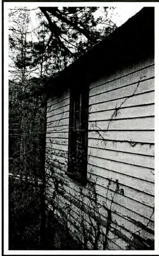
Figure 11 – Office at Stepp's Mill, south elevation
