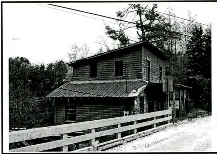
Figure 4 – Stepp’s Mill, south elevation
