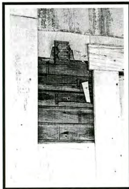
Figure 17 – Dwelling at Stepp's Mill, detail of wood siding
