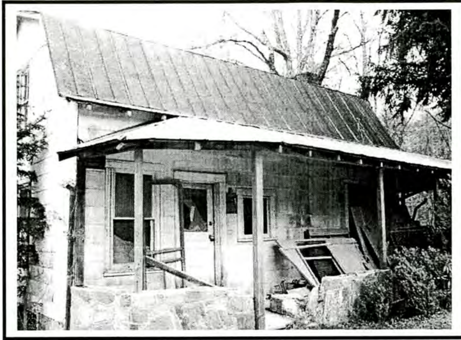
Figure 13 – Dwelling at Stepp's Mill, east elevation
