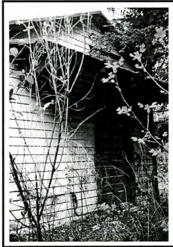
Figure 10 – Office at Stepp's Mill, east elevation
