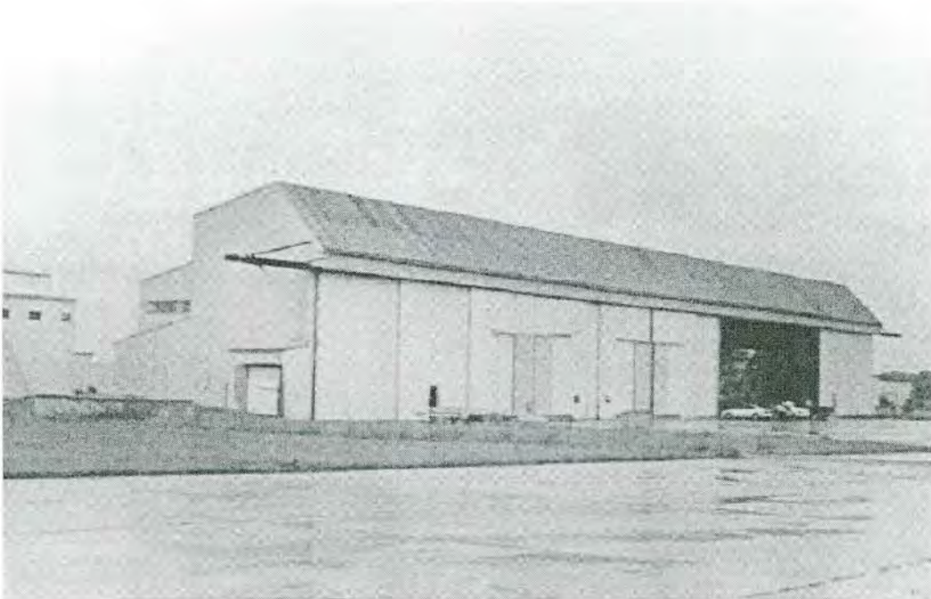
Figure 4-102. Multi-purpose Wing Hangar, front, designed by Luria Engineering, at former Lincoln Air Force Base, Nebraska (Source: Weitze 1999b).
