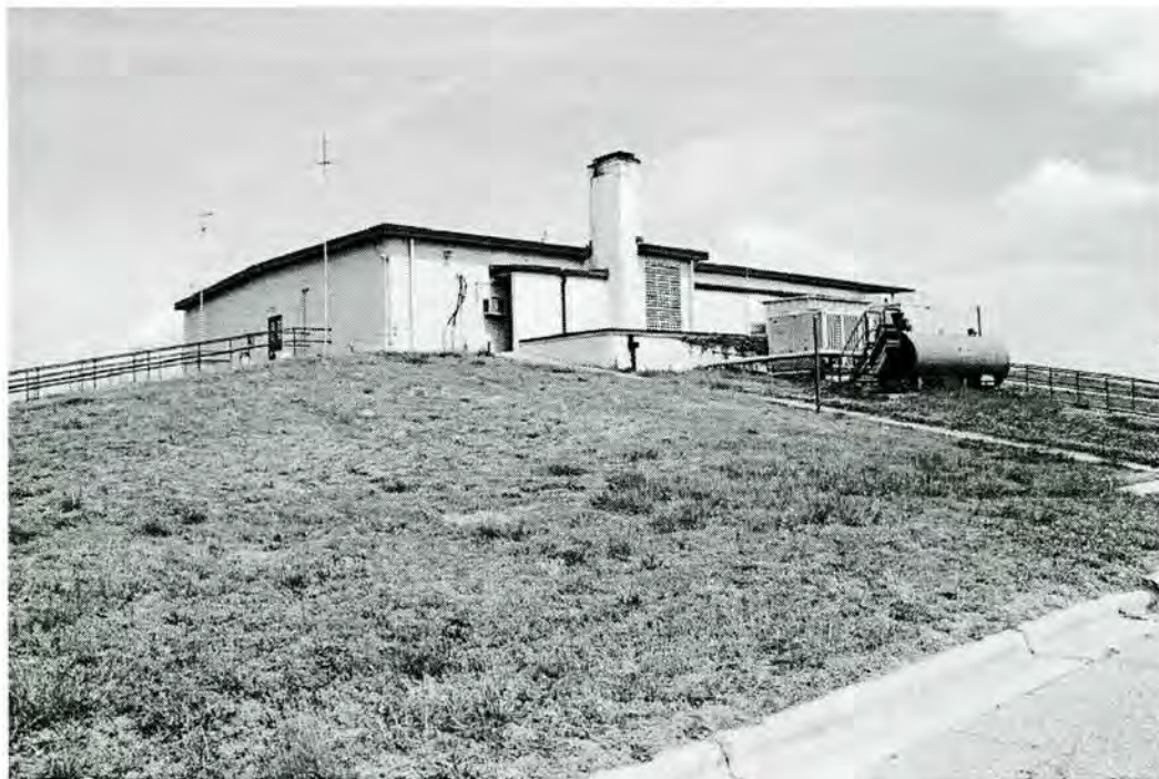
Figure 4-52. Building 2130, facing southeast (Photograph by Joe C. Freeman, 2004).
