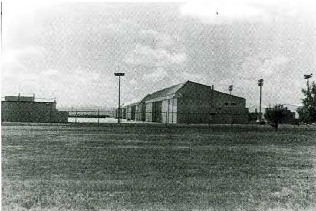
Figure 4-99. Multi-purpose Wing Hangar, front, designed by Luria Engineering, Ellsworth Air Force Base, South Dakota (Source: Weitze 1999b).
