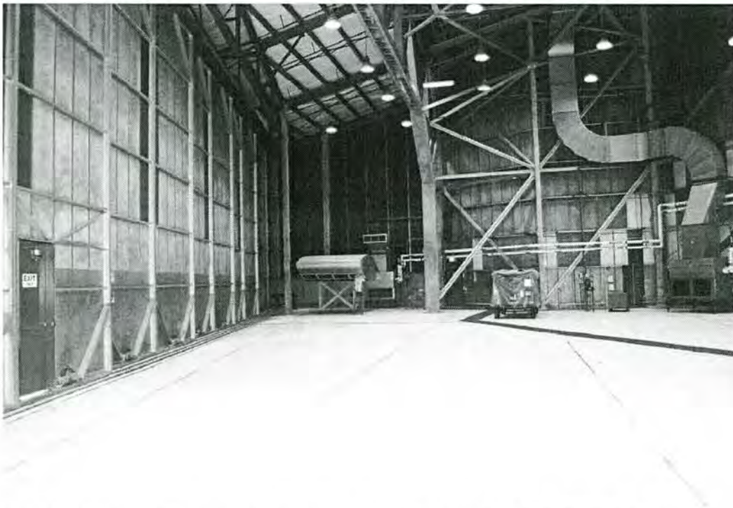
Figure 4-95. Building 4828, interior of bypassing rolling doors (Photograph by Joe C. Freeman, 2004).
