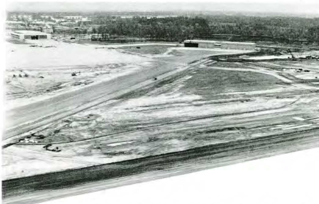
Figure 4-10. Building 5015, November 1958 (Source: 4 th Wing History Office, Seymour Johnson Air Force Base, North Carolina).
