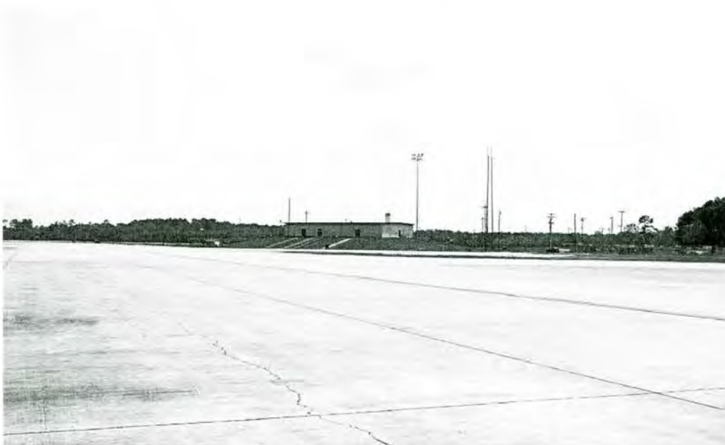
Figure 4-61. Alert apron in foreground and Building 2130 in background, facing southwest (Photograph by Joe C. Freeman, 2004).
