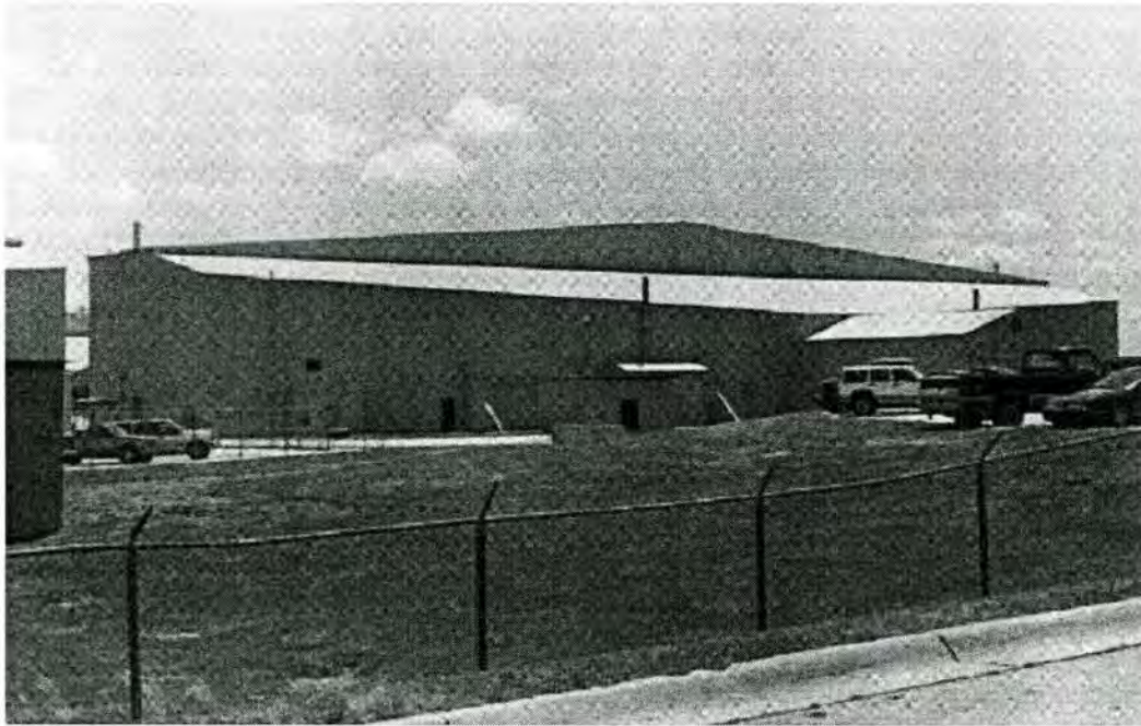
Figure 4-98. B-36 Wing Hangar, rear, at Ellsworth Air Force Base, South Dakota (Source: Weitze 1999b).
