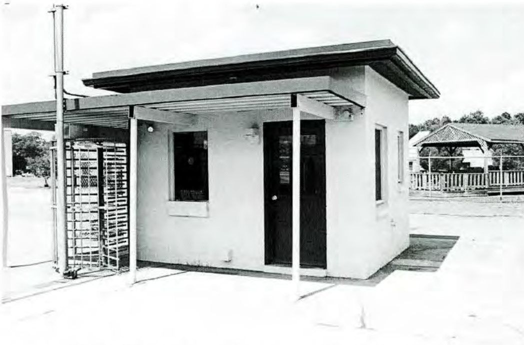
Figure 4-30. Building 5014, guardhouse and turnstile associated with ADC Alert Complex (Photograph by Joe C. Freeman, 2004)
