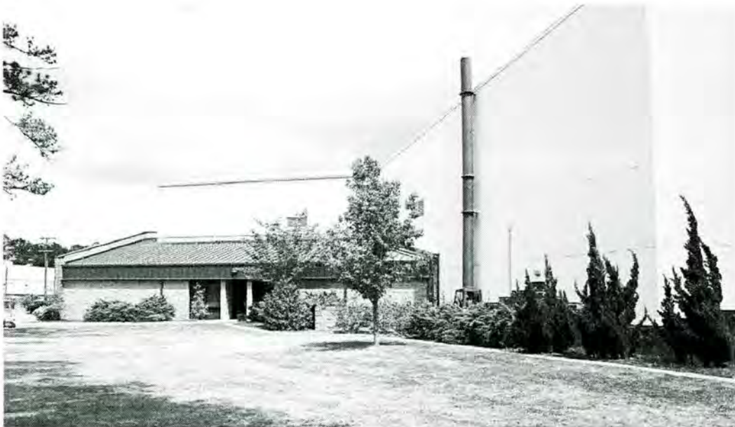
Figure 4-89. Building 4828, facing northeast, with one of the additions that replaced original concrete block structures (Photograph by Joe C. Freeman, 2004).
