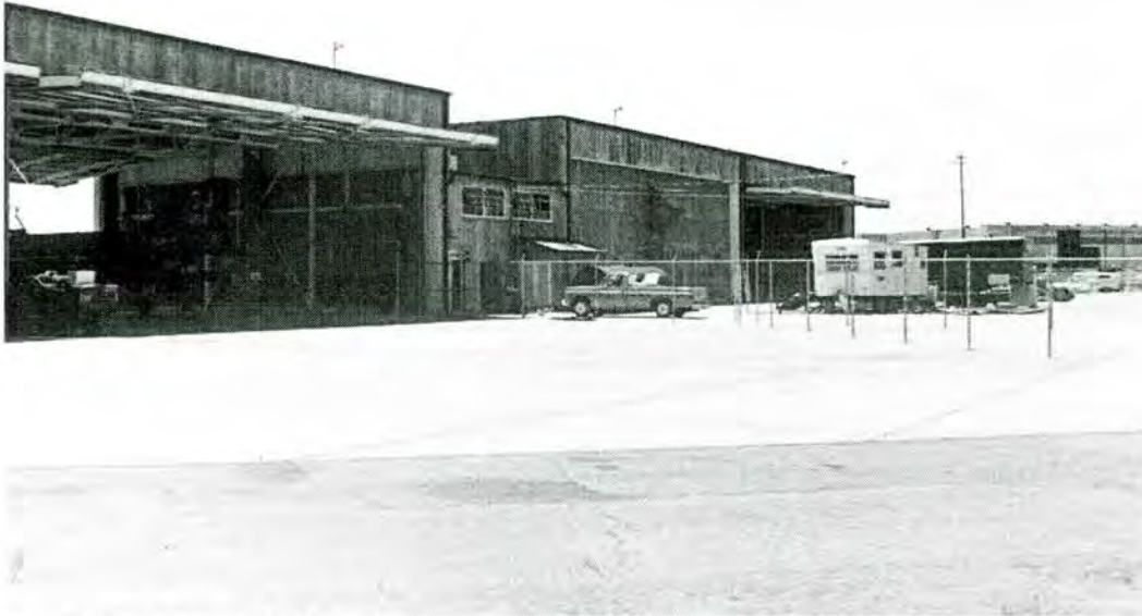
Figure 4-13. Building 5015, date unknown (Source: 4 th Wing History Office, Seymour Johnson Air Force Base, North Carolina).
