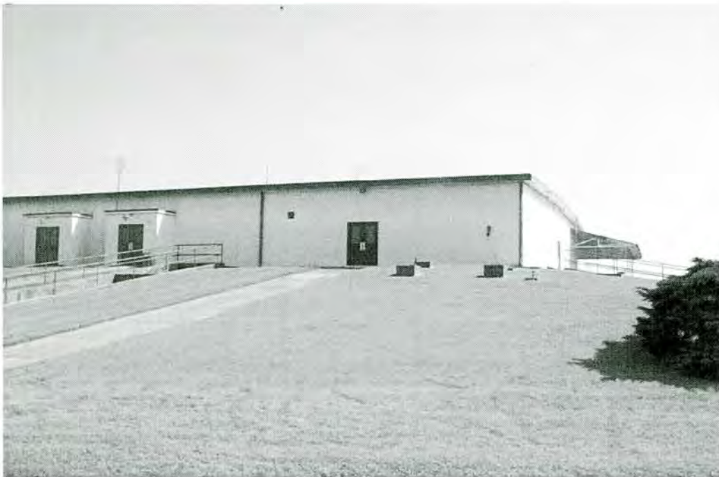
Figure 4-68. 70-man Readiness Crew Building, Columbus Air Force Base, Mississippi, 2003 (Source: Salo and Prior 2003).
