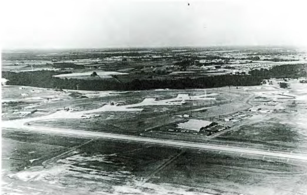
Figure 4-49. SAC alert complex under construction, ca. 1959. Note Christmas tree apron in center and Building 2130 on left hand side of photograph (Source: 4 th Wing History Office, Seymour Johnson Air Force Base, North Carolina).
