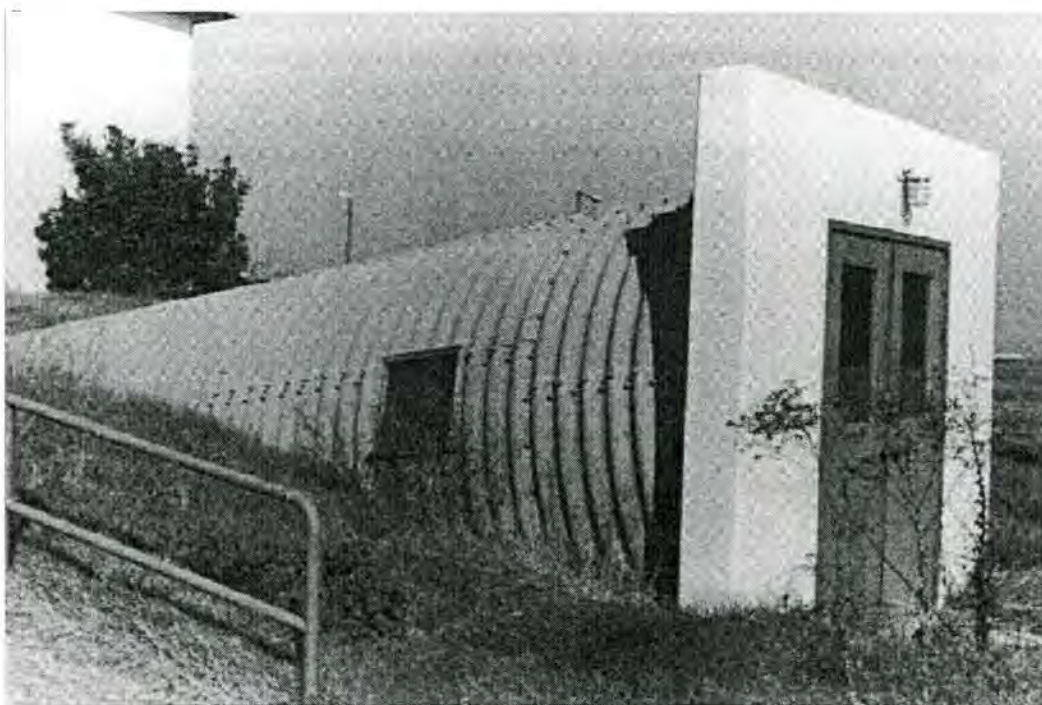
Figure 4-69. Tunnel egress for Readiness Crew Building, Castle Air Force Base, California (Source: Weitze 1999b).
