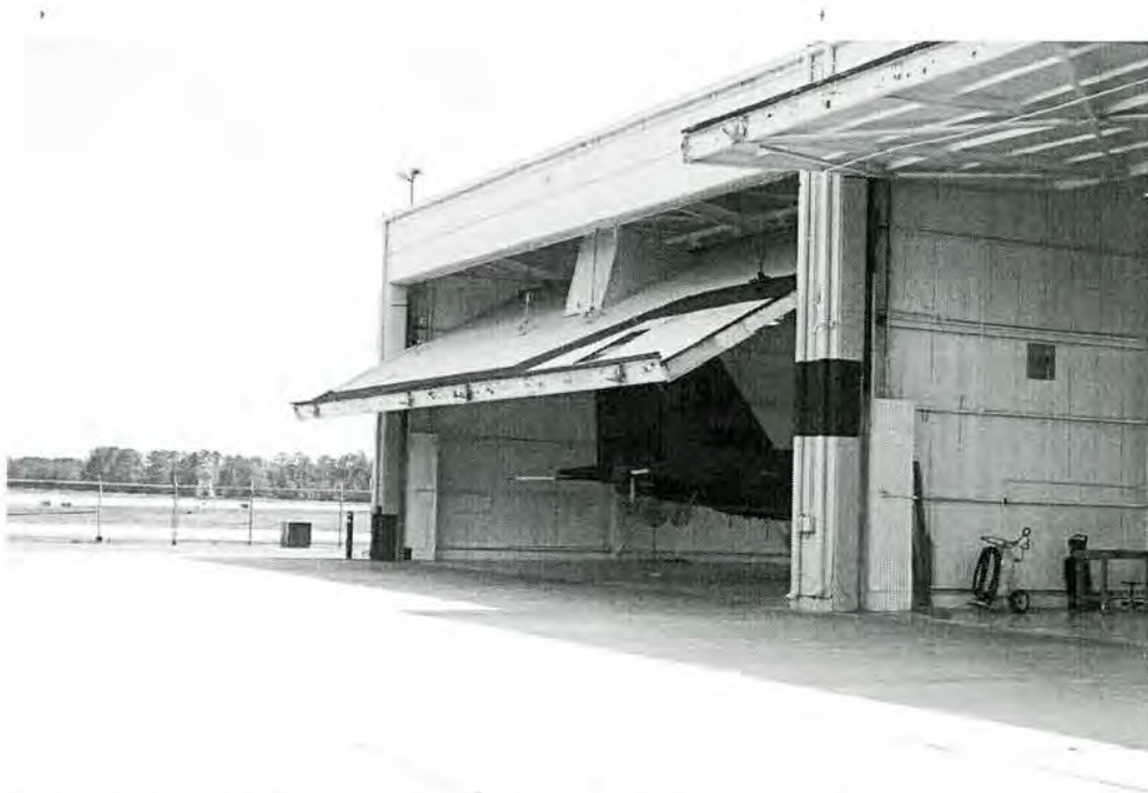
Figure 4-26. Building 5015, facing southeast (Photograph by Joe C. Freeman, 2004).
