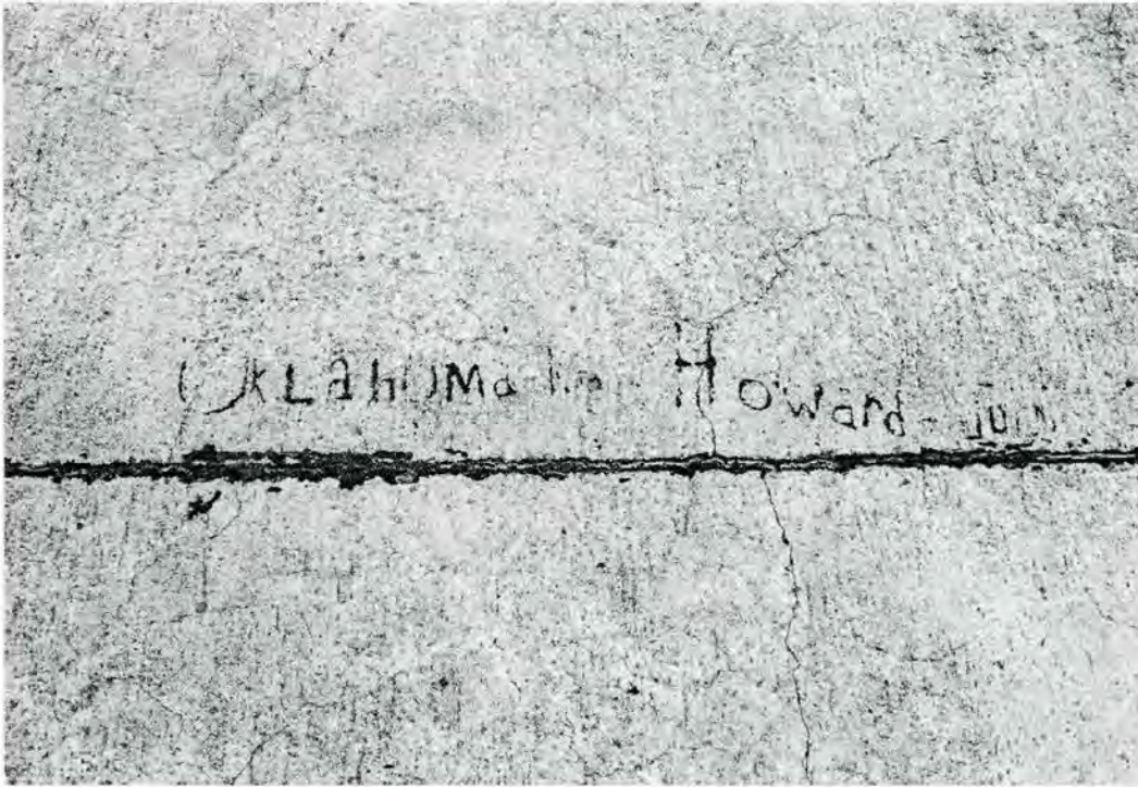
Figure 4-64. Graffiti on Christmas tree apron (Photograph by Joe C. Freeman, 2004).
