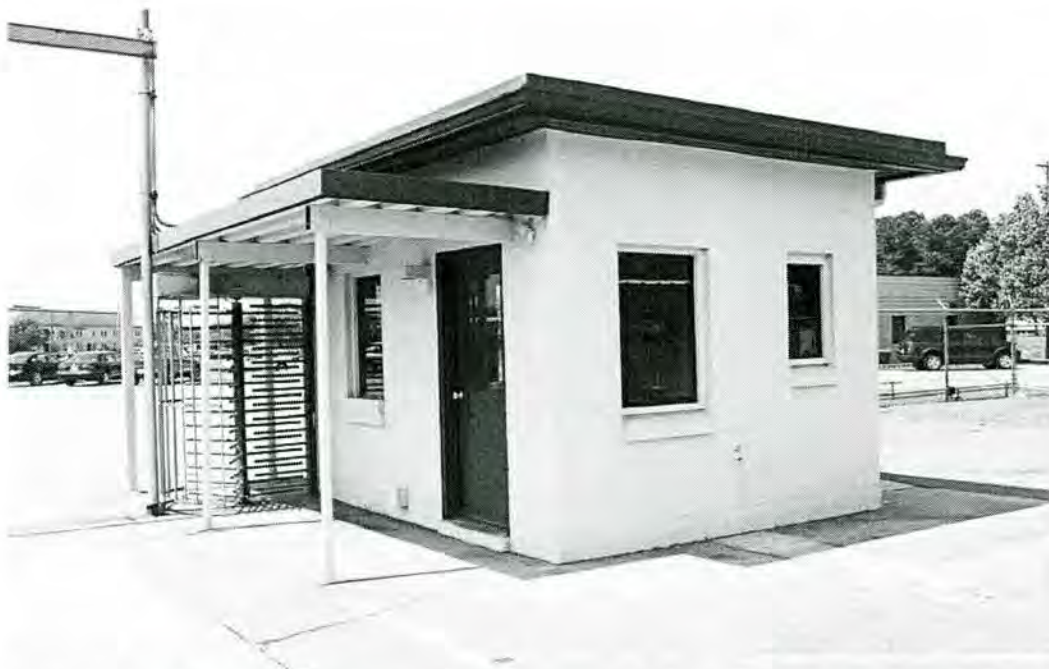
Figure 4-31. Building 5014, guardhouse and turnstile associated with ADC Alert Complex (Photograph by Joe C. Freeman, 2004).
