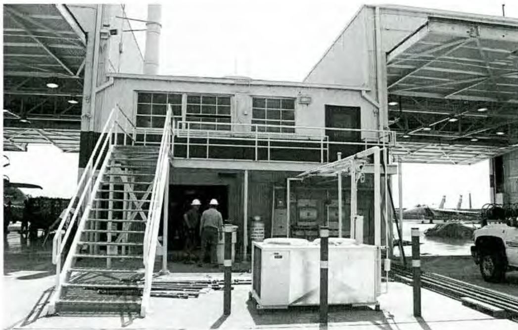
Figure 4-22. Building 5015, facing southwest (Photograph by Joe C. Freeman, 2004).
