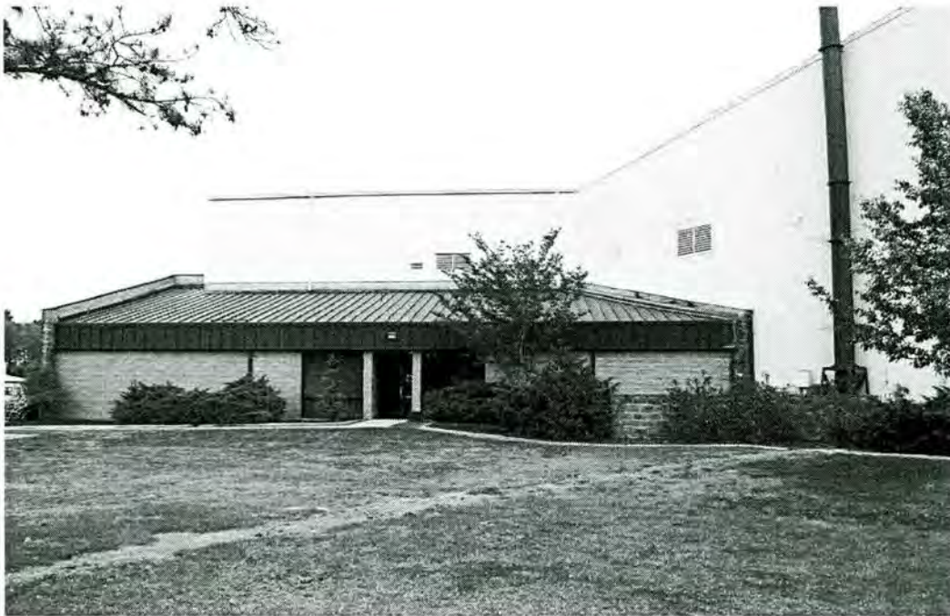
Figure 4-90. Building 4828, facing northeast, with one of the two additions placed on east and west side of building (Photograph by Joe C. Freeman, 2004).
