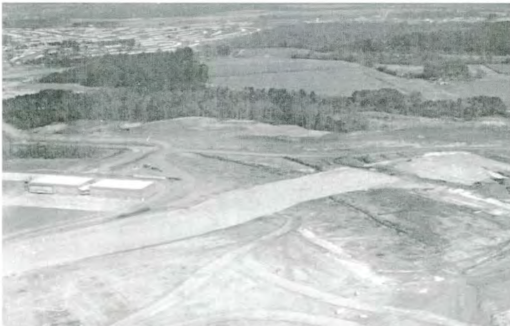
Figure 4-12. Building 5015, December 1958 (Source: 4 th Wing History Office, Seymour Johnson Air Force Base, North Carolina).
