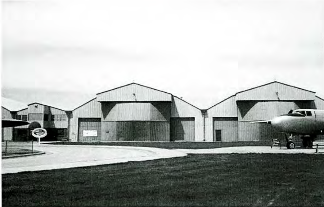
Figure 4-34. Butler Four Pocket Alert Hangar, Ellsworth Air Force Base, South Dakota (Scott D. Murdock personal collection © 2001, used with permission).
