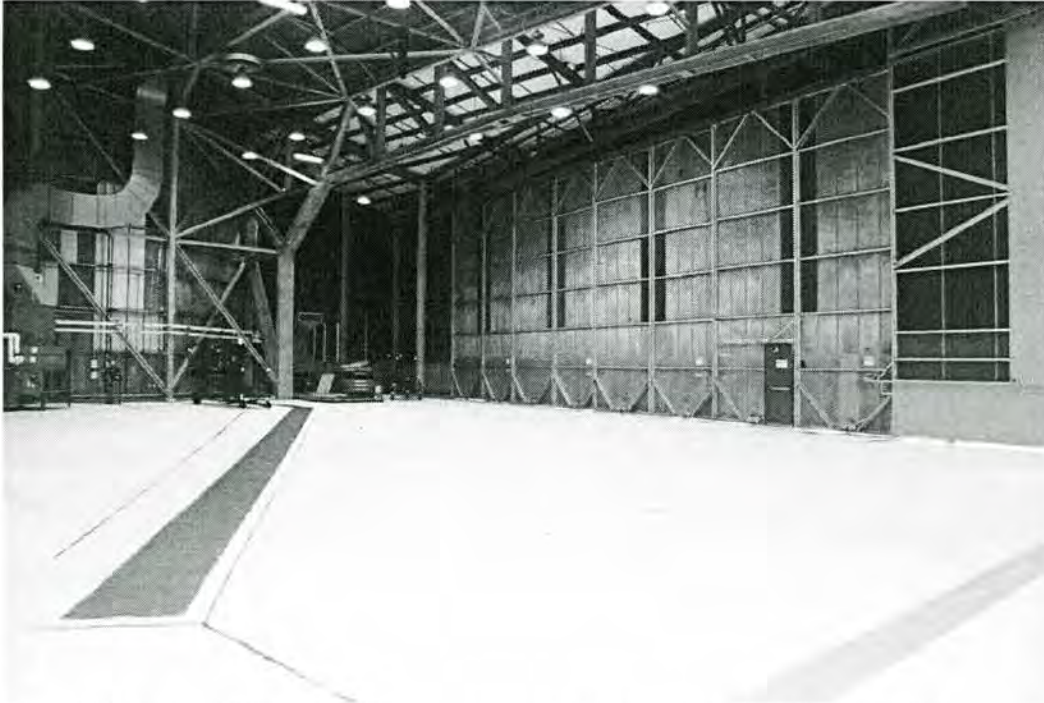
Figure 4-94. Building 4828, interior of bypassing rolling doors (Photograph by Joe C. Freeman, 2004).
