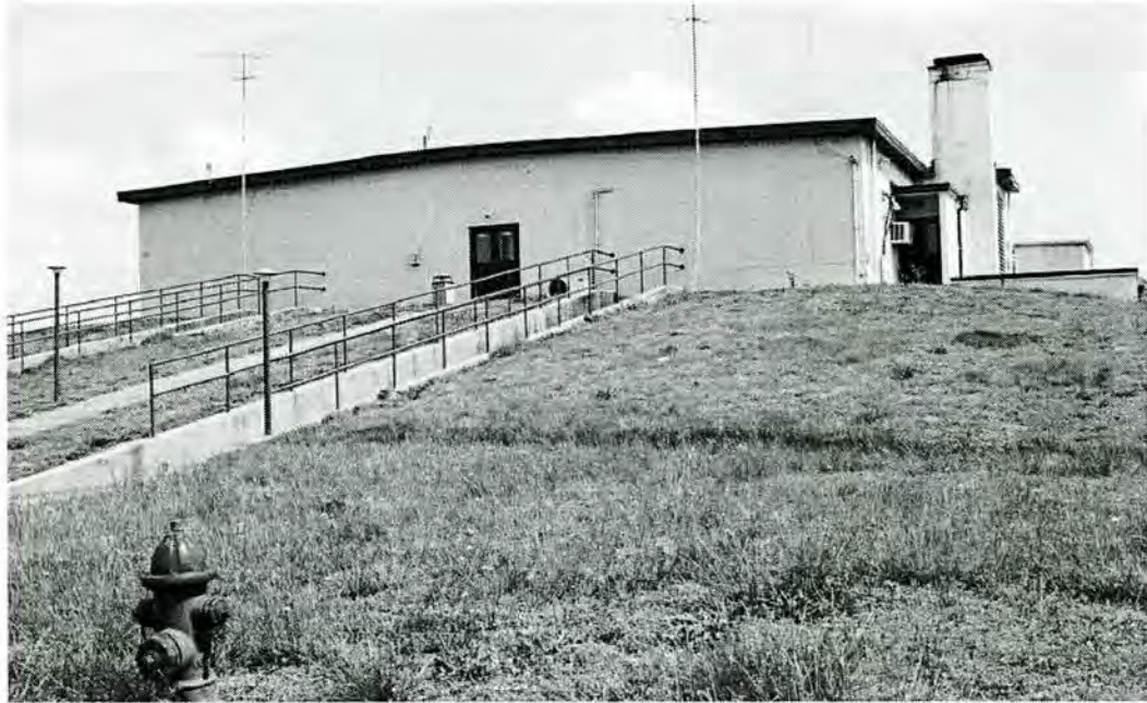
Figure 4-58. Building 2130, facing southwest (Photograph by Joe C. Freeman, 2004).
