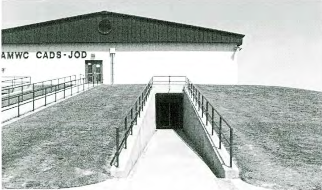
Figure 4-67. 100-man Readiness Crew Building (modified), Little Rock Air Force Base, Arkansas, 2002 (Source: Salo et al. 2002).
