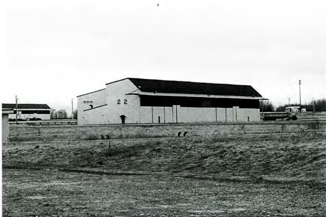
Figure 4-101. Multi-purpose Wing Hangar, front, designed by Luria Engineering, at former Loring Air Force Base, Maine (Scott D. Murdock personal collection © 2004, used with permission).
