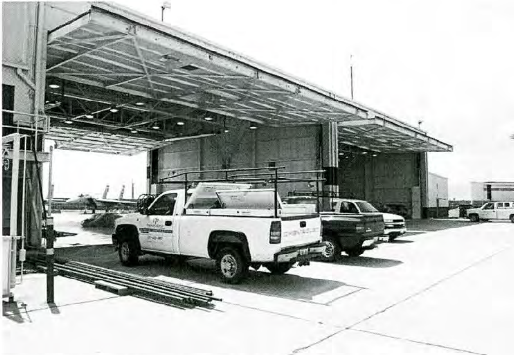
Figure 4-25. Building 5015, facing northwest (Photograph by Joe C. Freeman, 2004).
