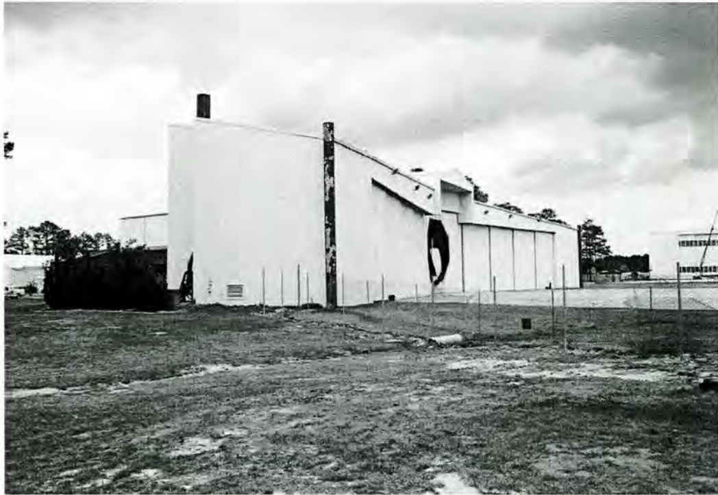
Figure 4-85. Building 4828, facing northeast (Photograph by Joe C. Freeman, 2004).
