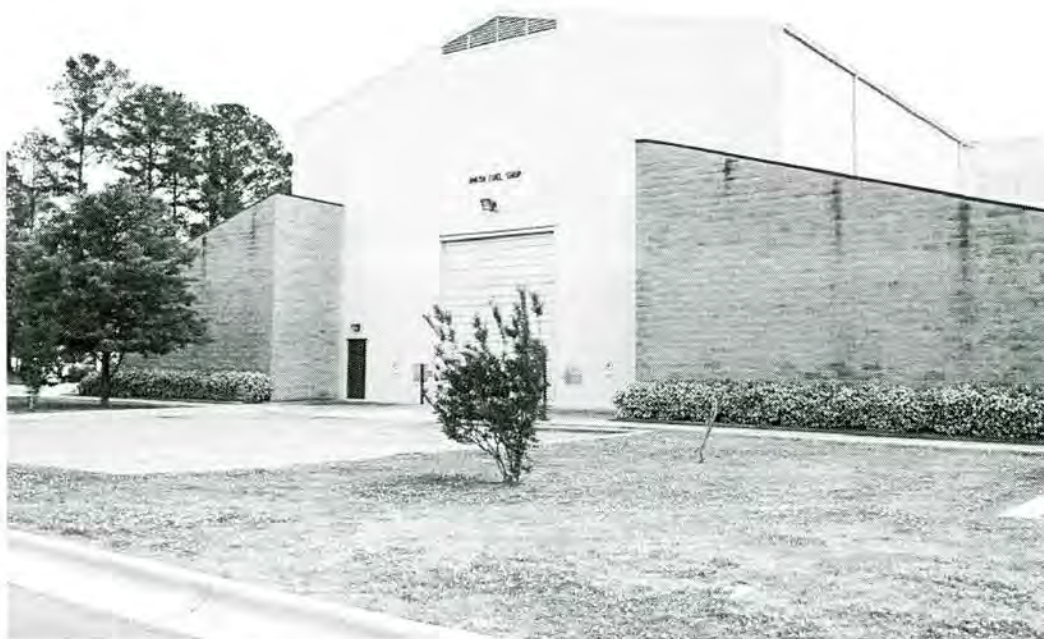
Figure 4-91. Building 4828, facing southeast, showing gable roof addition that replaced original shed roof and concrete block structures (Photograph by Joe C. Freeman, 2004).
