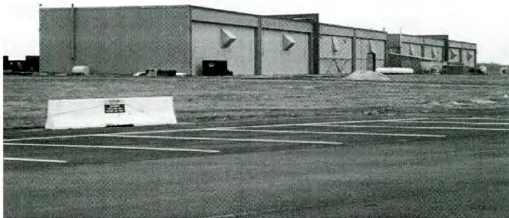
Figure 4-35. Strobel & Salzman Eight Pocket Alert Hangar, Dover Air Force Base, Delaware (Scott D. Murdock personal collection © 1997, used with permission).
