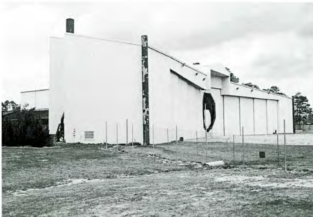
Figure 4-86. Building 4828, facing northeast (Photograph by Joe C. Freeman, 2004).
