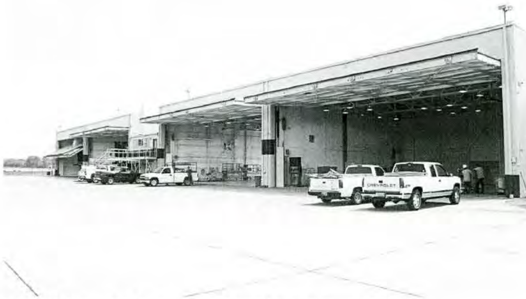
Figure 4-24. Building 5015, facing southeast (Photograph by Joe C. Freeman, 2004).
