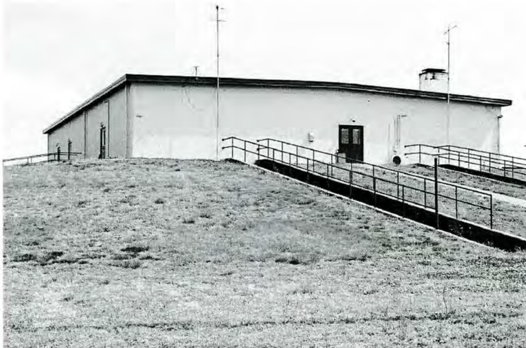
Figure 4-51. Building 2130, facing south (Photograph by Joe C. Freeman, 2004).
