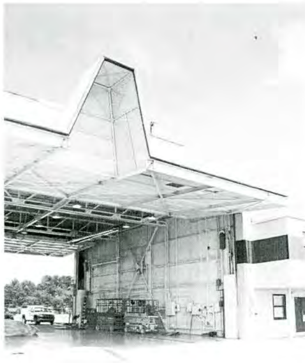
Figure 4-28. Building 5015, facing southeast (Photograph by Joe C. Freeman, 2004).
