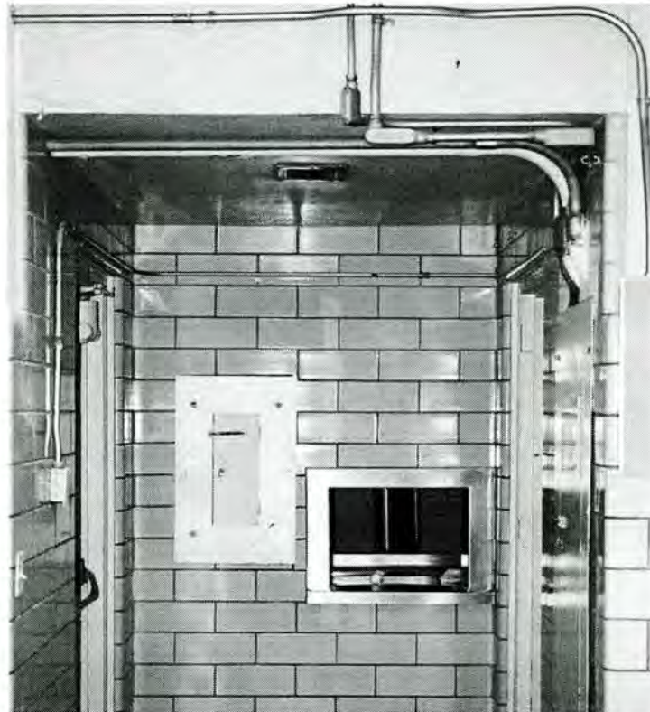
Figure 4-59. Building 2130, interior detail of upper floor (Photograph by Joe C. Freeman, 2004).
