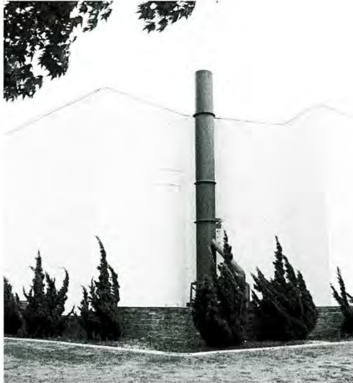
Figure 4-88. Building 4828, chimney vent (Photograph by Joe C. Freeman, 2004).
