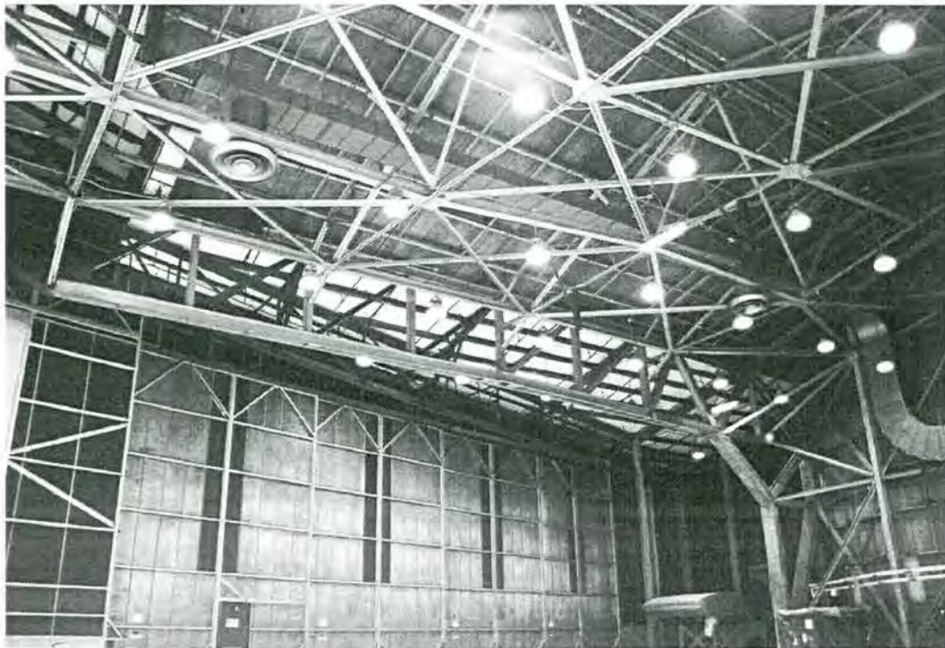
Figure 4-97. Building 4828, truss system (Photograph by Joe C. Freeman, 2004).
