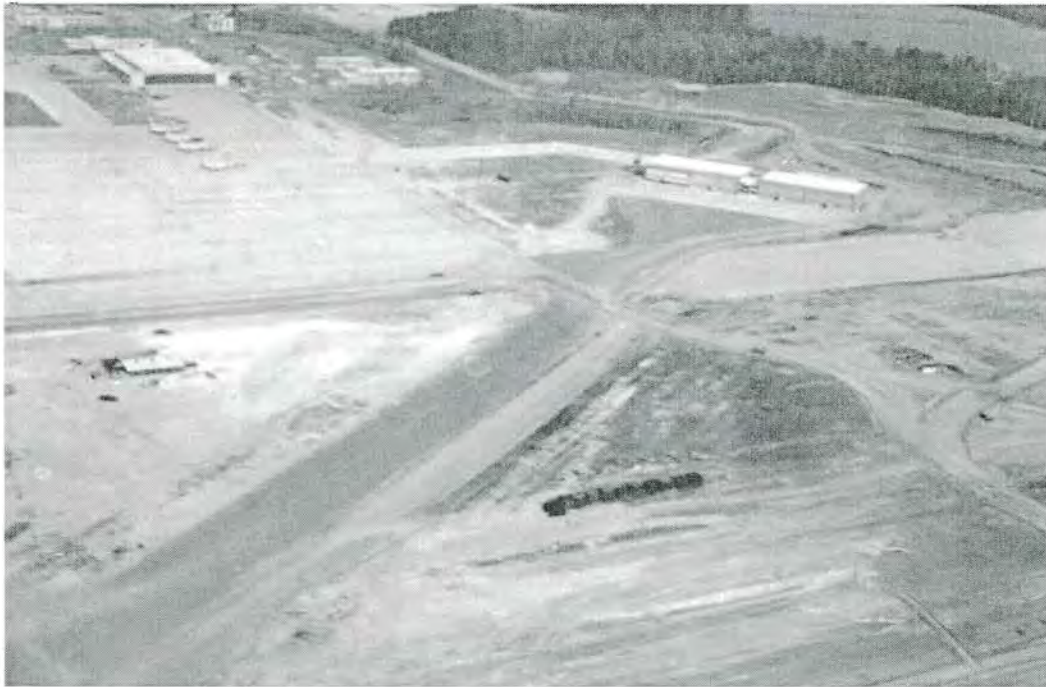
Figure 4-11. Building 5015, December 1958 (Source: 4 th Wing History Office, Seymour Johnson Air Force Base, North Carolina).
