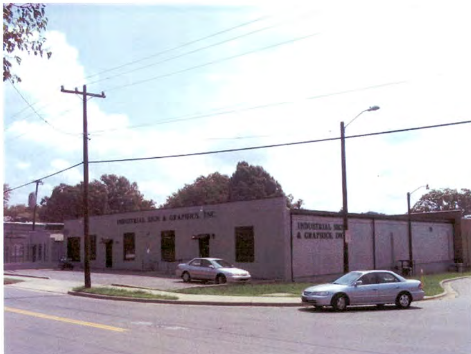
Industrial Building (No. 17).
