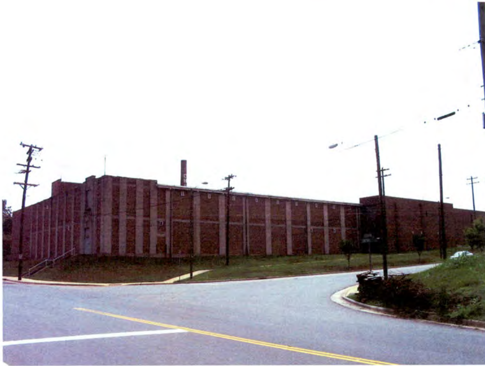
Plate 20. Chadbourn Hosiery Mills, Overall View, Looking Northeast Along North Brevard Street.
