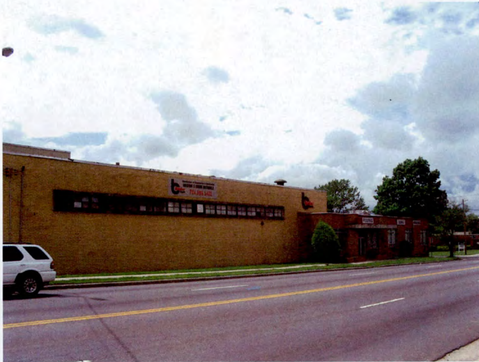
Plate 42. Standard Chemical Products Plant, Overall View, Looking Northwest Across Sugar Creek Road.
