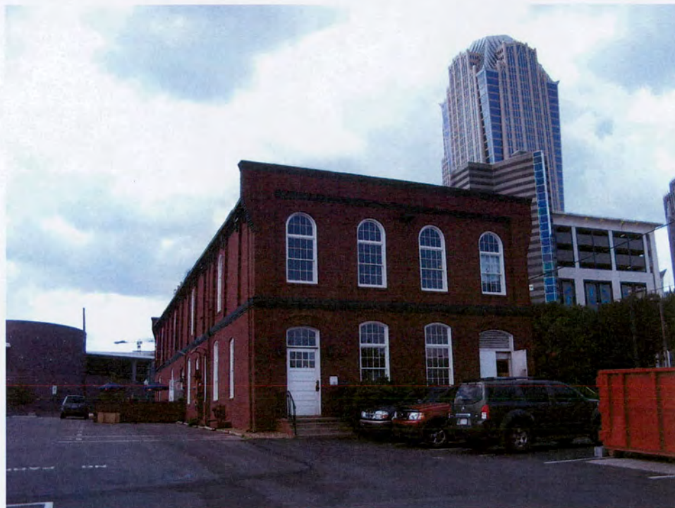
Plate 4. Philip Carey Company Warehouse, Rear (North) Elevation, Looking Southwest.
