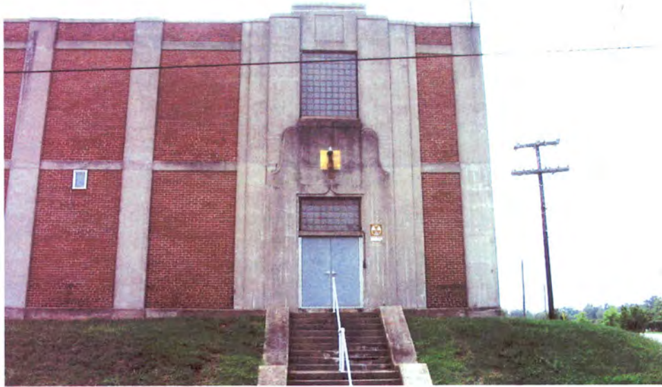
Plate 22. Chadbourn Hosiery Mills, Front (West) Elevation, Entrance.
