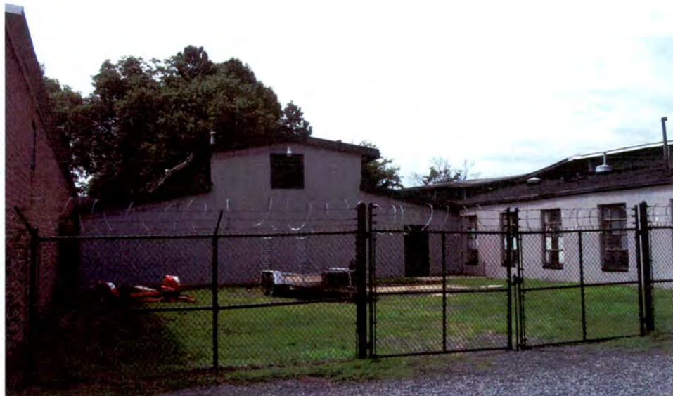
Machine Shop Complex (No. 18).
