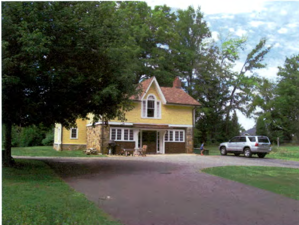
Plate 94. W.T. Alexander House, 1936 Garage/Apartment, Looking Northwest.
