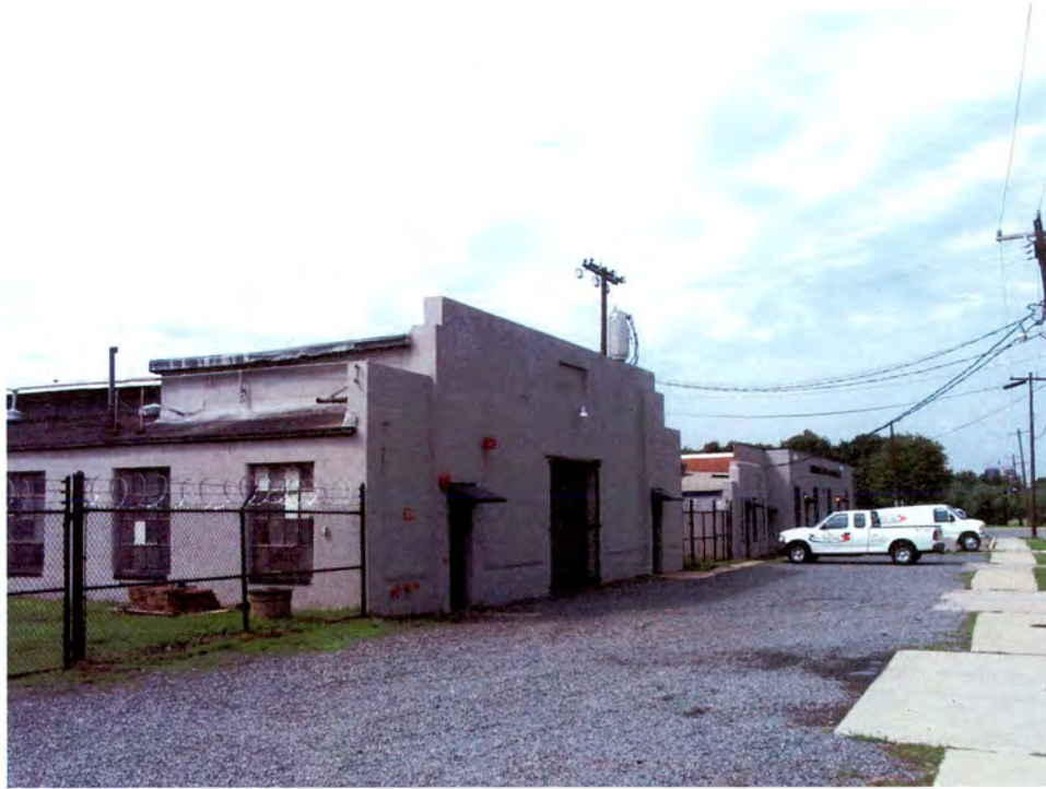
Machine Shop Complex (No. 18).
