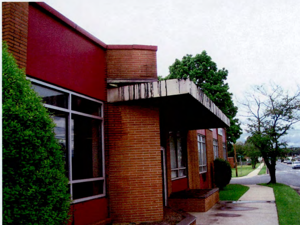
Plate 43. Standard Chemical Products Plant, Office, Front (East) Elevation, Looking North.
