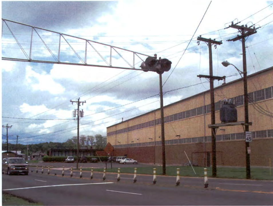
Plate 52. Republic Steel Corporation Plant, Overall View, Looking North From Railroad Corridor.
