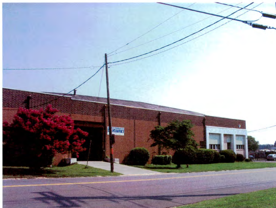
Industrial Building (No. 59).
