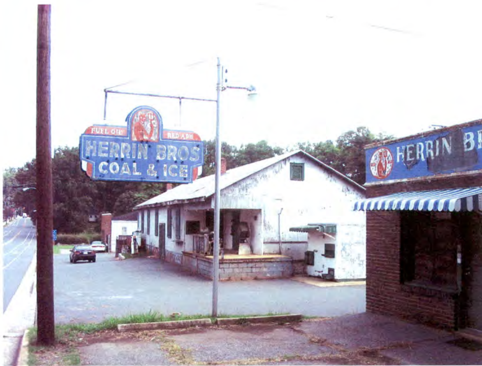
Plate 36. Herrin Brothers Coal and Ice Company Complex, Office (Right Foreground) and Ice House (Center), Looking North Along East 36 th Street.
