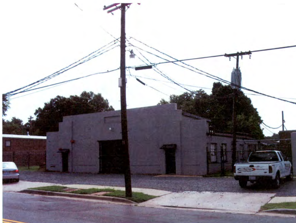
Machine Shop Complex (No. 18).
