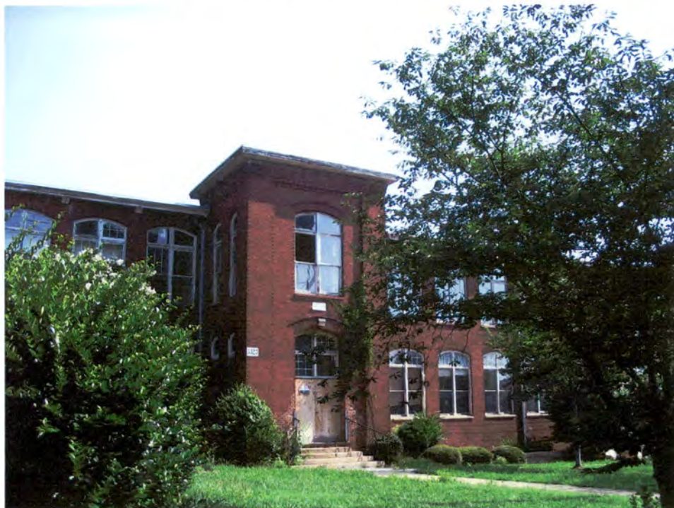
Plate 32. North Charlotte Historic District, Mecklenburg Mill, Looking North.
