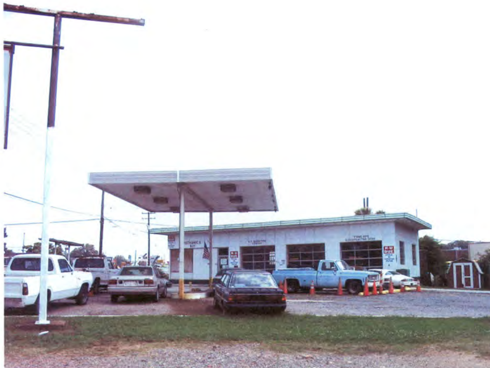
Queen City Texaco Service Station (No. 87).
