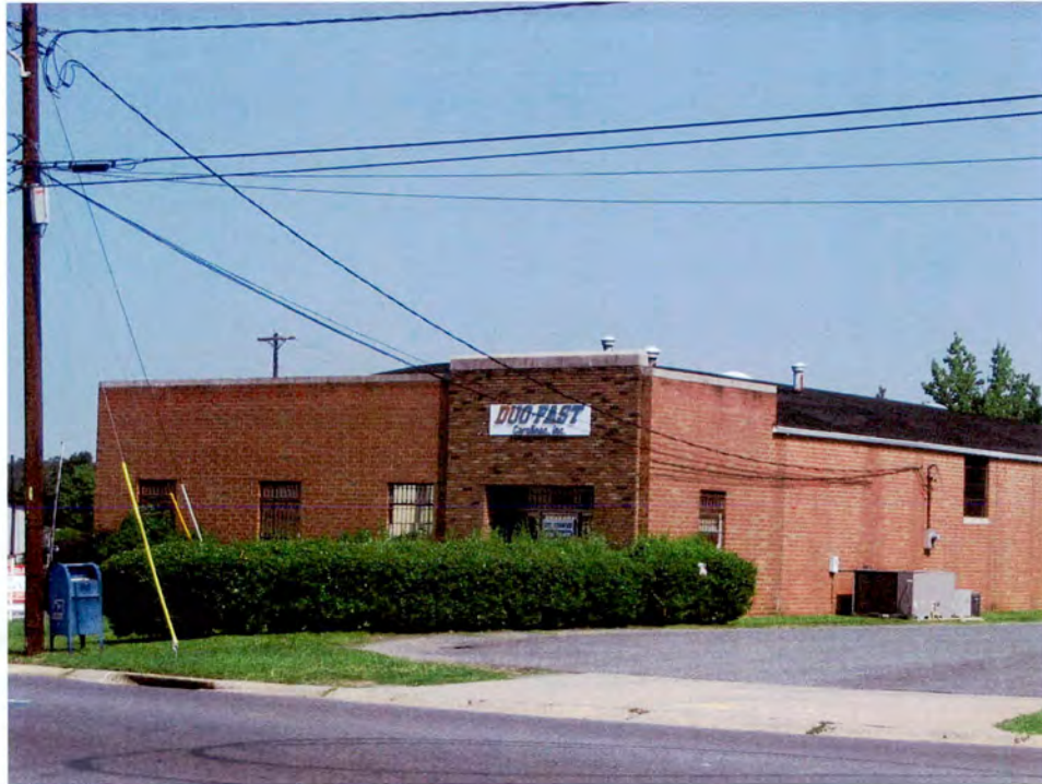
Industrial Building (No. 54).
