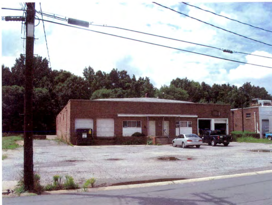
Industrial Building (No. 39).
