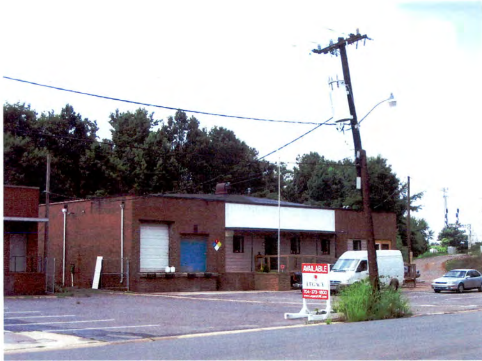
Industrial Building (No. 43).
