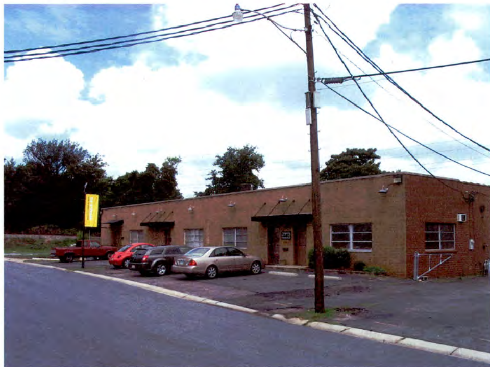
Industrial Building (No. 44).
