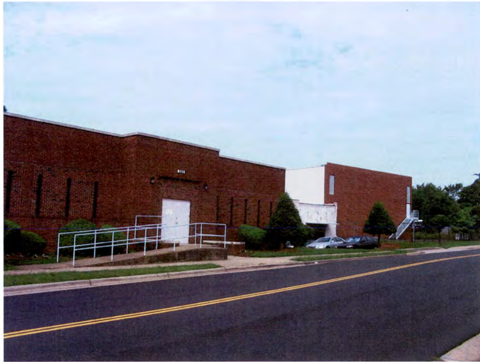
Highland Park Manufacturing Company (No. 7), 16 th Street Elevation.
