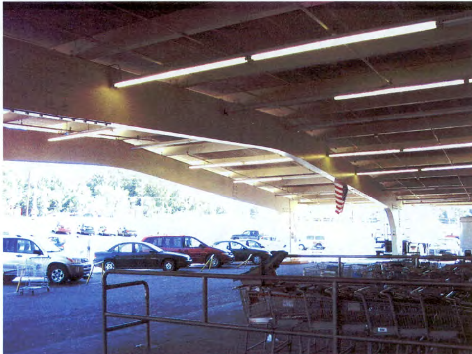
Plate 66. Park-n-Shop Supermart, Porte Cochere, Looking North.
