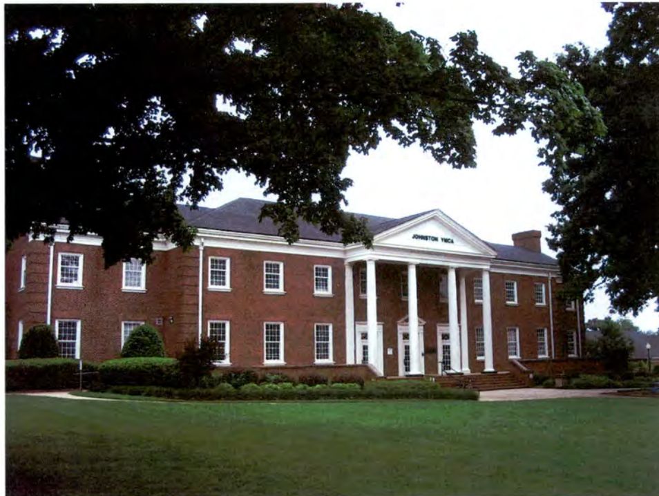
Plate 34. North Charlotte Historic District, Johnston YMCA, Looking North From North Davidson Street.
