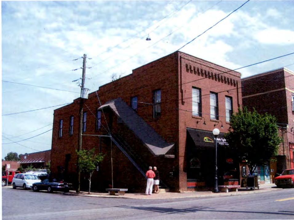
Plate 35. North Charlotte Historic District, Hand Pharmacy and Commercial Buildings on North Davidson Street, Looking North.
