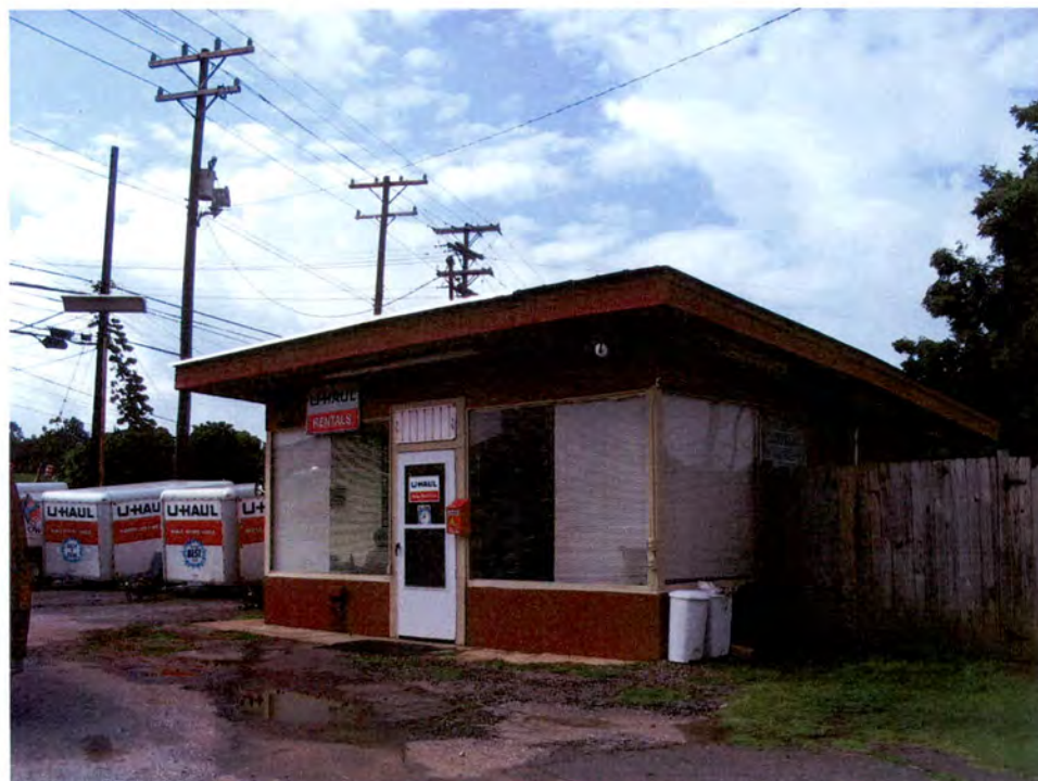
J-R Gas Station (No. 97).
