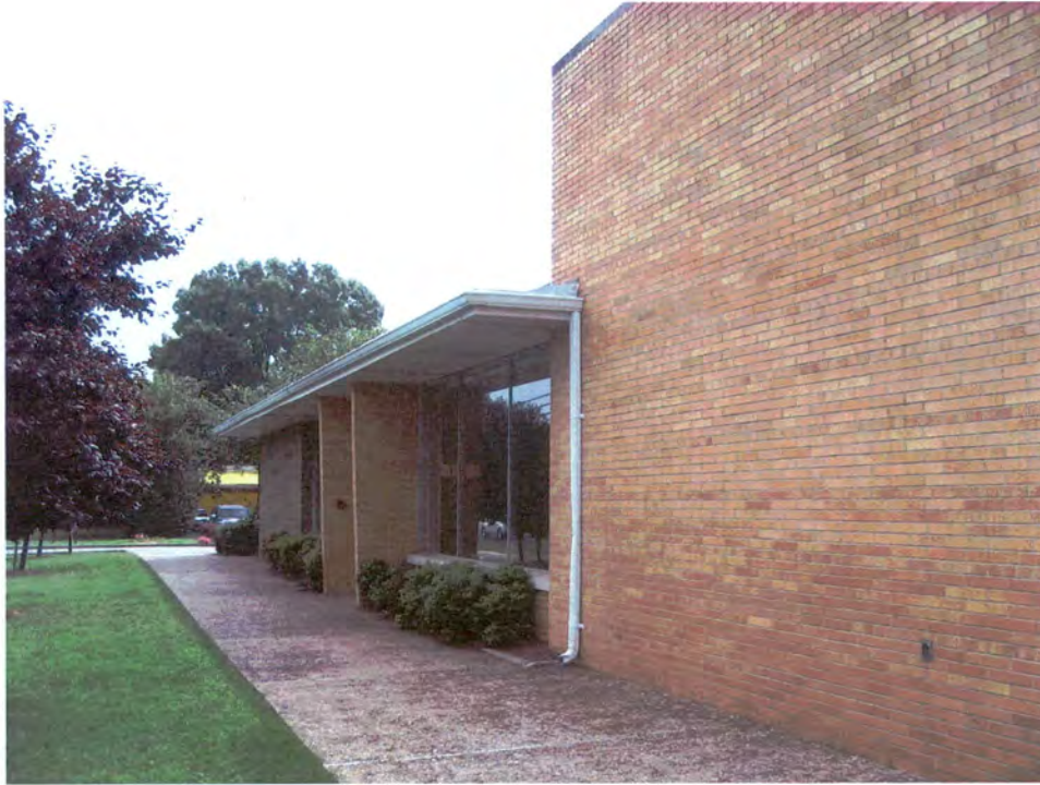
Plate 82. General Motors Corporation Training Center, Office and Auditorium, Façade (North Elevation), Looking Northeast.
