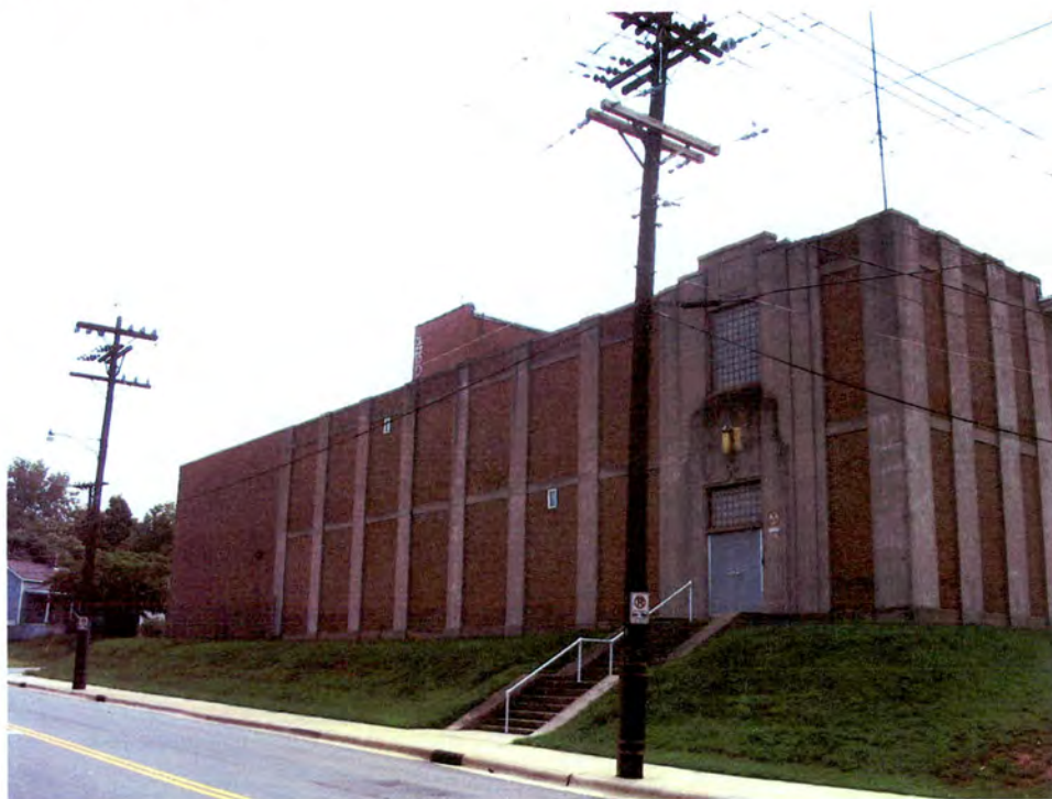
Plate 21. Chadbourn Hosiery Mills, Front (West) Elevation, Looking Northeast From North Brevard Street.
