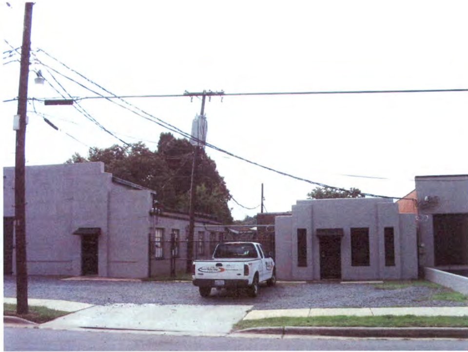
Machine Shop Complex (No. 18).
