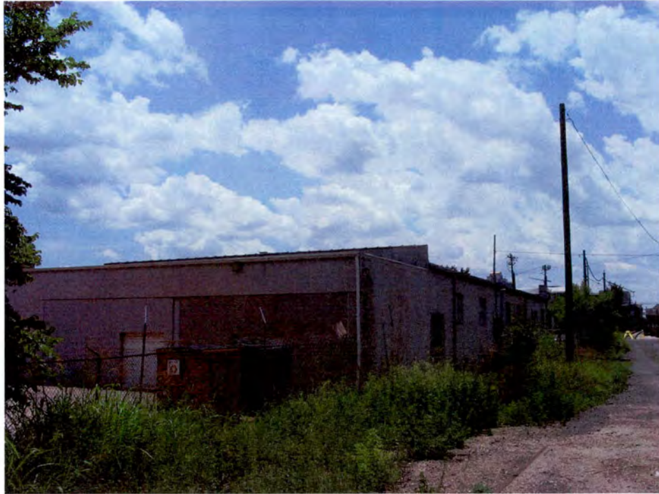
Warehouse (No. 3), Rear Elevation.
