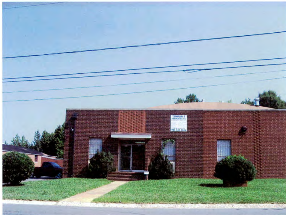
Industrial Building (No. 55).
