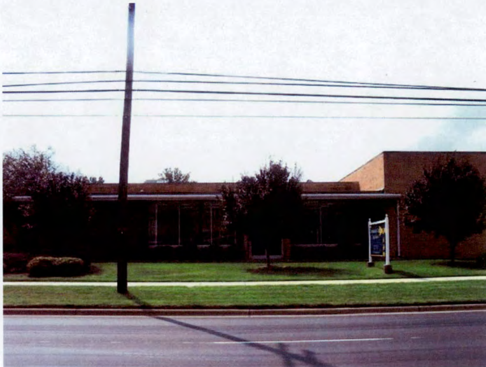
Plate 81. General Motors Corporation Training Center, Overall View, Office Façade (North Elevation), Looking Southeast.
