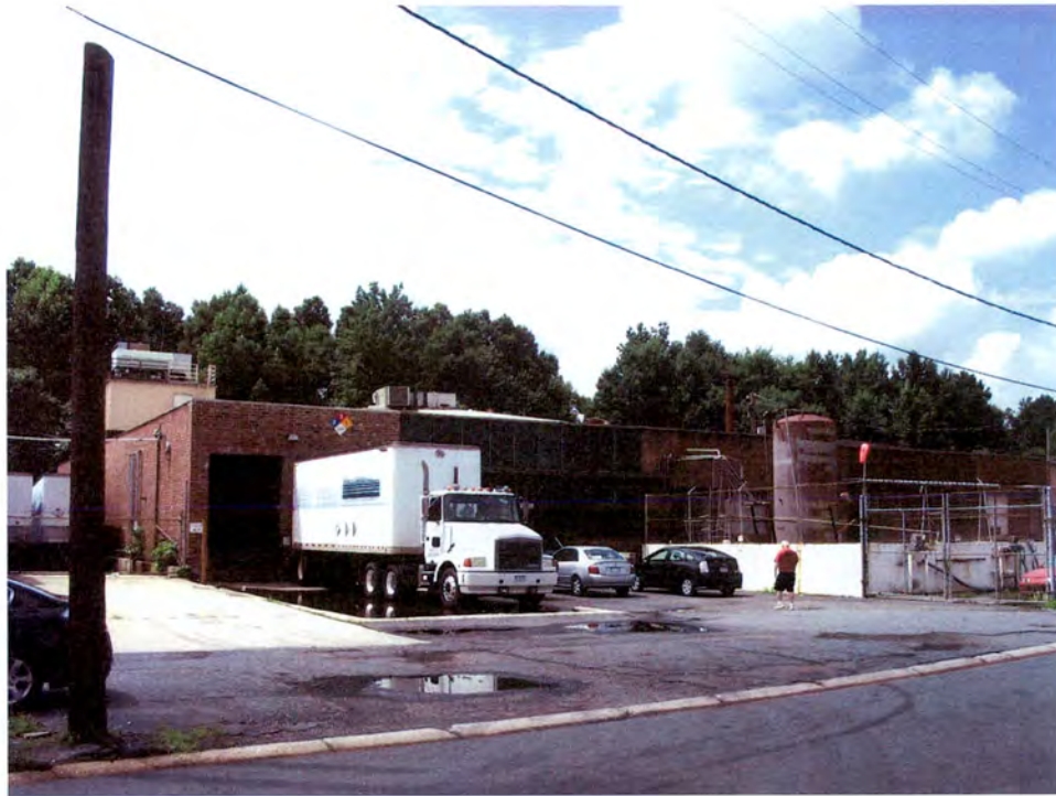
Industrial Building (No. 41).
