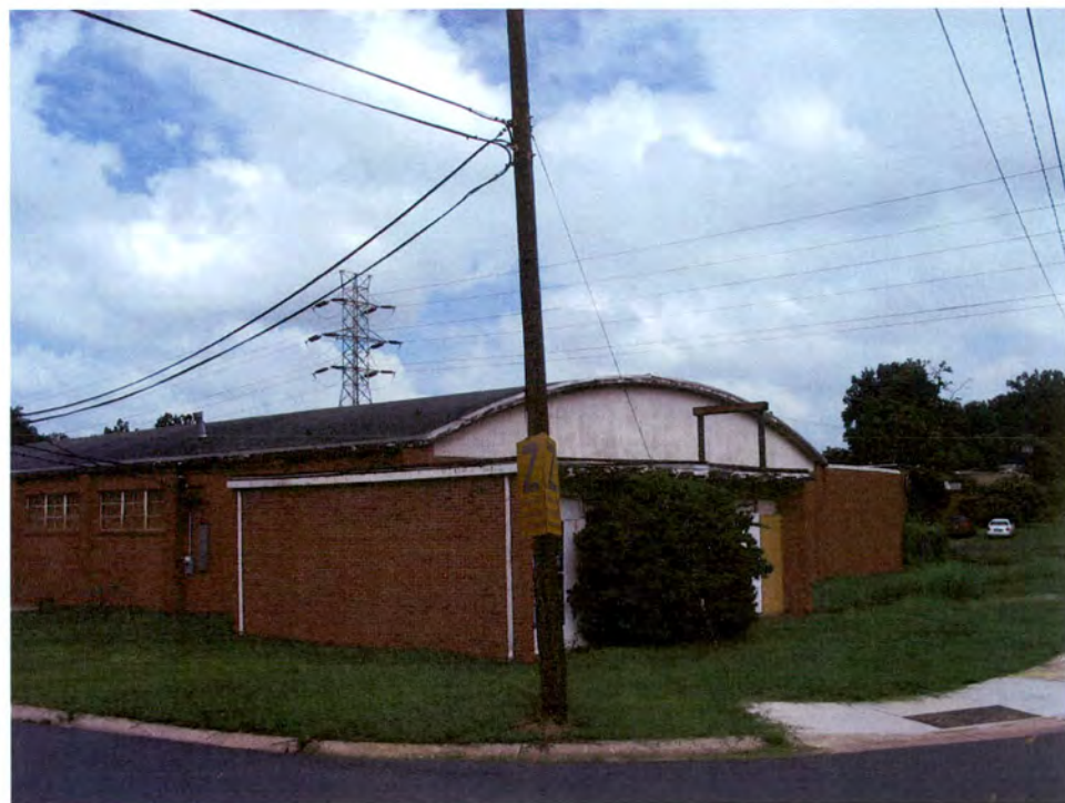
Industrial Building (No. 48).
