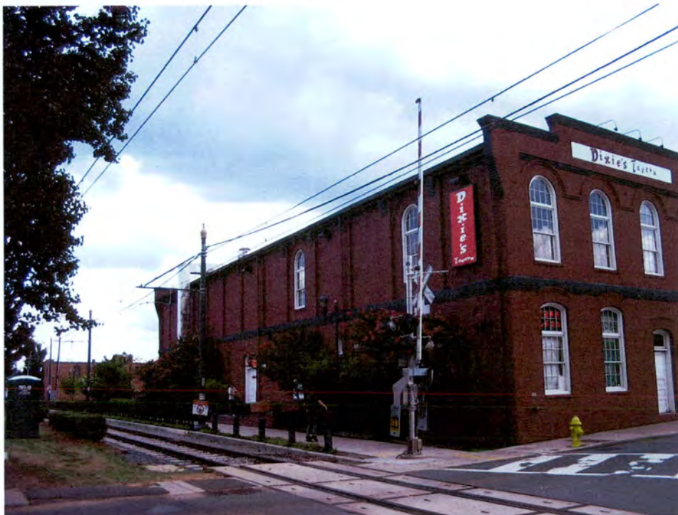
Plate 2. Philip Carey Company Warehouse, Façade and Side (West) Elevation, Looking Northeast Across Existing LYNX Blue Line.
