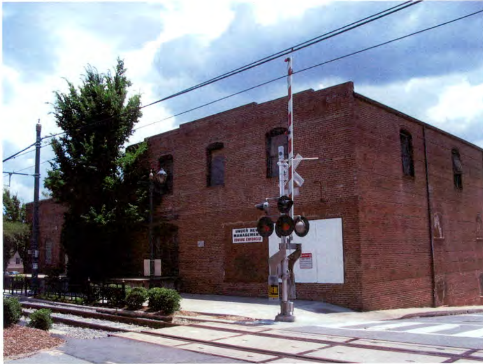
Plate 7. McNeil Paper Company Warehouse Complex, 301-303 East 8 th Street, Façade (West Elevation), Looking East Across Existing LYNX Blue Line.
