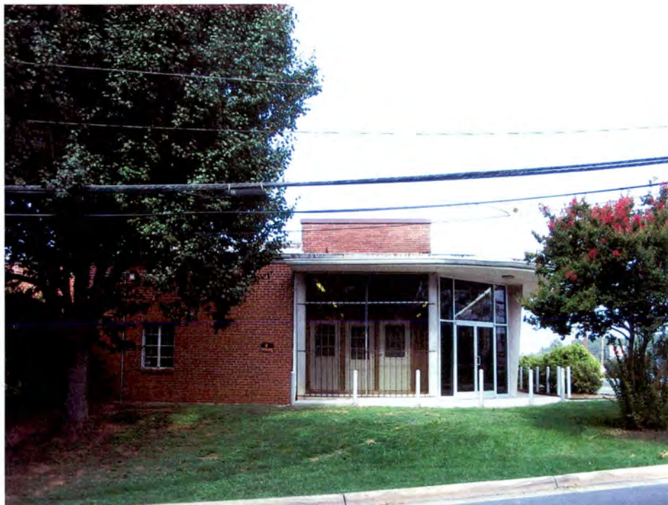
Mobile Home Supply Company Building (No. 75).
