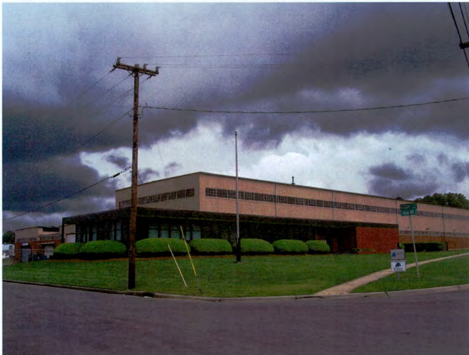
Plate 53. Republic Steel Corporation Plant, Office and Warehouse, Looking Southeast From Sugar Creek Road.
