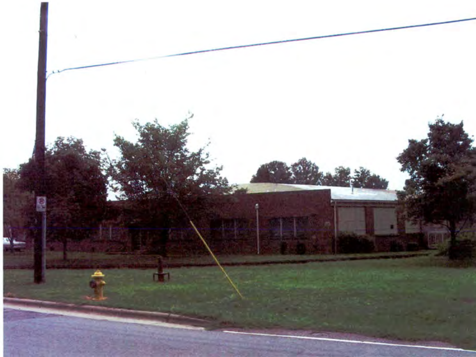
Industrial Building (No. 30).
