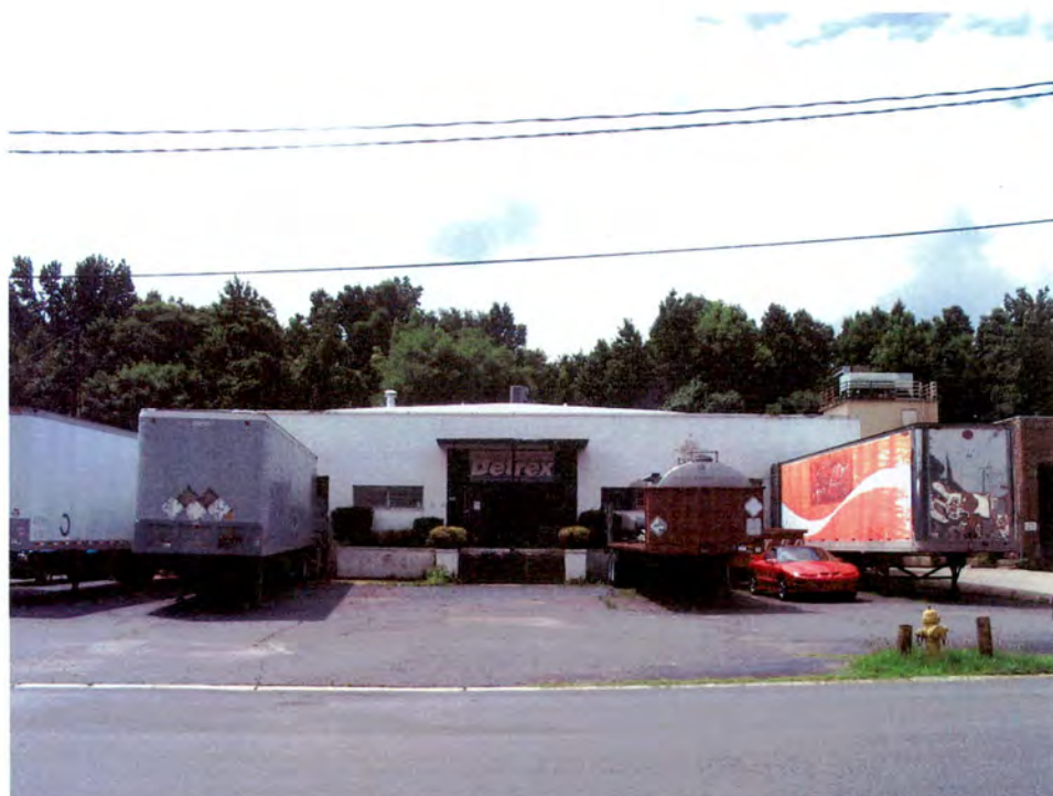
Industrial Building (No. 40).
