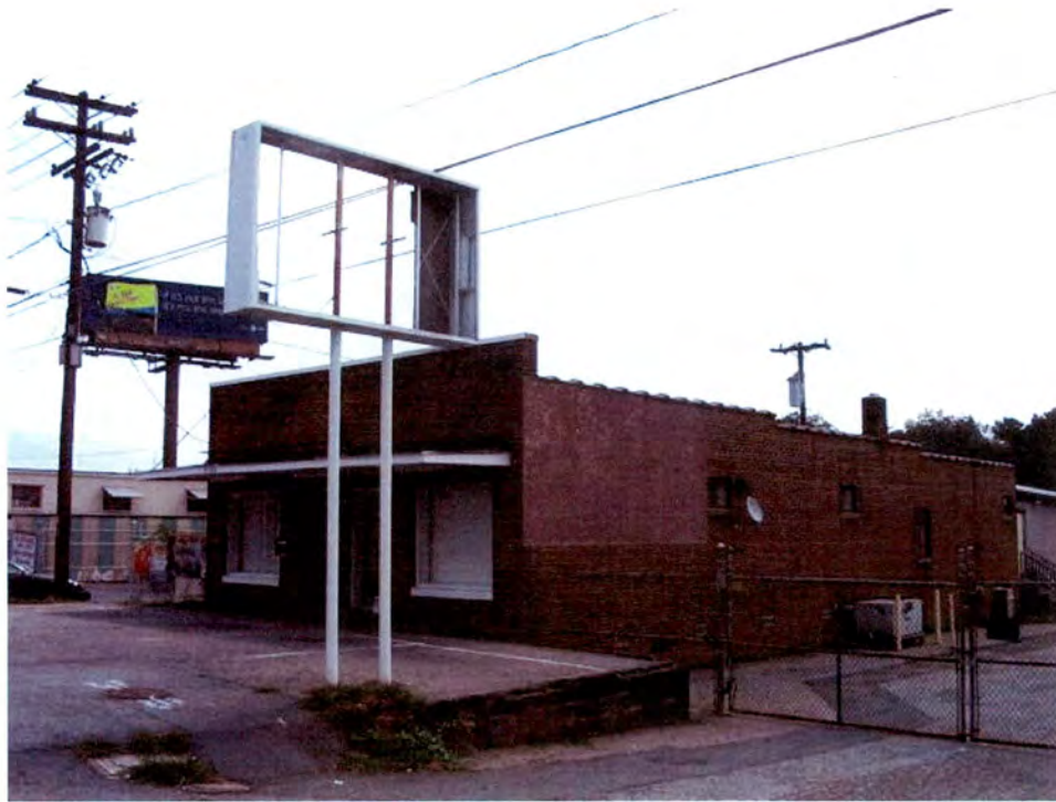
Commercial Building (No. 90).
