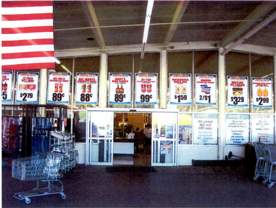
Plate 65. Park-n-Shop Supermart, Front (North) Elevation, Main Entrance.
