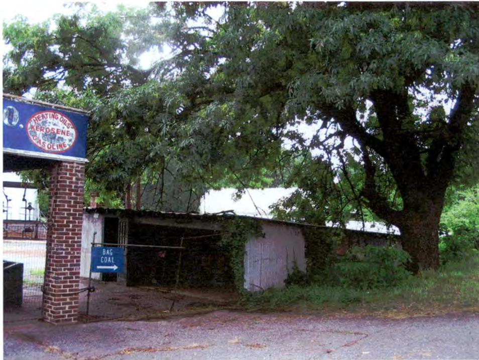
Plate 40. Herrin Brothers Coal and Ice Company Complex, Shed, Looking Southeast.
