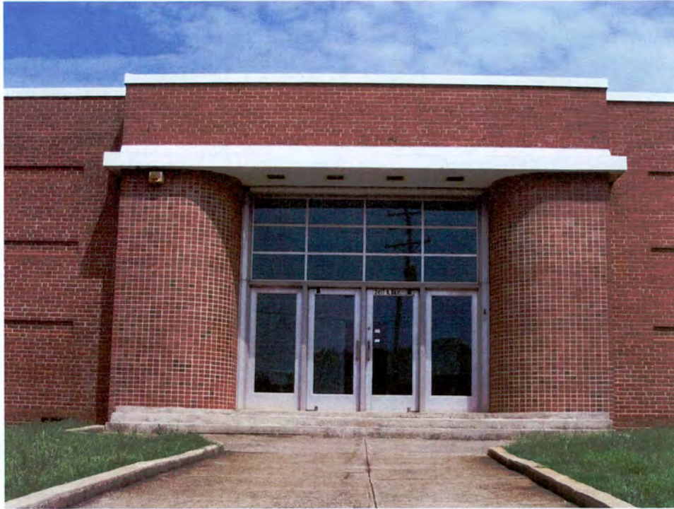
Plate 26. Chadbourn Hosiery Mills, East Elevation, Entrance Detail.
