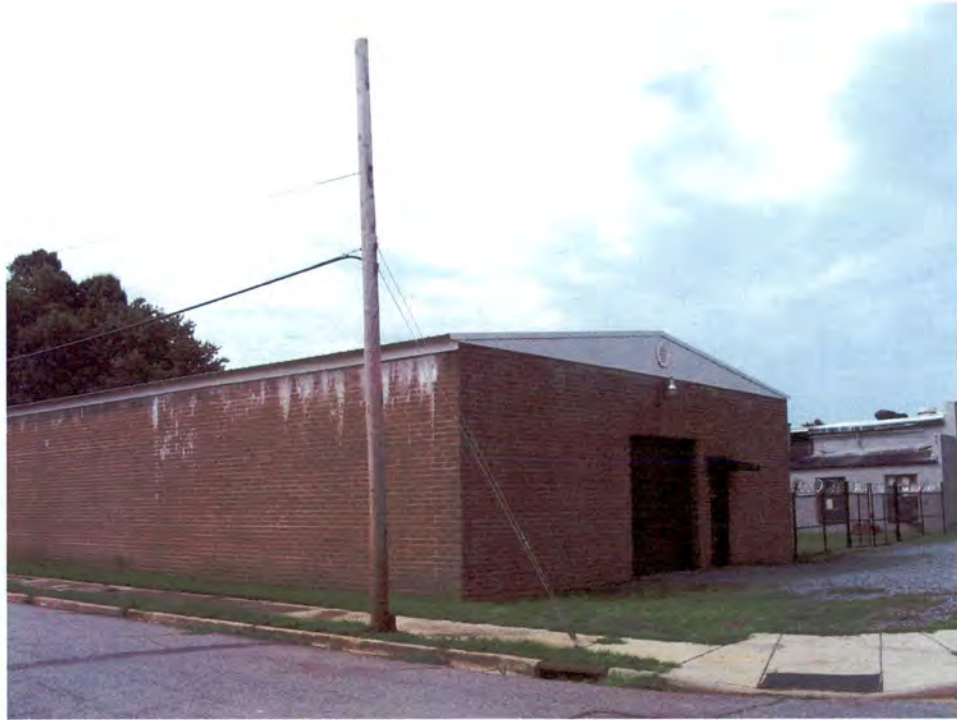
Machine Shop Complex (No. 18), 1960s Warehouse.
