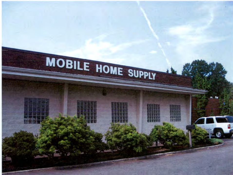
Mobile Home Supply Company Building (No. 75), Storefront Windows Infilled with Concrete Block and Glass Block.
