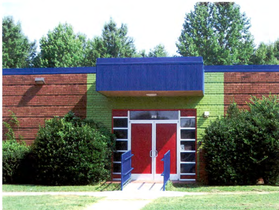
Industrial Building (No. 56), Entrance Detail.
