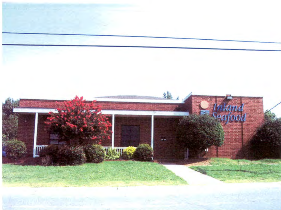
Industrial Building (No. 57), Front Elevation.
