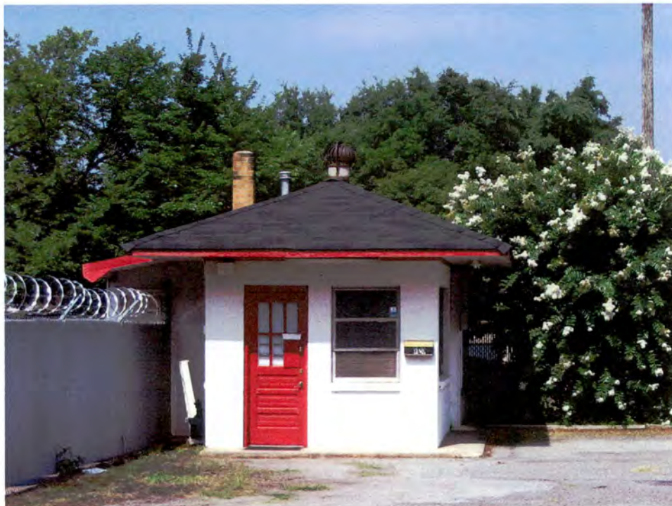
Plate 75. Elmore Trailer Sales and Trailer Park, Sales Office, Looking West.
