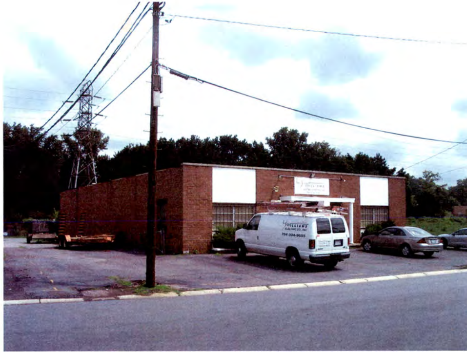
Industrial Building (No. 45).
