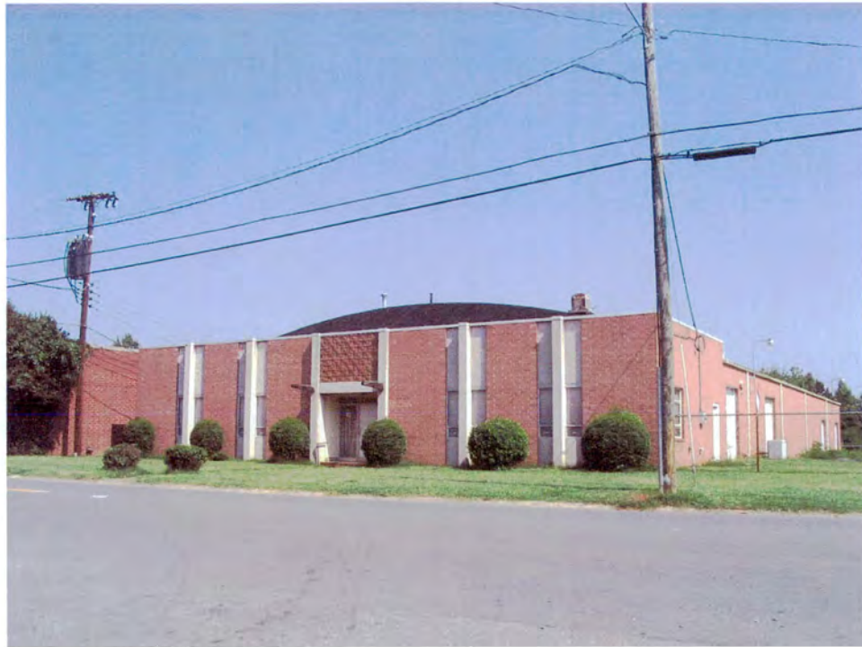
Industrial Building (No. 58).
