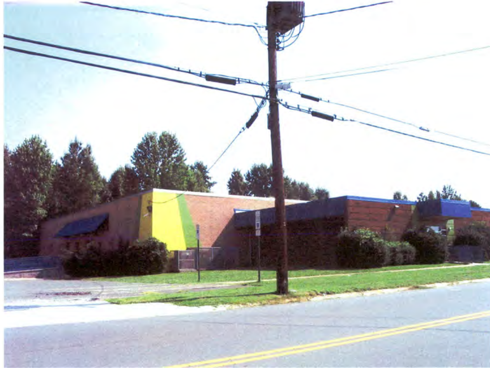
Industrial Building (No. 56).
