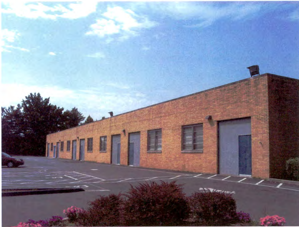
Plate 84. General Motors Corporation Training Center, Classroom Wing, East Elevation, Looking Southwest.
