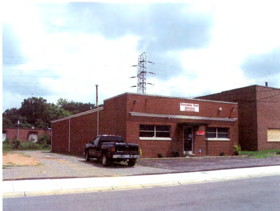
Industrial Building (No. 46).
