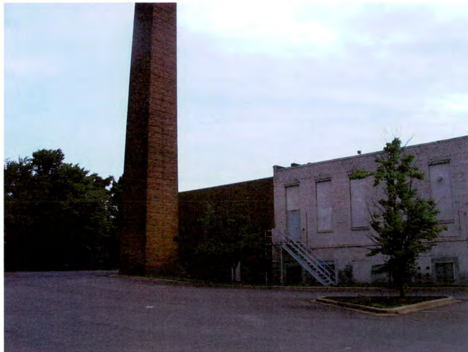
Highland Park Manufacturing Company (No. 7), Smokestack and Sections of Original South Elevation.
