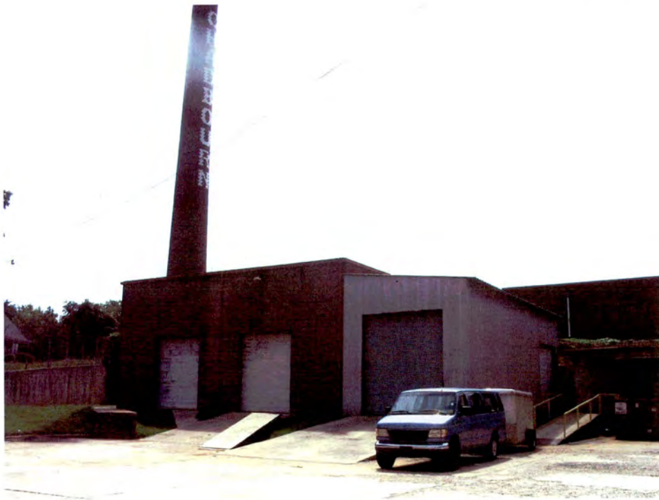
Plate 24. Chadbourn Hosiery Mills, Boiler House and Chimney Stack, Looking East.
