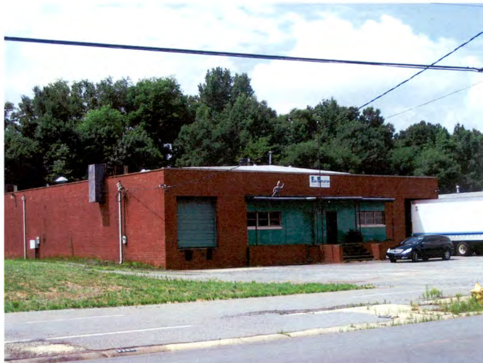
Industrial Building (No. 38).
