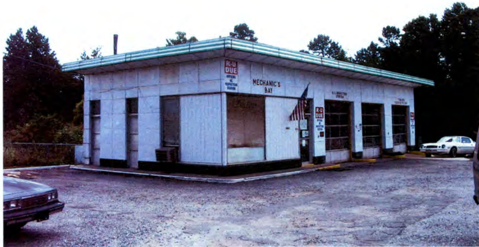
Queen City Texaco Service Station (No. 87).
