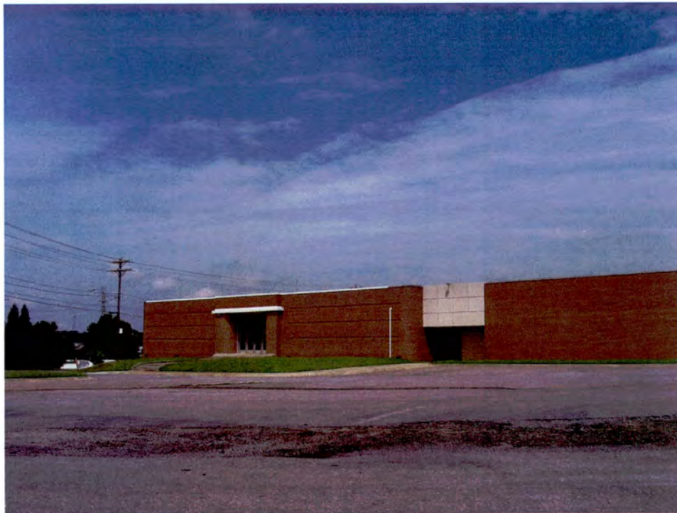
Plate 25. Chadbourn Hosiery Mills, 1947 Mill, Rear (East) Elevation, and ca. 1960 Addition (on Right), Looking West.
