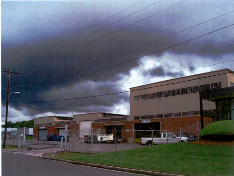
Plate 58. Republic Steel Corporation Plant, Fabricating and Warehousing Units, North Elevations, Looking Southeast.
