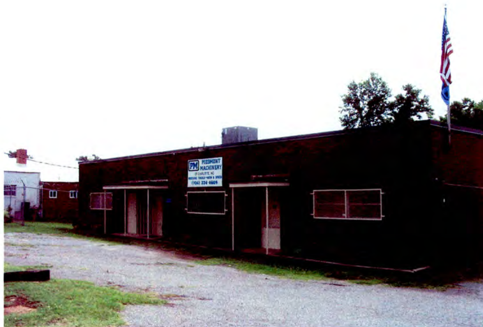
Machine Shop Complex (No. 28).
