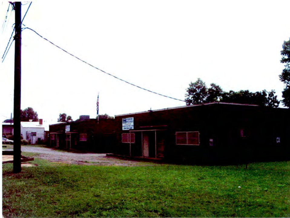
Machine Shop Complex (No. 28).
