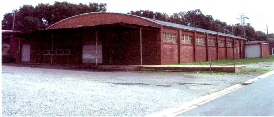
Industrial Building (No. 48), Rear (West) and Side (South) Elevations.
