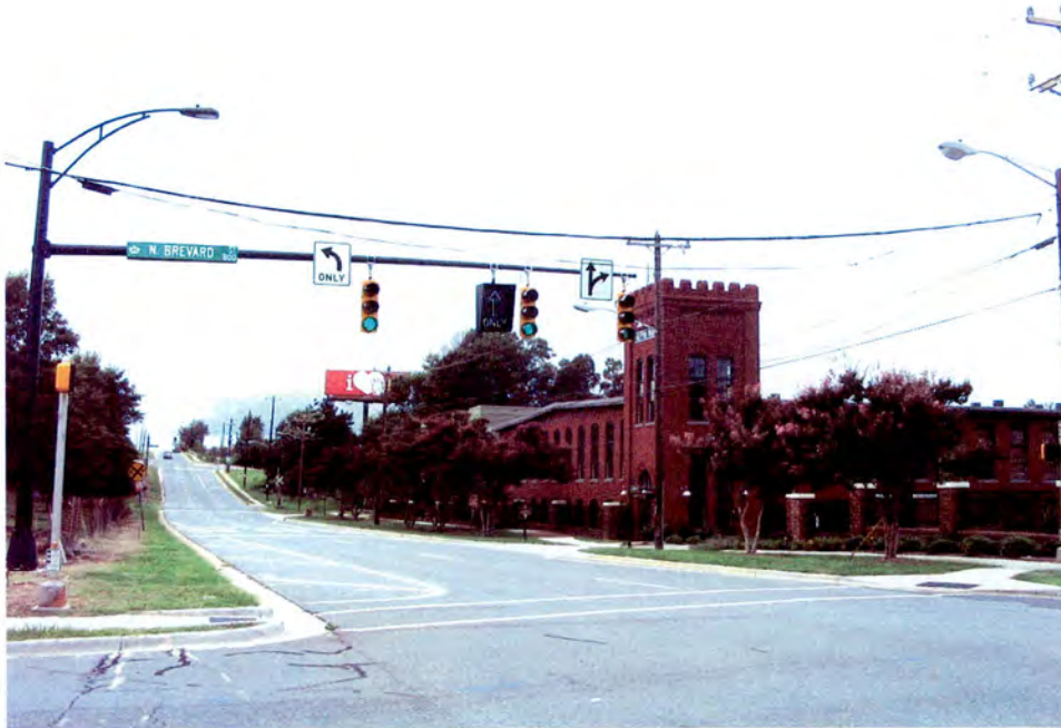
Plate 13. Orient Manufacturing Company/Chadwick-Hoskins No. 3, Overall View Looking Northwest Along East 12 th Street.
