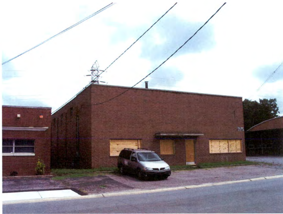
Industrial Building (No. 47).
