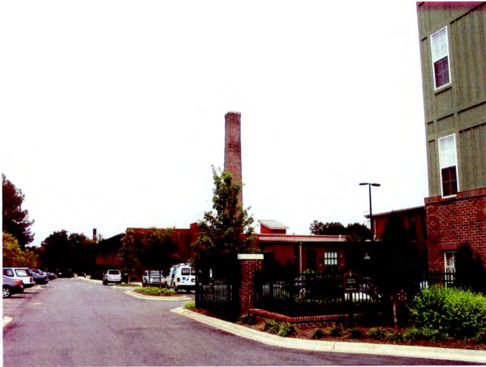
Plate 16. Orient Manufacturing Company/Chadwick-Hoskins No. 3, ca. 1911 Weaving Building (in Background) and Modern Apartment Building (Right Foreground), Looking Northeast From East 12 th Street.
