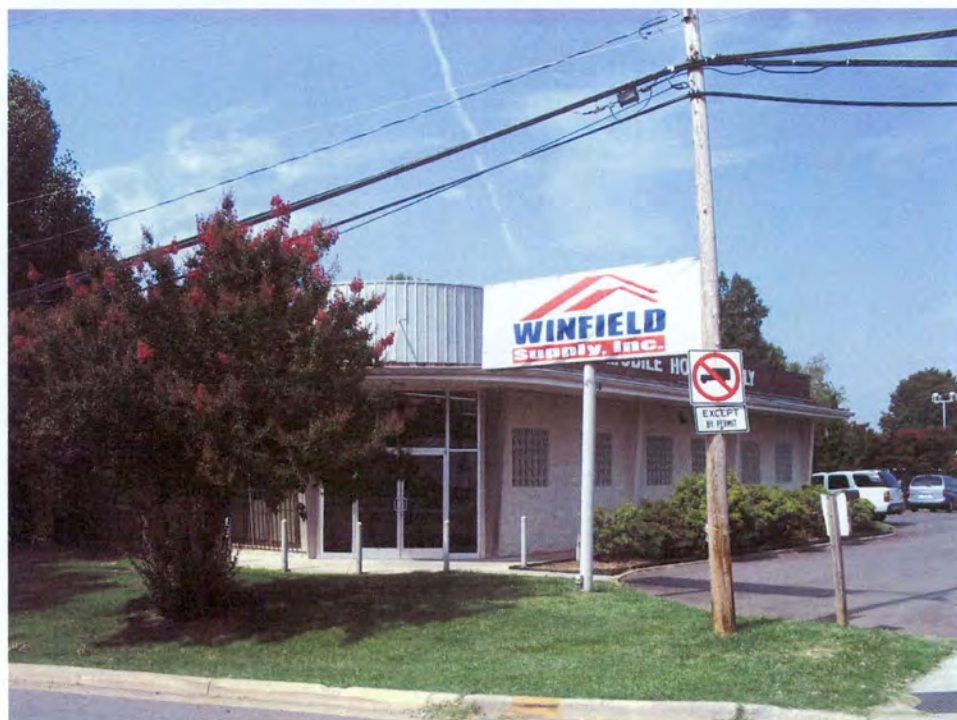
Mobile Home Supply Company Building (No. 75).
