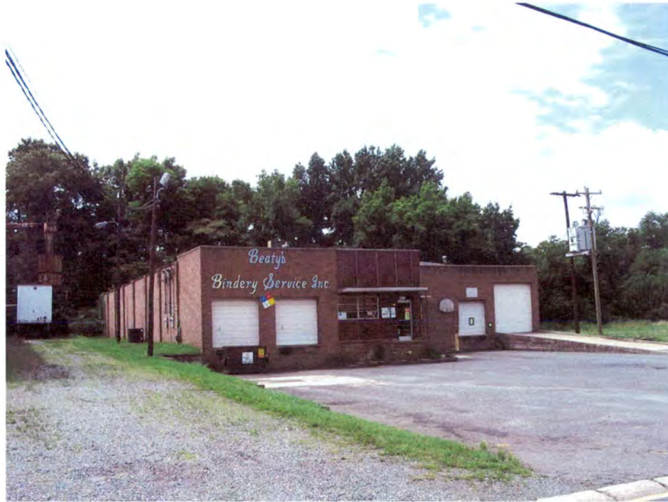
Industrial Building (No. 37).
