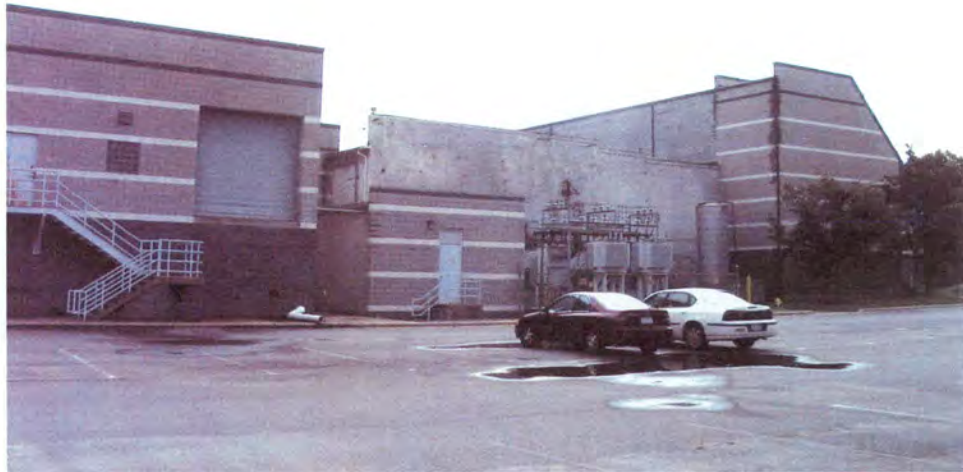
Highland Park Manufacturing Company (No. 7), Altered South Elevation.
