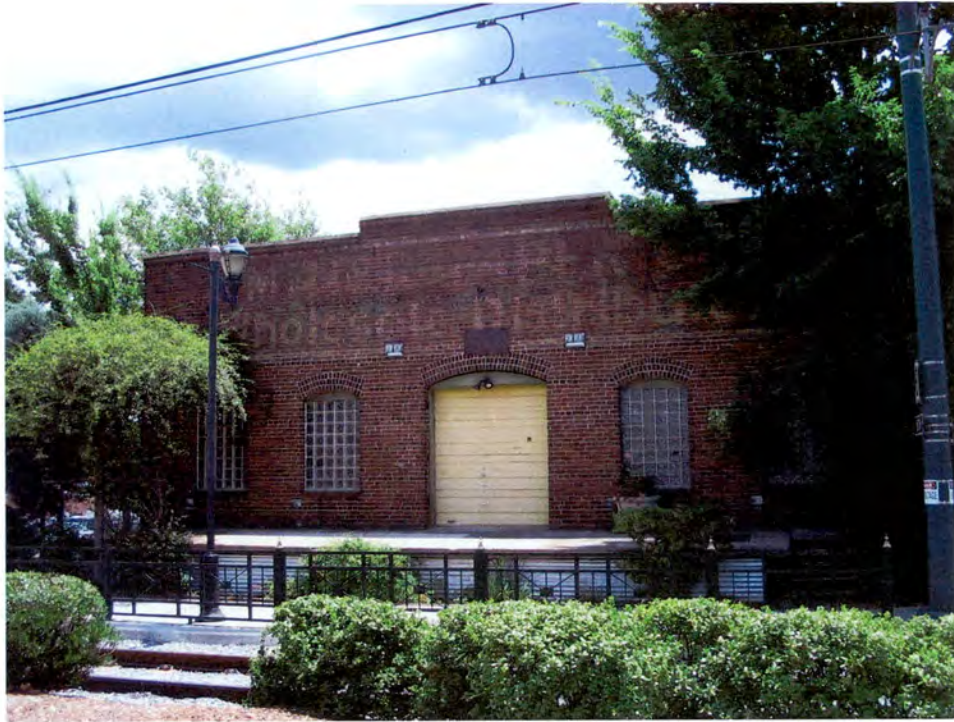
Plate 9. McNeil Paper Company Warehouse Complex, 305-307 East 8 th Street, Façade, Looking East Across Existing LYNX Blue Line.
