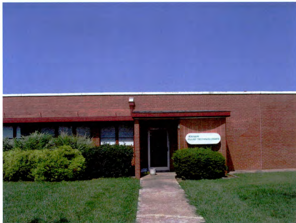
Kaiser Fluid Technologies Company Plant (No. 72), Main Entrance.
