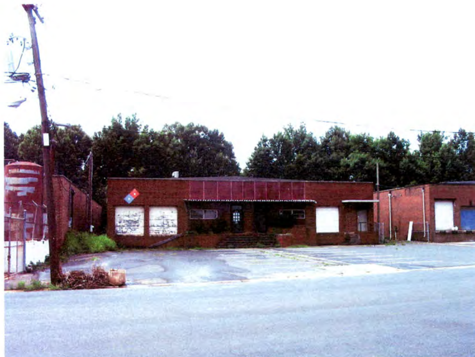
Industrial Building (No. 42).
