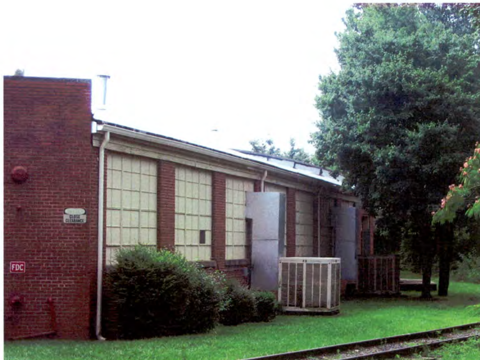
Industrial Building (No. 30), Side (South) Elevation Along Spur Line.
