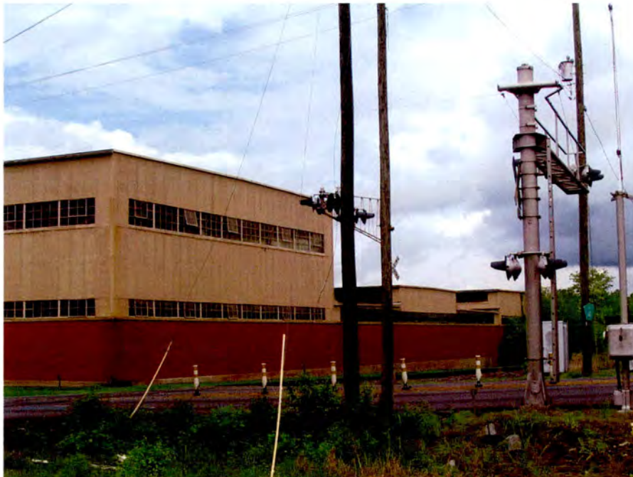
Republic Steel Corporation Plant, Warehouse Sections, East Elevation, Looking Northwest From Railroad.
