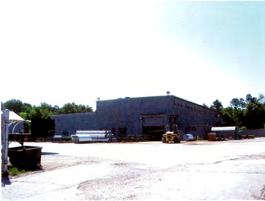
Republic Steel Corporation Plant, Pipe Fabrication Building, West Elevation, Looking East.
