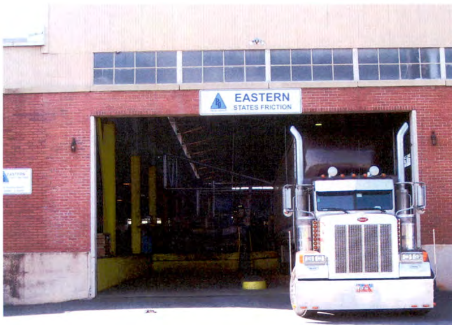
Republic Steel Corporation Plant, Warehouse, West Elevation, Truck Bay.
