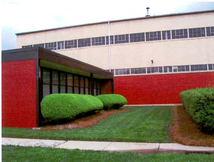
Republic Steel Corporation Plant, Office, East Elevation, Looking North Towards Warehouse.
