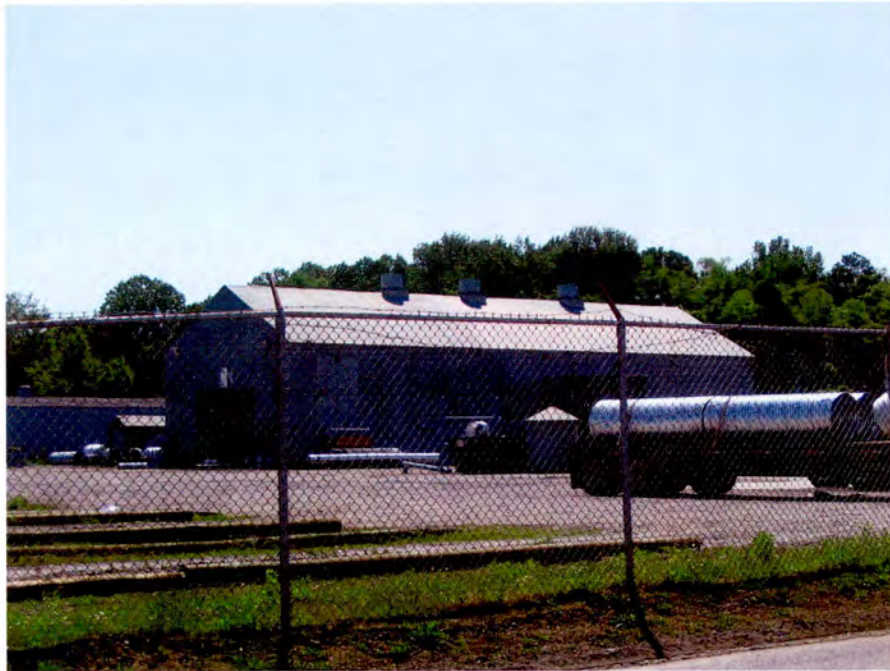
Republic Steel Corporation Plant, Pipe Fabrication Building at North End of Tract, Looking North.
