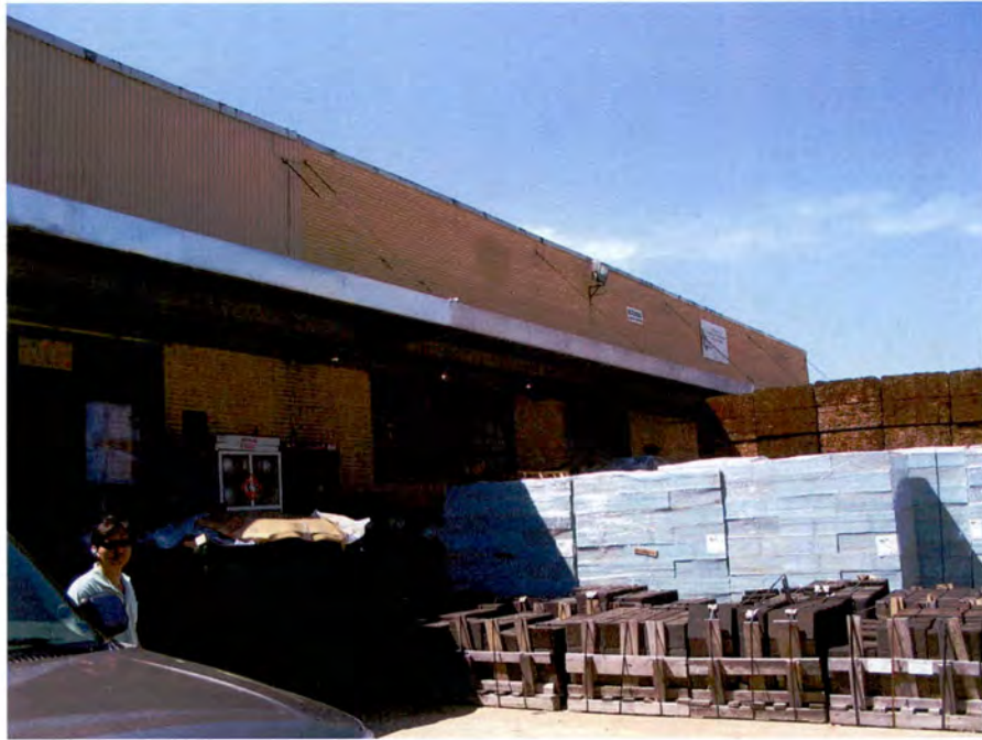
Standard Chemical Products Plant, Rear Warehouse, West Elevation, Looking South.
