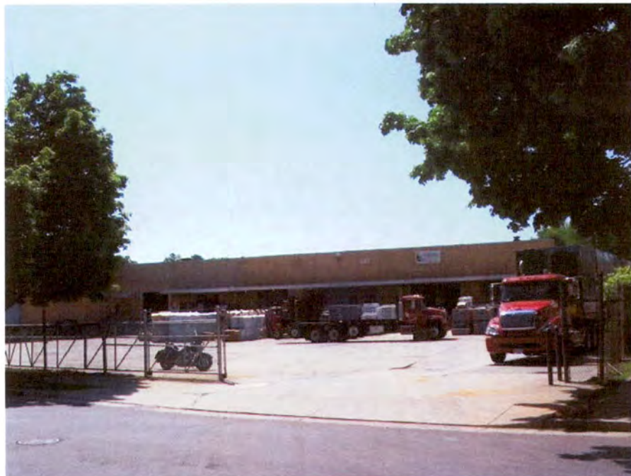
Standard Chemical Products Plant, Rear Warehouse and Loading Docks, Looking East.
