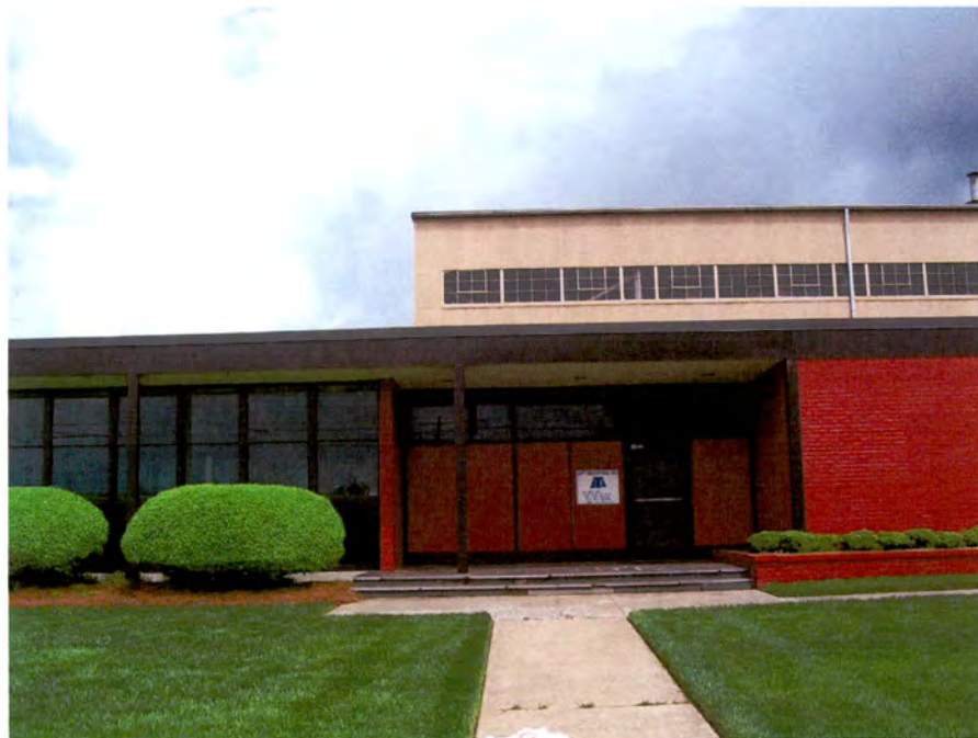
Republic Steel Corporation Plant, Office Entrance, Looking North.
