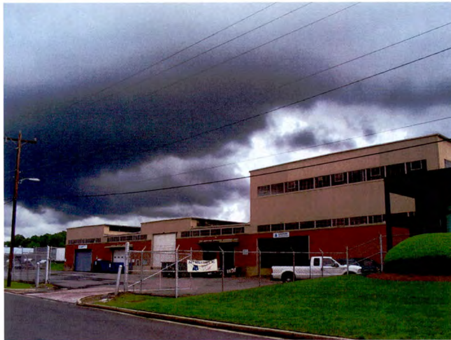
Republic Steel Corporation Plant, Warehouse, West Elevation, Looking East.
