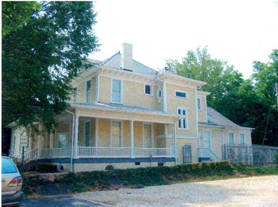
No. 17 R.C. Biberstein House, Side (West) Elevation.
