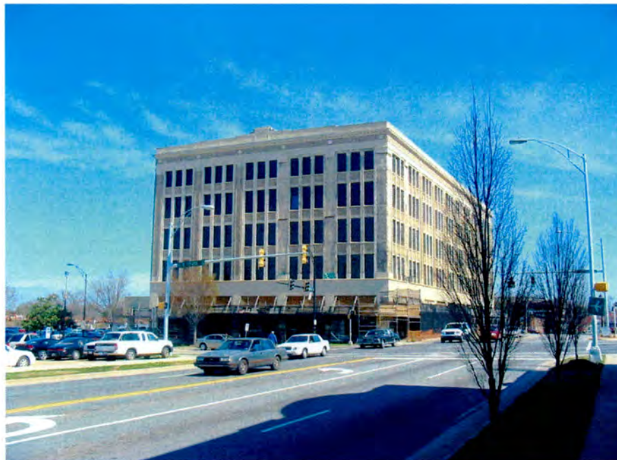
No. 2 Coddington Building (Polk Building), Façade and Side (East) Elevation.
