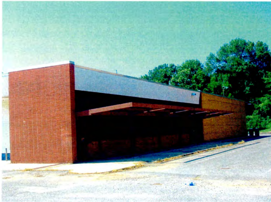
No. 25 Commercial Strip, 2100 Block of Independence Boulevard, Side (West) Elevation, Looking South.
