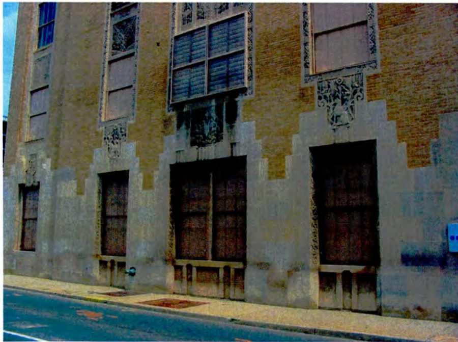
No. 8 Southern Bell Telephone Exchange Building, Façade Detail.
