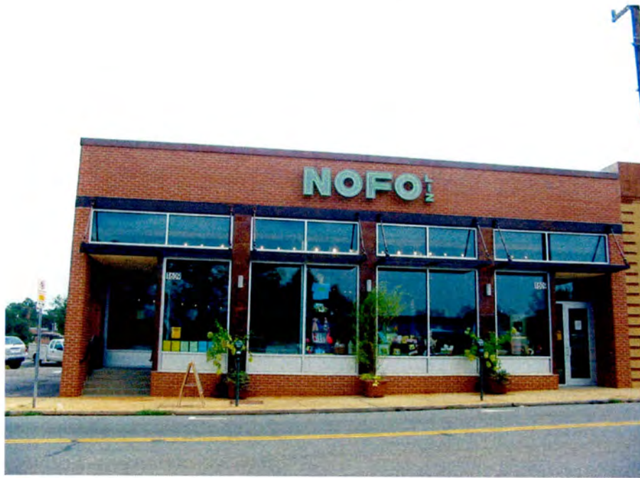
No. 20 Commercial Buildings, 1609-1617 Elizabeth Avenue, Looking North.
