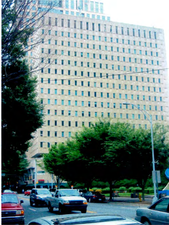
No. 7 Wachovia Bank and Trust Company Building, Building and Setting, Looking East Along Trade Street.
