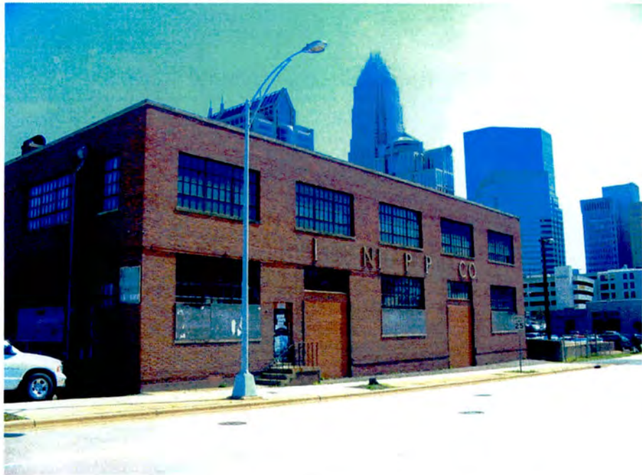
No. 4 Virginia Paper Company Warehouse, Façade (North) Elevation.
