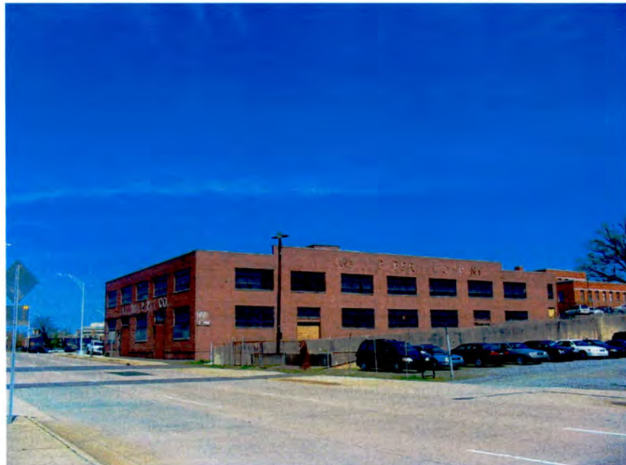
No. 4 Virginia Paper Company Warehouse, Side (East) Elevation.
