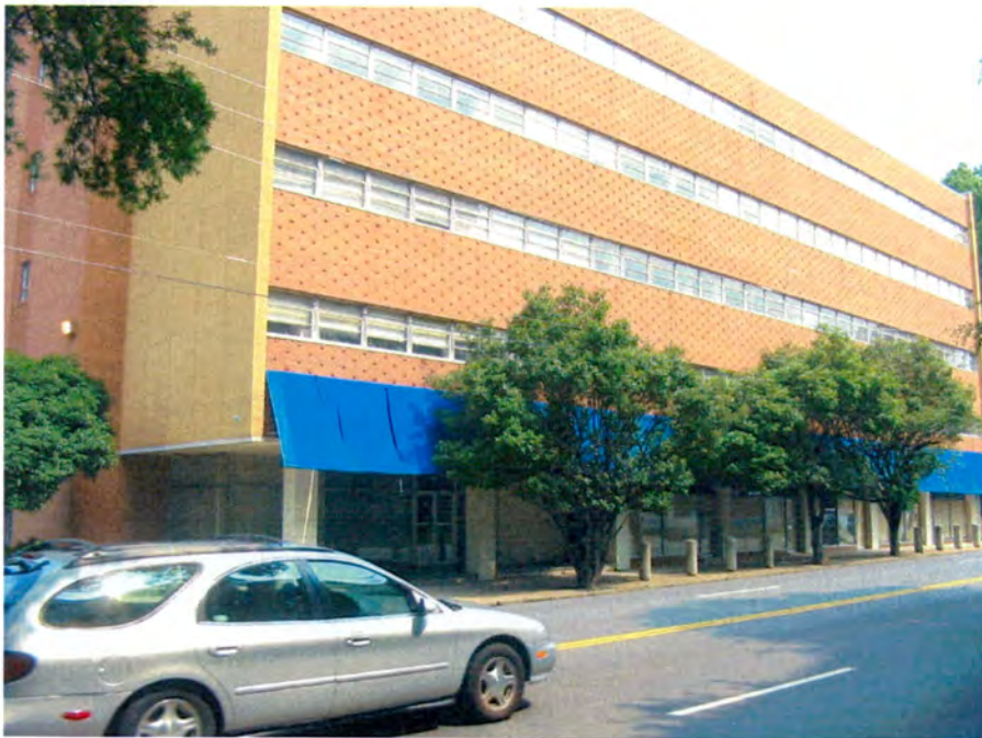
No. 21 Hawthorne Medical Center, Looking North Along Hawthorne Lane.
