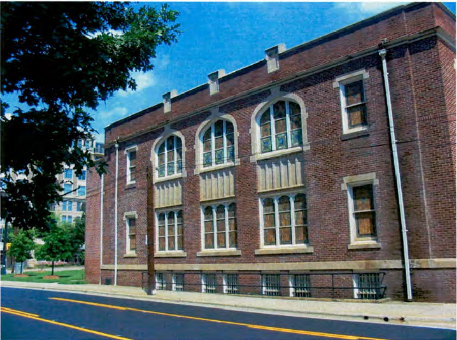
No. 1 West Avenue Presbyterian Church, Side (West Elevation).
