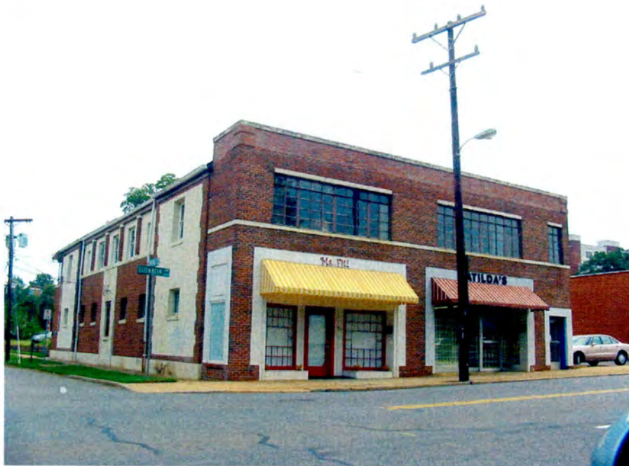
No. 19 Commercial Block, 1601-1605 Elizabeth Avenue, Looking East.
