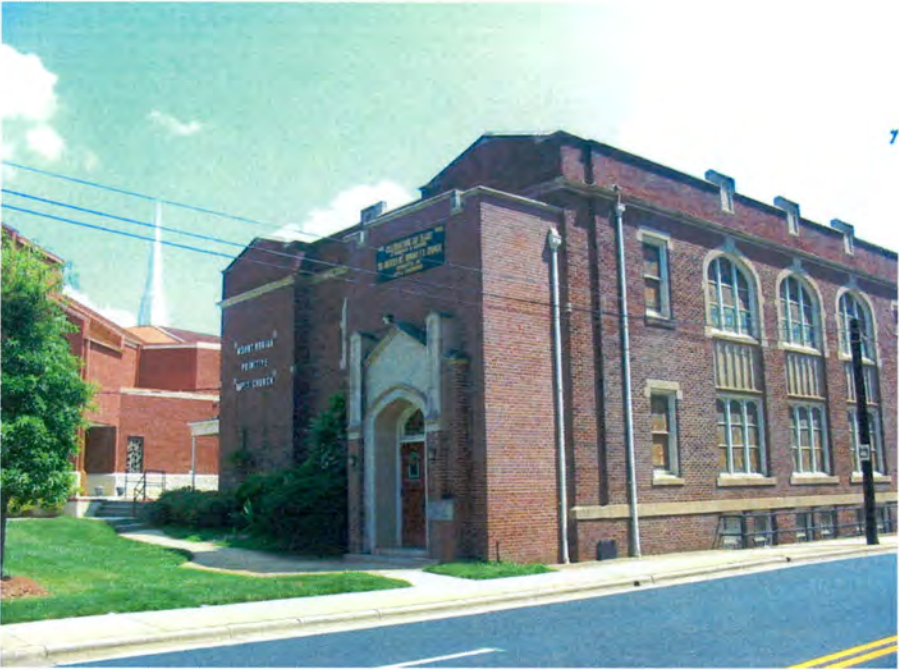
No. 1 West Avenue Presbyterian Church, Façade and Side (West) Elevation.
