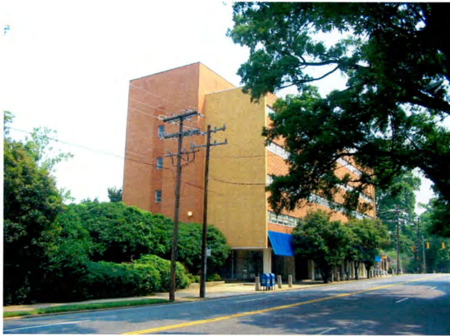
No. 21 Hawthorne Medical Center, Building and Setting, Looking North Along Hawthorne Lane.
