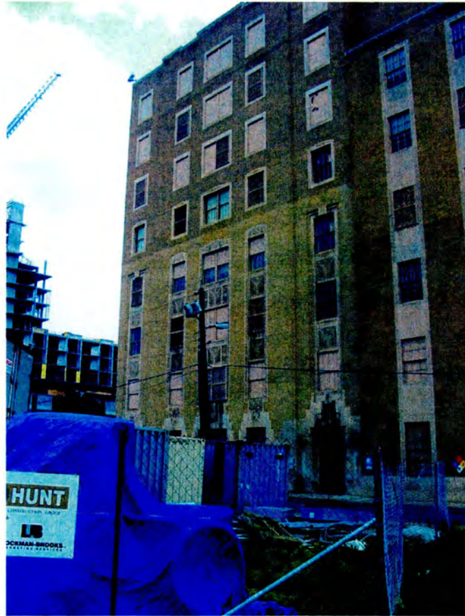
No. 8 Southern Bell Telephone Exchange Building, Façade (West) Elevation, Showing Additions.
