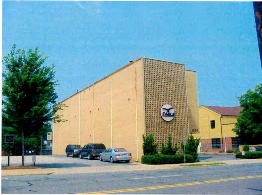
No. 18 Medical Office Building, Looking West.
