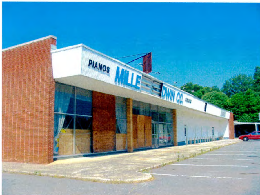
No. 25 Commercial Strip, 2100 Block of Independence Boulevard, Facades.
