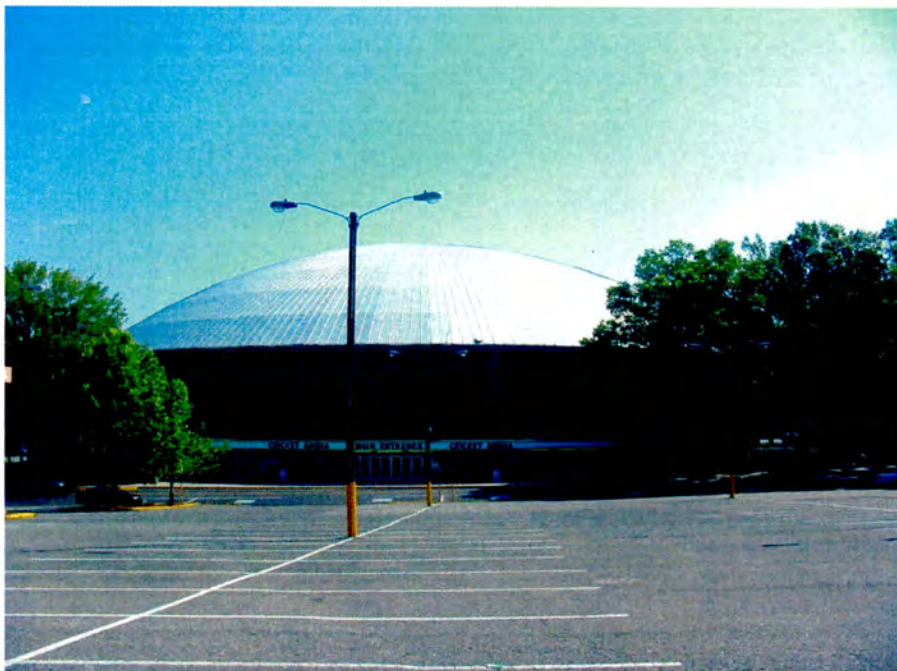
No. 26 Charlotte Coliseum and Ovens Auditorium, Looking North.
