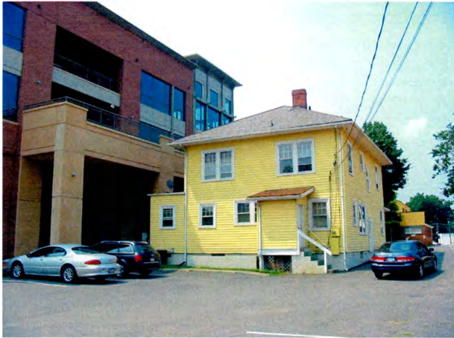
No. 16 House, Rear Elevation, Looking West.
