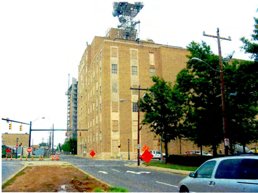
No. 8 Southern Bell Telephone Exchange Building, Building and Setting, Looking North Along Caldwell Street.
