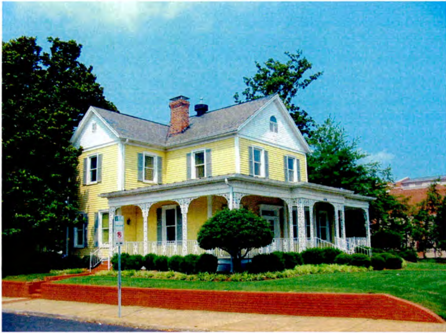
No. 15 House, House and Setting, Looking North.
