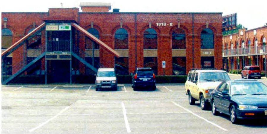
No. 23 Cole Manufacturing Company, Looking South.
