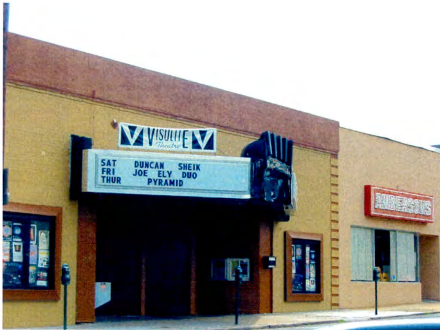
No. 20 Commercial Buildings, 1609-1617 Elizabeth Avenue, Looking North.
