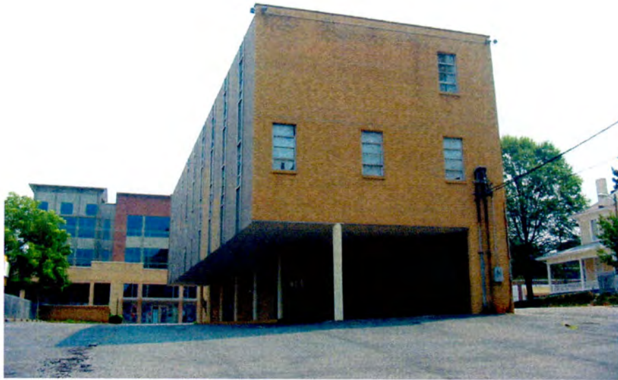
No. 18 Medical Office Building, Rear, Looking North.
