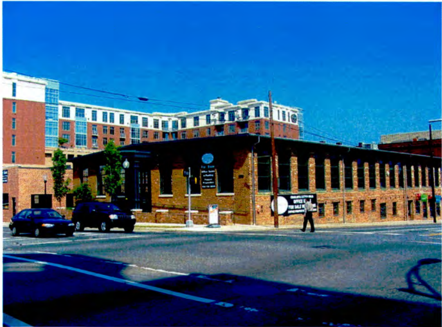
No. 5 Charlotte Cotton Mills, Buildings and Setting, Looking North.
