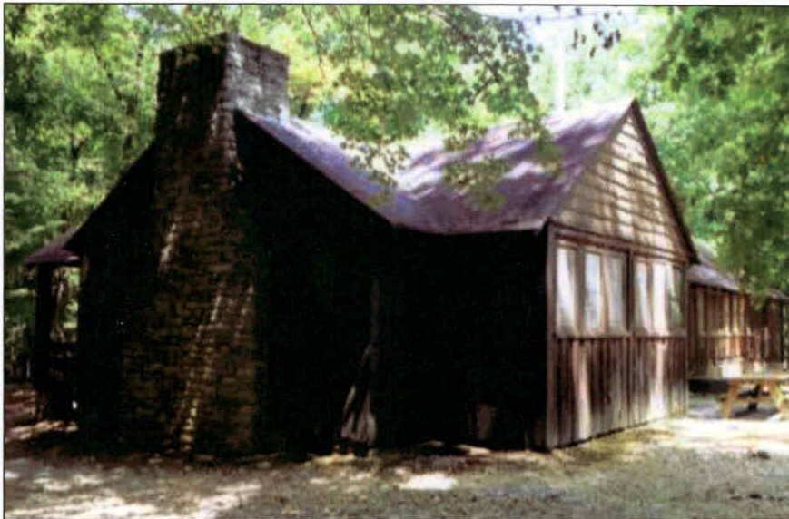
Figure 7: Frame mess hall at "Camp Crabtree," ca. 1930s, Umstead State Park, Wake County.
