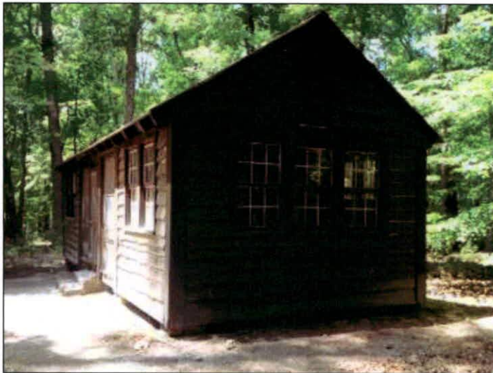
Figure 6: Frame structure at "Camp Crabtree," ca. 1930s, Umstead State Park, Wake County.
