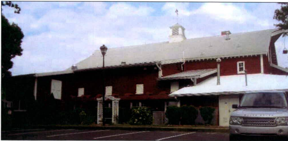
Figure 30: Angus Barn, North Elevation
