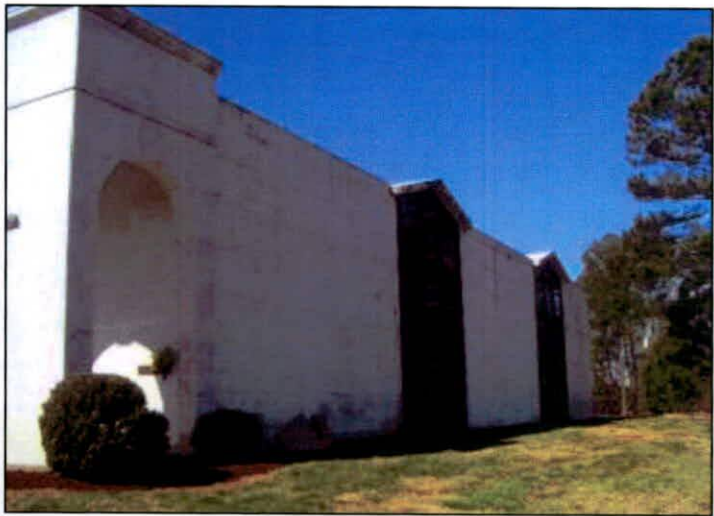
Figure 42: Chapel Mausoleum, east elevation
