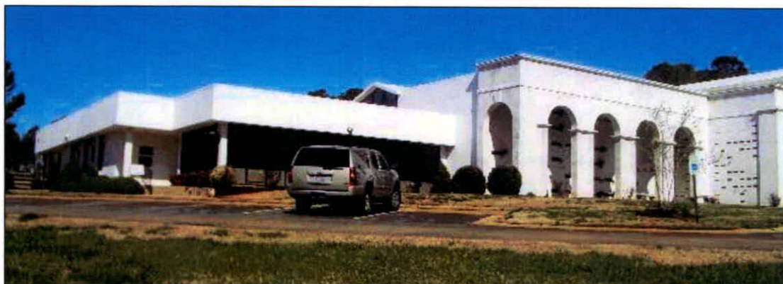
Figure 40: Chapel Mausoleum and addition onto the western elevation
