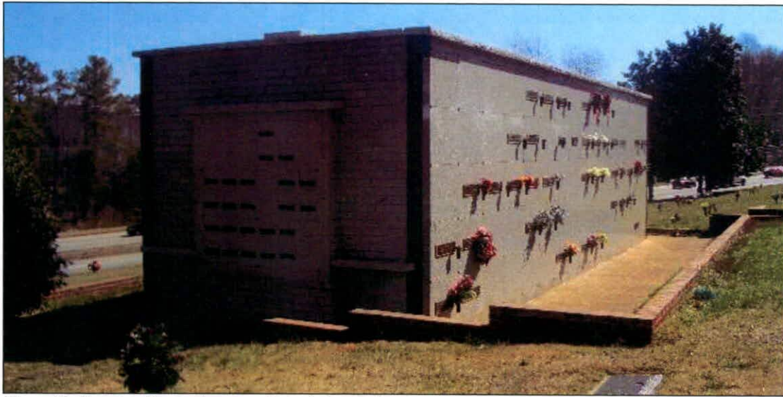
Figure 45: Free-standing garden mausoleum, facing southeast
