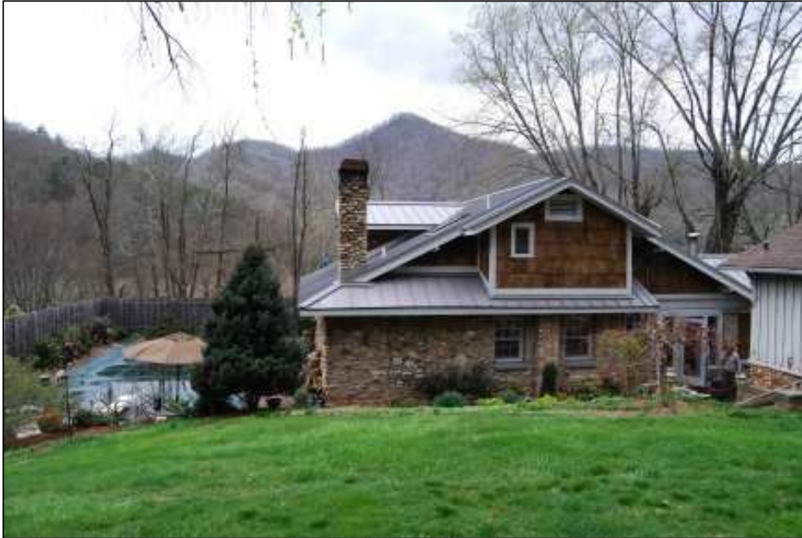
View of north (rear) elevation
