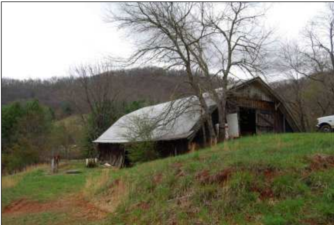
View of small barn looking north west
