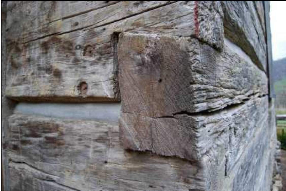
Detail of Poplar logs of Minnie Stephens House
