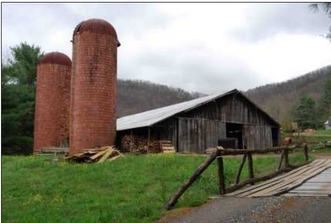
View of large barn and silos looking north west
