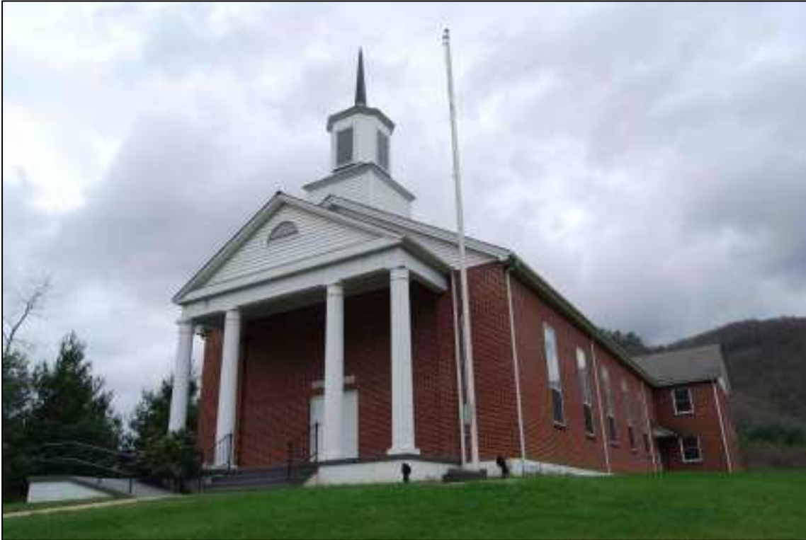
Tuckasegee Baptist Church looking south
