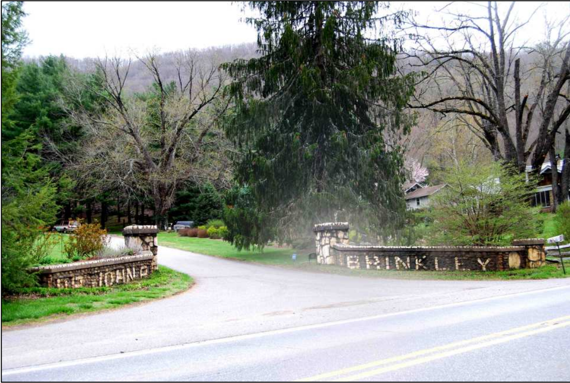
Rock Wall Entry to the Dr. John R. Brinkley House
