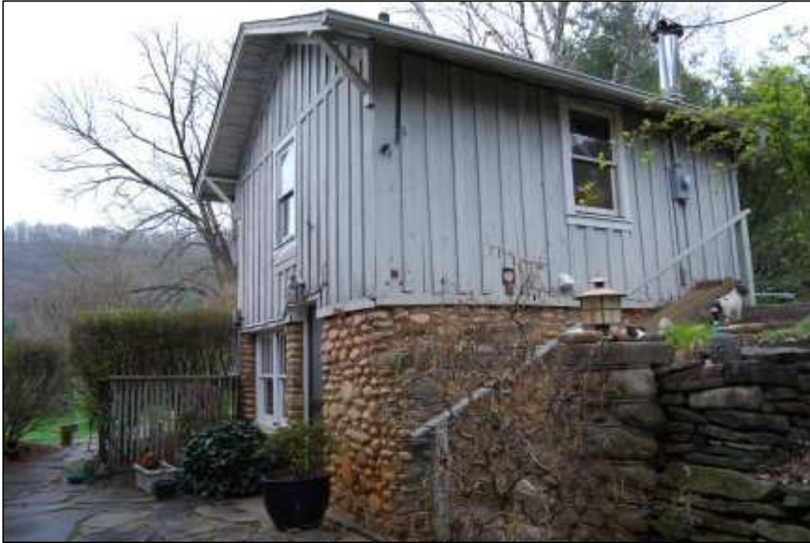
Root cellar and maids quarters
