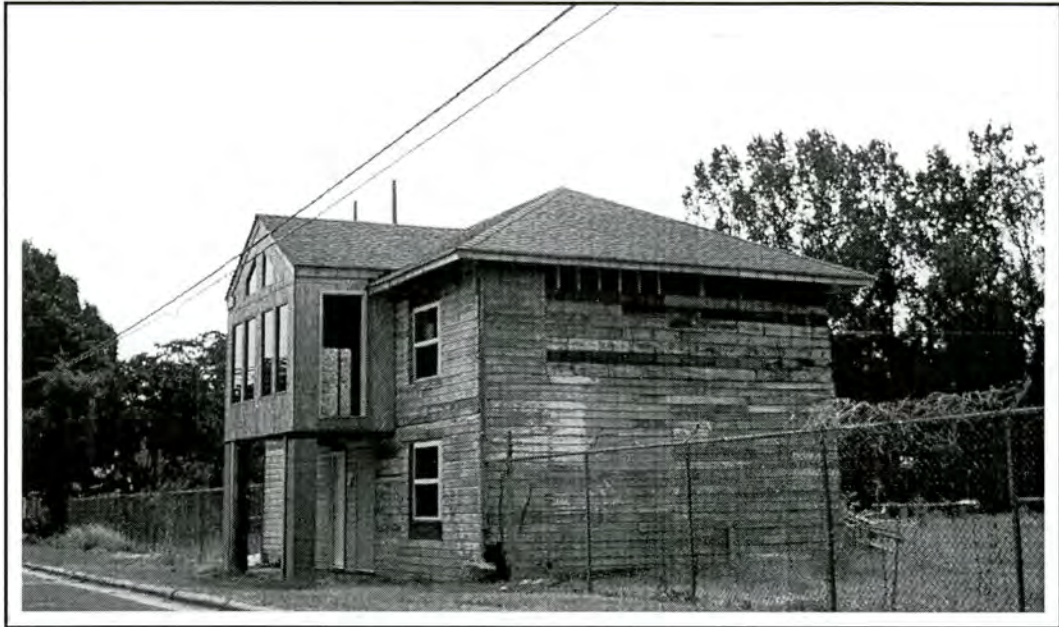
Figure 25. Property 12 - School. The property has been determined not eligible for the National Register because it is neither historically nor architecturally significant. Photographed August 24, 2000.
