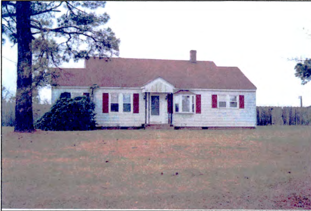
Property 15: House, 730 SR 1222, ca. 1950 CK0440
