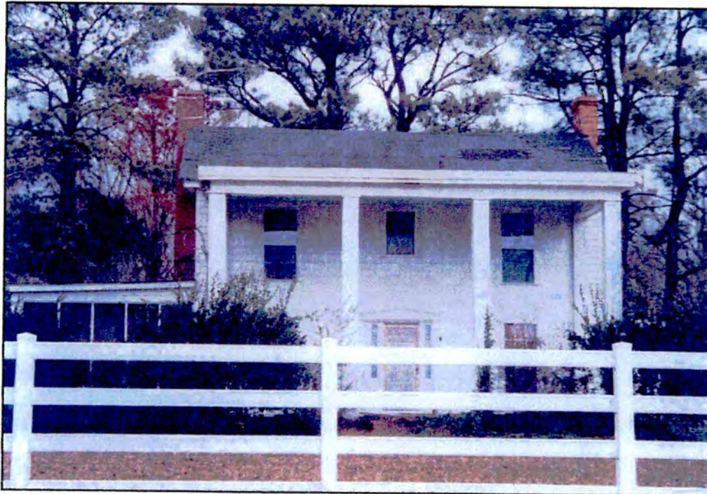
Property 10: House, 409 SR 1222. Front elevation. Ca. 1890-1900, with 1950s-1960s alterations. CK 0435
