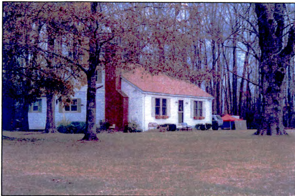
Property 11: House, 413 SR 1222, ca. 1950-1960 CK0436
