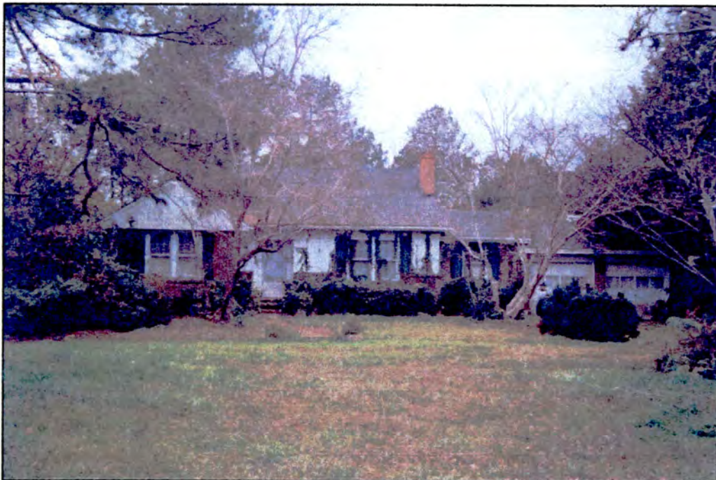
Property 3: House, 256 SR 1222, ca. 1950 CK0432
