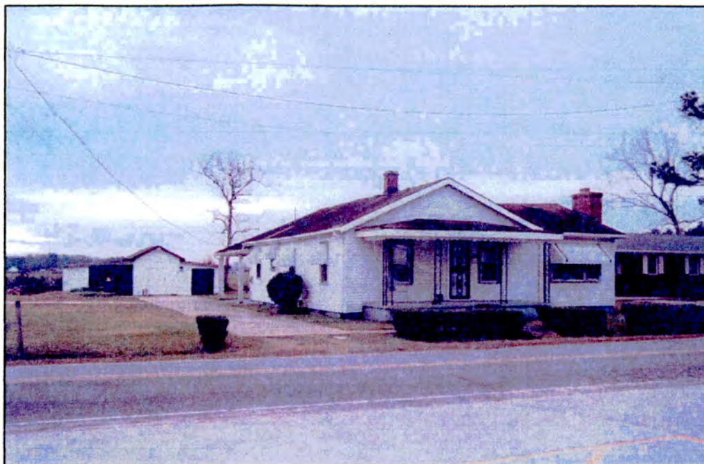
Property 4: House, 105 Puddin Ridge Road (SWC SR 1222 and SR 1216), ca. 1920-1940 CK0433
