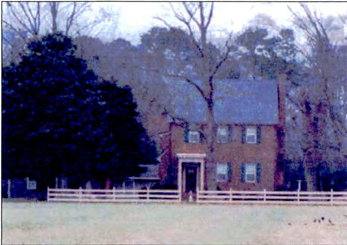
Figure 16: Sanderson House, south elevation
