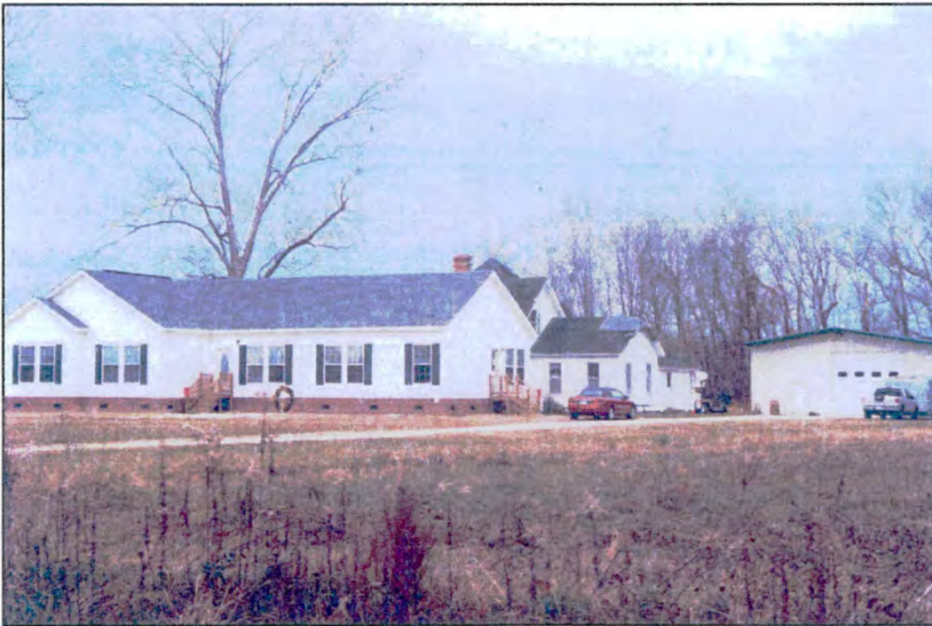
Property 8: House, in December 2004; one chimney removed, and manufactured house in foreground.
