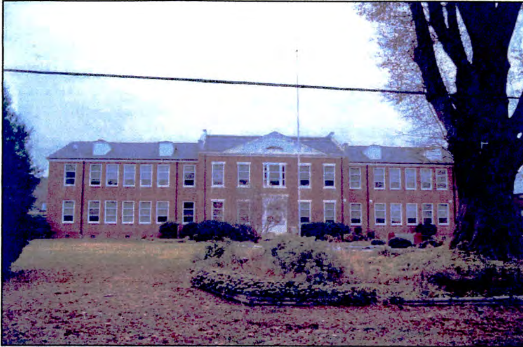
Property 2: Moyock School, front elevation and landscaping
