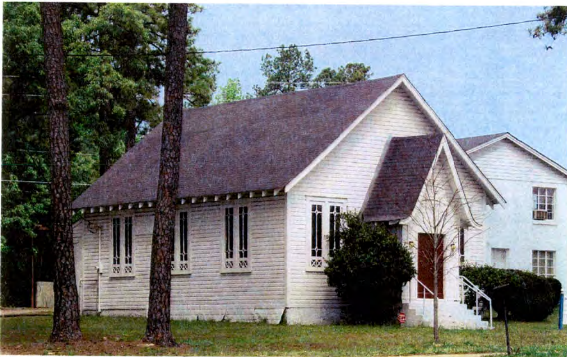
Photo 4: East front and south side elevations.
