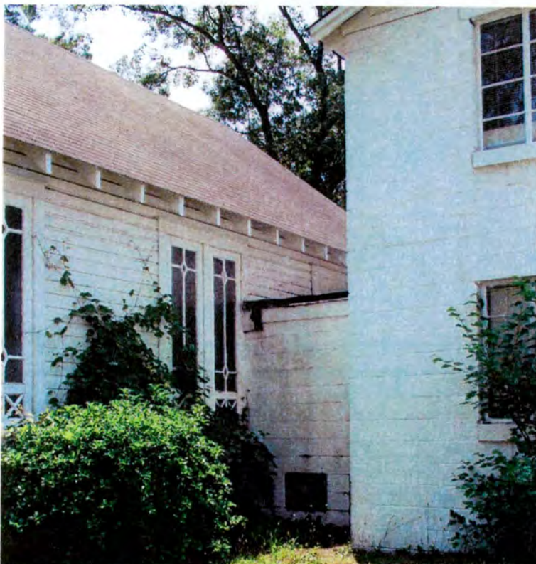
Photo 6: Detail view of concrete block connection between church and fellowship hall.
