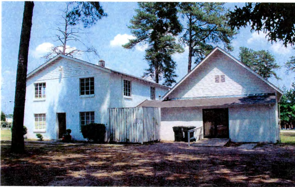
Photo 8: Rear of building, now the main entrance of the church.
