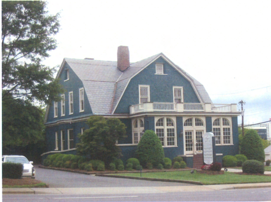
Façade and West Elevation, Looking Northeast.
