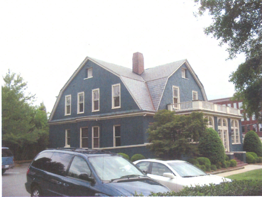
Side (West) Elevation, Looking Northeast.
