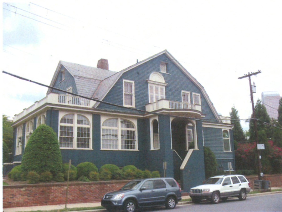
Side (East) Elevation, Looking West.
