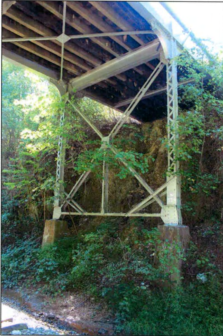
Figure 8: Bridge No. 88, detail of substructure and block piers. Penne Sandbeck/NCDOT, September 2007.
