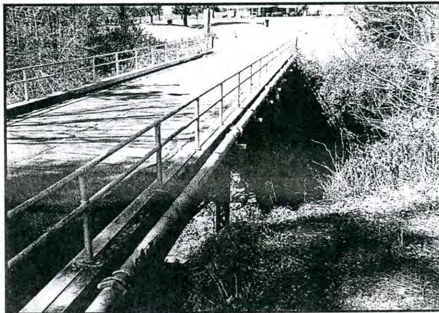
UTILITY ON NORTH SIDE OF BRIDGE, LOOKING EAST
