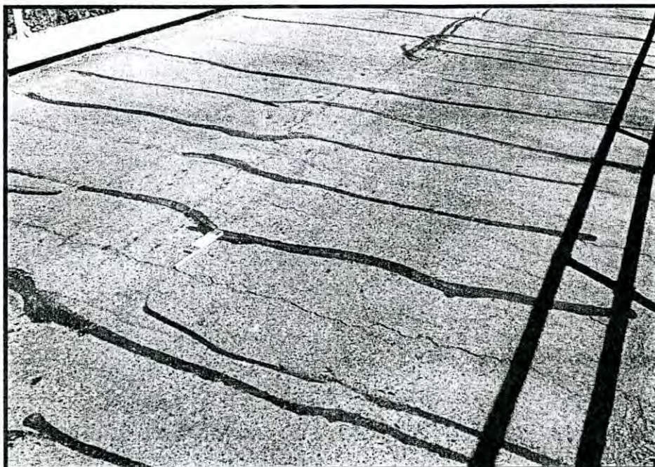
ASPHALT WEARING SURFACE IN SPAN A
