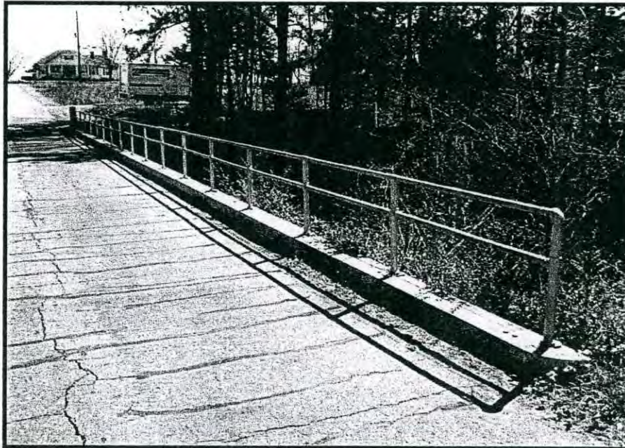
RAIL ON SOUTH SIDE, LOOKING EAST
