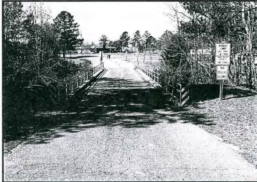
EAST APPROACH, LOOKING WEST
