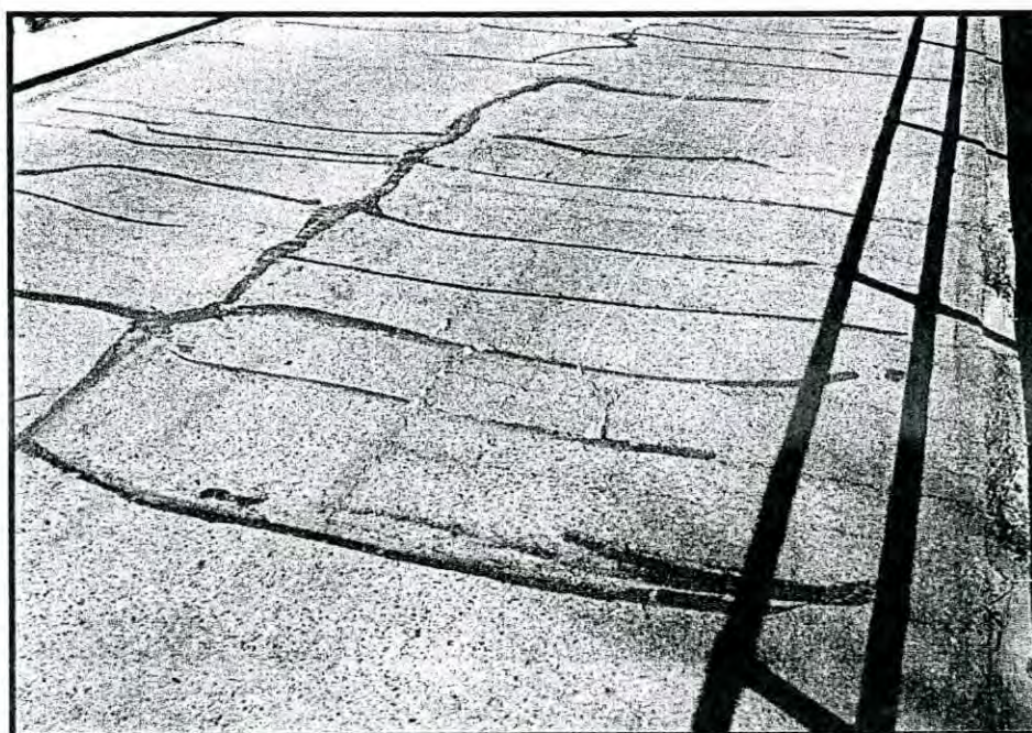
ASPHALT WEARING SURFACE IN SPAN B
