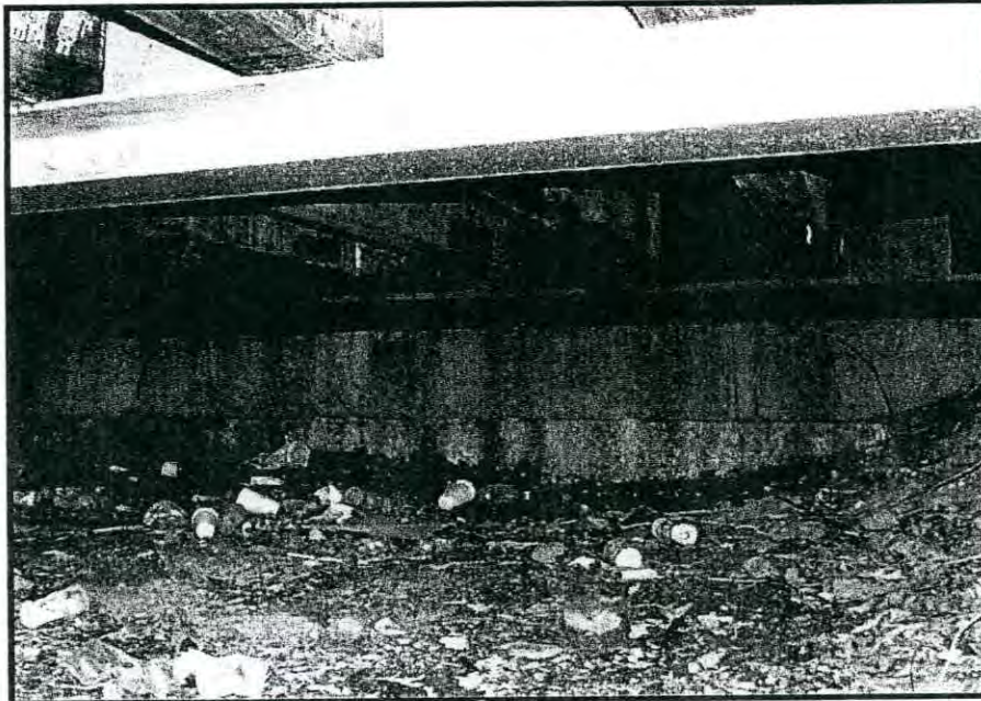
VIEW OF ABUTMENT 1
