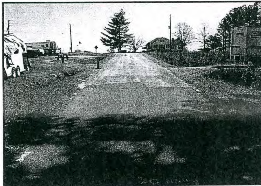
EAST APPROACH, LOOKING EAST
