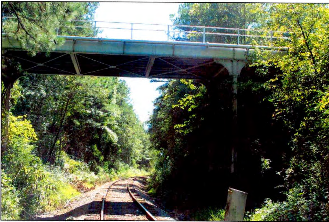
Figure 2: Bridge No. 88, north elevation, Penne Sandbeck/NCDOT, September 2007
