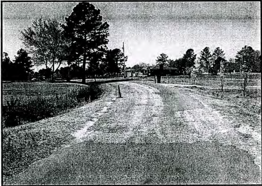
WEST APPROACH, LOOKING WEST
