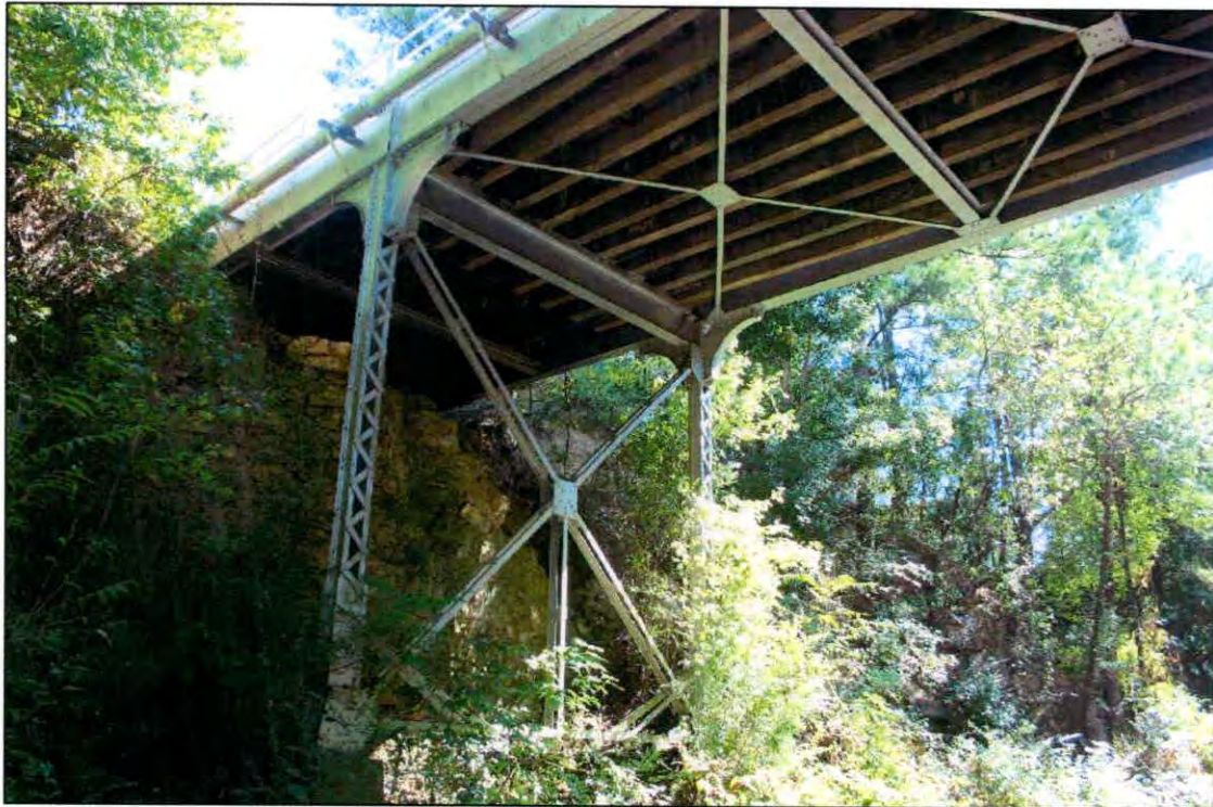
Figure 7: Bridge No. 88, detail of substructure, north elevation. Penne Sandbeck/NCDOT, September 2007.
