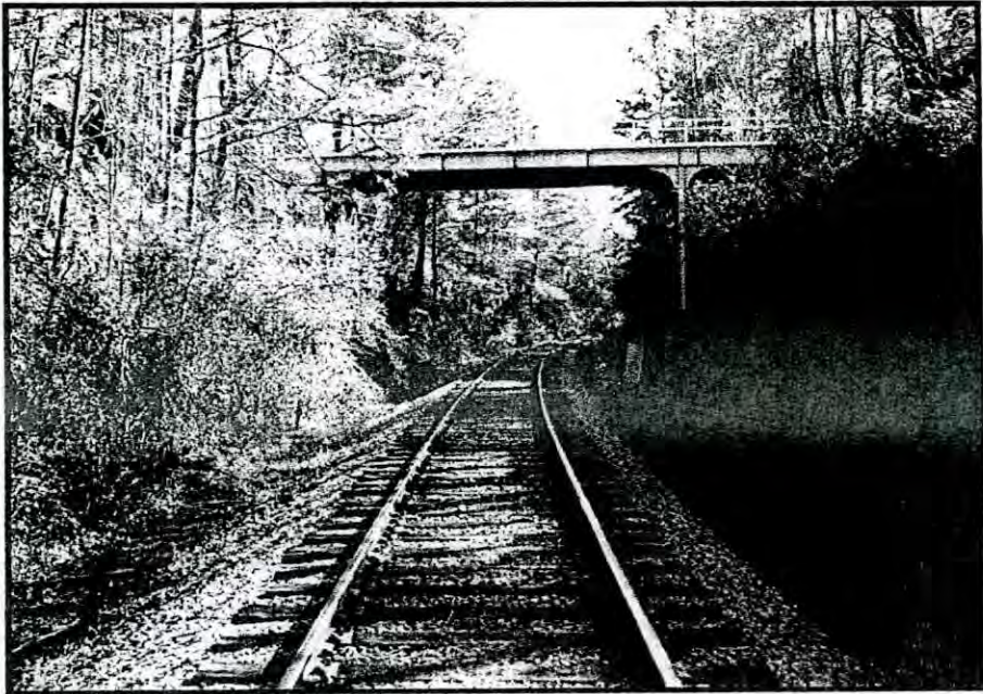
NORTH STRUCTURE PROFILE, LOOKING SOUTH
