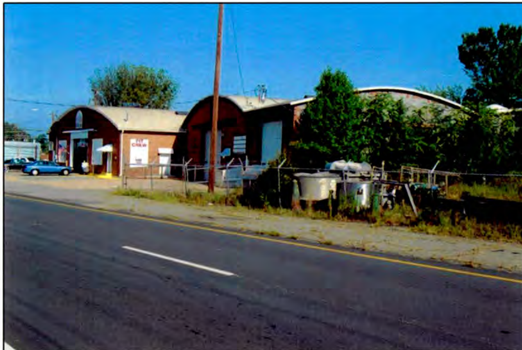
Figure 51. Pit Crew Service Center: looking northwest at western building at left, recessed central building at center and, at right, eastern building with front portion of arched roof turned to the side
