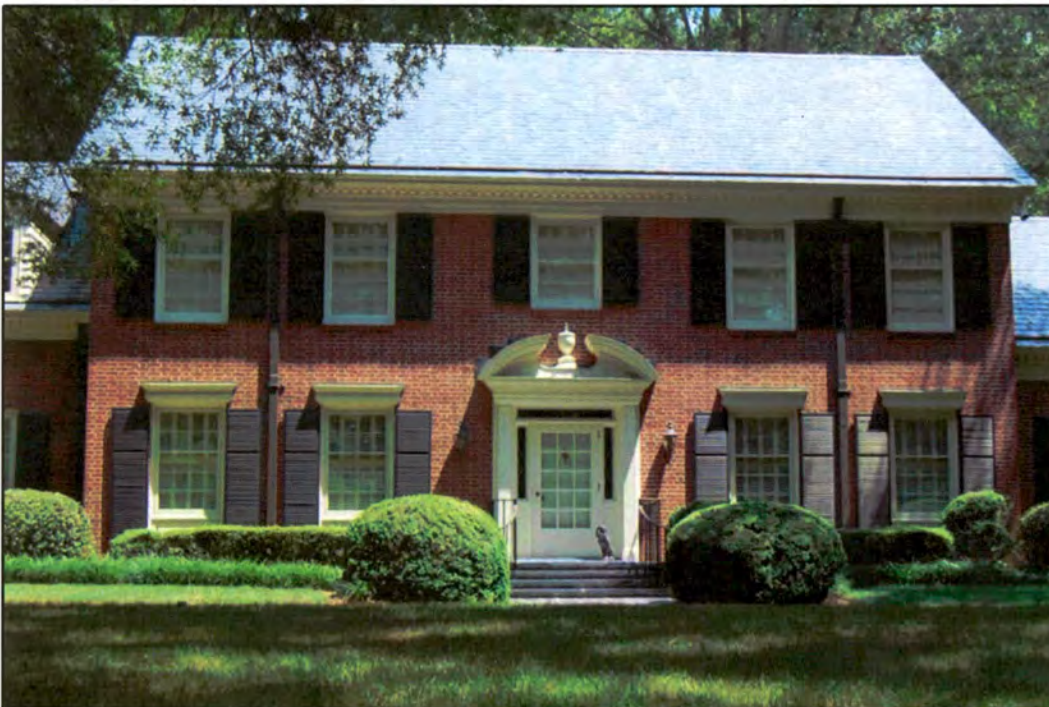
Figure 69. Sen. James T. Broyhill House: main block, west front façade
