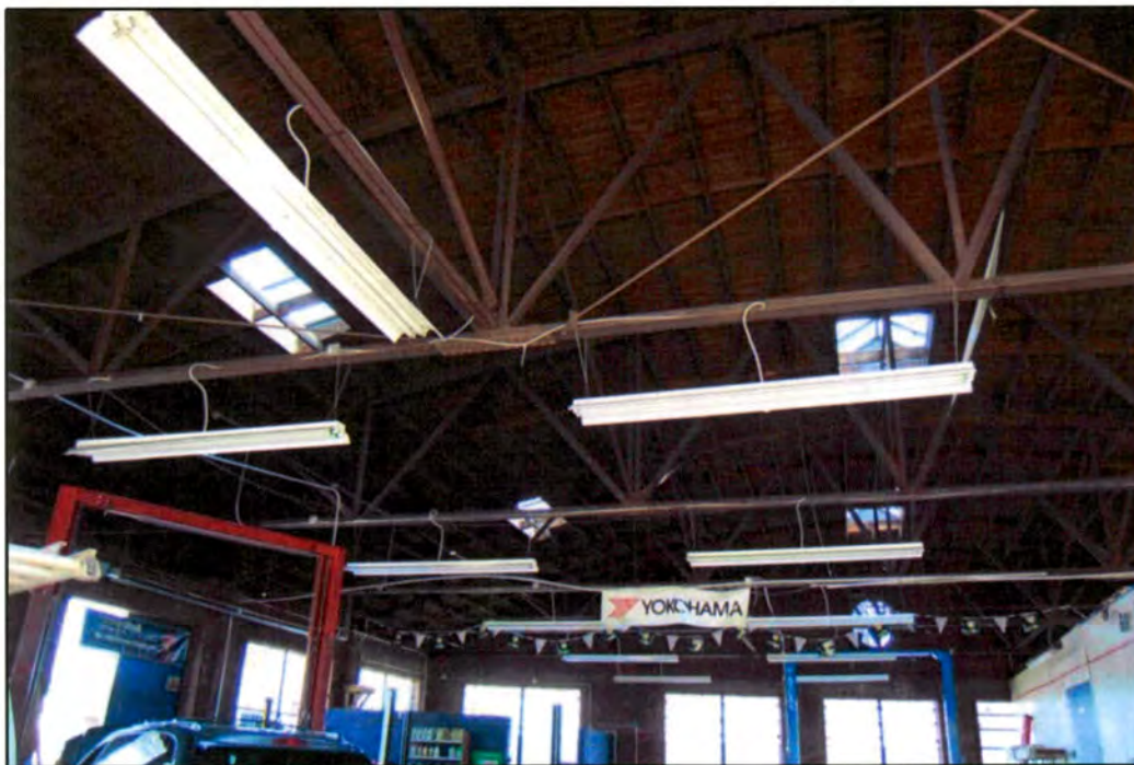
Figure 55. Pit Crew Service Center: open interior bay of western building; note metal ceiling trusses, arched wooden roof and, at right, wall of inserted office space
