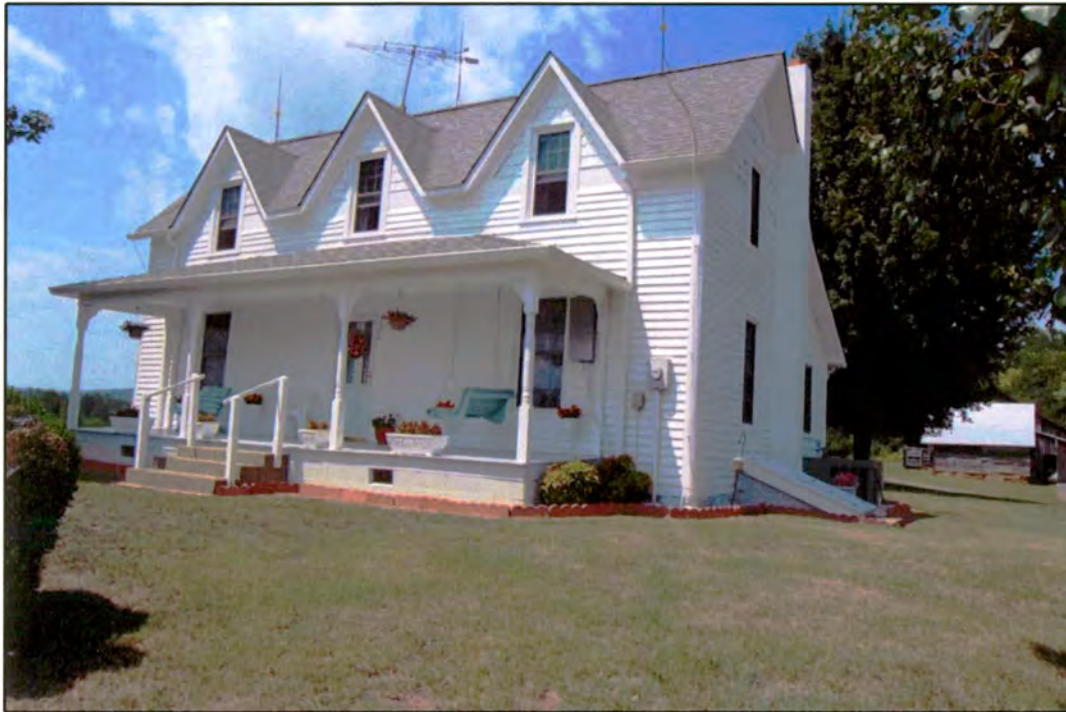
Figure 15. G. Haywood Hartley House: south front and east side elevations of house [A]; granary [B] at far right
