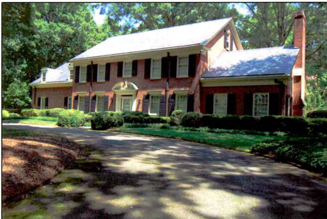
Figure 71. Sen. James T. Broyhill House: west front and south side elevations
