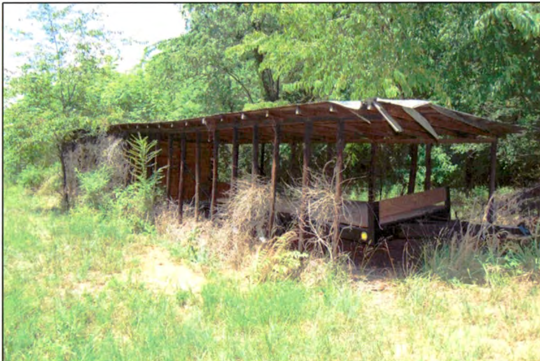
Figure 22. G. Haywood Hartley House: looking northwest at pole barn/shed [E]
