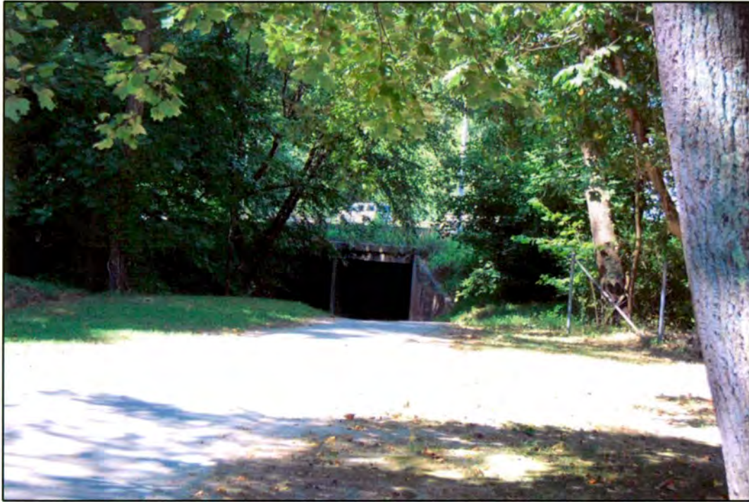
Figure 88. Lenoir Golf Club: southernmost of two concrete tunnels that carry golf cart paths beneath US 321
