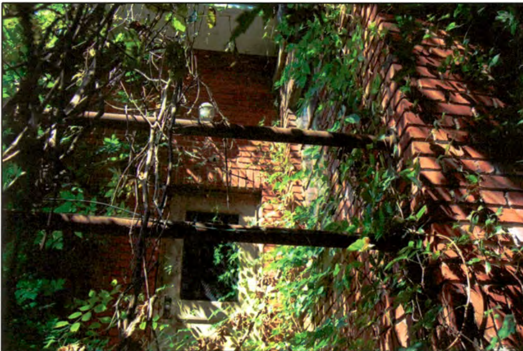
Figure 66. Hickory Waterworks Pumping Station: entry, pipe railings, and ell at east elevation
