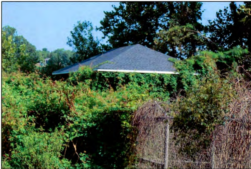
Figure 62. Hickory Waterworks Pumping Station: south and west elevations obscured by fence and heavy overgrowth
