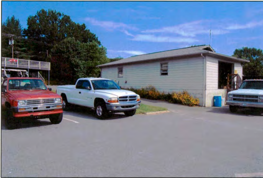
Figure 86. Lenoir Golf Club: modern service building to front (east) of clubhouse, corner of which is visible at left
