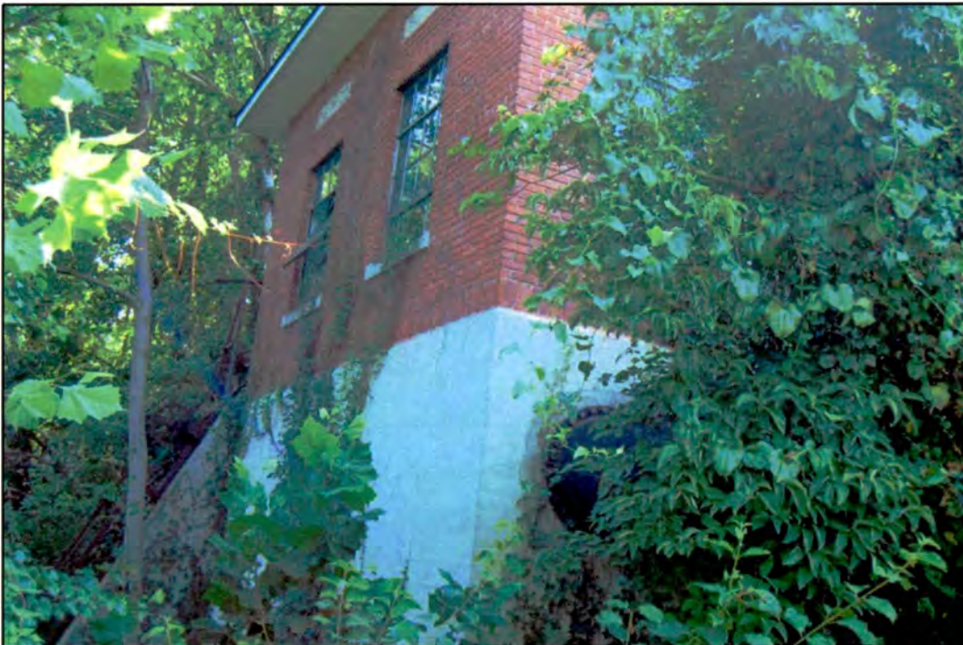
Figure 64. Hickory Waterworks Pumping Station: west and north elevations; note outtake pipe extending out of base of east elevation and concrete-butressed spillway at side of north river elevation
