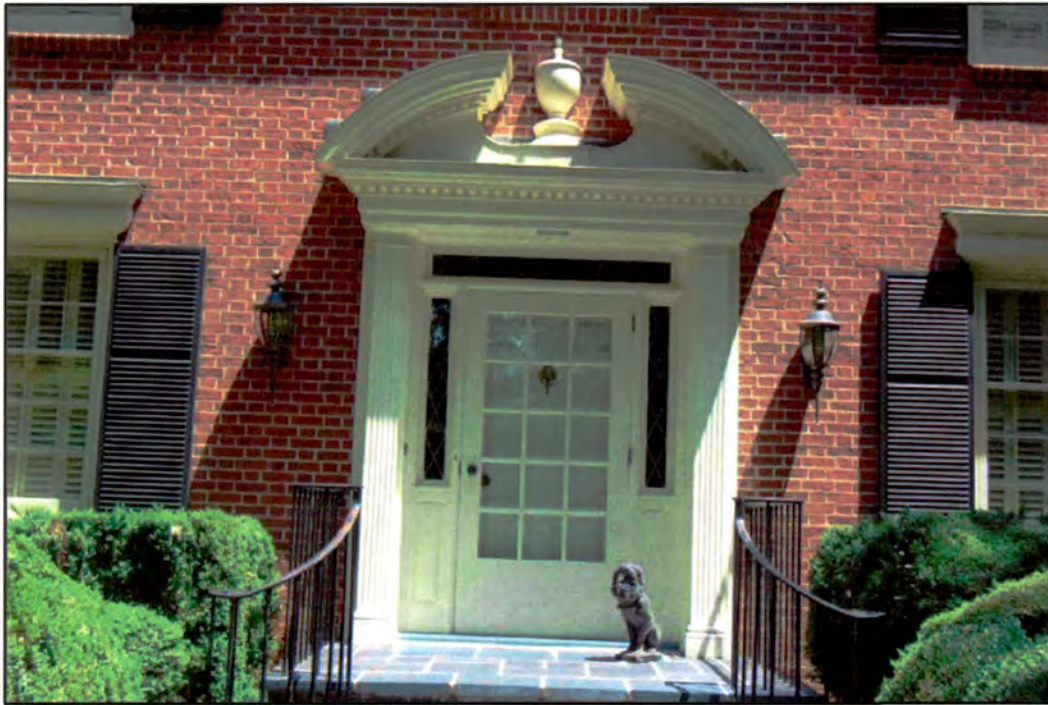
Figure 70. Sen. James T. Broyhill House: detail of west front facade
