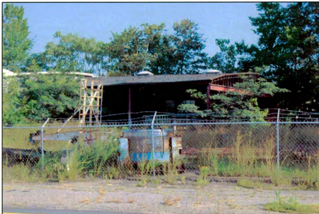
Figure 57. Pit Crew Service Center: looking northwest at open arch-roofed building at far right of building complex; note east-facing arch of eastern building peeking above heavy overgrowth at left
