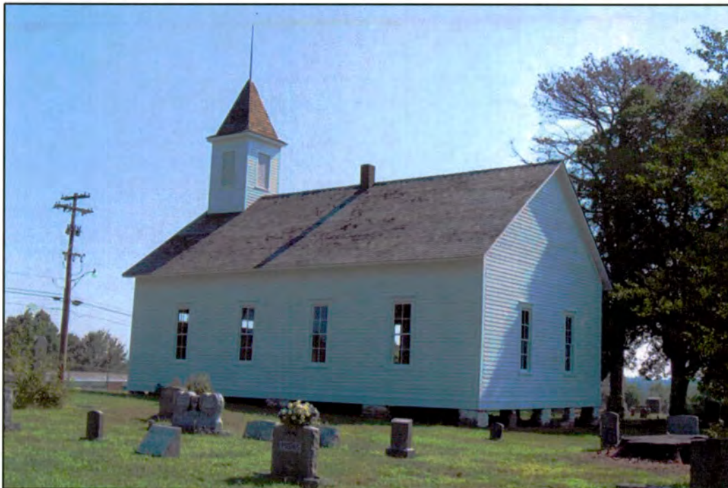
Figure 6: Houck's Chapel: south rear and west side elevations
