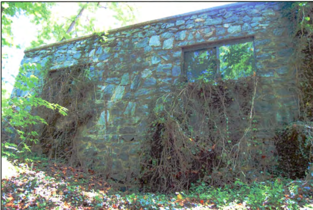
Figure 44. James Edgar Broyhill Estate: looking east at pool utility building [E]
