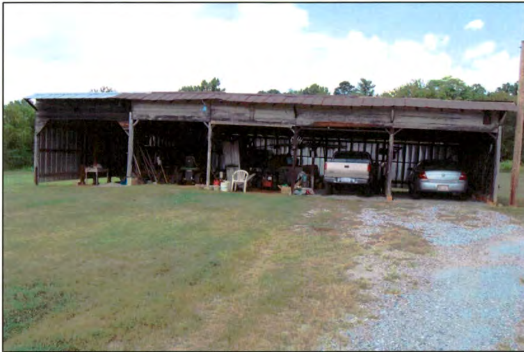
Figure 21. G. Haywood Hartley House: looking north at equipment shed [D]
