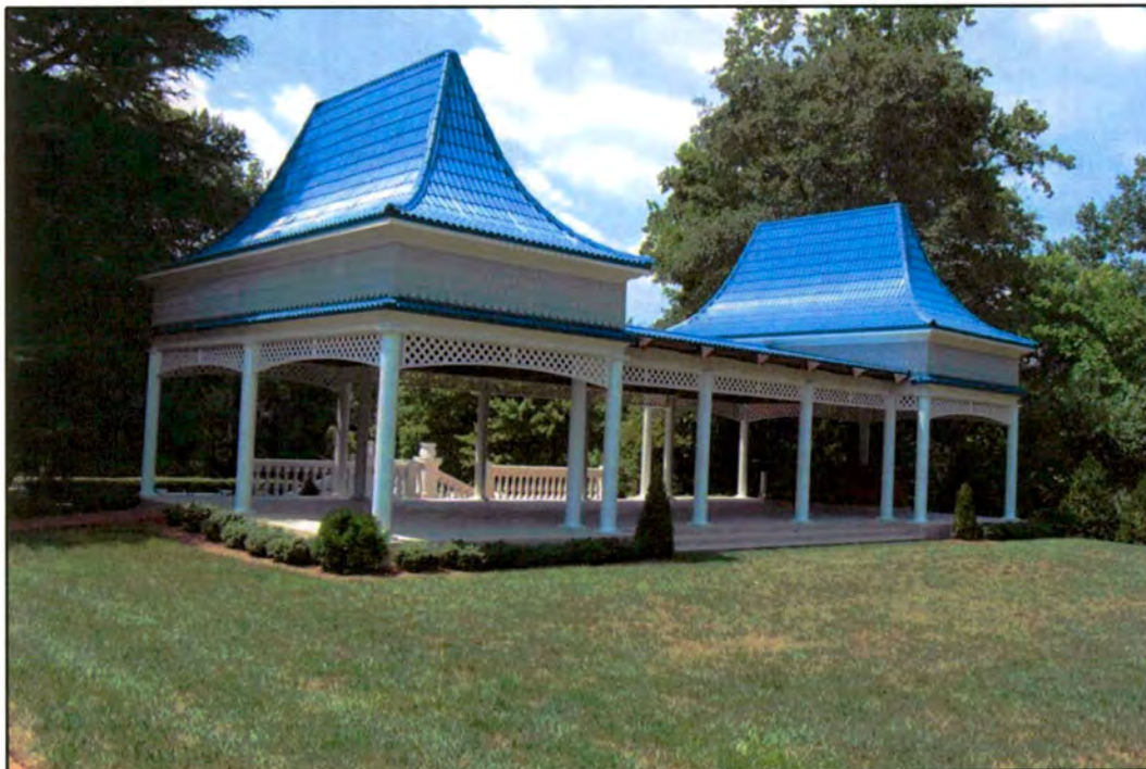
Figure 42. James Edgar Broyhill Estate: looking southwest at modern pavilion [C]
