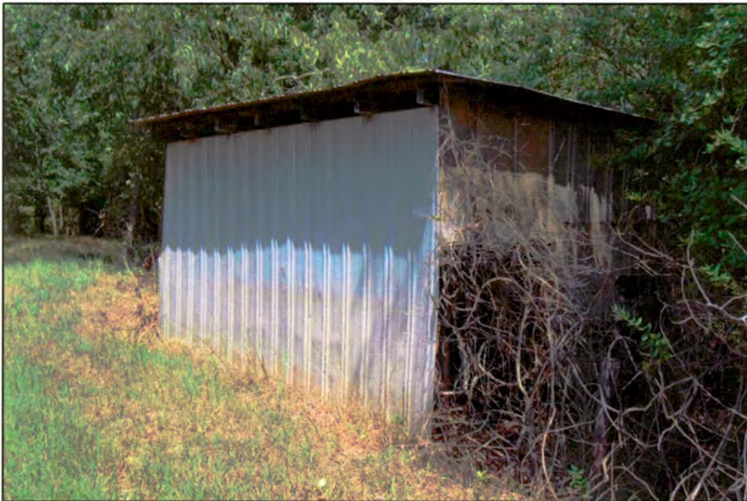
Figure 24. G. Haywood Hartley House: looking northeast at shed [G]
