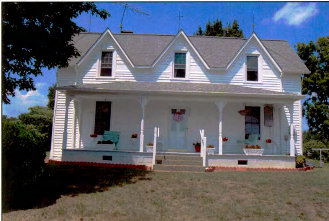
Figure 14. G. Haywood Hartley House: south front façade of house [A]
