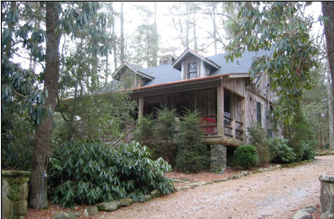
Figure 14 (above): 251 Cullasaja Drive, noncontributing property, property 8 on Figures 2 and 3
