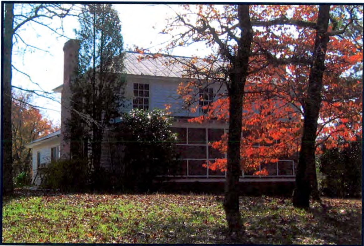
Figure 9. Property No. 5 – House. Northwest (main) and northeast elevations. Photographed November 9, 2006.
