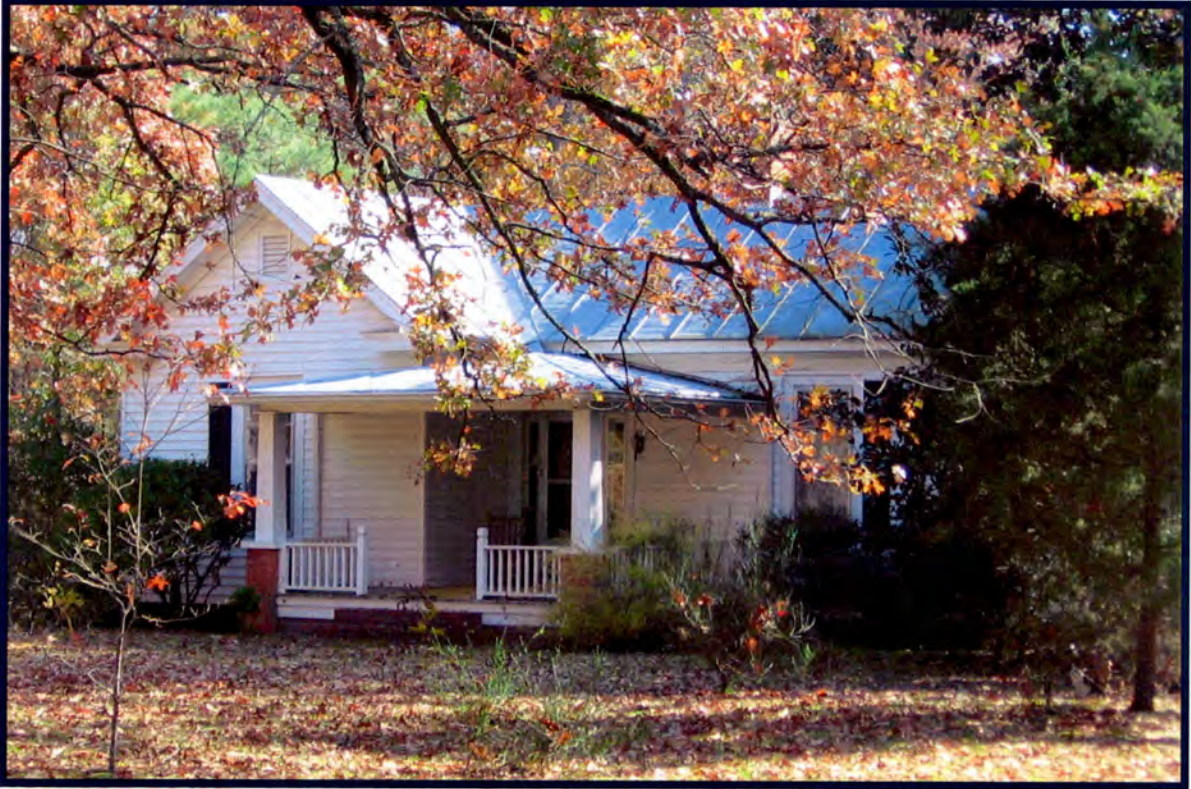
Figure 5. Property No. 7 – House. Northwest (main) elevation. Photographed November 9, 2006.
