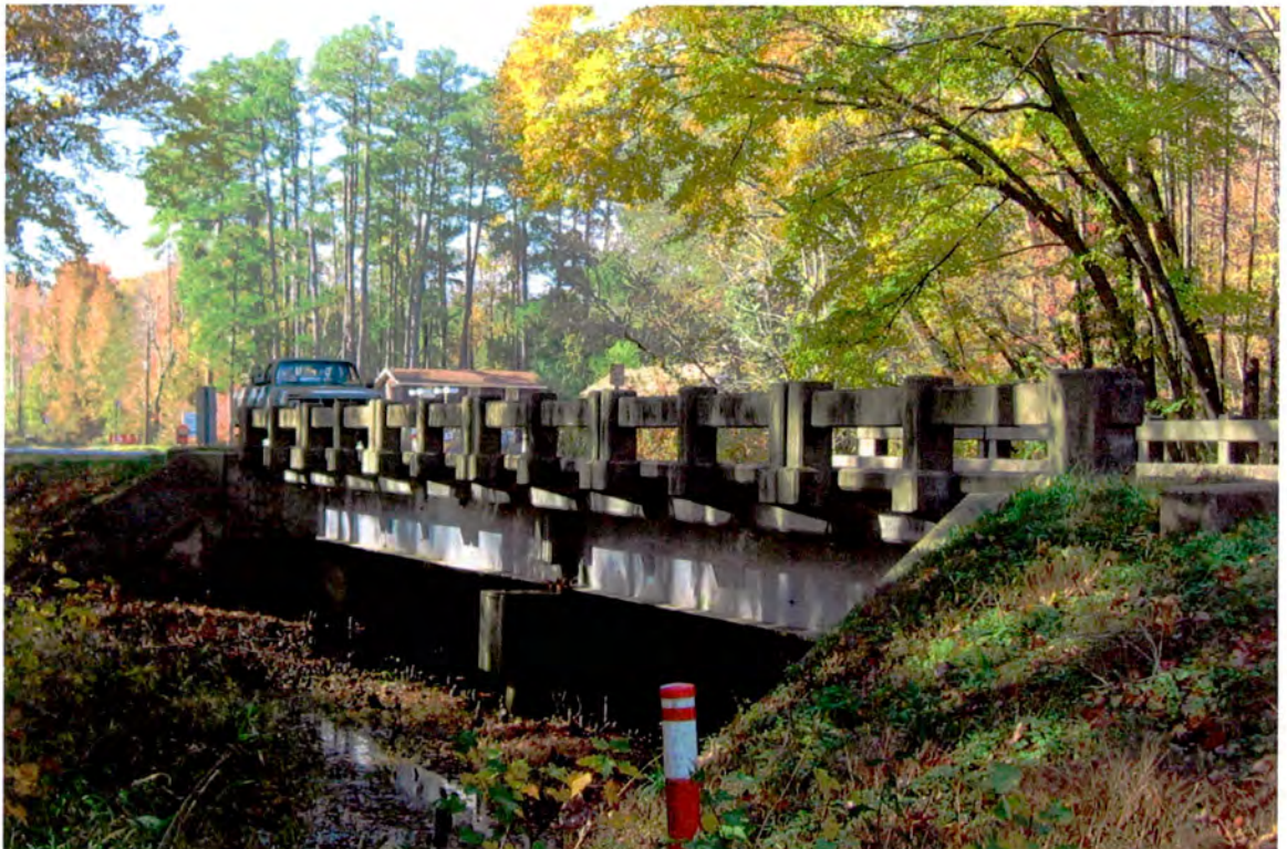
Figure 15. Property No. 2 – Bridge No. 9. US 13/158, Buckhorn Creek.
