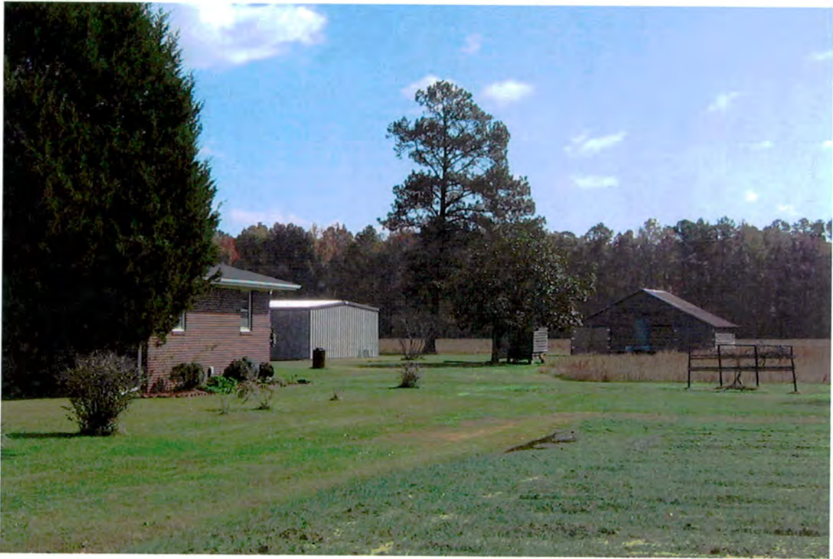
Figure 20. Property No. 10 - House and Outbuildings. #80 US 13/158.
