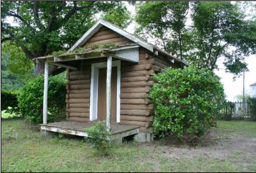
Figure 24: Moses R. White, Jr., House, log "playhouse," ca. 1945, front and west elevations
