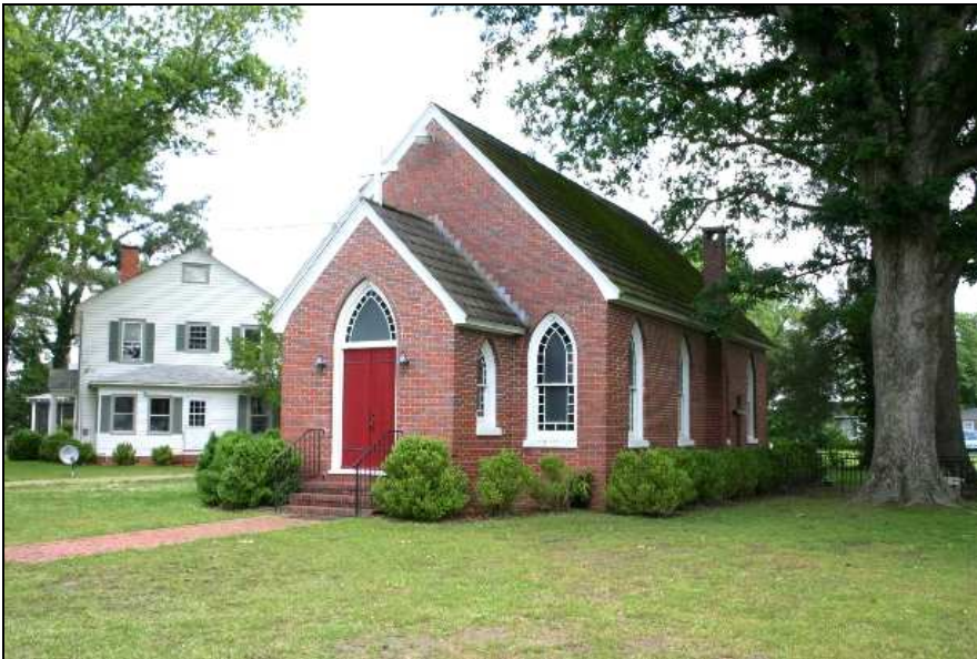
Property 107: St. Peter's Episcopal Church, 61 NC 32 N. PIN 0500186. Rebuilt 1939, in style and form of original 1908 church on site.
