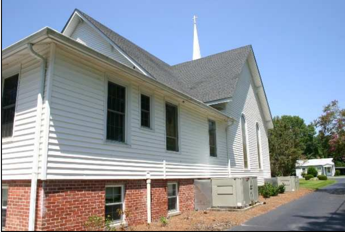
Figure 98: Beulah Baptist Church, view of east elevation. Penne Sandbeck NCDOT, August 2009.
