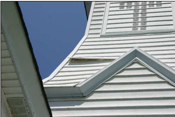
Figure 50: Church tower, showing shingles beneath replacement siding.
