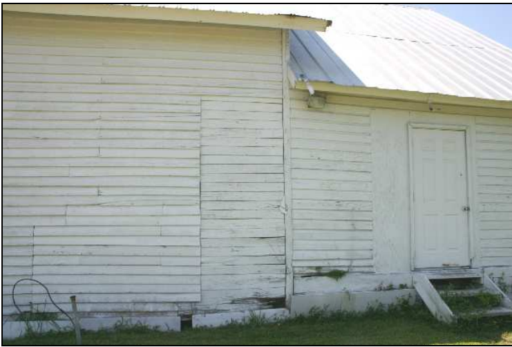
Figure 36: Perry-Harris-Jones Store, east elevation, detail of enclosed door and alterations to siding.
