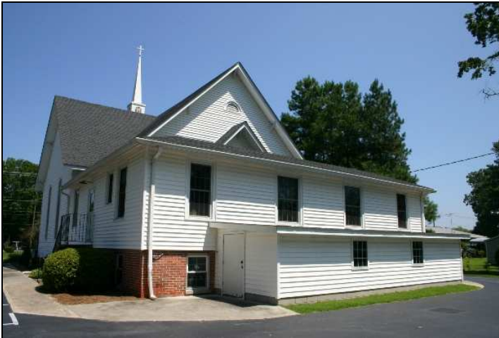
Figure 99: Beulah Baptist Church, rear elevation. Penne Sandbeck NCDOT, August 2009.
