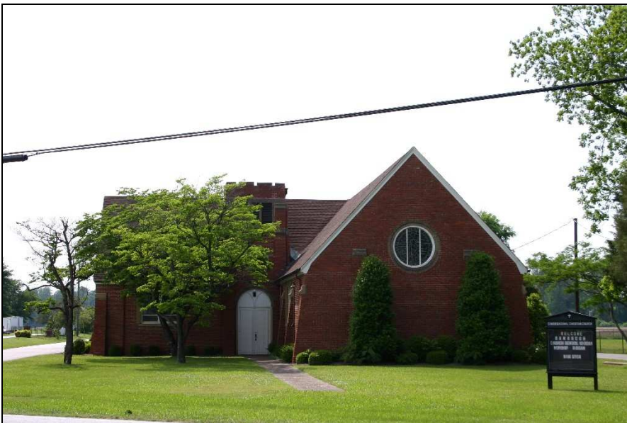
Property 111: Damascus Congregational Christian Church, ca. 1980 (noncontributing due to age, but a nicely-designed building and will eventually be contributing if it's not badly altered)., 84 NC 32 N. PIN 0501386
