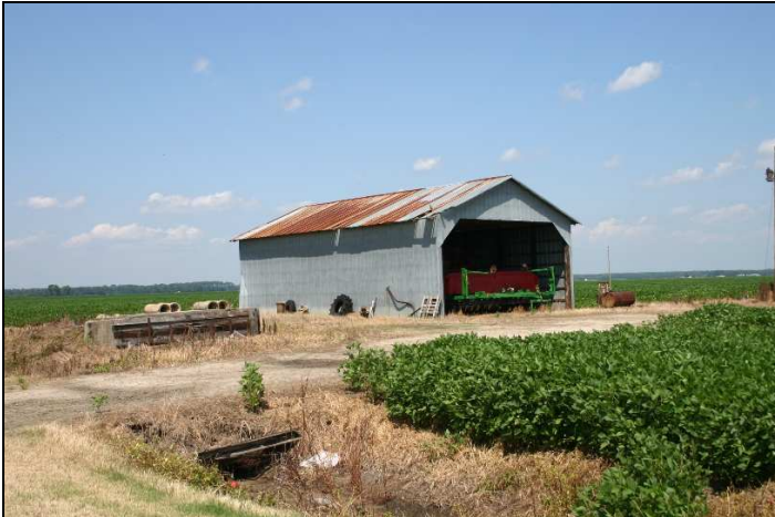
Figure 68: 1960s tractor shed, Black Acre Farm, with site of large transverse barn where pipes are placed. Penne Sandbeck, NCDOT, August 2009.
