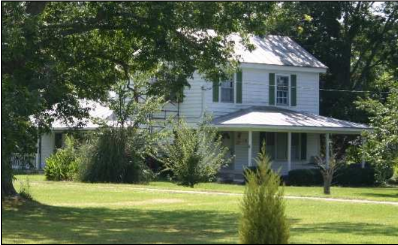
Figure 81: Benjamin F. Pierce House, 1299 US 158 E (taken from right-of-way). Penne Sandbeck, NCDOT, August 2009.
