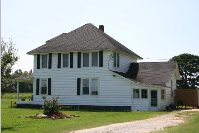
Figure 67: East elevation and part of north elevation, Black Acre Farm , showing enclosure of porch. Penne Sandbeck, NCDOT, August 2009.
