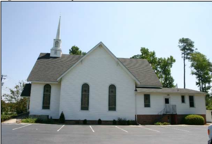
Figure 96: Beulah Baptist Church, west elevation, Penne Sandbeck, NCDOT, August 2009.
