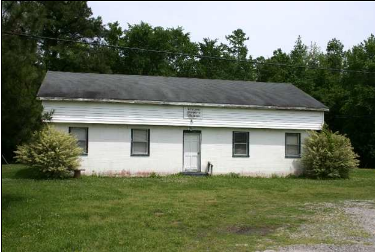
Property 50: Community Club of Newland, SE corner US 158 and SR 1359. PIN 7978320124. Determined Not Eligible.
