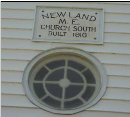
Figure 47: Newland United Methodist Church, detail of sign, front elevation.
