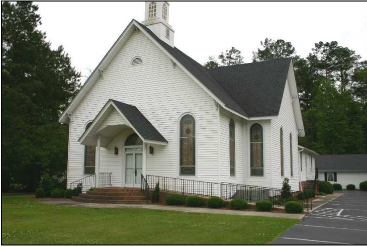
Figure 94: Beulah Baptist Church, 967 US 158, Sunbury. Penne Sandbeck, NCDOT, May 2009.
