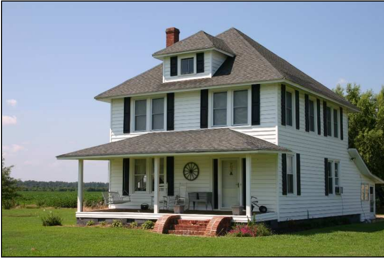
Figure 65: Black Acre Farm, 284 US 158, Tadmore vic. Front elevation of house. Penne Sandbeck NCDOT, August 2009.
