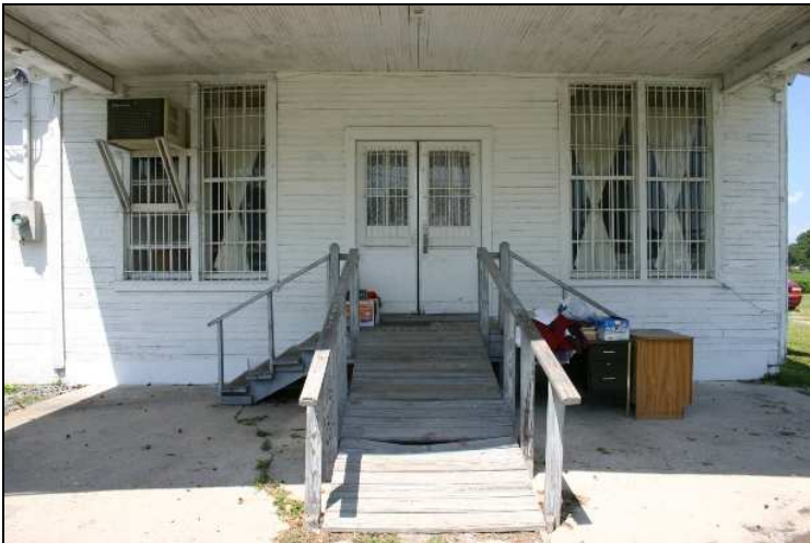
Figure 40: Perry-Harris-Jones Store, entrance.
