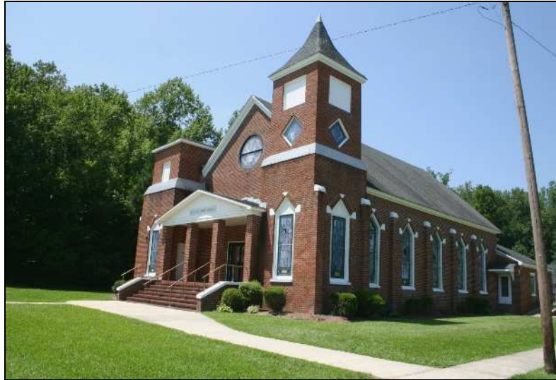
Figure 28: Mount Carmel Missionary Baptist Church, 834 US 158, Jackson's Corner vic. Penne Sandbeck, NCDOT, August 2009.
