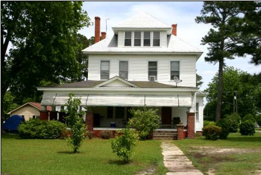
Property 501167: Crump-Hill House, ca. 1922, 14 Virginia Avenue. 0501167
