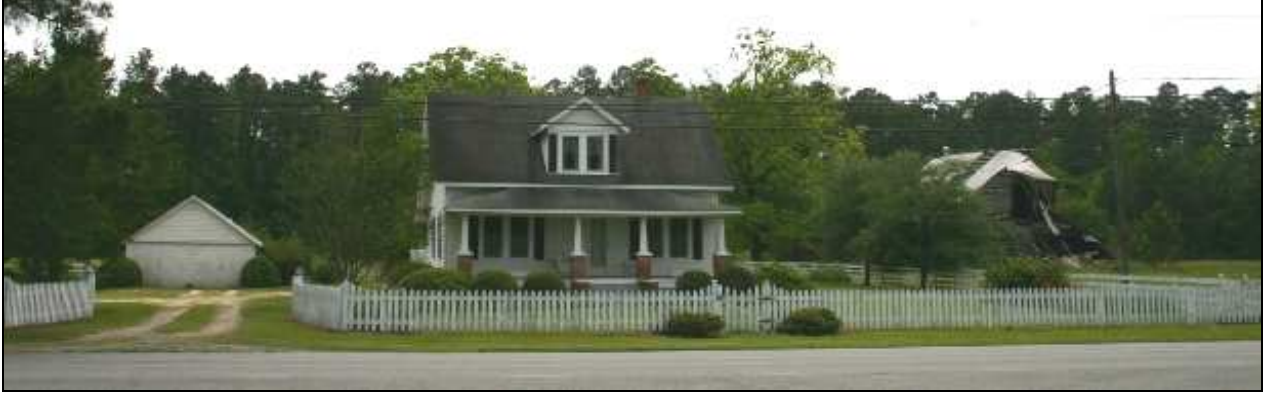
Figure 56: Johnnie Temple Farm, front overall view. Penne Sandbeck, NCDOT, May 2009.
