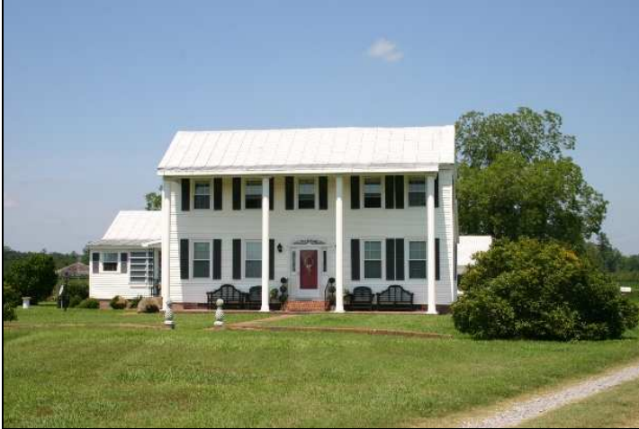
Figure 76: James W. Hill Farm, front elevation. Penne Sandbeck, NCDOT, August 2009.
