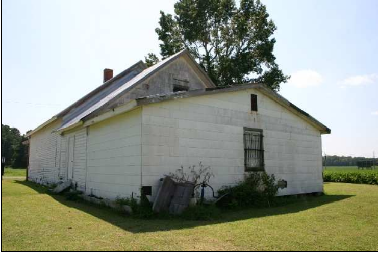
Figure 37: Perry-Harris-Jones Store, east and north elevations.
