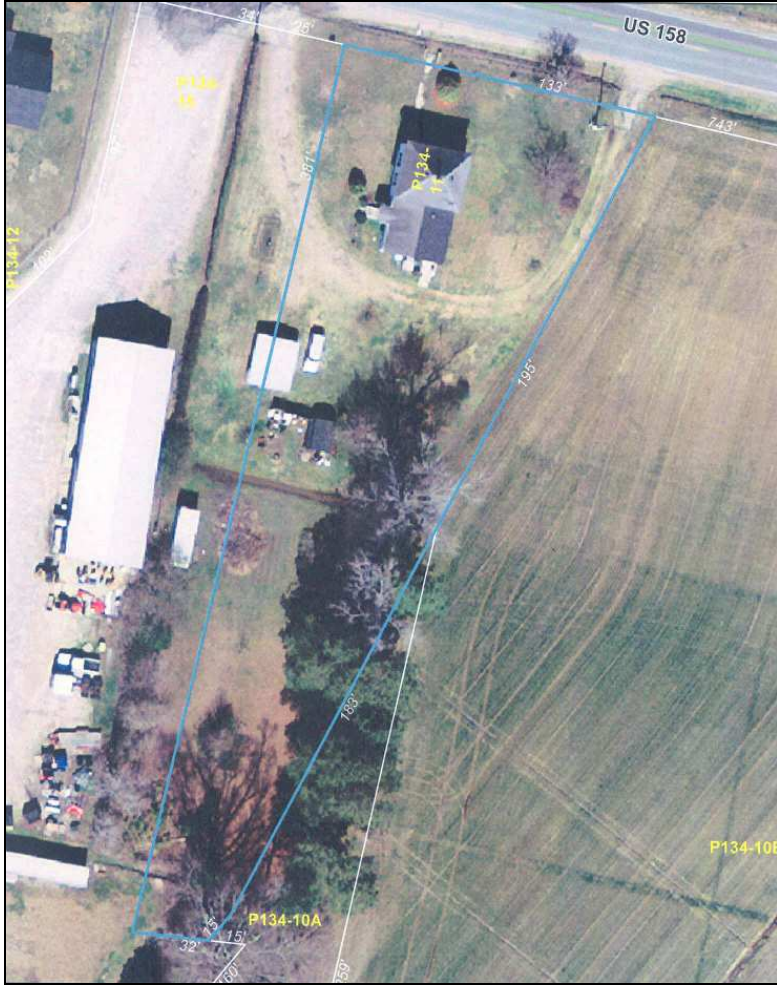
Figure 70: Sawyer House, aerial view from Pasquotank County GIS maps (blue line is parcel boundary), 2008.
