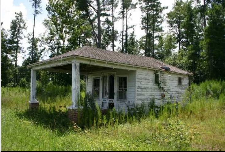
Figure 43: Country Store, N. Winfall vic., north and front elevations.
