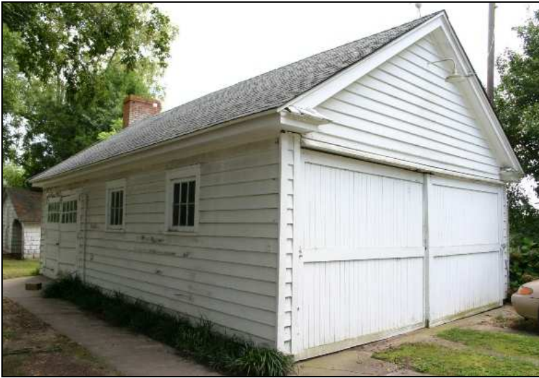
Figure 21: Garage, front and east elevations
