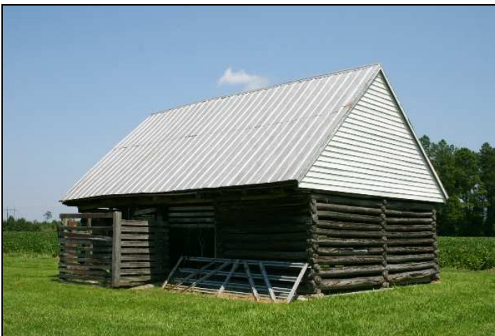
Figure 78: James W. Hill Farm, log barn. Penne Sandbeck, NCDOT, August 2009.
