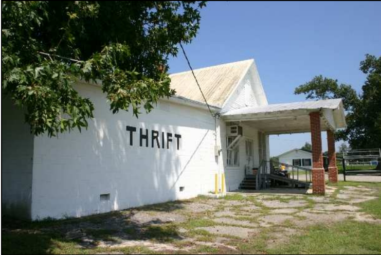
Figure 39: Perry-Harris-Jones Store, front elevation from west angle.
