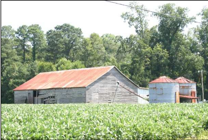
Figure 63: William J. Spence House, frame barn and silos. Penne Sandbeck, NCDOT, August 2009.
