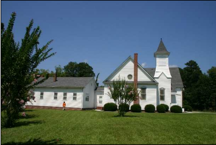
Figure 45: Newland United Methodist Church, south elevation (1949 annex in foreground). Penne Sandbeck, NCDOT, August 2009.
