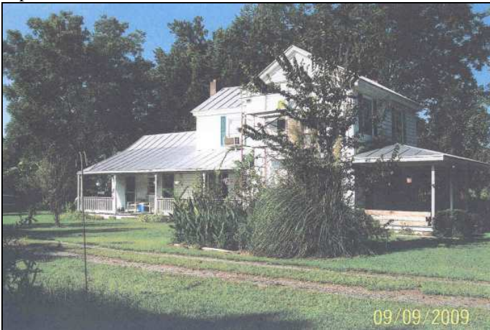
Figure 83: Benjamin F. Pierce House, east elevation, Madelin Becker, Sunbury, NC, September 2009.
