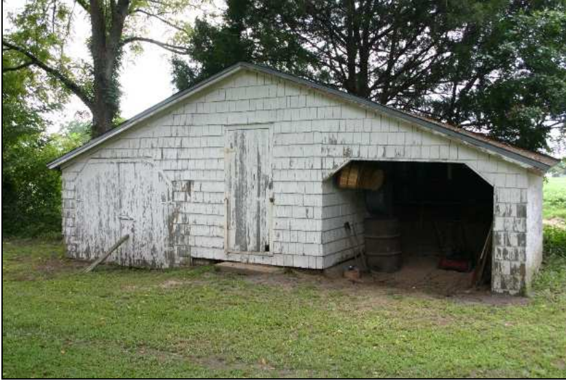
Figure 22: Moses R. White, Jr., House, shed
