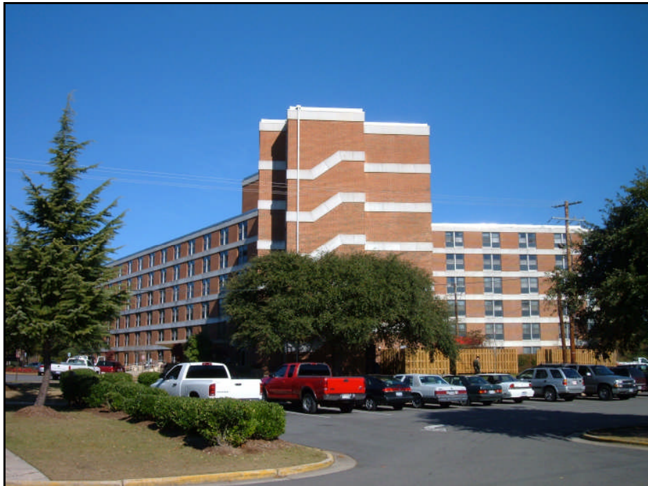
South elevation of Building D-3601 showing its “Y” shaped configuration.
