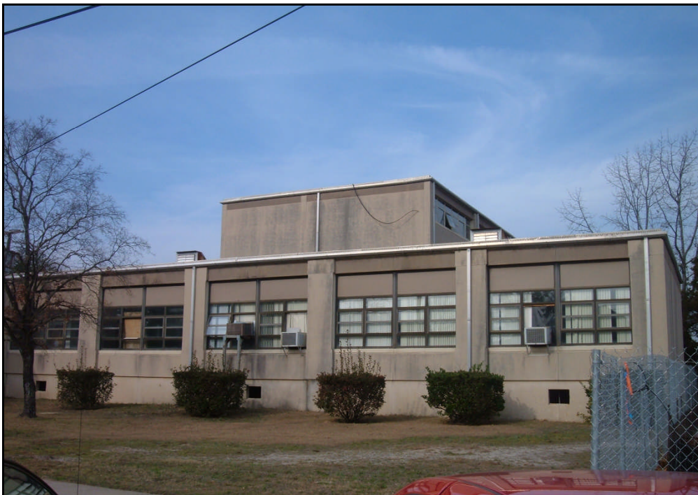
South elevation of the one-story wing on Building C-6525.
