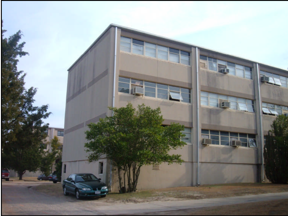
West and north elevations of Building C-6525.
