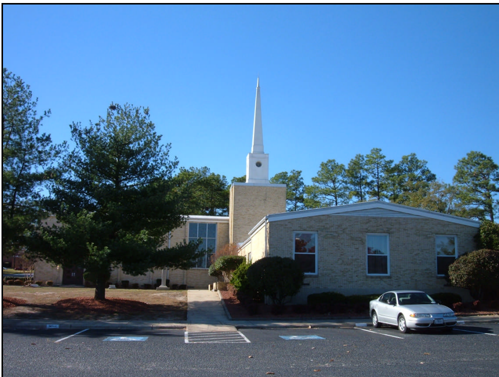
Figure 19: Building D-3116, John F. Kennedy Memorial Chapel, east elevation.
