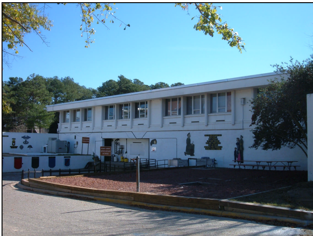
Figure 15: Kennedy Hall, north elevation.
