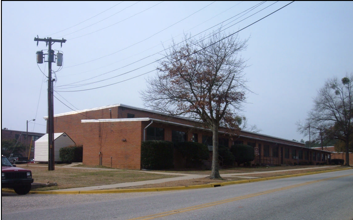
Building D-3022, north and east elevations.
