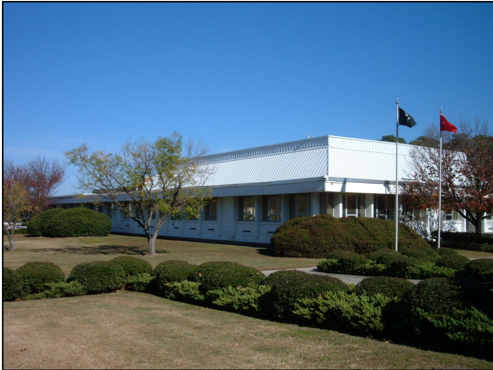
Figure 12: Kennedy Hall, south and west elevations.
