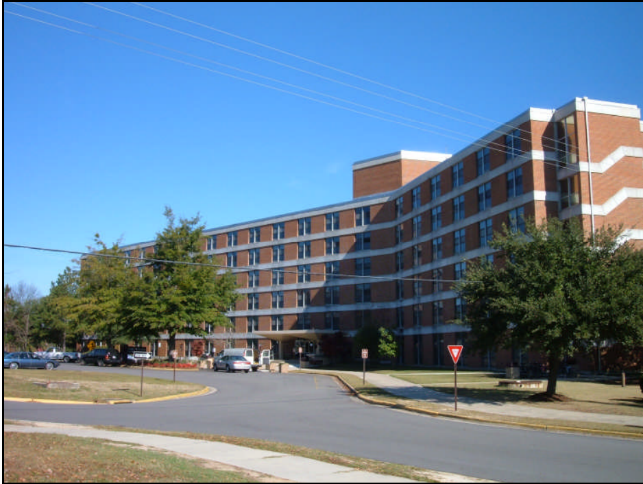
Building D-3601, Moon Hall, south and west elevations.
