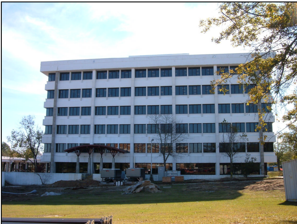
Figure 17: Building D-3206, Bryant Hall, view of the north elevation.
