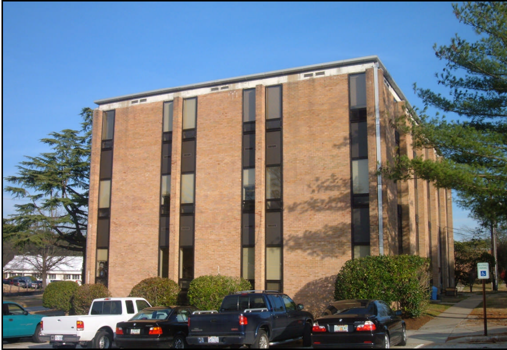
Building D-2609, south and west elevations.
