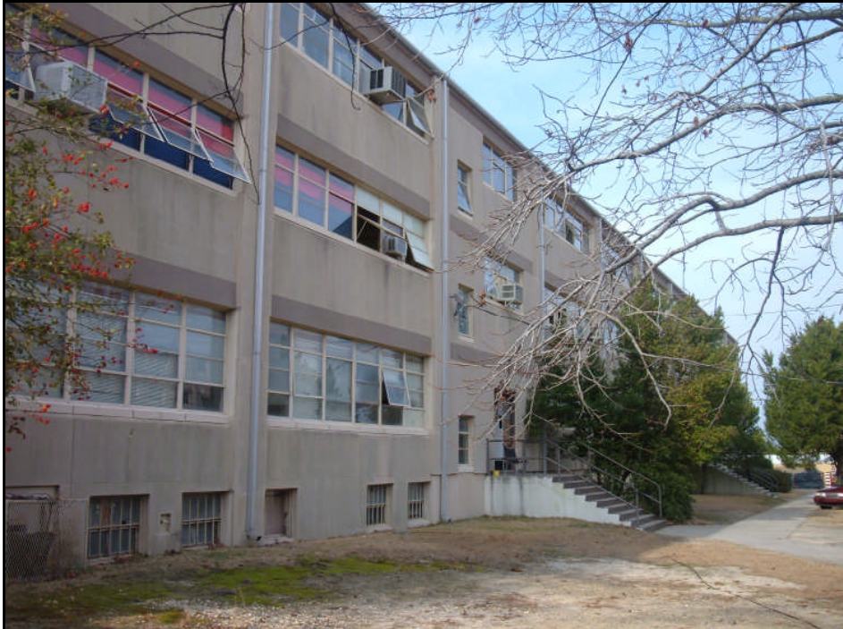
East elevation of Building C-6525.
