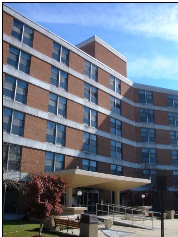
Building D-3705, main entrance on the east façade.
