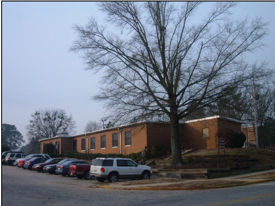
Building D-2612, north and east elevations.
