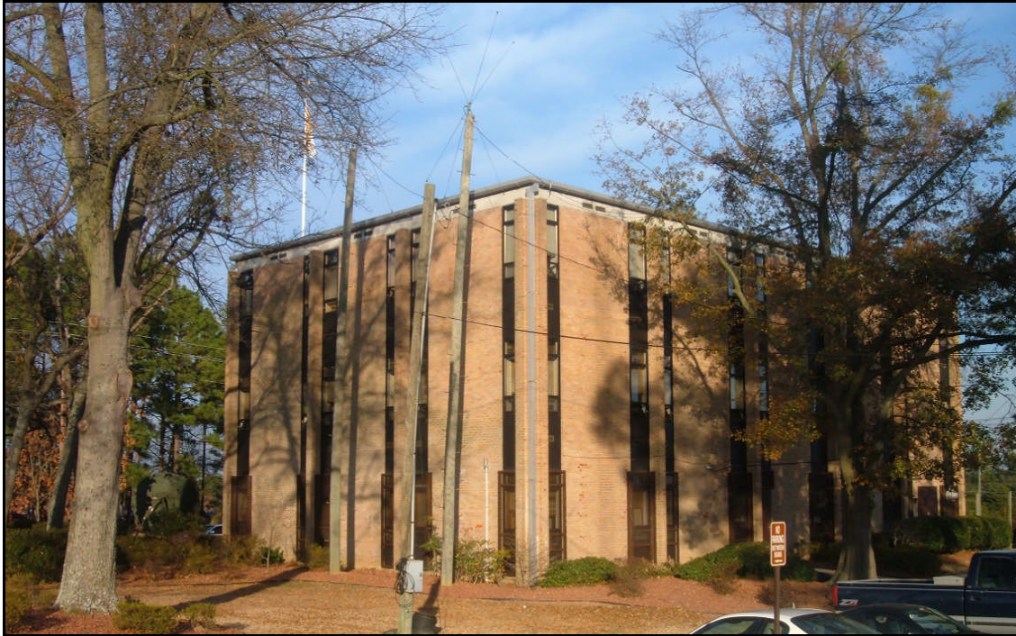
Building D-2919, south and west elevations.
