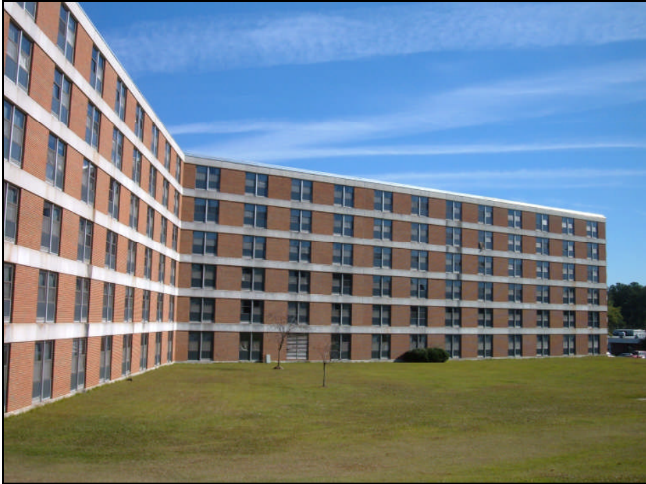
Building D-3705, west elevation.
