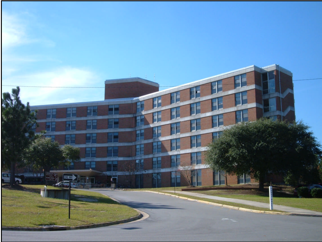
East and north elevations of Building D-3705.
