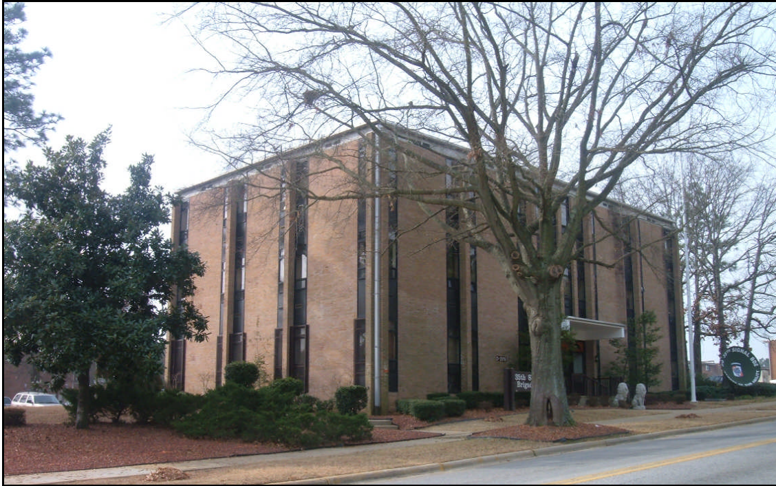
Building D-2919, north and east elevations.
