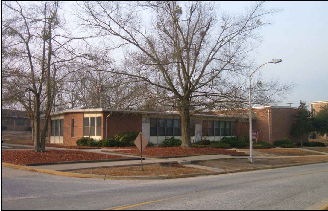
Building D-2507, north and east façades.
