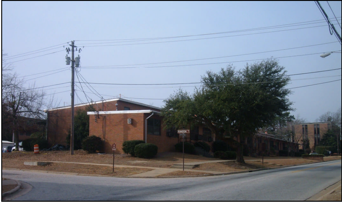
Building D-2815, north and east elevations.
