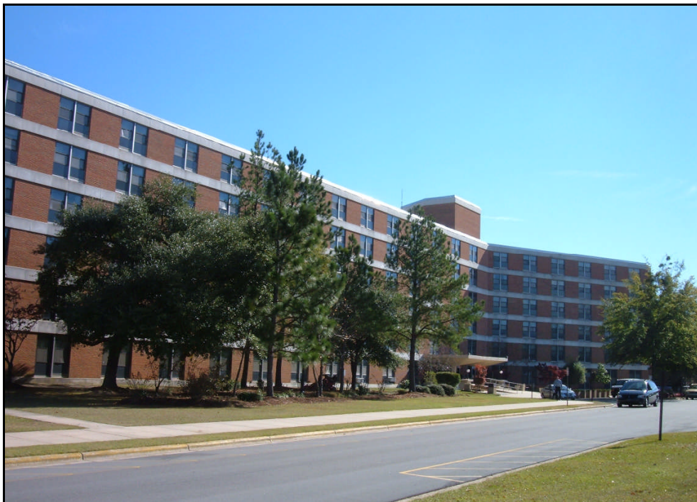
West elevation of Building D-3601.
