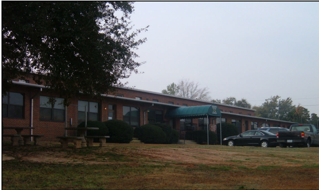
Building D-2302, north façade.
