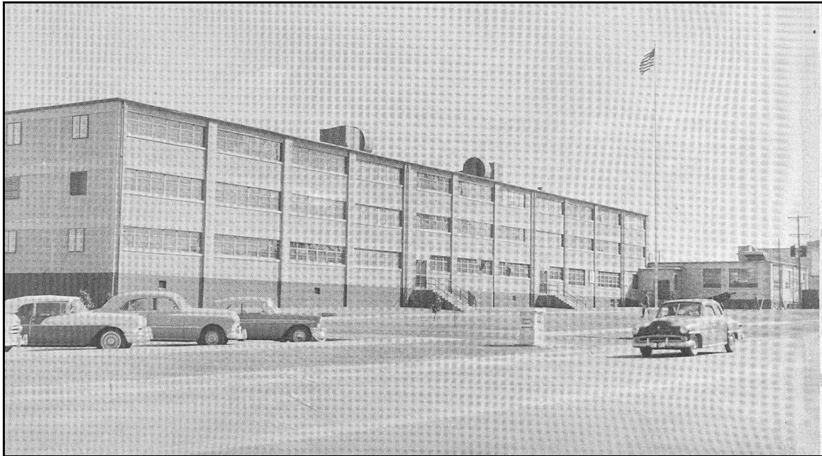
Building C-6525 in 1958, (Photo courtesy of the 82 nd Airborne Division Museum).
