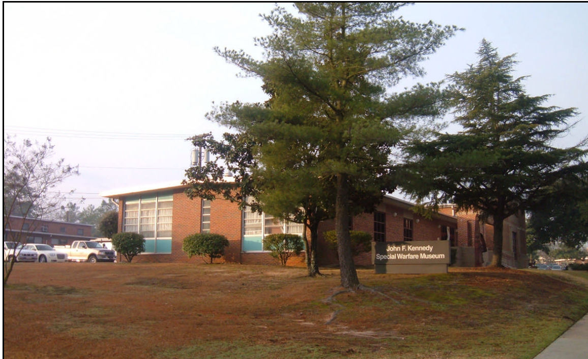
Building D-2502, north and east elevations.
