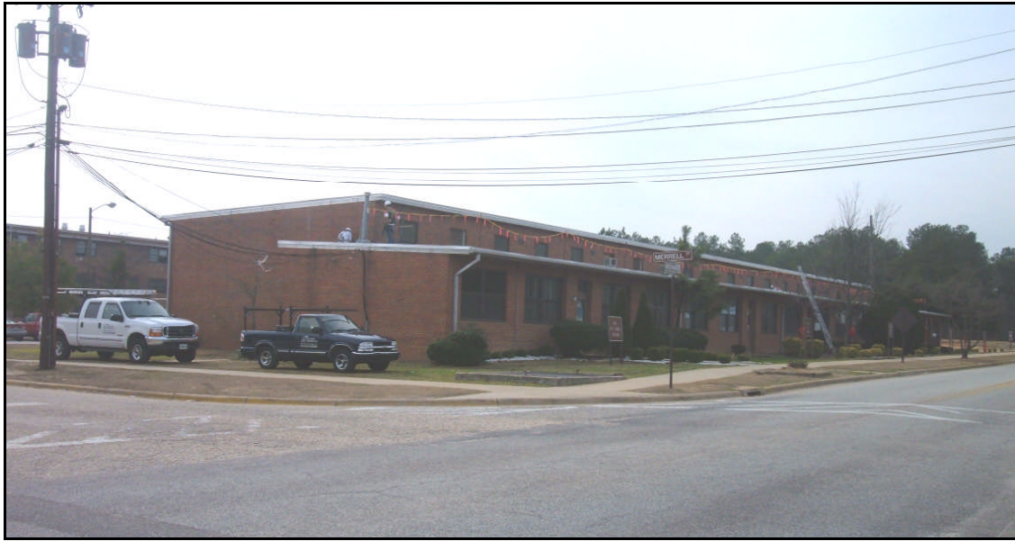
Building D-3225, north and west elevations.
