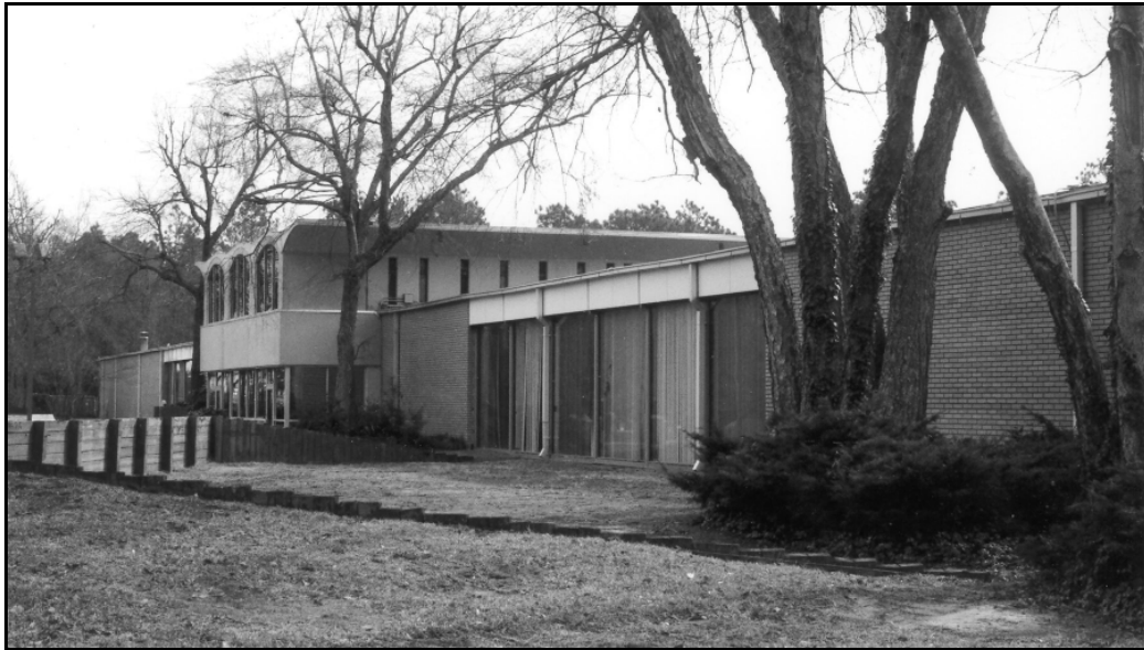
View of the main (north) façade of Ridgway Hall.
