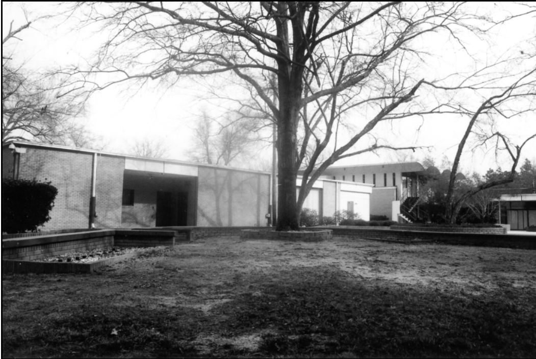
South elevation of Ridgway Hall.
