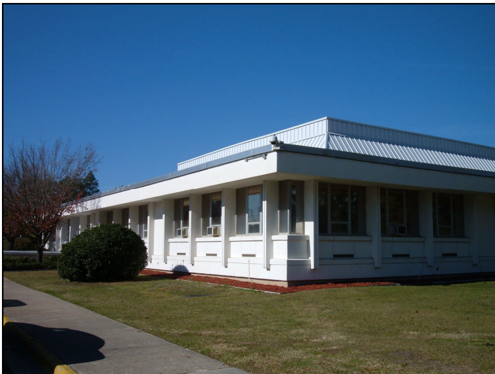
Figure 13: Kennedy Hall, south and east elevations.
