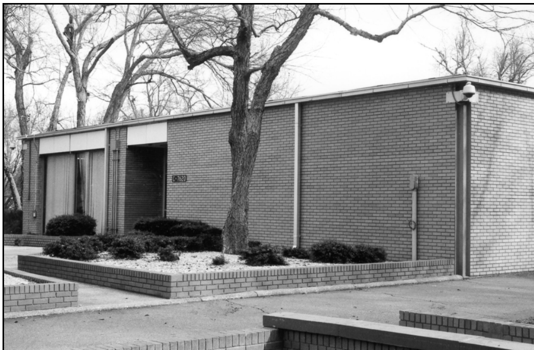
West elevation of Ridgway Hall.
