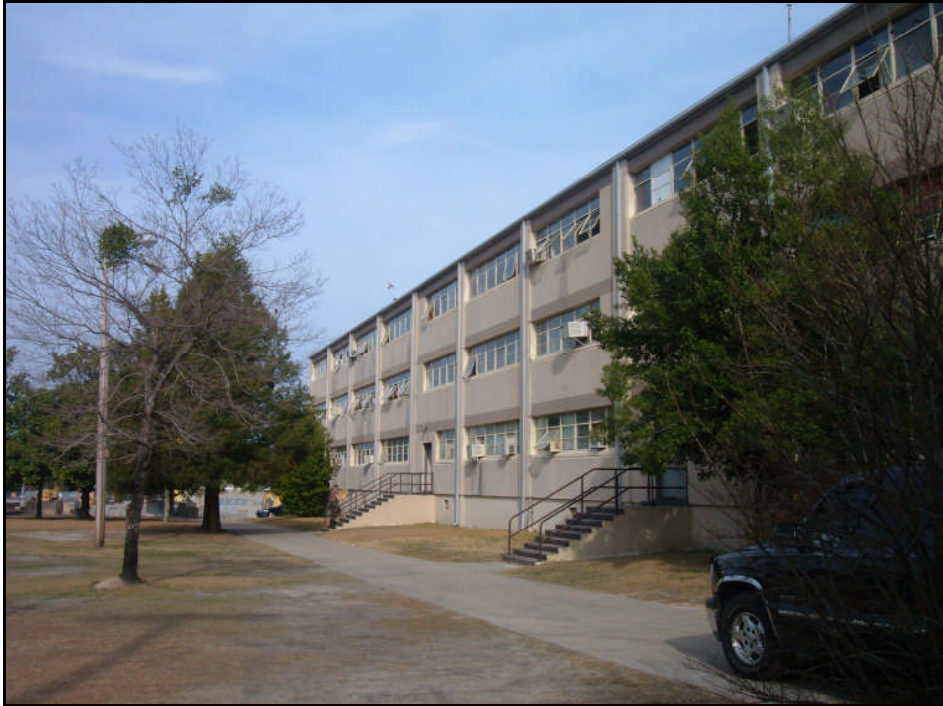
Building C-6525, west façade.
