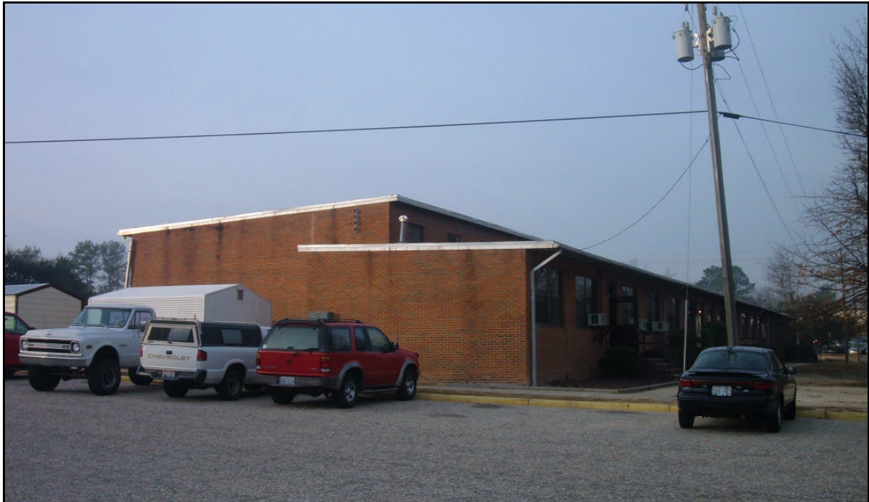
Building D-2307, north and east elevations.
