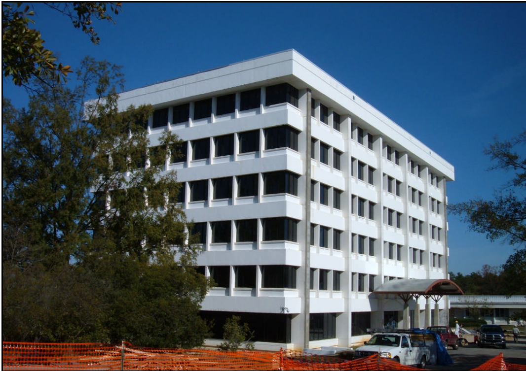
Figure 16: Building D-3206, Bryant Hall, north and west elevations.
