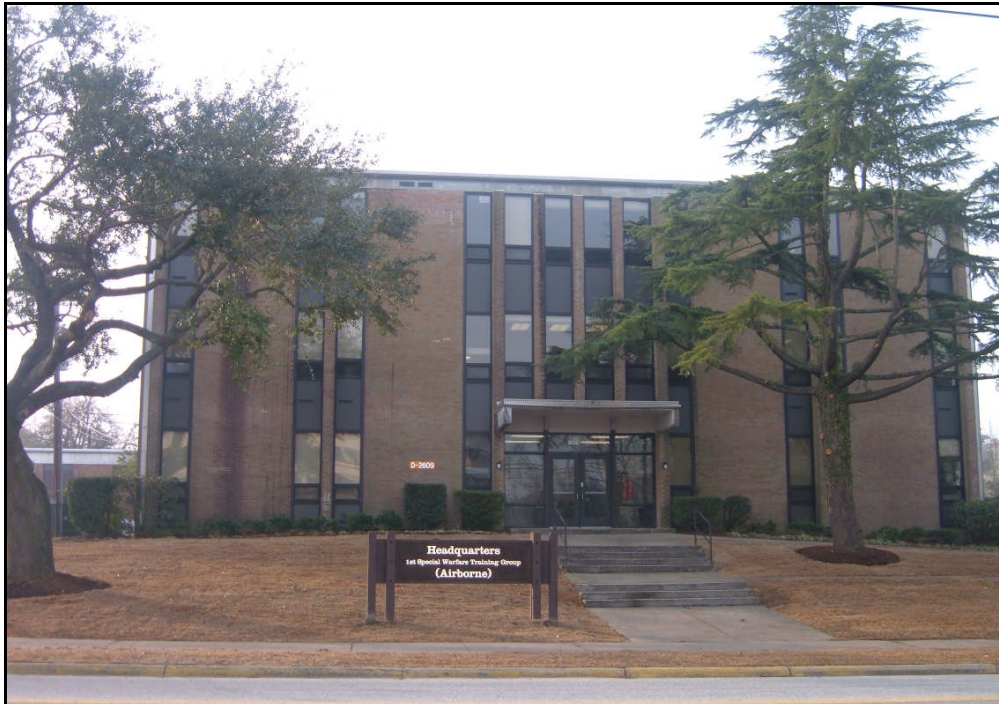
Building D-2609, north façade.
