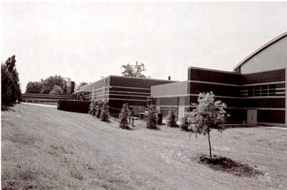
Plate 42: Former West Charlotte High School – looking southeast at modern classroom blocks and barrel-roofed gymnasium
