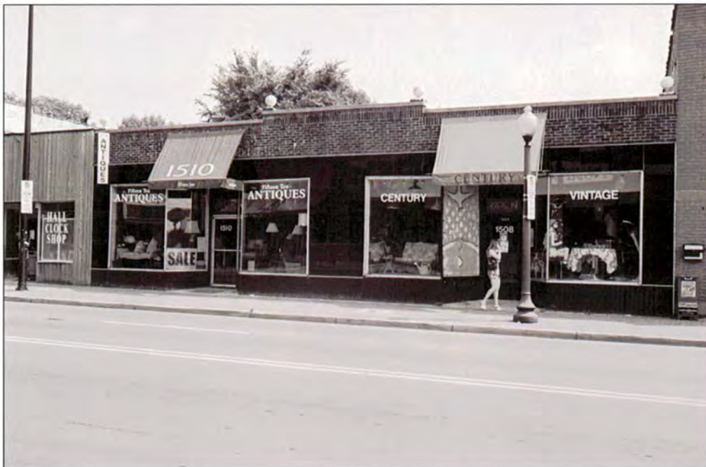
Plate 54: Central Avenue Commercial Historic District – looking southeast at Century Vintage Antiques and Fifteen Ten Antiques at 1508 and 1510 Central Avenue
