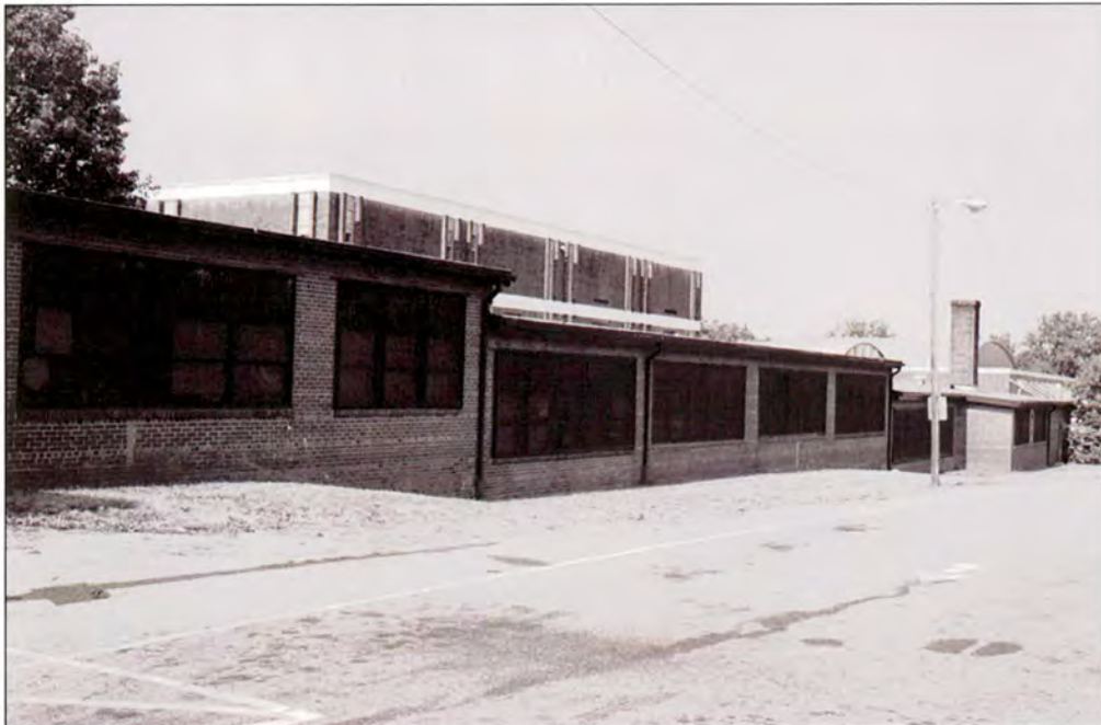
Plate 40: Former West Charlotte High School – looking southwest at 1950s one- and two story classroom wings; at right, flanking chimney stack, are barrel roofs of 1950s and modern gymnasium
