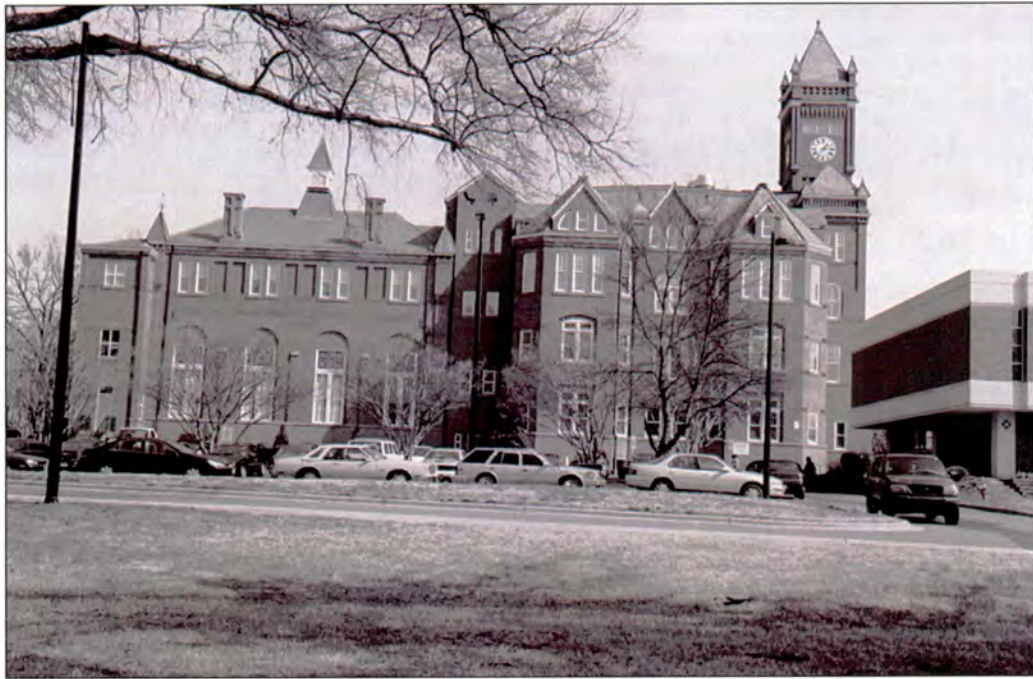
Plate 17: Johnson C. Smith University Historic District, Biddle Memorial Hall – Beatties Ford Road elevation
