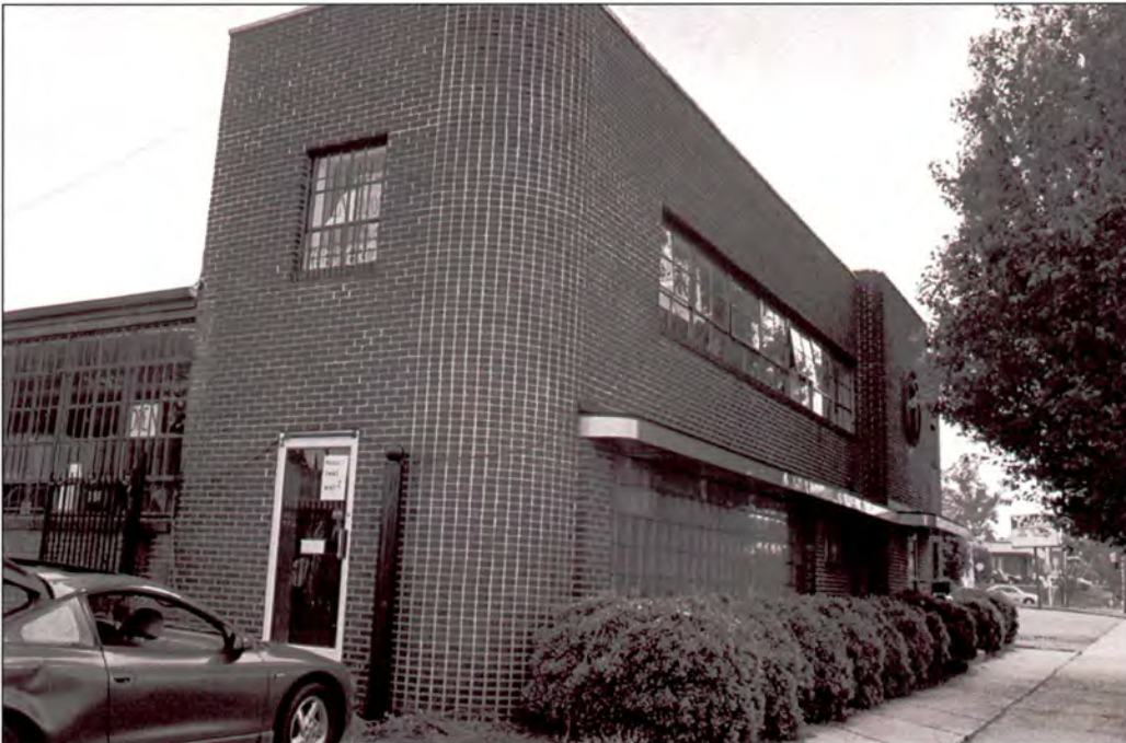
Plate 84: Former Queens Pie Company Building – east side and north (Central Avenue) front elevations
