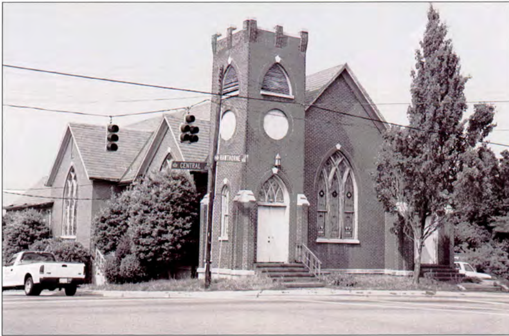
Plate 81: Former First Methodist Protestant Episcopal Church – south front and west side (Hawthorne Lane) elevations
