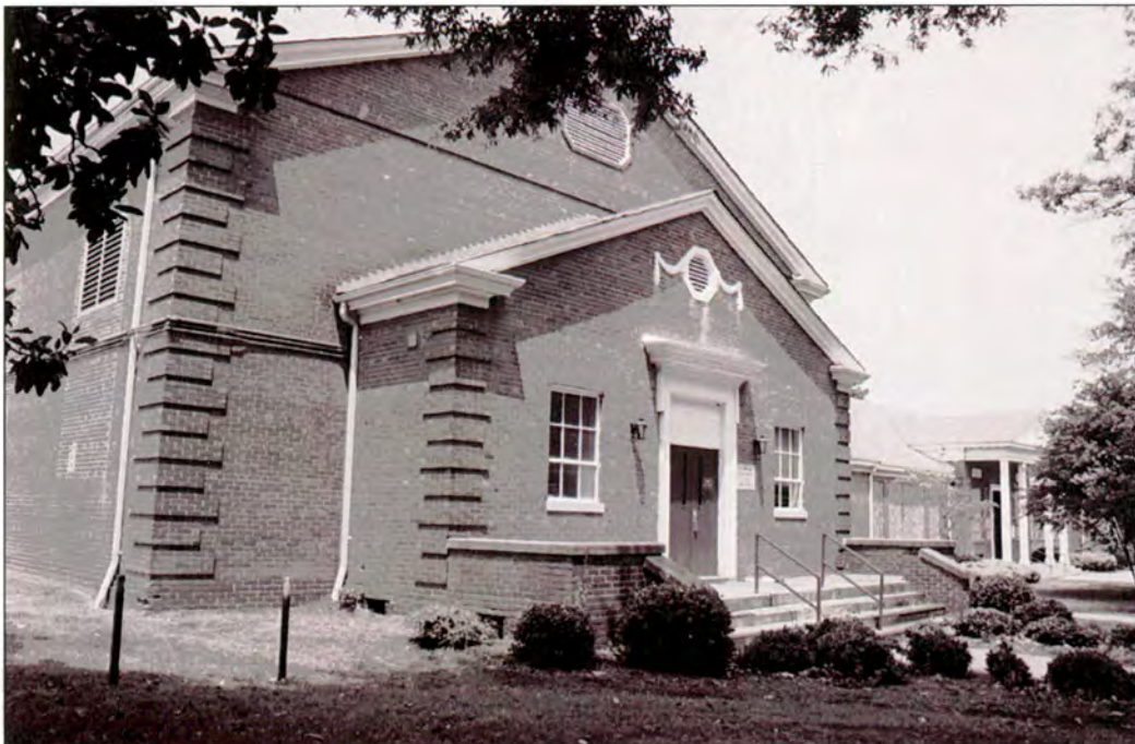
Plate 61: Former Midwood School – Central Avenue elevations of 1941 auditorium/gymnasium at left and 1935 classroom block at right
