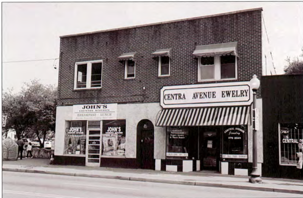
Plate 56: Central Avenue Commercial Historic District – looking southeast at Central Avenue Jewelry and John’s Country Kitchen at 1516 and 1518 Central Avenue
