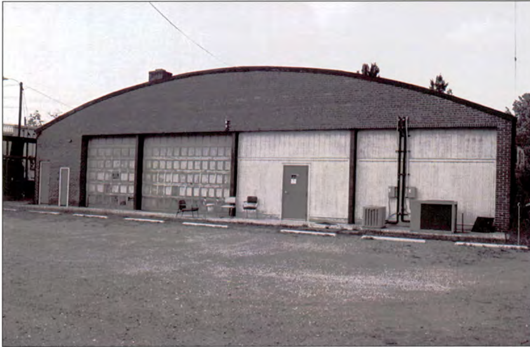
Plate 85: Former Queens Pie Company Building – south rear elevation
