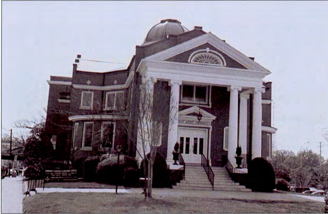
Plate 6: (Former) East Avenue Tabernacle Associated Reformed Presbyterian Church – east front elevation
