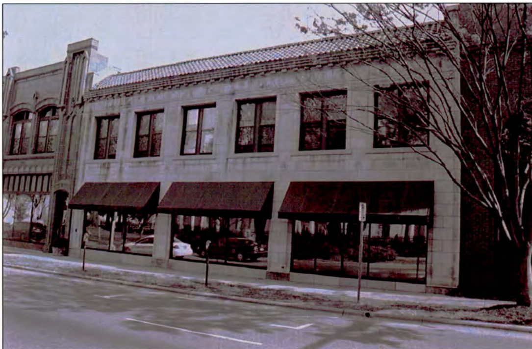
Plate 22: Fourth Ward Historic District, Gateway Building – West Trade Street elevation
