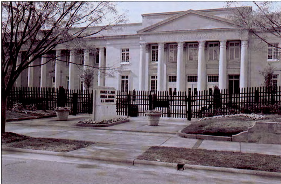
Plate 3: Charles R. Jonas Federal Building – north front (Trade Street) elevation
