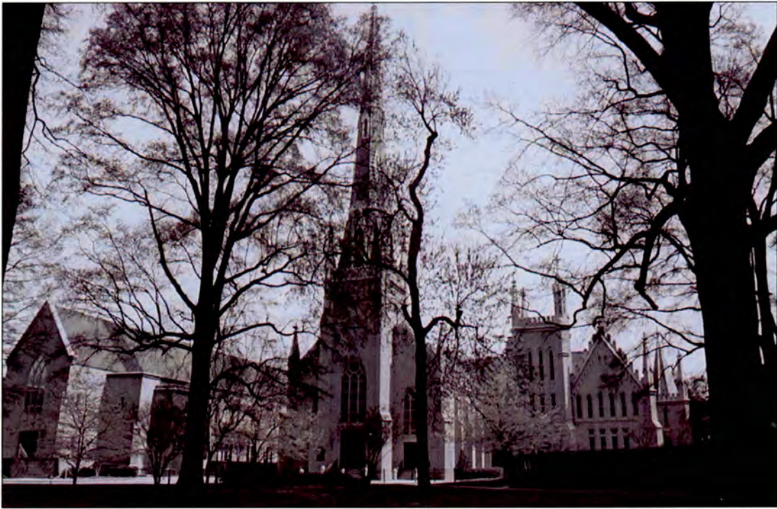
Plate 4: First Presbyterian Church – south front (Trade Street) elevation
