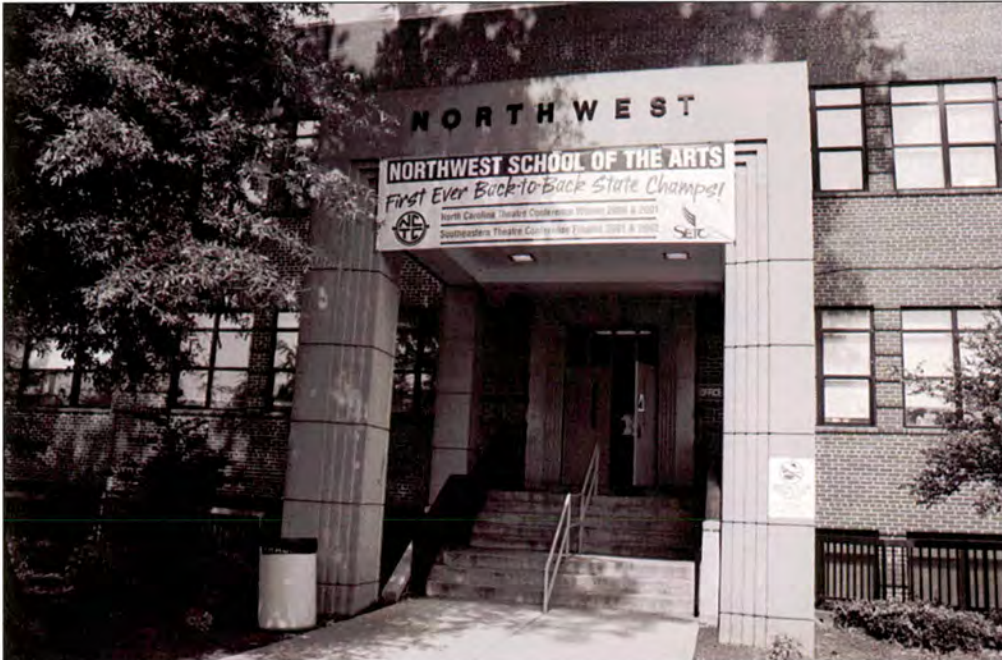
Plate 38: Former West Charlotte High School – front portico of original classroom block
