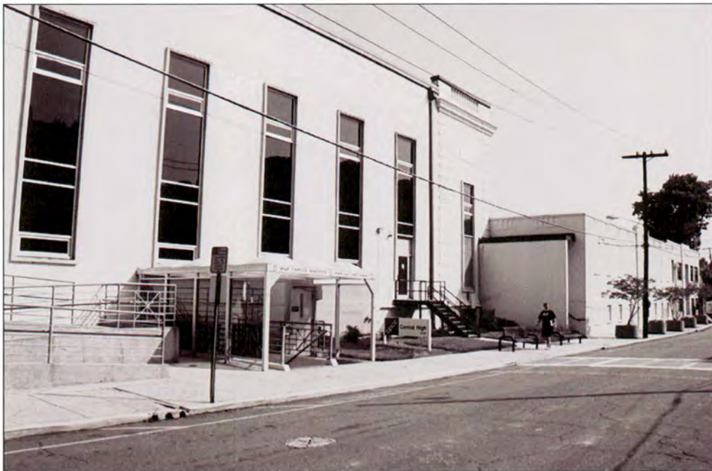
Plate 77: Former Central High School – Pease Lane elevations of auditorium at left, and gymnasium at right; note altered windows and finish and remnant of balustrade and quoins at rear of auditorium
