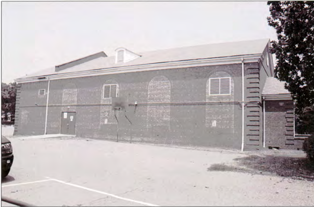
Plate 60: Former Midwood School – east side elevation of 1941 auditorium/gymnasium
