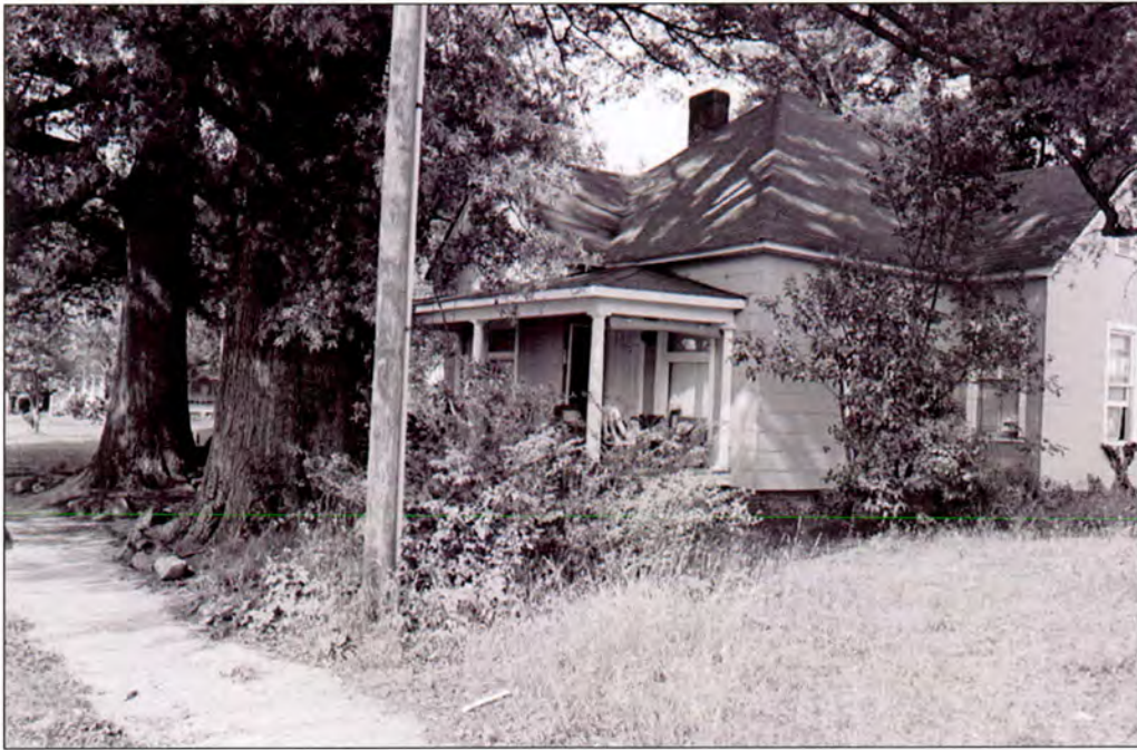
Plate 36: Plaza-Midwood local historic district, Clement Avenue resources – 1116 at right and 1200, barely visible, at far left
