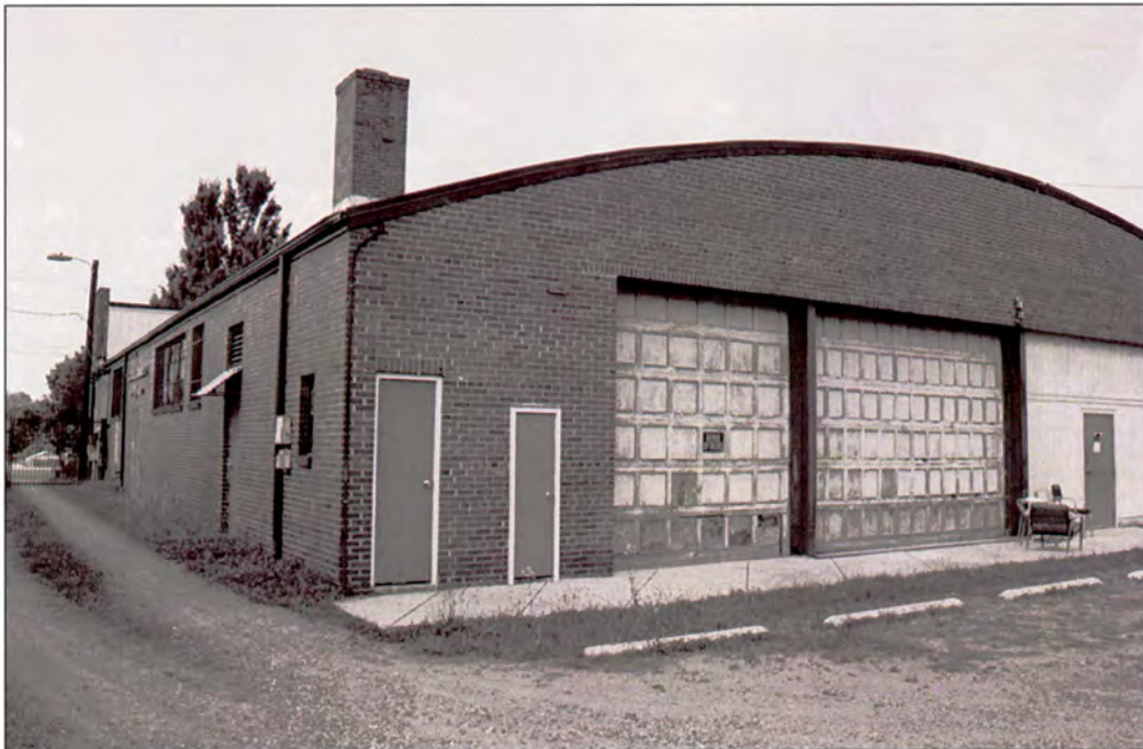
Plate 86: Former Queens Pie Company Building – west side and south rear elevations
