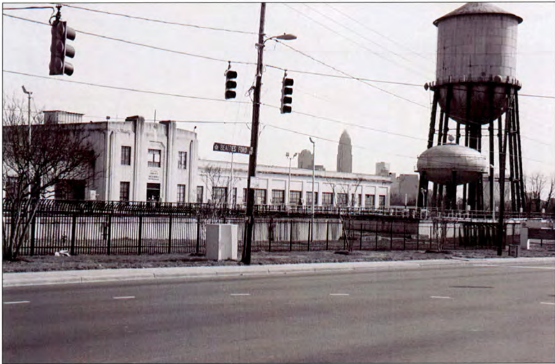
Plate 30: Charlotte Water Works / Vest Station – Beatties Ford Road elevation
