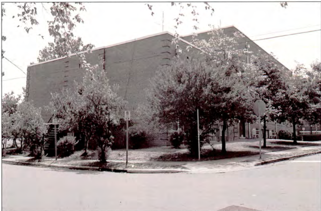
Plate 65: Former Midwood School – looking southwest from intersection of Nandina Street and Hamorton Place at 1943 wing in foreground and taller 1941 wing to rear
