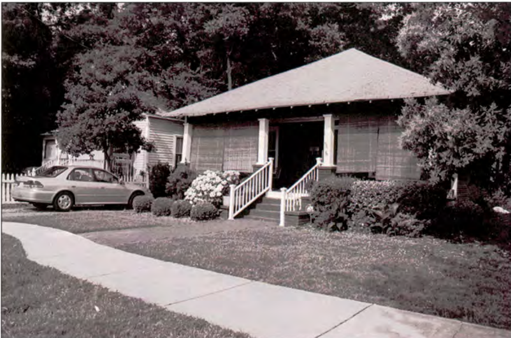
Plate 35: Plaza-Midwood local historic district, Clement Avenue resources – 1204 at right and 1208 at left
