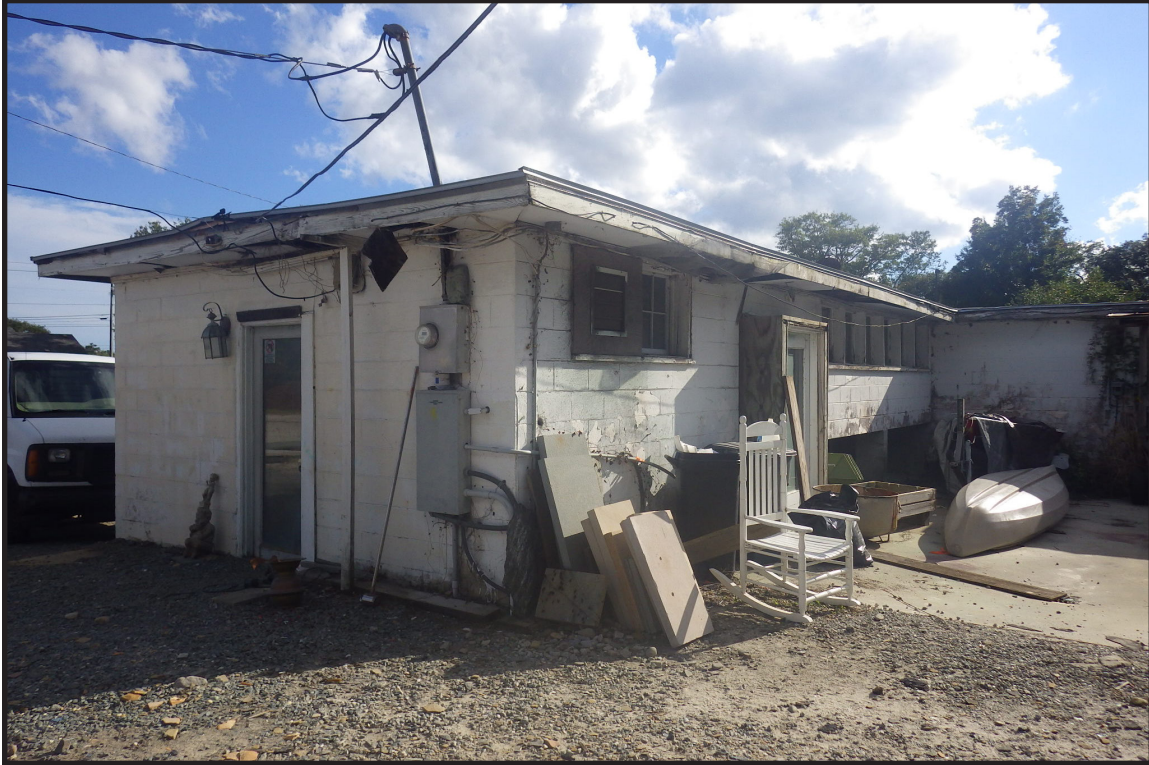
Figure 11. Processing Building, Northeast and Northwest (Rear) Side
