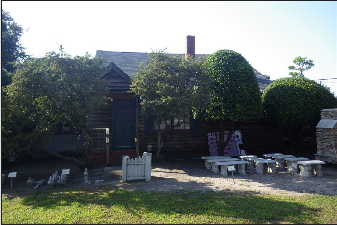
Figure 3. Cornelius Nixon House, Front, Southeast Side
