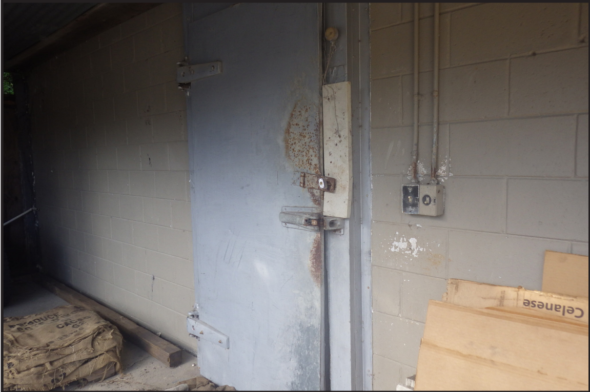
Figure 18. Cooler Building Door
