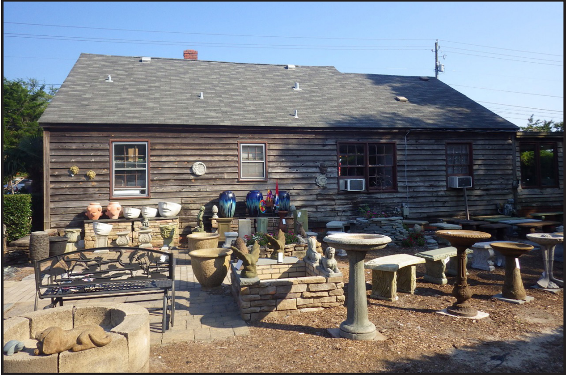
Figure 5. Cornelius Nixon House, Rear, Northwest Side
