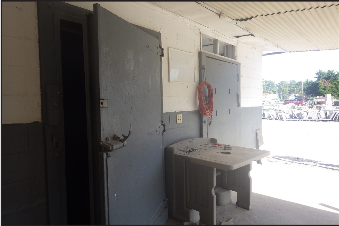
Figure 13. Processing Building, Southwest Side Under Shed Showing Office and Middle Cooler Doors
