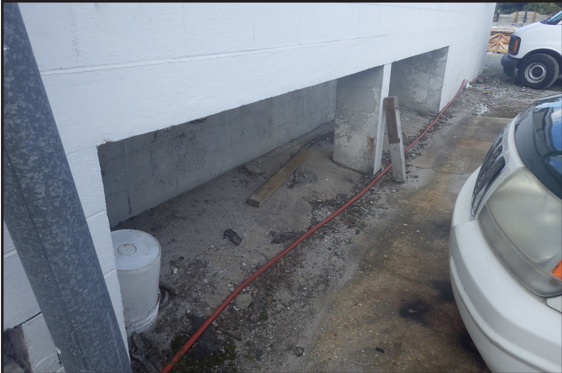
Figure 10. Processing Building, Front Oyster Shell Bays
