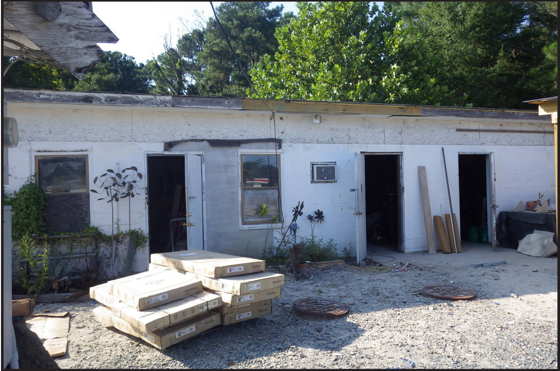
Figure 21. Storage Building, Southeast Side
