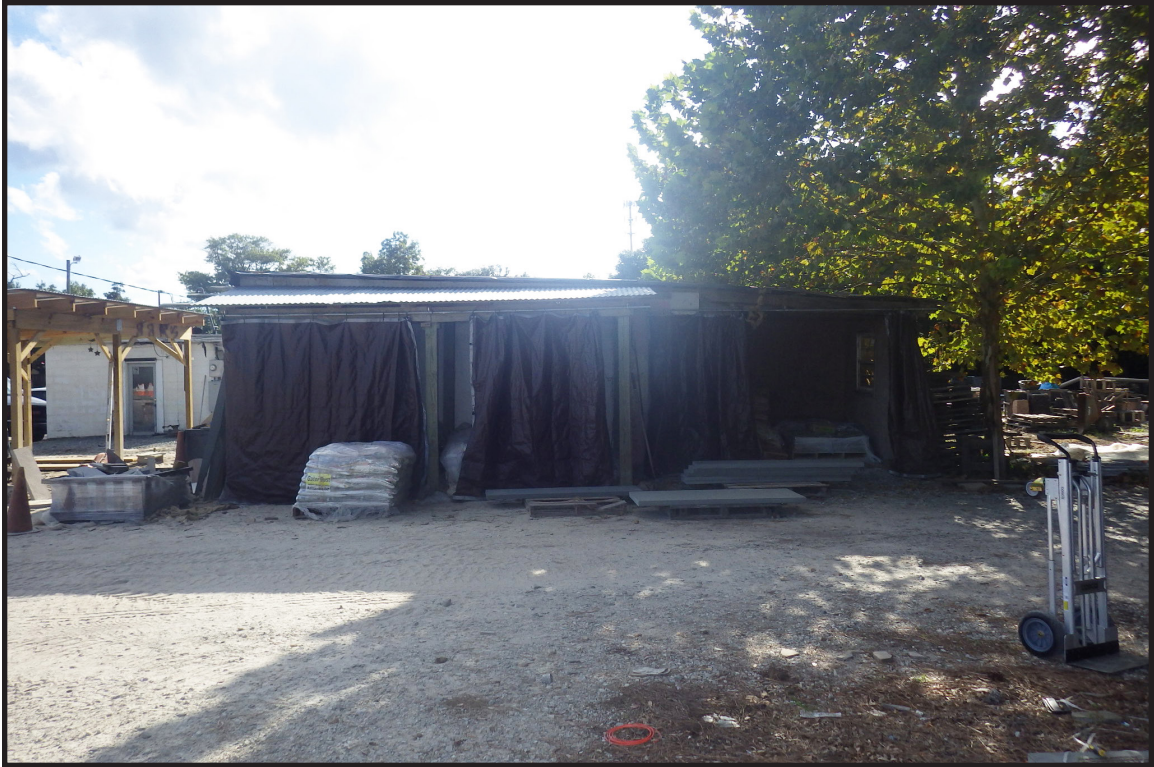
Figure 23. Storage Sheds on Northeast and Northwest Sides
