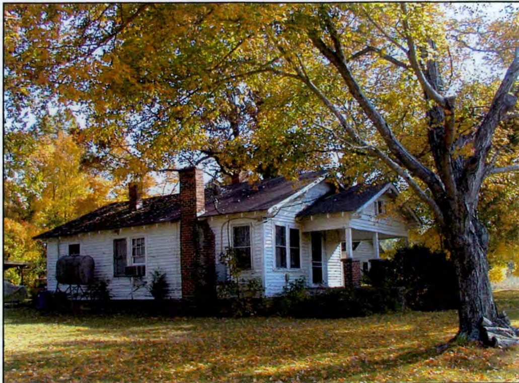
Daniel Smith House looking southeast.
