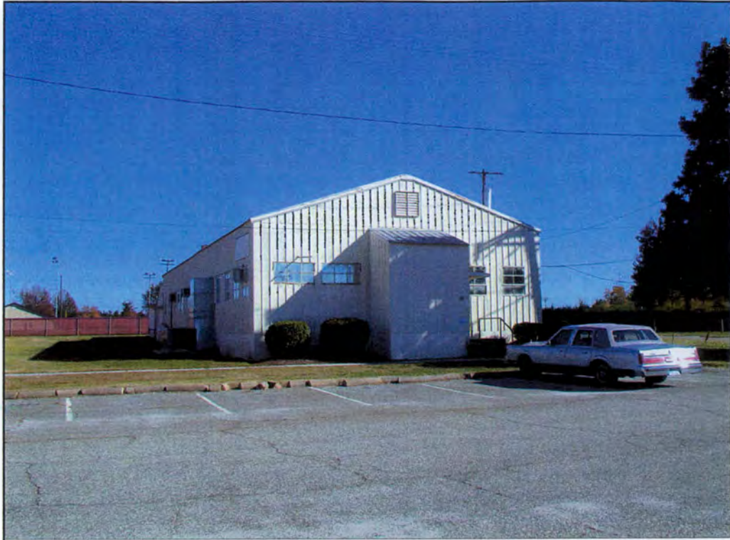
Building (A4) looking northeast.
