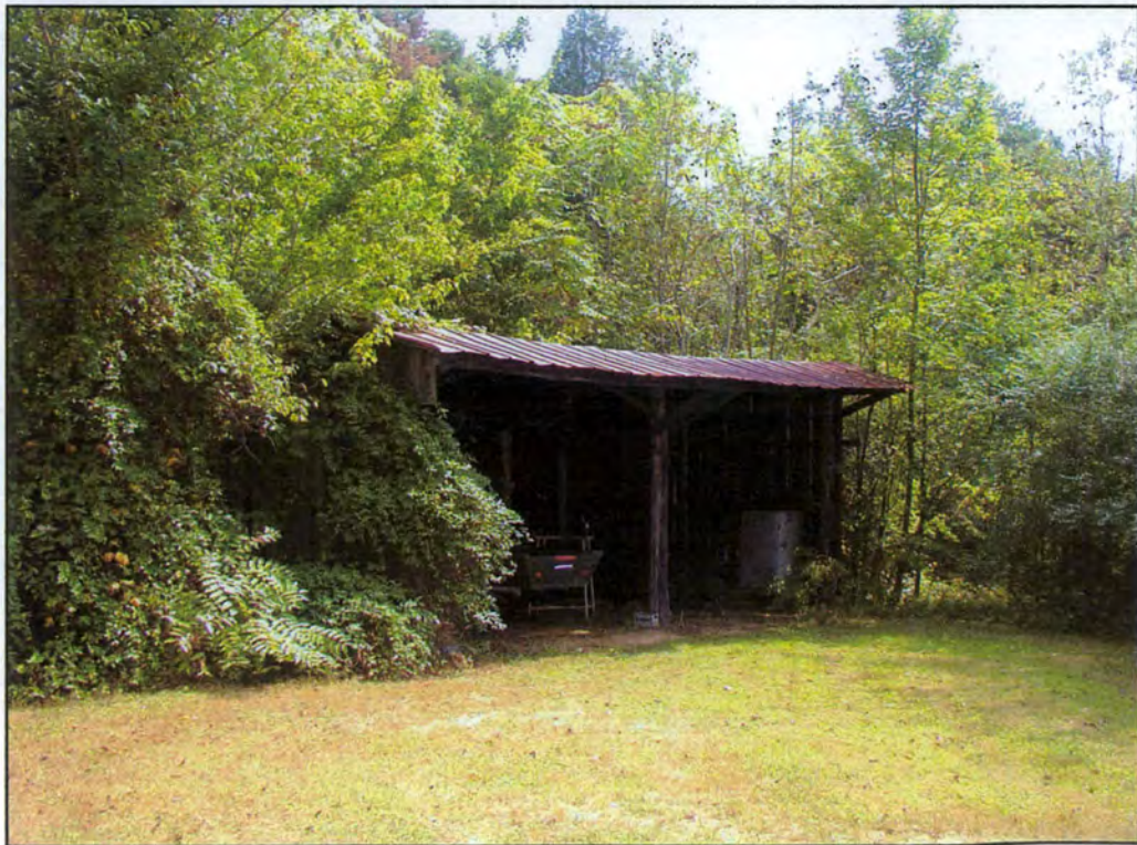
Weavil machine shed (F) looking northeast.
