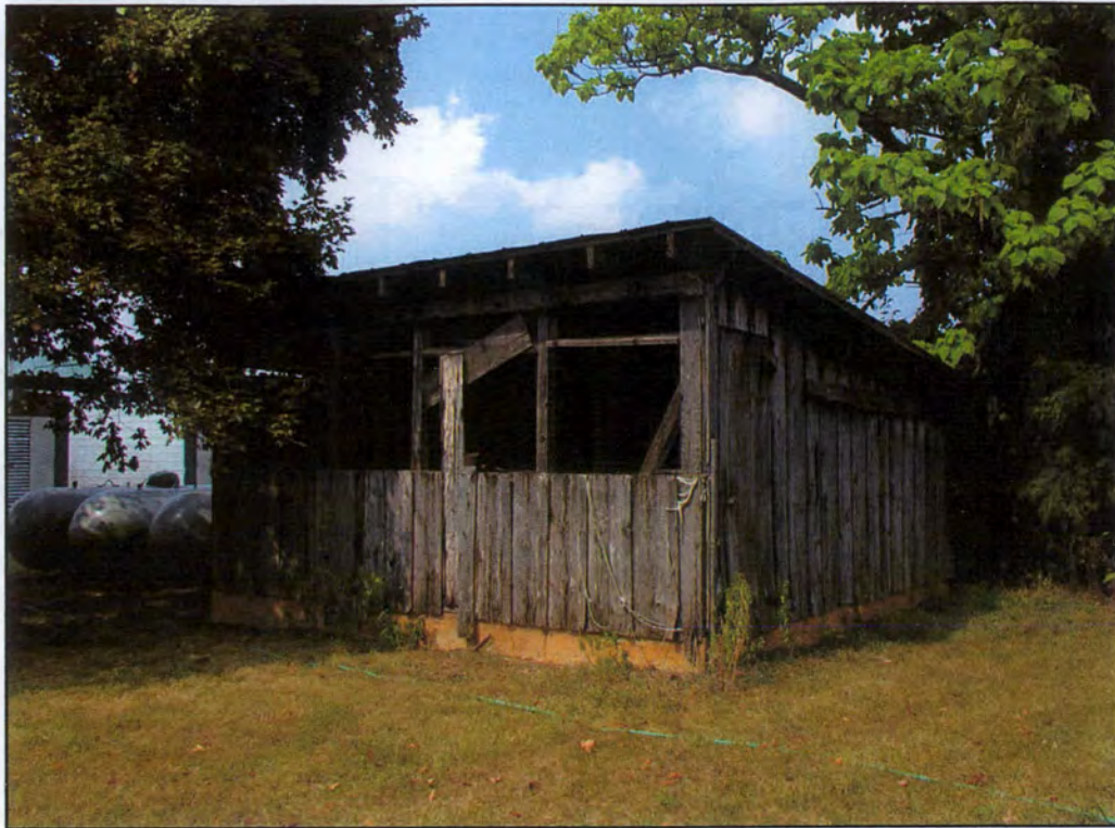
Smith tenant farm chicken house (C) looking northwest.
