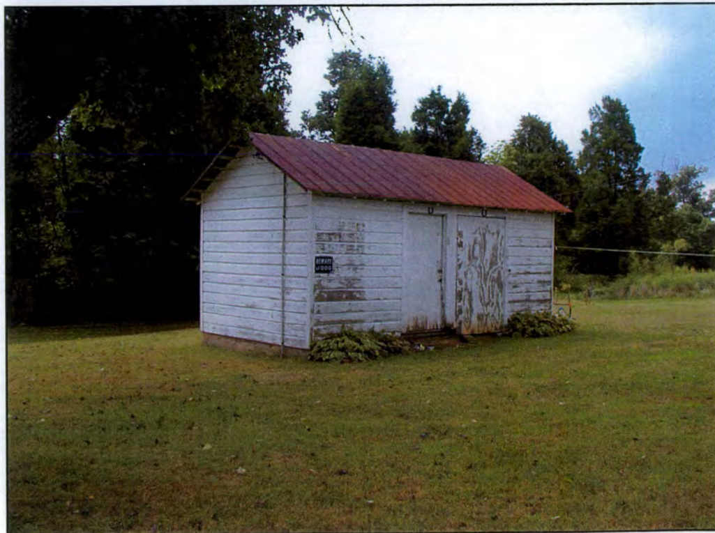
Weavil washhouse (B) looking southeast.
