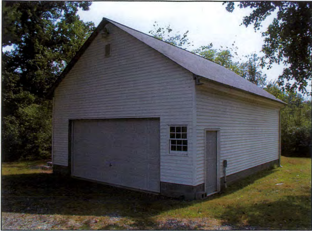
Garage (E) added to Weavil complex looking northeast.
