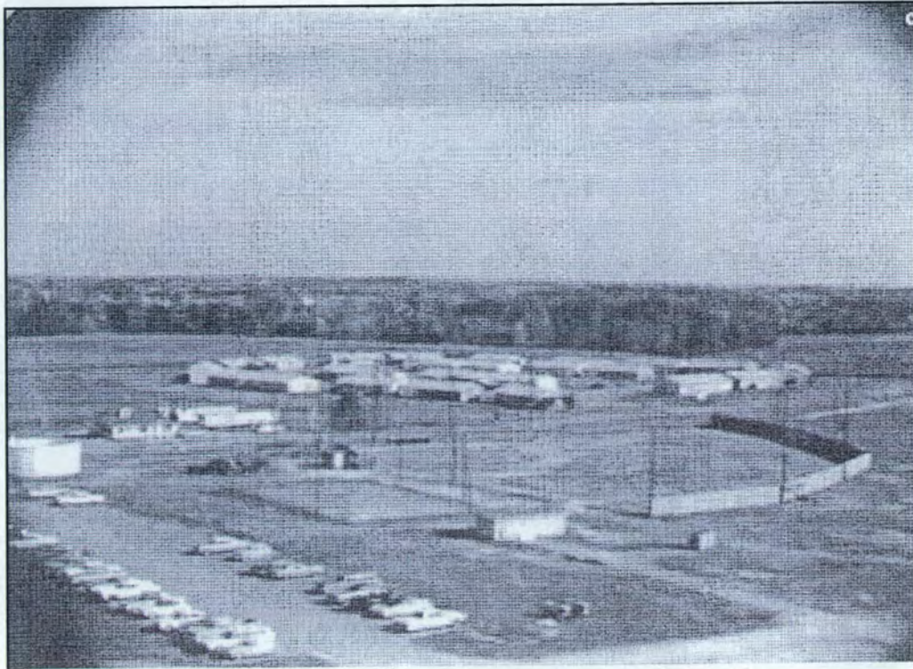
Figure 13. Housing development (B) from radar tower (D1), looking northwest. Baseball field (D2), tennis court (D3), and utility building (D4), are in same approximate locations as those at present-day Union Cross Park.
