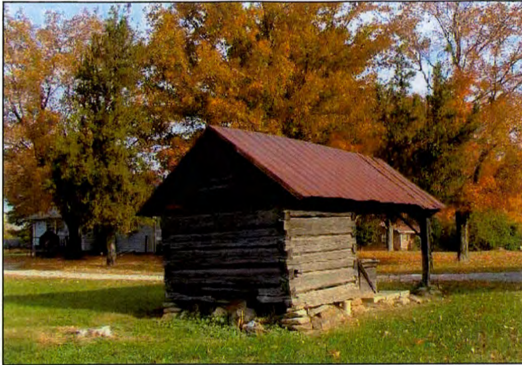
Well house looking northwest.
