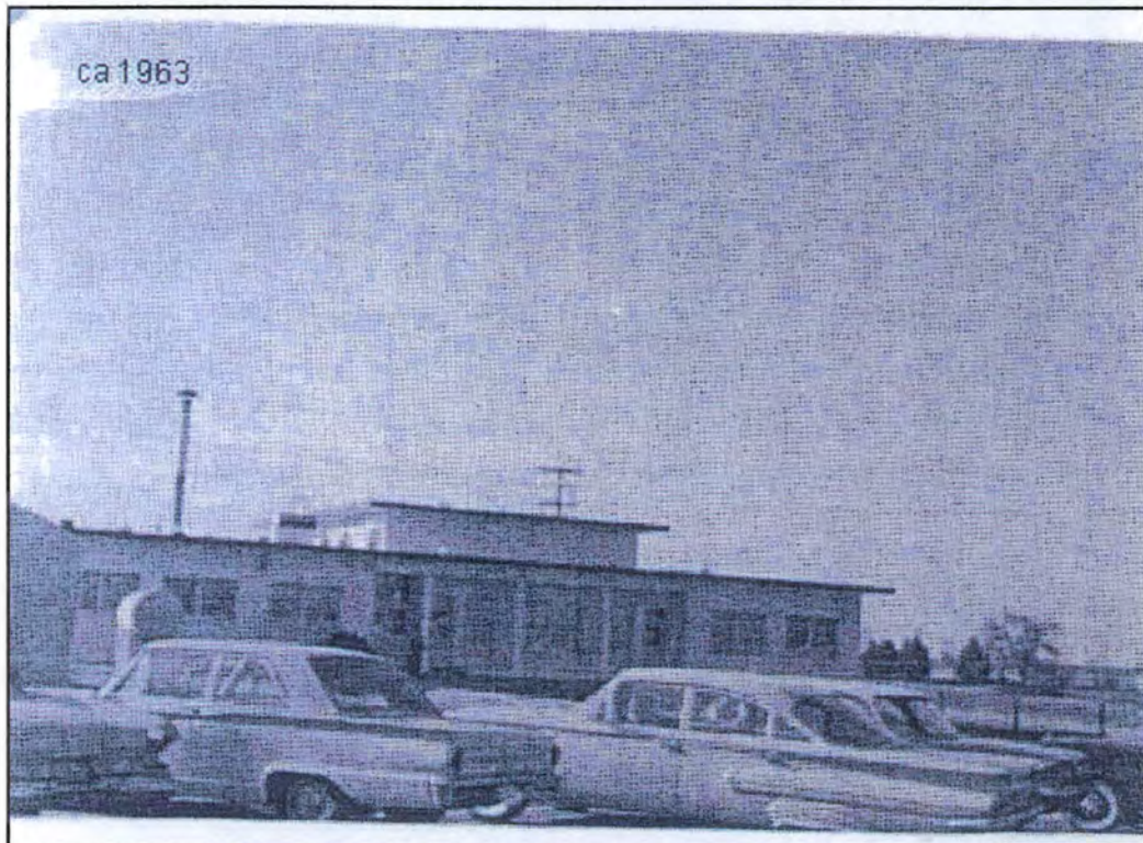
Figure 8. Circa 1963 view of building (A1) looking southwest. The Radomes website identifies this building as the recreation hall, PX, and library.
