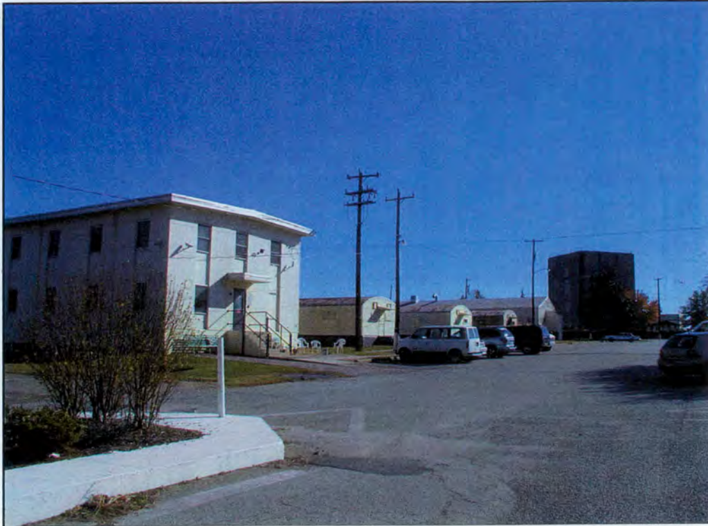
Concrete block building (A2) and Quonset huts (A3), looking northeast towards radar tower (B1) and Wallburg Road.
