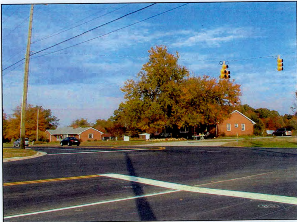
Ina L Smith House (left) and Paul and Ina Jean Tucker Stephens House (right) looking northwest.
