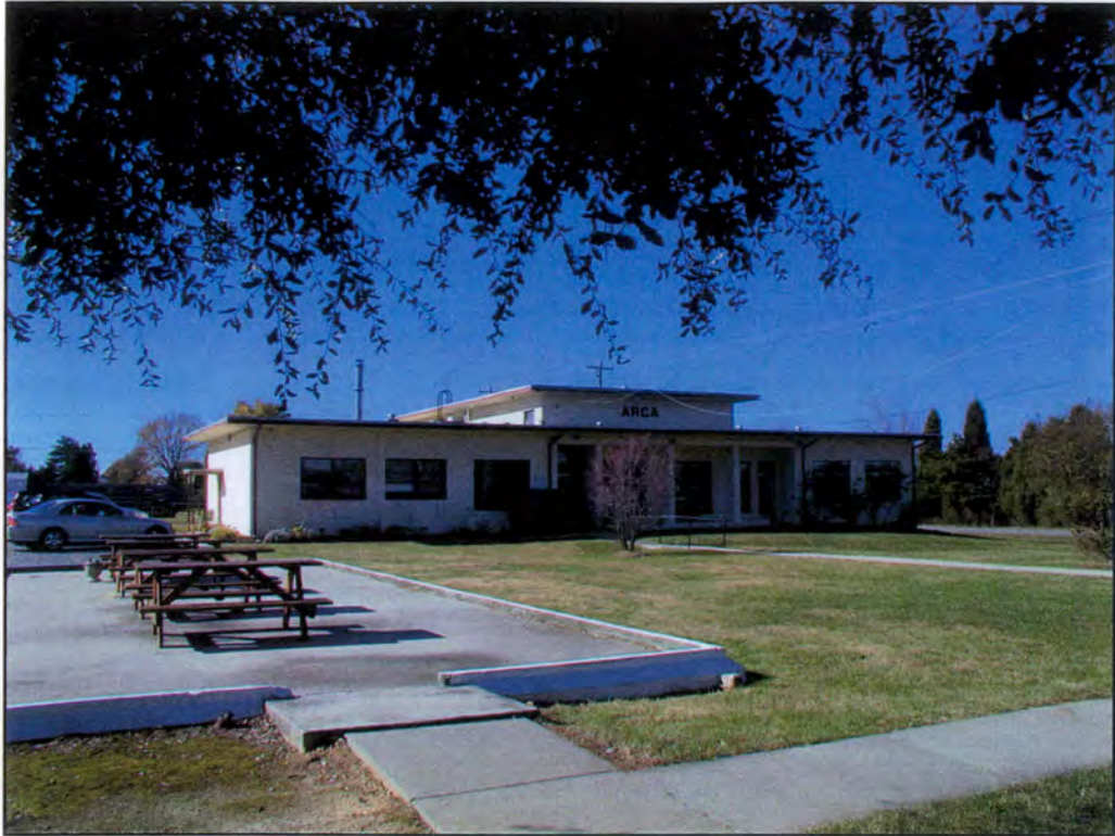
Radar station building (A1), currently administrative offices of ARCA, looking southwest.
