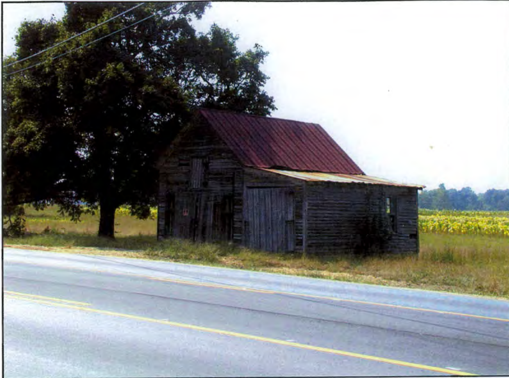
Smith Farm garage looking southwest.
