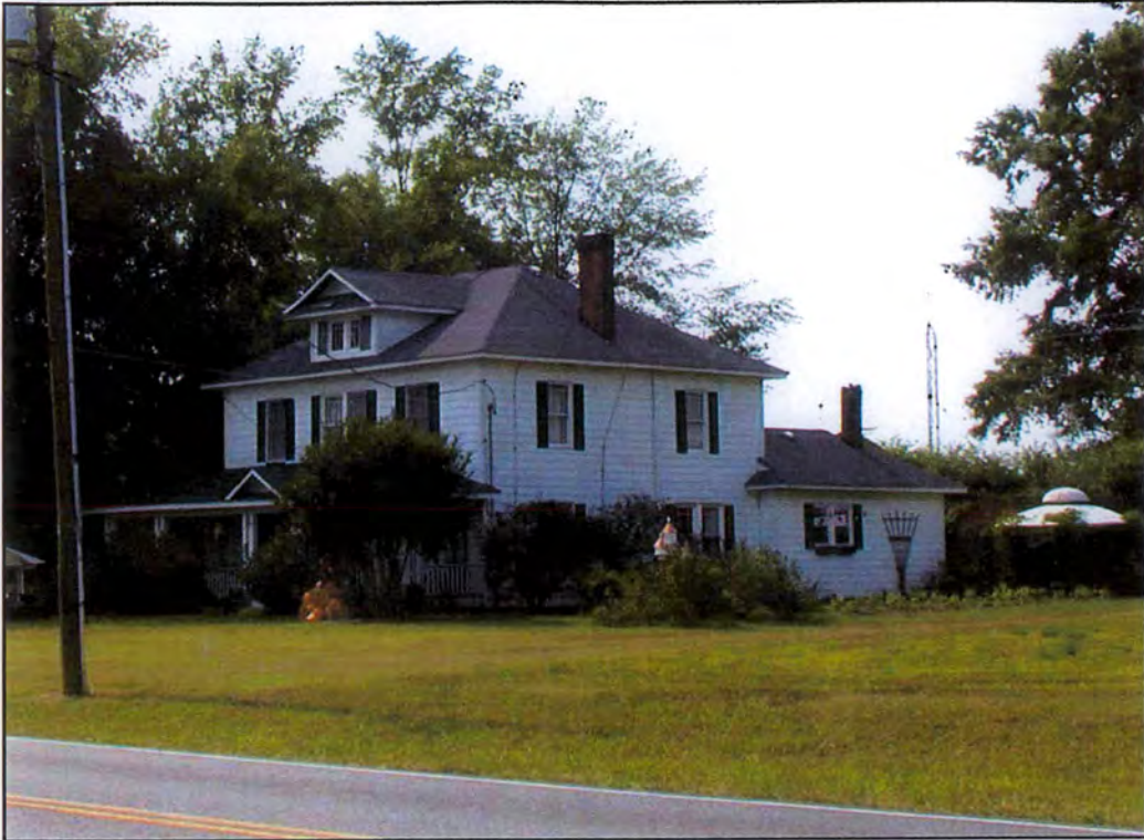
Motsinger House looking southwest.
