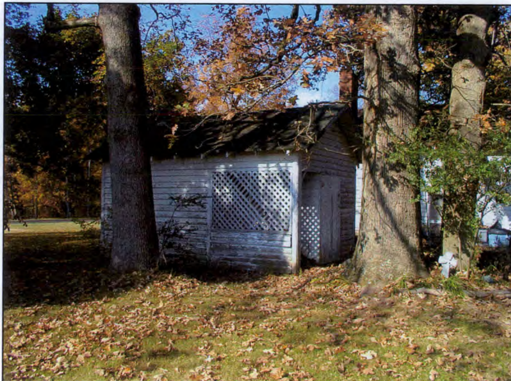
Daniel Smith well house looking north.
