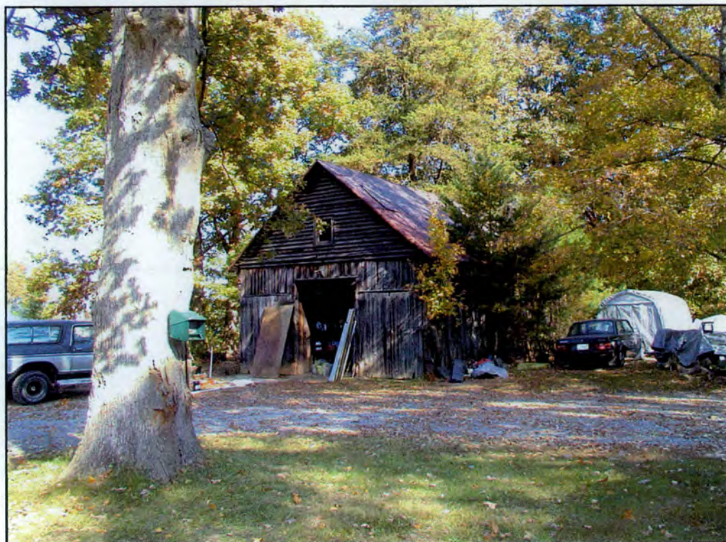
Daniel Smith barn looking northeast.
