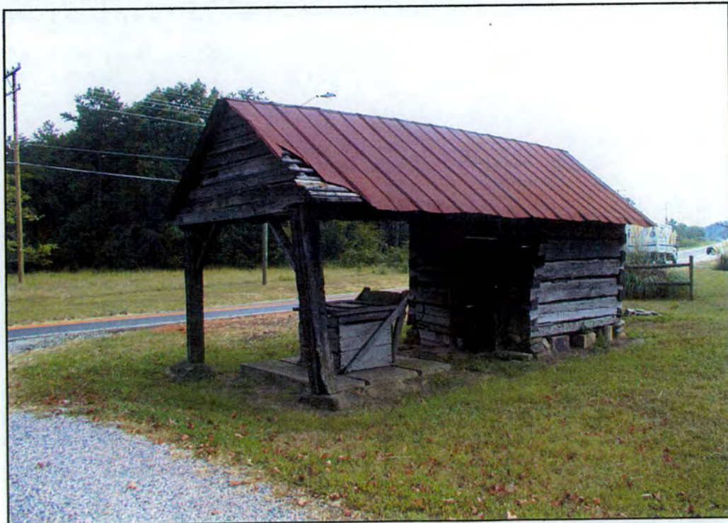
Well house looking southeast.
