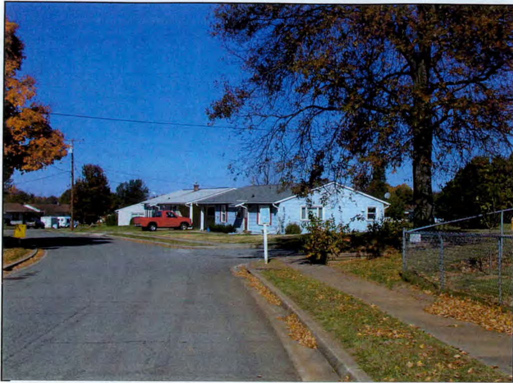
Housing development (B) looking northeast.
