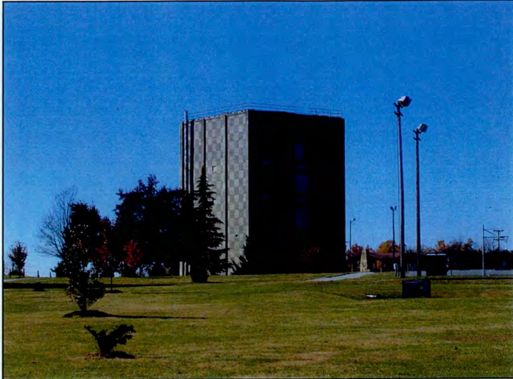
Radar tower (D1) looking south from Union Cross Park.
