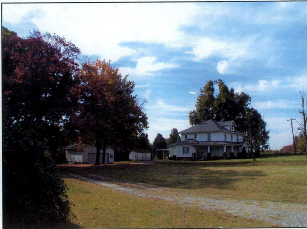
Weavil House (A), washhouse (B), and garage (E) looking southeast from Union Cross Road.
