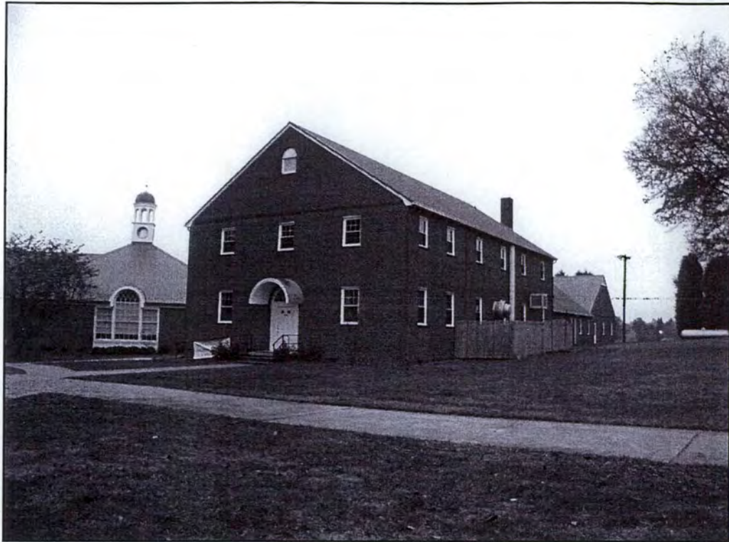
28. Sunday School Building, Union Cross Moravian Church, 4295 High Point Rd.
