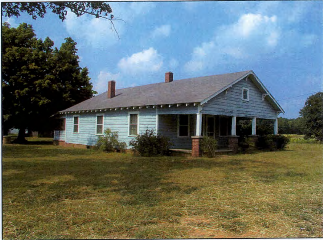
Smith tenant house (A) looking northwest.
