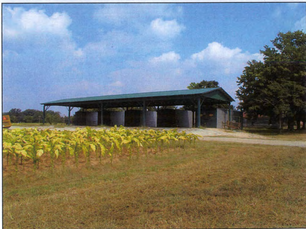
Tobacco bulk barn complex at rear of Smith tenant farm complex, looking northeast.
