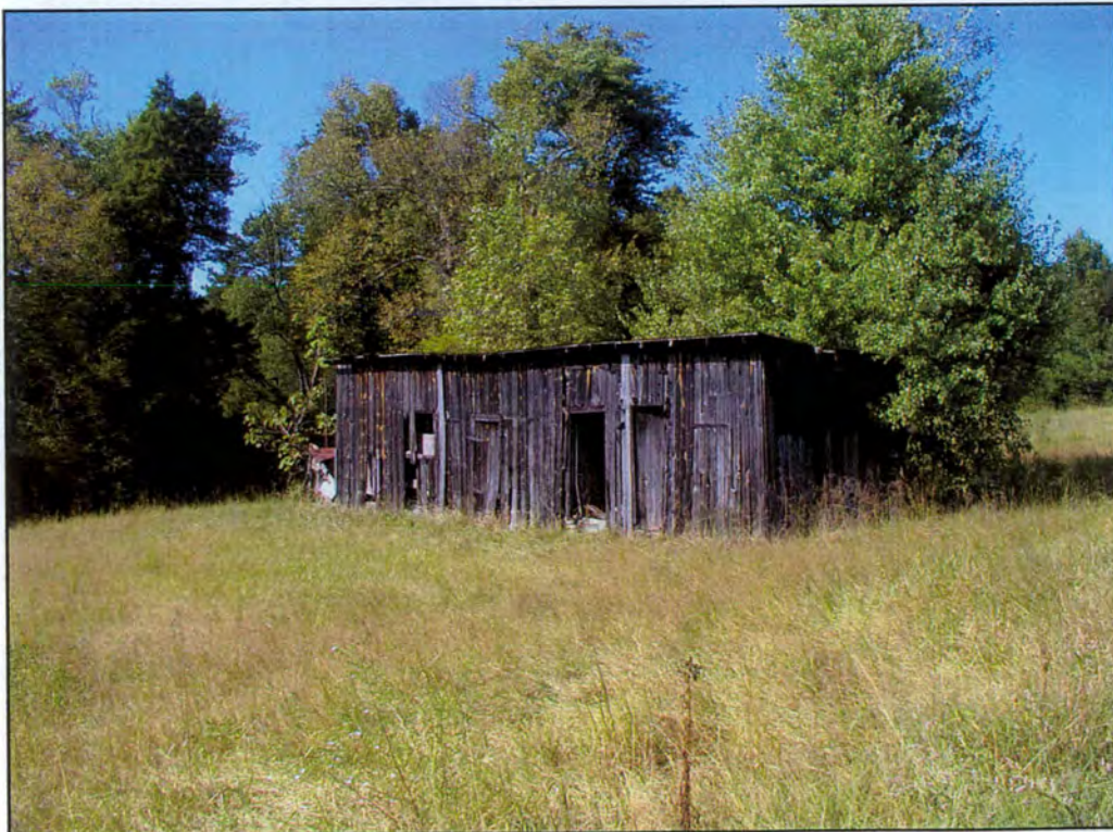
Smith Farm storage building looking northwest.
