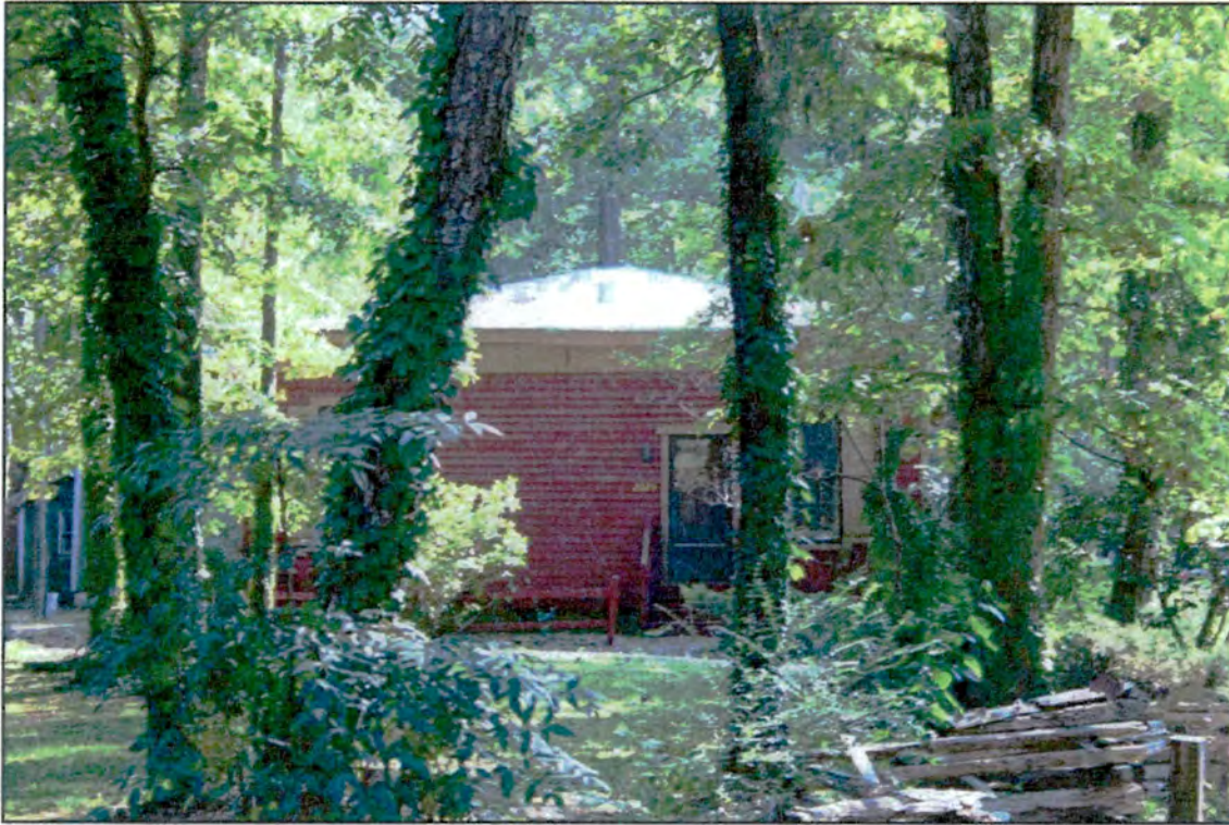
Property 5: House, 2025 NC 97. This appears to be a moved and altered building as well. Low brick foundation, and door cut in.
