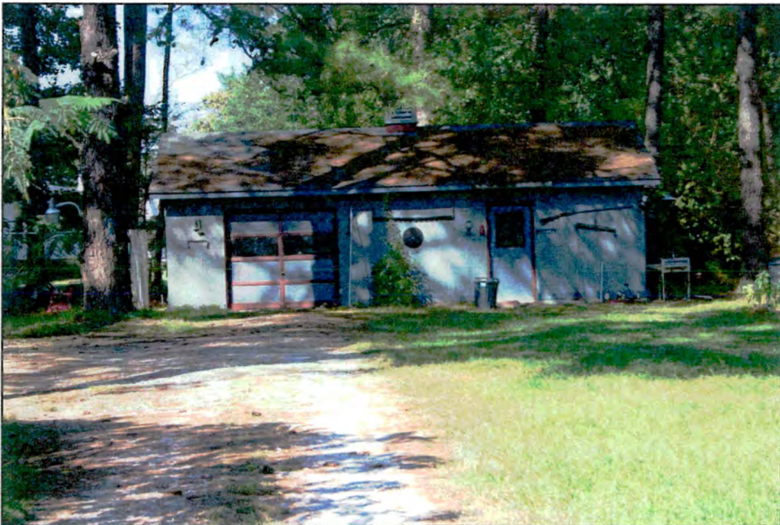
Property 7 : Garage, 11100 NC 97 (ca. 1960s as well)
