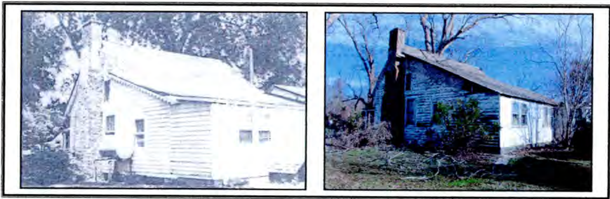
Figure 4: Photo from 1980 Hyde County Survey illustrating the original broken pitched roofline (left) with a photo from February 2006 showing the altered roofline for comparison.
