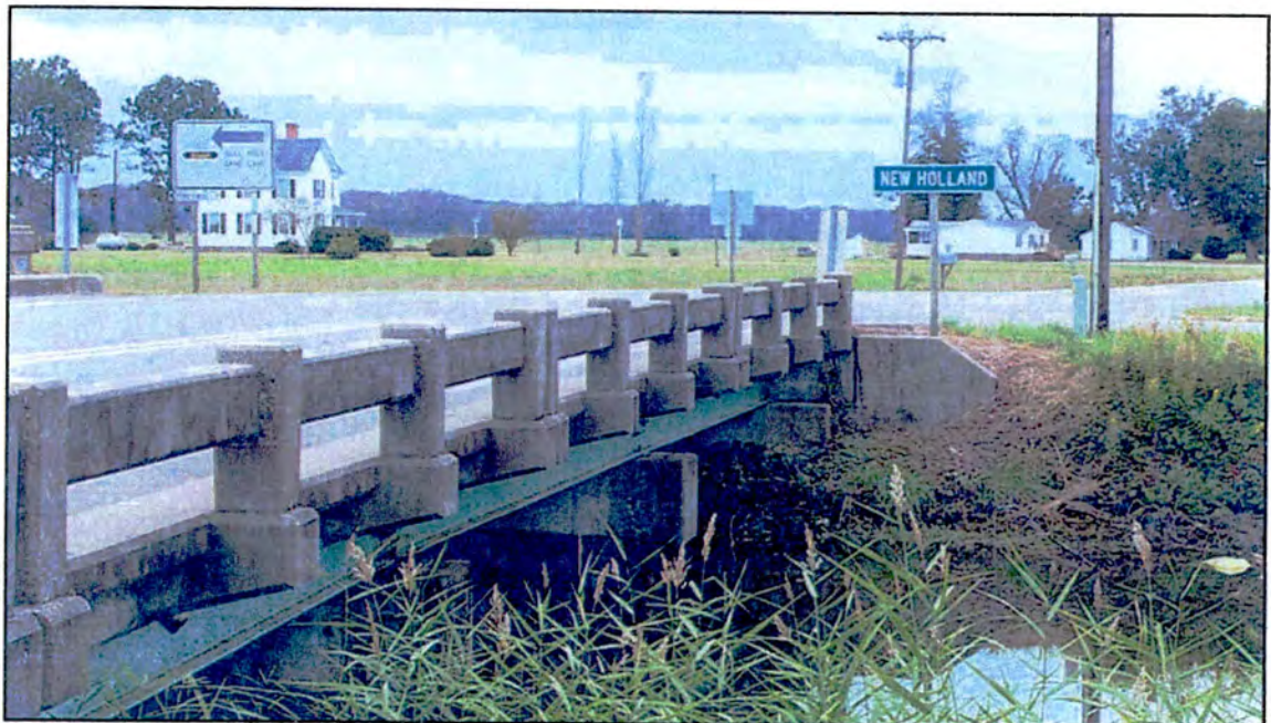
Photo 12: Looking west from Bridge No. 45. Alonza O'Neal House on left.
