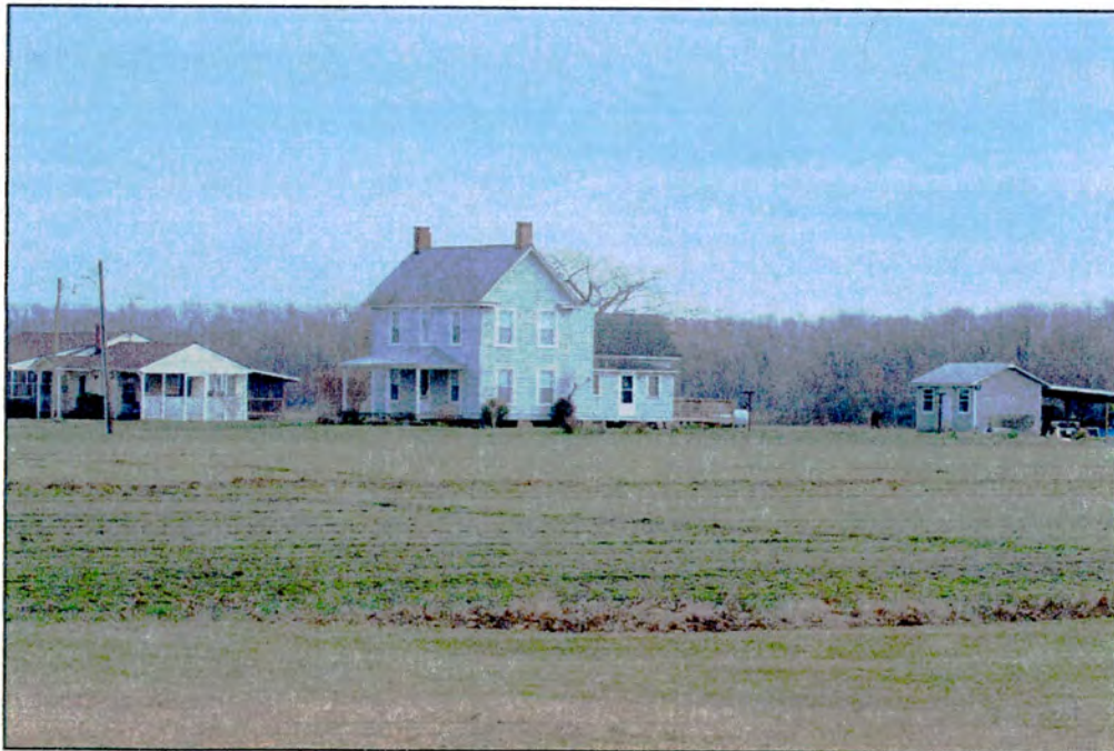
Photo 17: North front and east side elevations. Note close proximity of nonhistoric house on left.
