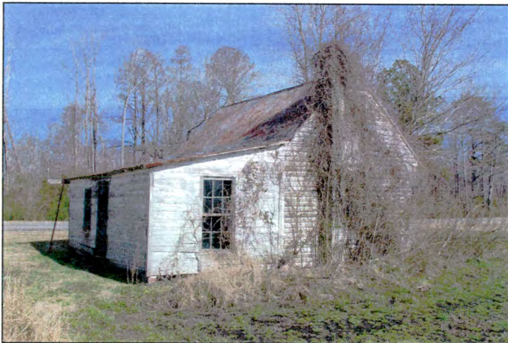
Photo 10: Weston Store - South rear elevation.
