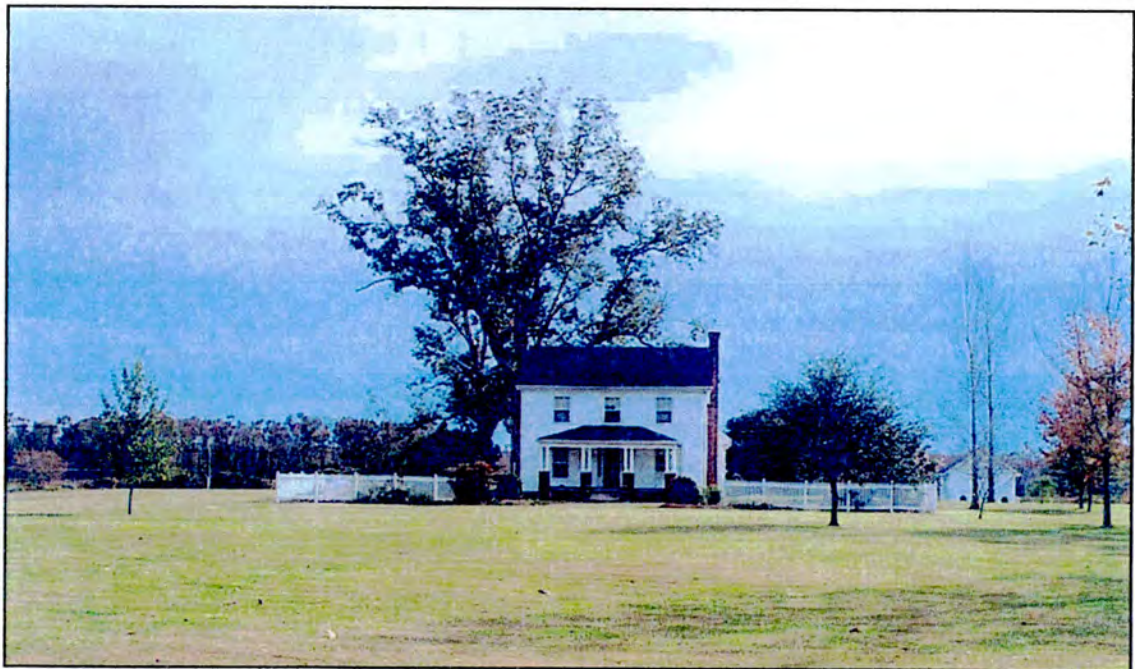
Photo 23: View of B. A. Credle House from US 264. Note black chain-link fencing enclosing tennis court on left.
