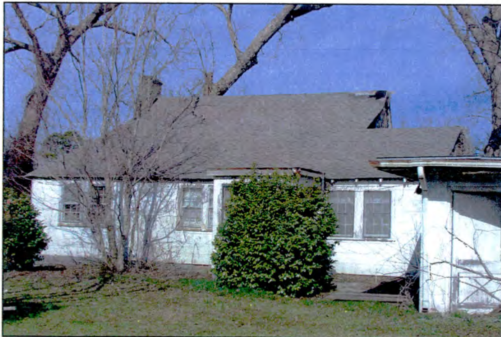
Photo 4: South rear elevation.
