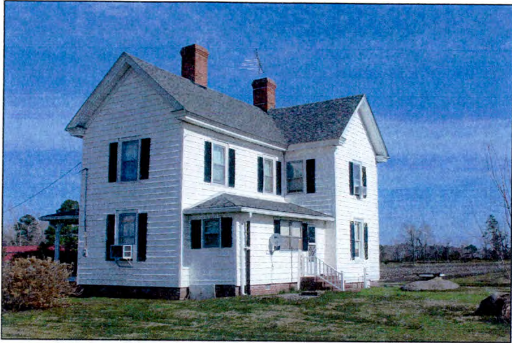
Photo 15: West side and south rear elevations showing enclosed rear porch.
