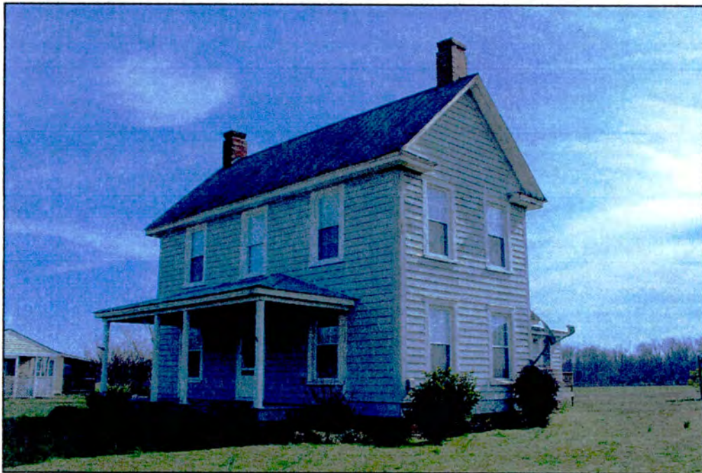
Photo 19: North front and east side elevations.
