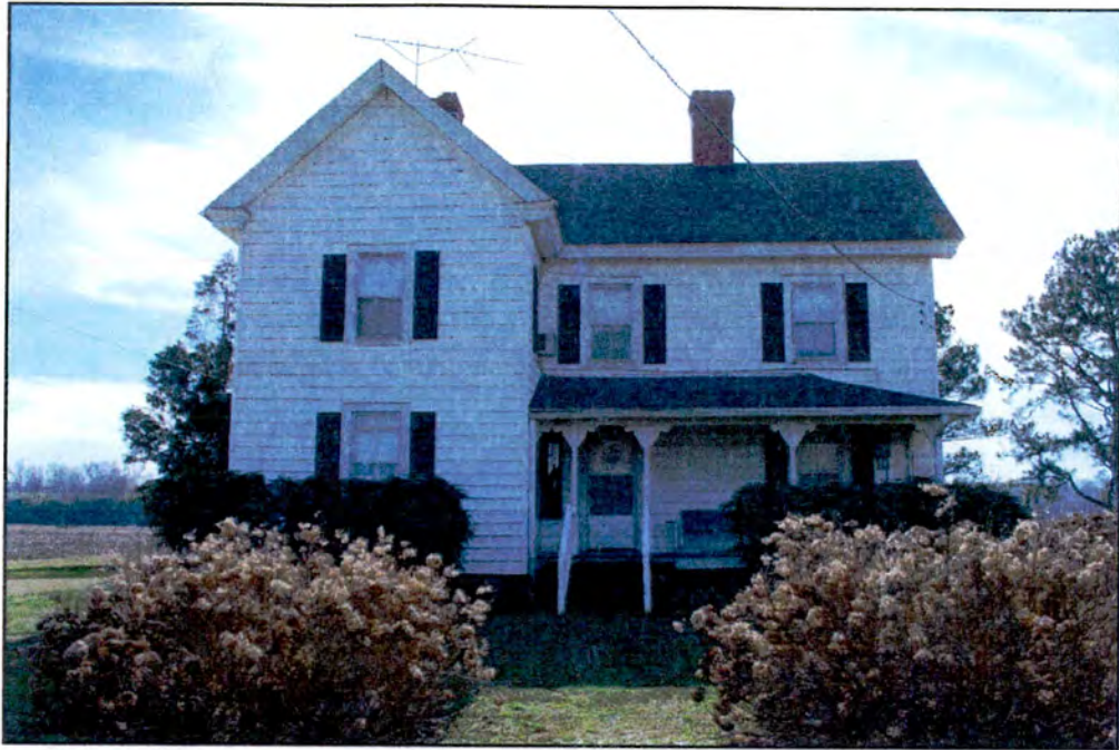
Photo 13: North facade. Note altered cornice returns.
