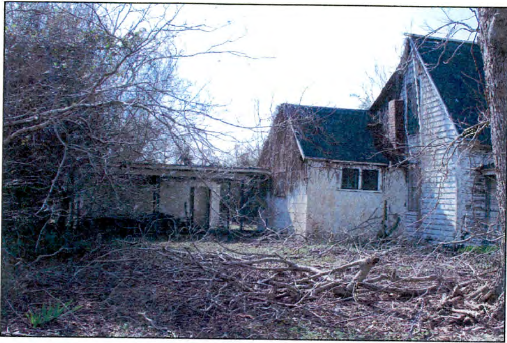
Photo 5: East side elevation and carport.
