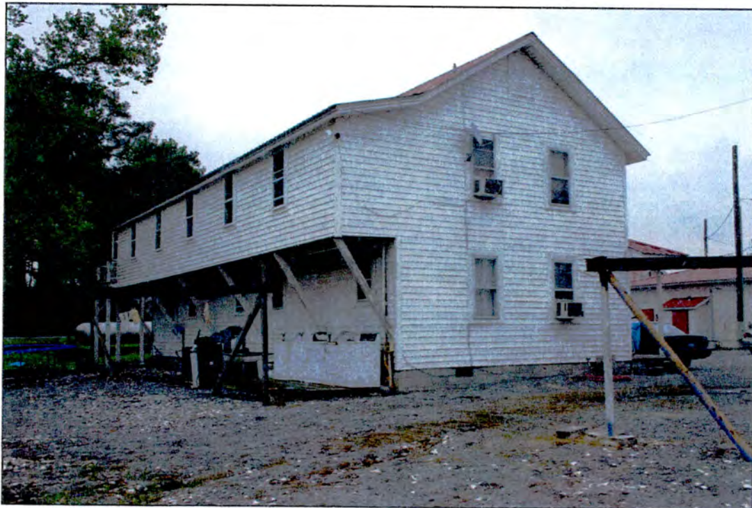
Property 5: west and north elevations
