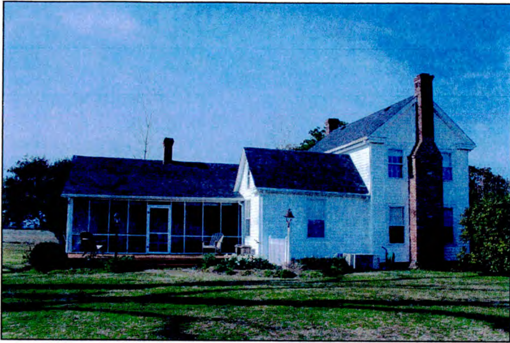
Photo 22: East side elevation.
