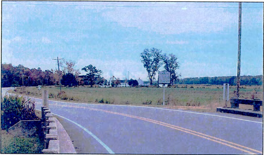
Photo 16: Looking east from Bridge No. 45 towards the Swindell House, on right in distance.
