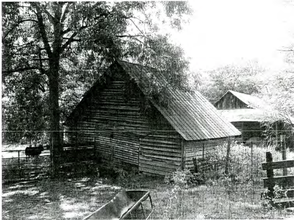
Property #21 - Granary (foreground) & Cow Barn (background)
