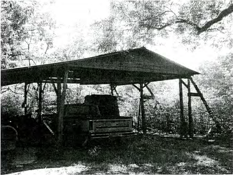
Property #21 - Truck Shed
