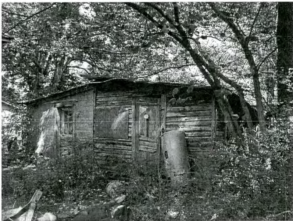
Property #21 - Wash House
