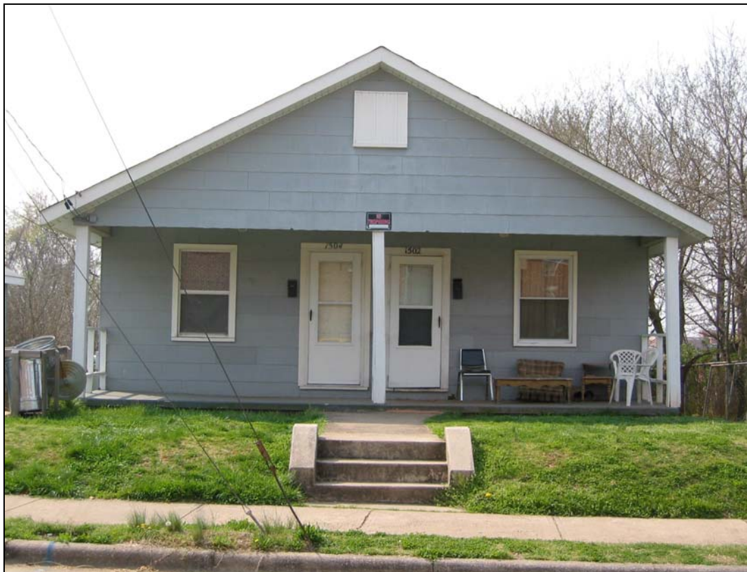
Figure 28: Duplex at 1502-1504 East First Street
