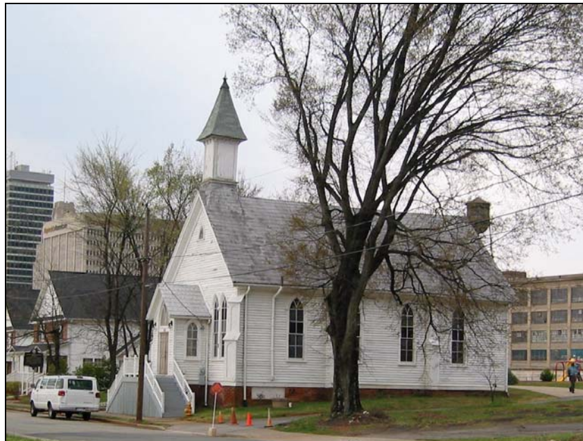
Figure 5: Lloyd Presbyterian Church, northeast corner
