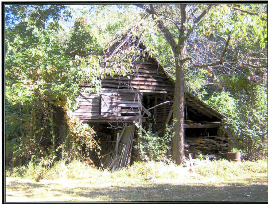
Figure 7 - Blake House, Barn (A)
