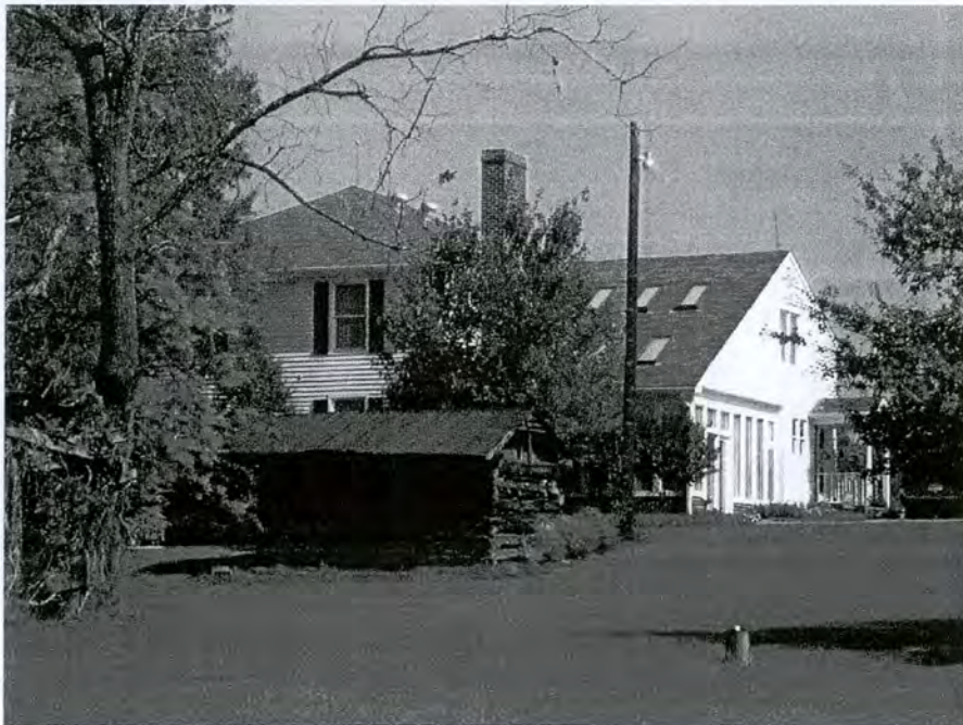
No. 57 Charles Daughtery House (side and rear elevations)
