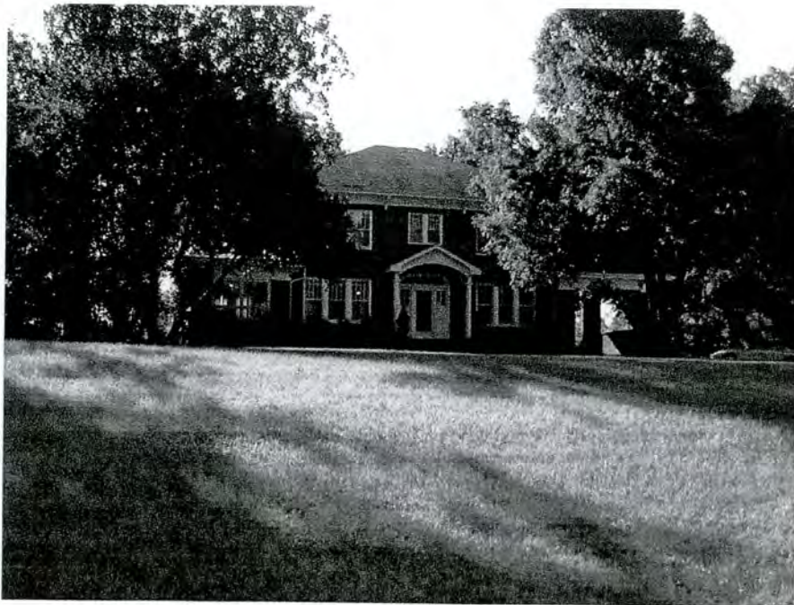
No. 71 House (front elevation)
