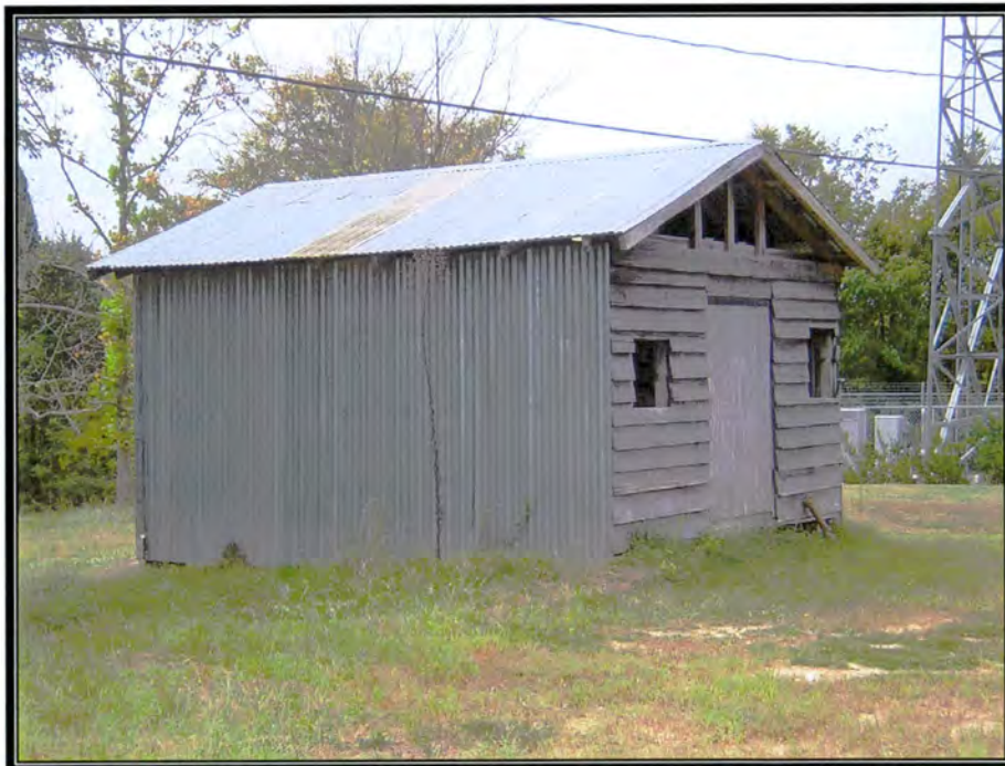
Figure 28 - Samuel Deal House, Outbuilding
