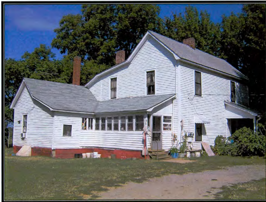
Figure 13 - Goodman Farmhouse, rear elevation
