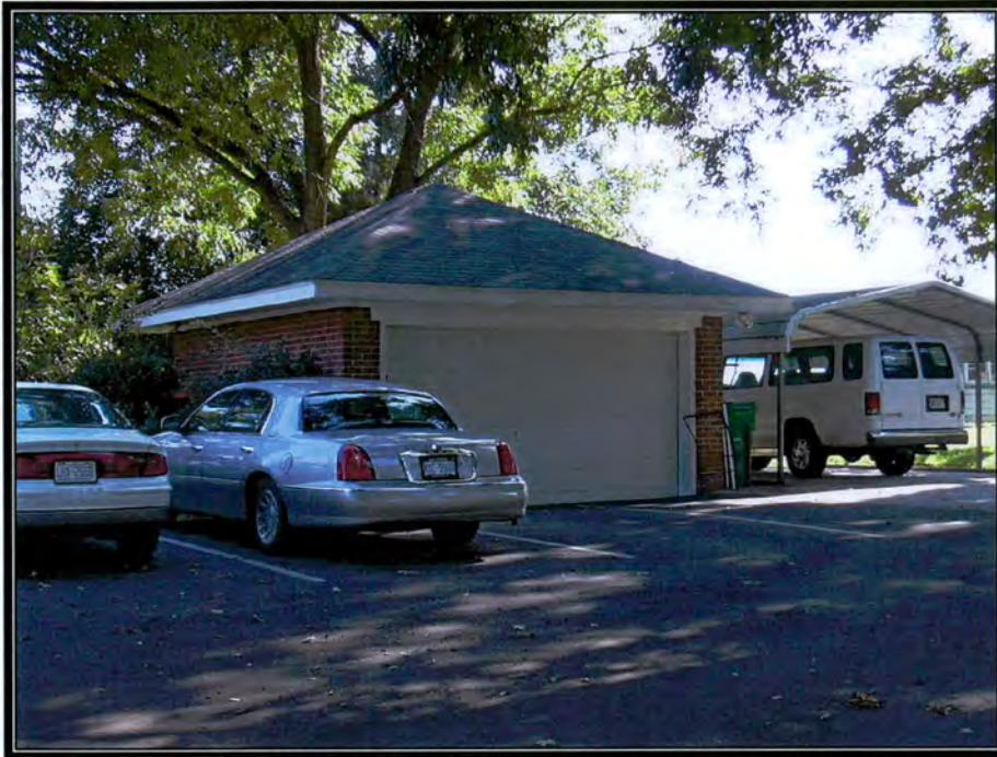
Figure 35 – Shinn House, Garage and Carport
