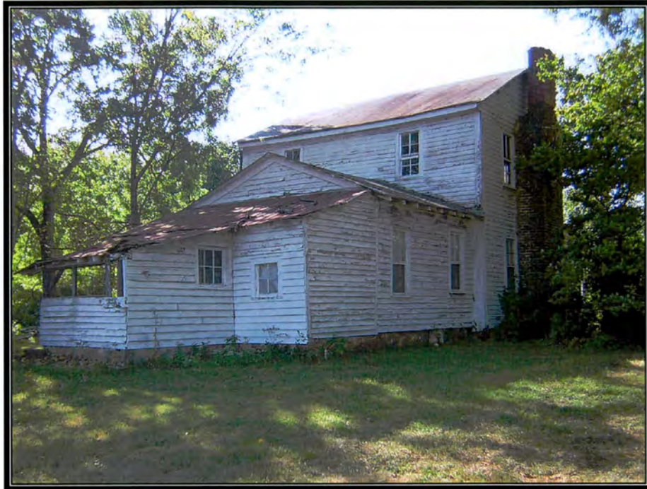
Figure 4 - Blake House, Rear Elevation
