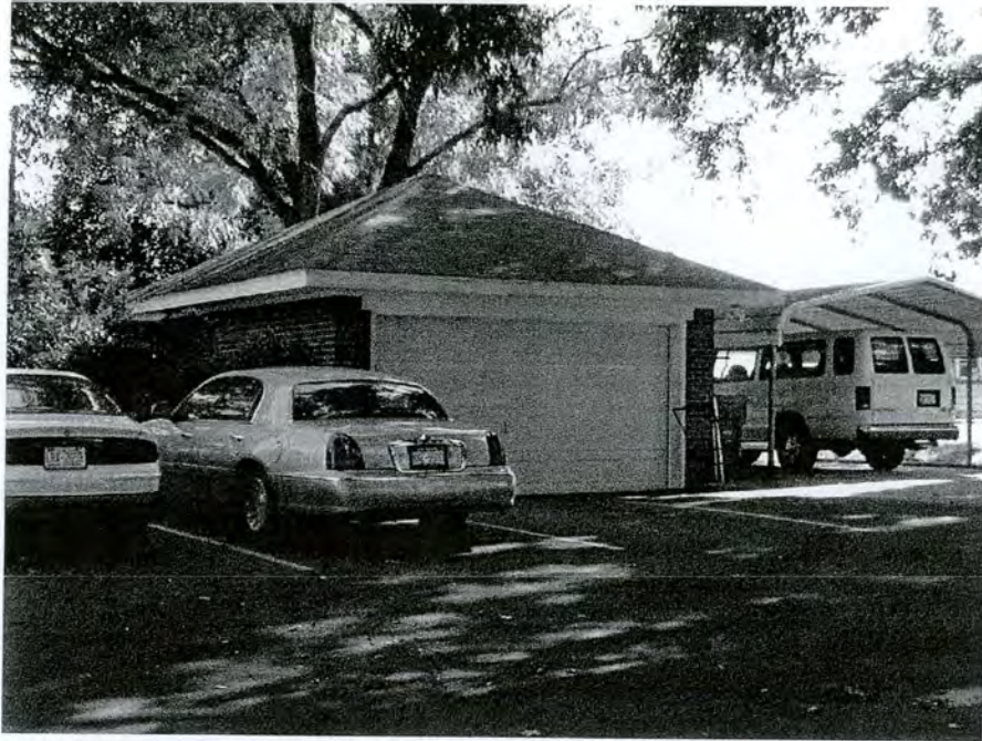
No. 71 House (garage)
