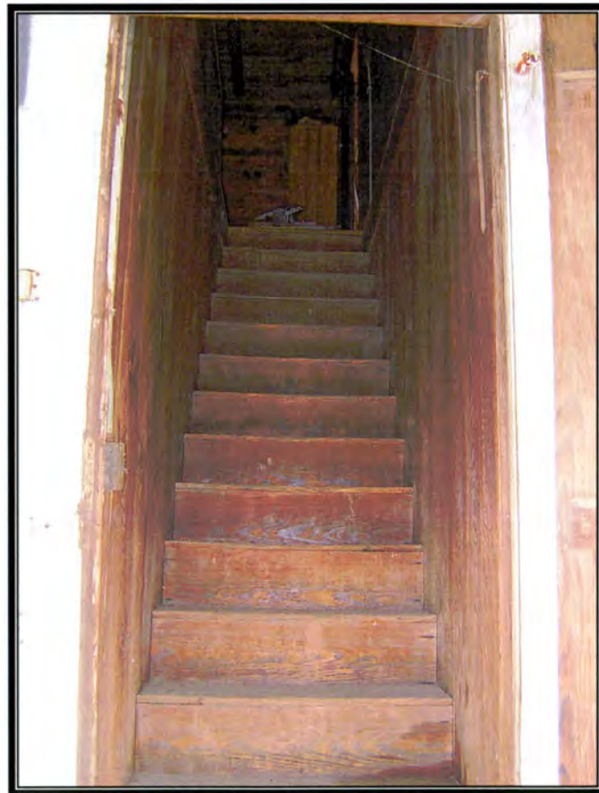
Figure 5 - Blake House, Enclosed Stair
