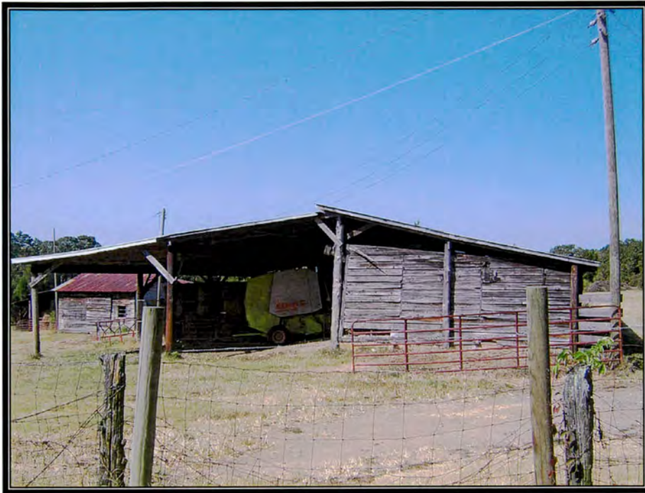
Figure 20 - Goodman Farm, Outbuilding (H)
