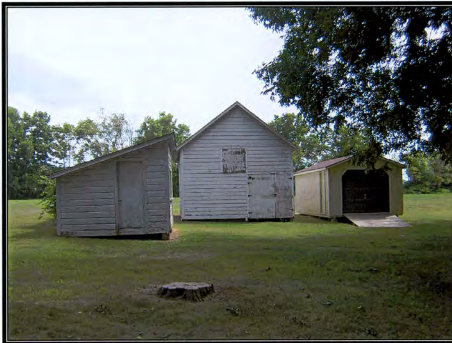
Figure 36 – Shinn House, Outbuildings
