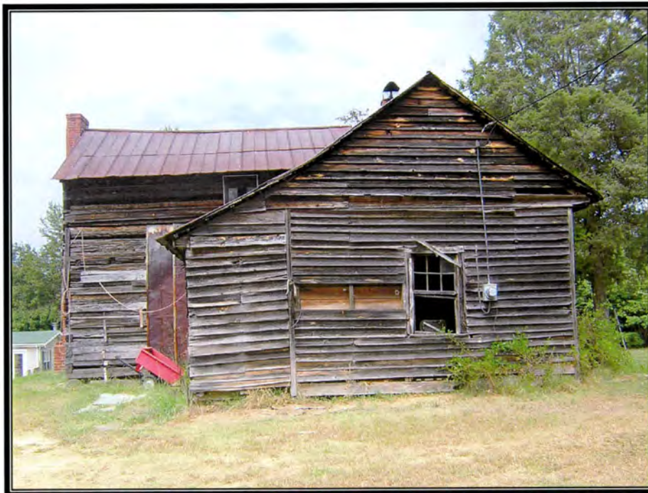
Figure 26 - Samuel Deal House, Rear Elevation
