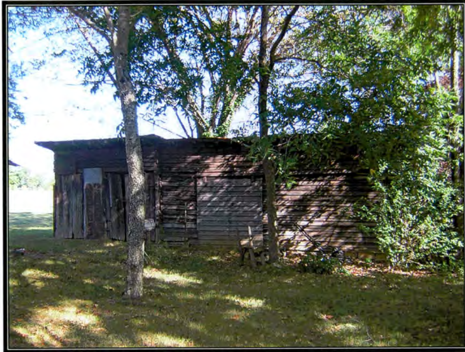
Figure 8 - Blake House, Shed (B)
