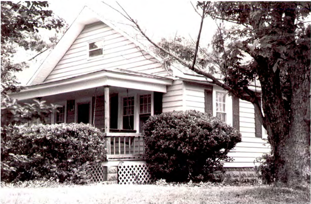
Plate 151: Neva Barnett and Thomas J. Evans House (#5) in Buxton, south front and east side elevations
