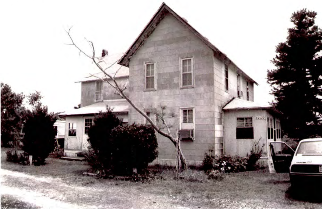
Plate 69: Banister B. and Blanch Gray Gray House (#22) in Avon, west side and south front elevations
