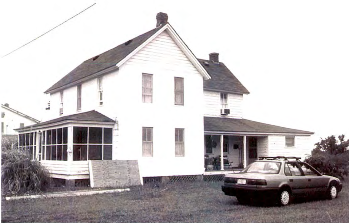
Plate 52: E. Blucher and Beulah Gray Scarborough House (#5) in Avon, east side and south front elevations
