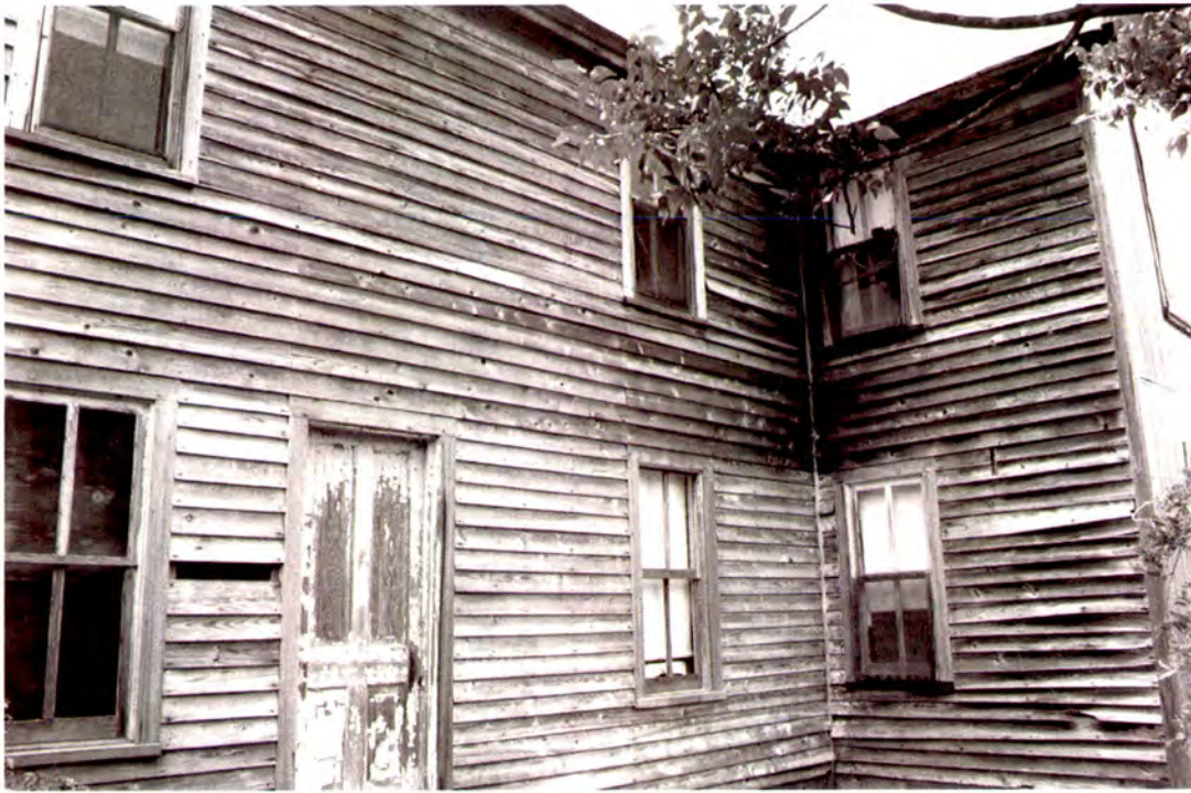
Plate 131: Emma Farrow Morgan Gray House (#24) – south rear elevation of main block and east side elevation of ell; modern siding visible at far right
