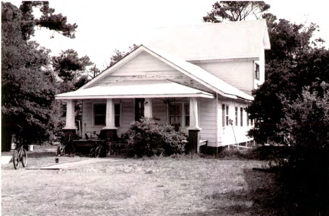
Plate 203: Whidbee-Williams House (#41) in Buxton, north front and west side elevations
