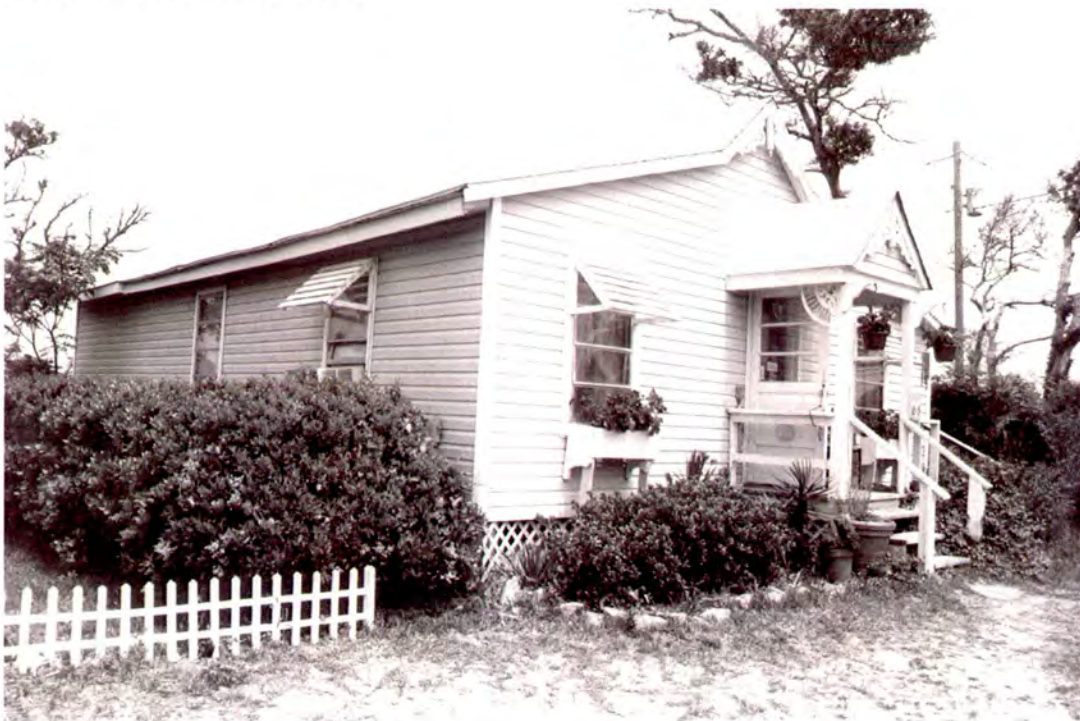
Plate 171: S. Burden and Charlotte Austin Smith House (#20) in Buxton, south side and west front elevations of former kitchen building
