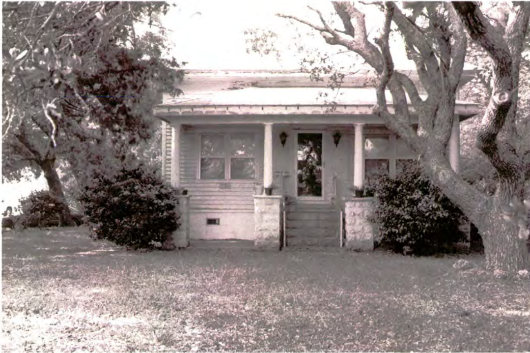
Plate 212: Lafayette D. and Pearl Bragg Midgette House (#49) in Buxton, south front elevation in 2001 prior to modernization
