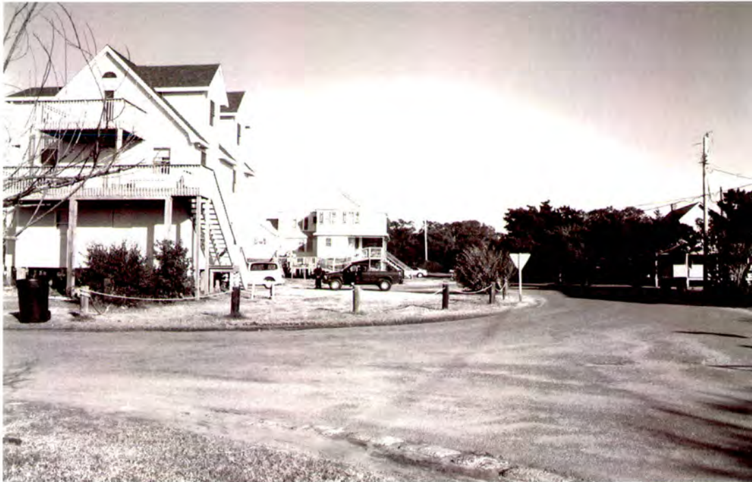
Plate 122: Avon looking northeast up McMullen Road from intersection with Harbor Road; Hooper House (#45) at center left
