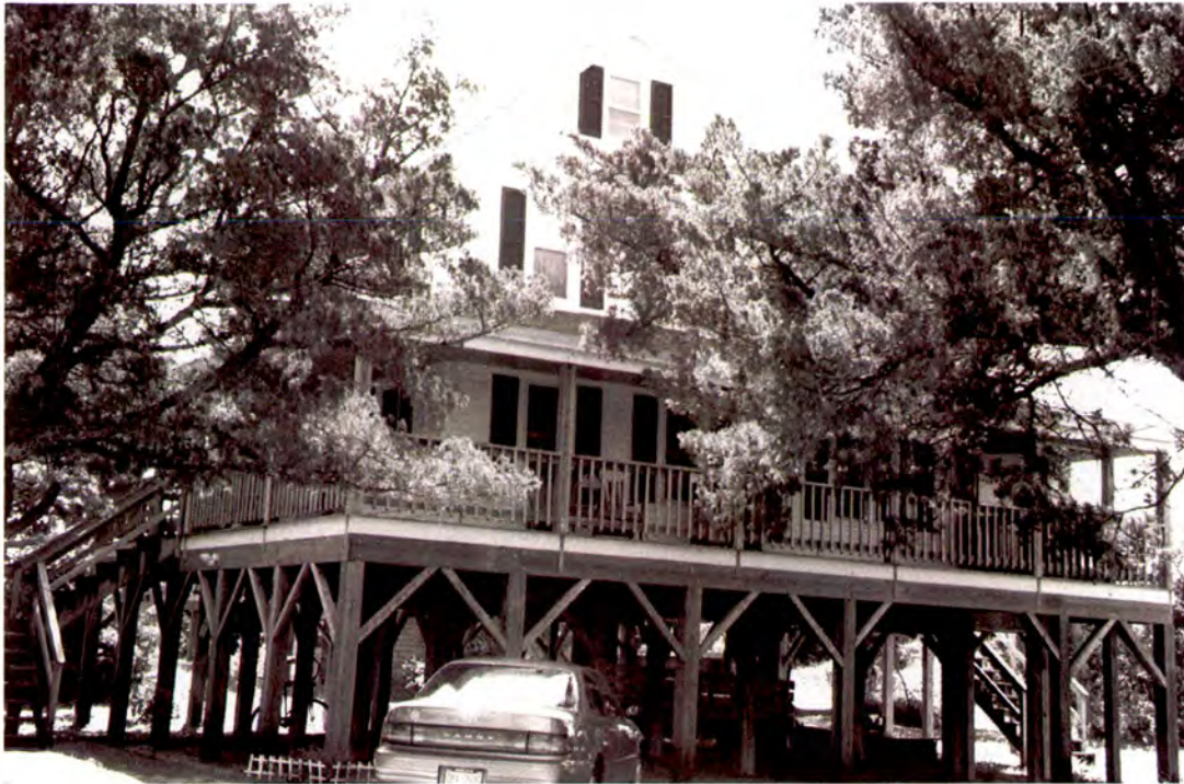
Plate 104: Fred G. and Selina Williams Gray House (#57) in Avon, east side elevation
