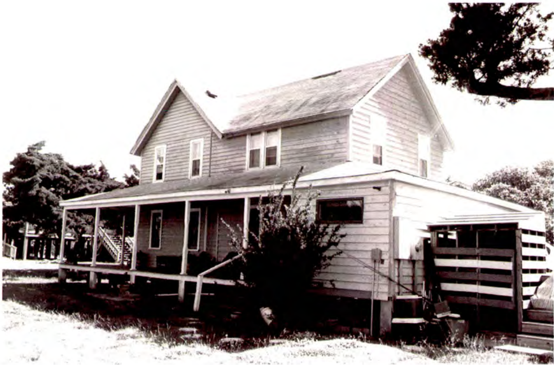
Plate 98: Homer S. Gray House (#51) in Avon, west side and north rear elevations
