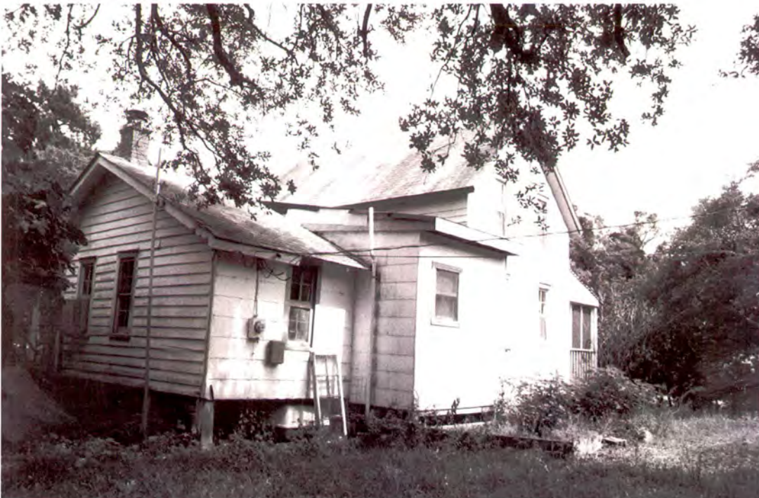
Plate 191: John A. and Brittonia Williams Gray House (#33) in Buxton, west side and north rear elevations
