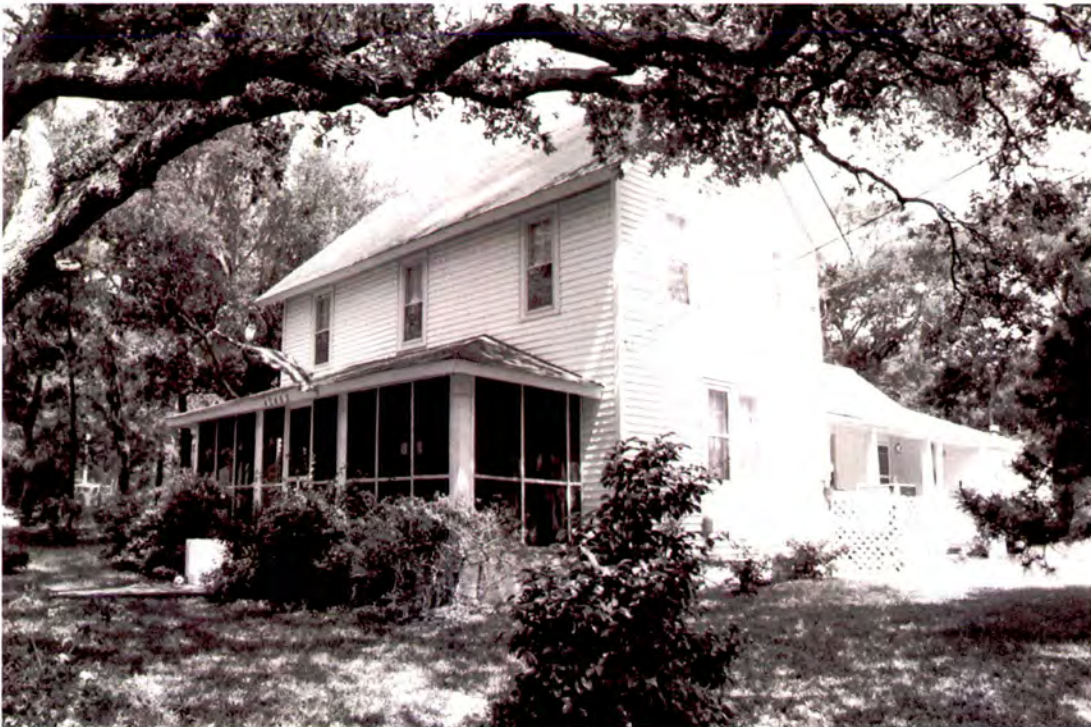
Plate 153: W. Rocky and Cynthia Tolson Rollinson House (#7) in Buxton, south front and east side elevations
