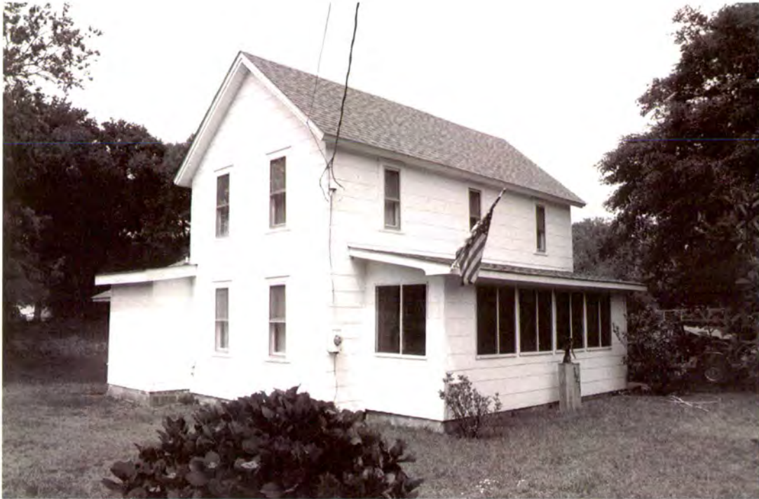
Plate 184: Gray-Midgett-Gaskins House (#29) in Buxton, south front and west side elevations
