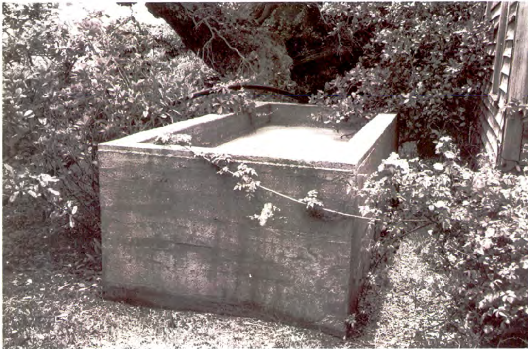
Plate 133: Emma Farrow Morgan Gray House (#24) – cistern to south rear of ell
