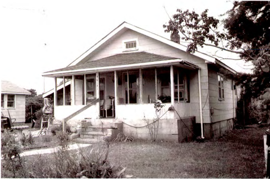
Plate 54: Edna Midgett and Walker B. Scarborough, Sr. House (#7) in Avon, south front and east side elevations
