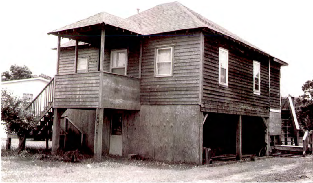
Plate 64: Franklin P. and Susan Austin Williams House (#17) in Avon, north front and west side elevations
