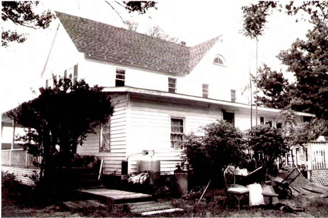
Plate 206: Williams-Gaskins House (#43) in Buxton, south rear and west side elevations
