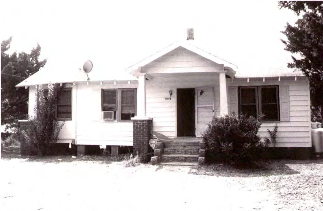
Plate 89: Dallas B. and Lucy Farrow Miller House (#42) in Avon, east front elevation
