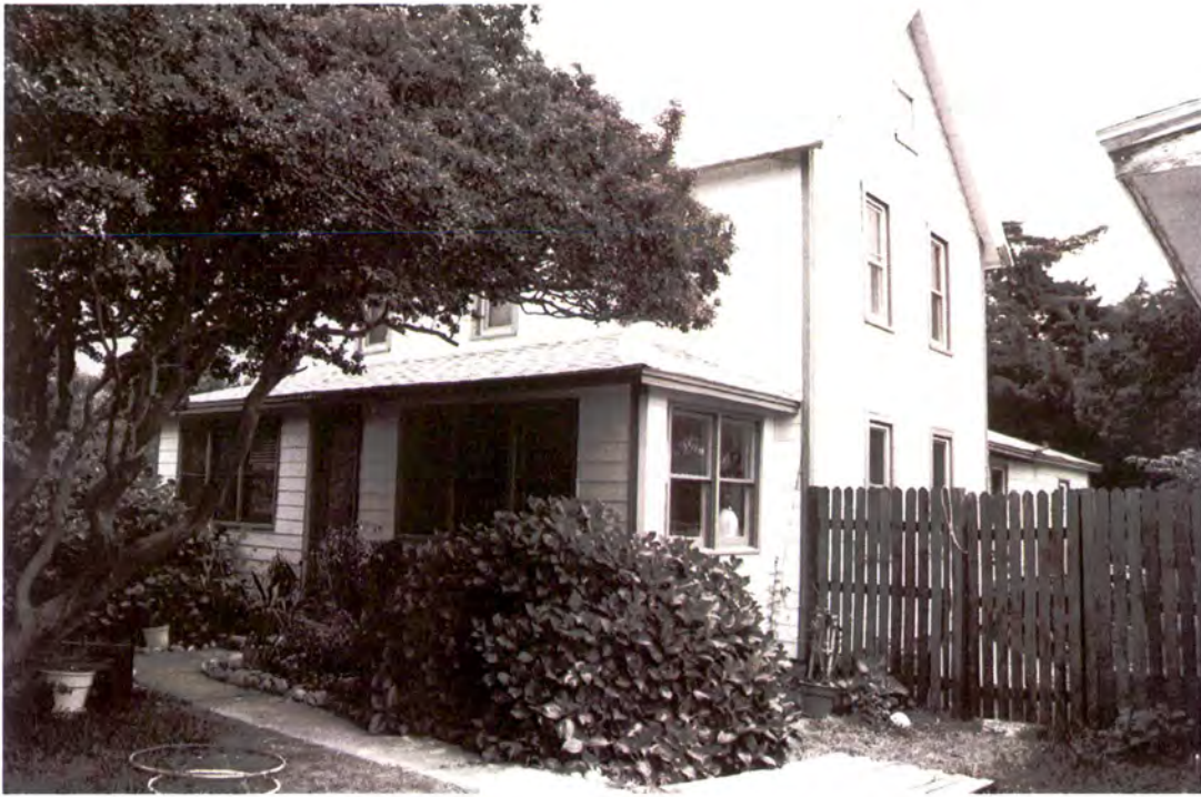
Plate 178: Utah C. and Mary Clark Jennett House (#25) in Buxton, north front and west side elevations
