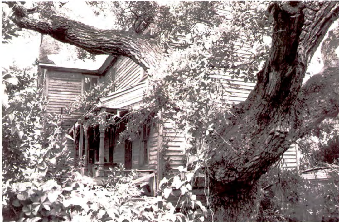
Plate 134: Emma Farrow Morgan Gray House (#24) – north rear and west side elevations of ell; cistern in shadow of massive oak at lower right
