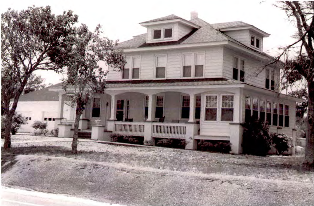
Plate 167: Bernice R. and Buena Midgett Ballance House (#19) in Buxton, north front and west side elevations; modern garage at left
