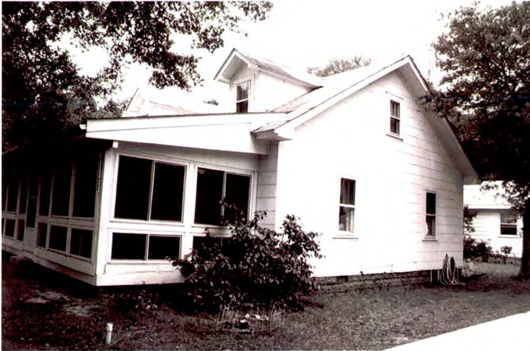
Plate 156: Zeb F. Miller House and Miller Cemetery [I]/ (#9) in Buxton, south front and east side elevations of house
