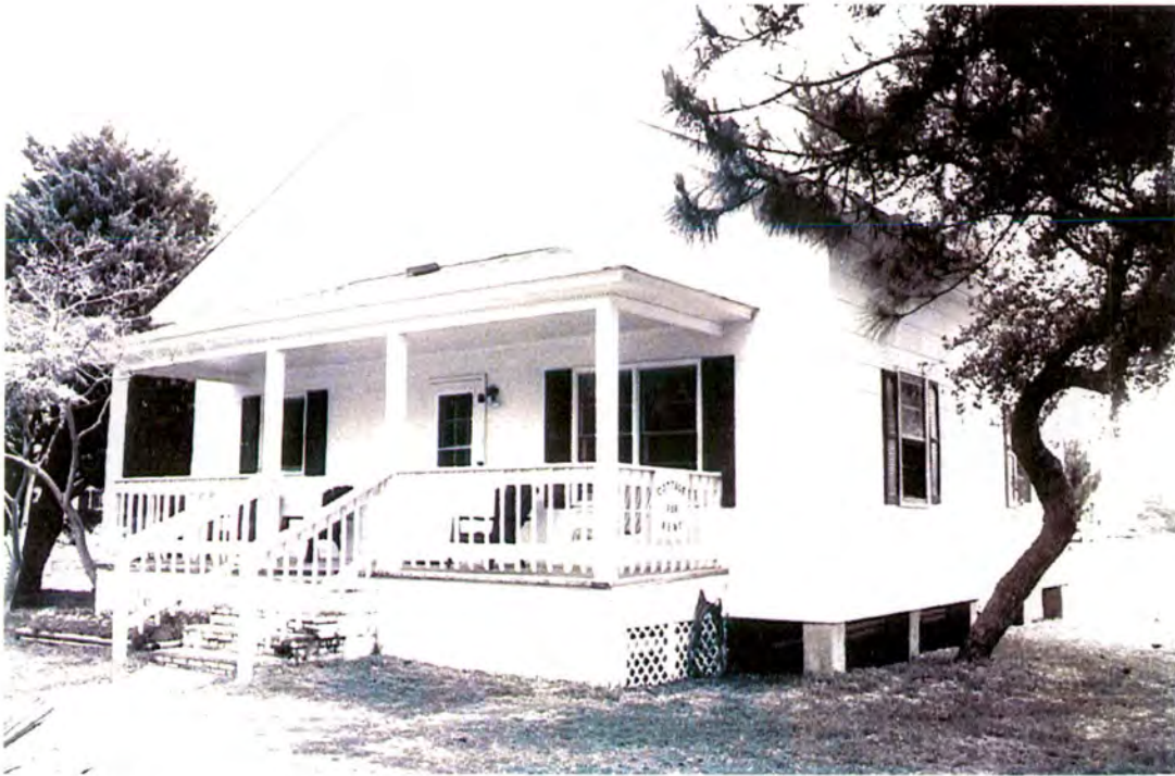
Plate 48: Dammon E. and Alice Meekins House (#1) in Avon, west front and south side elevations
