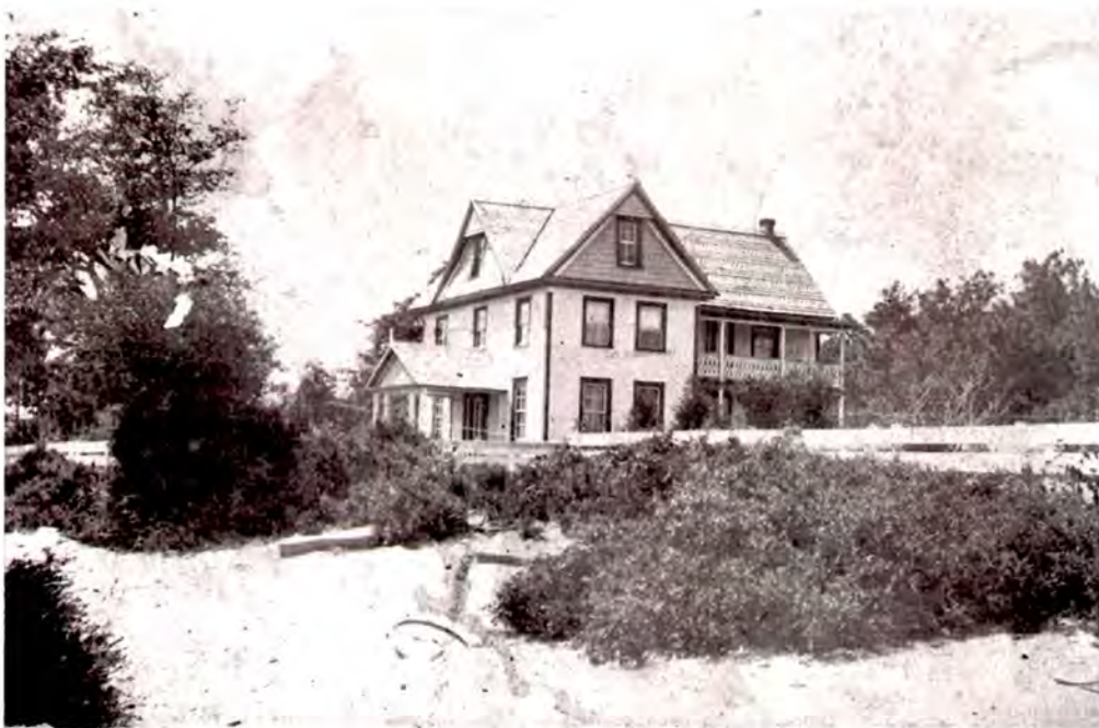
Plate 30: Baxter B. and Josephine Gray Miller House (1890s) (#12), at opening of twentieth century, with fine porches in place (Courtesy of the North Carolina State Archives)
