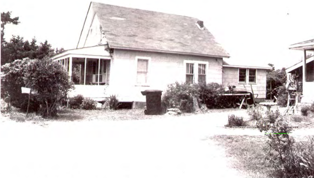
Plate 55: Elsie Scarborough and James Sawyer House (#8) in Avon, east side and south front elevations
