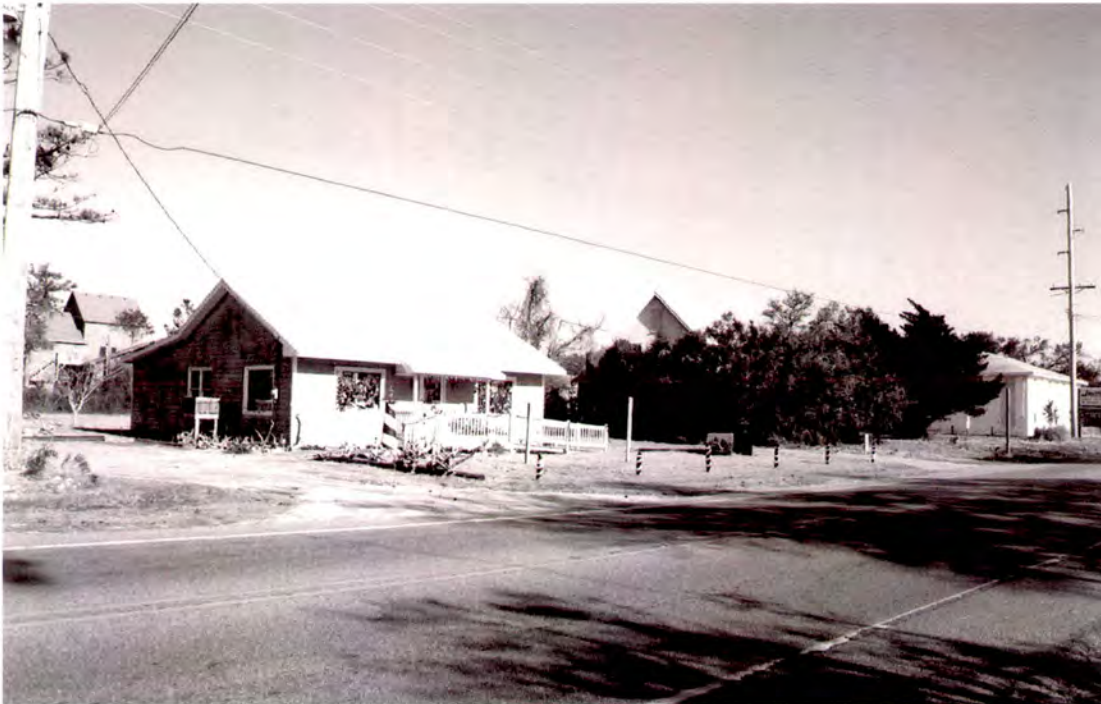
Plate 225: Buxton looking northeast along NC 12; roof of Farrow House (#36) at right center
