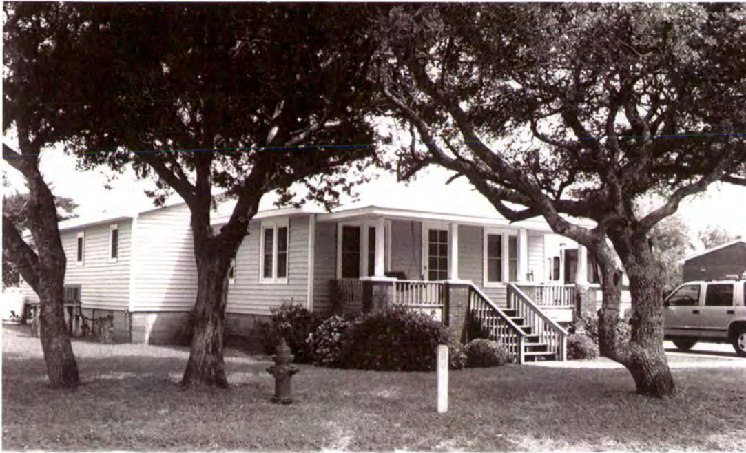
Plate 82: Carrie G. O'Neal House (#35) in Avon, west front and north side elevations
