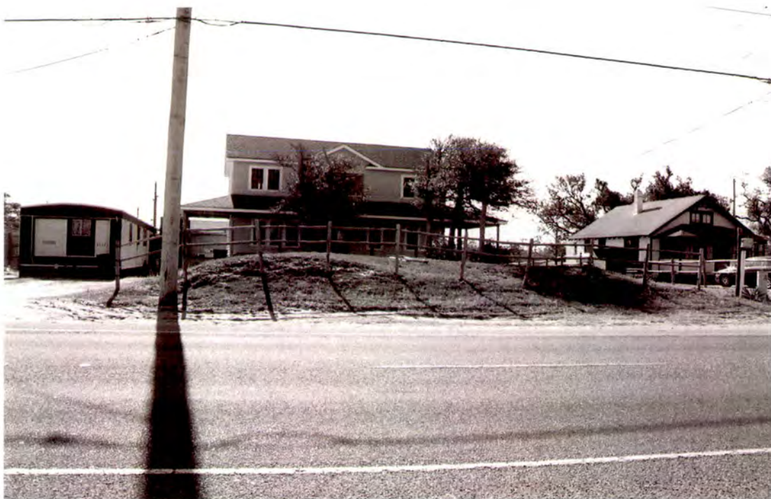
Plate 232: Buxton looking south across NC 12; Farrow House (#47) at right
