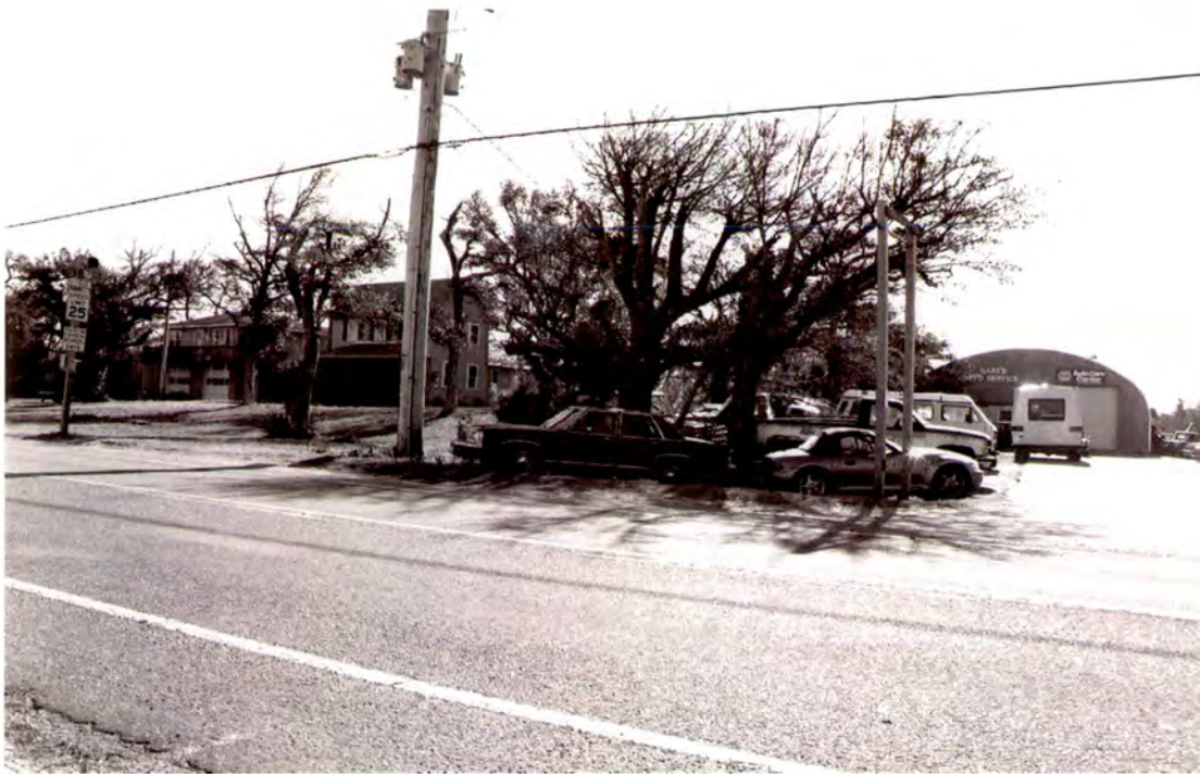
Plate 230: Buxton looking southeast along NC 12; Simpson-Barnett House (#45) at left center
