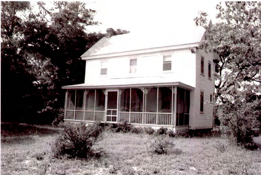
Plate 201: Jennette-Brady House (#40) in Buxton, south front and east side elevations
