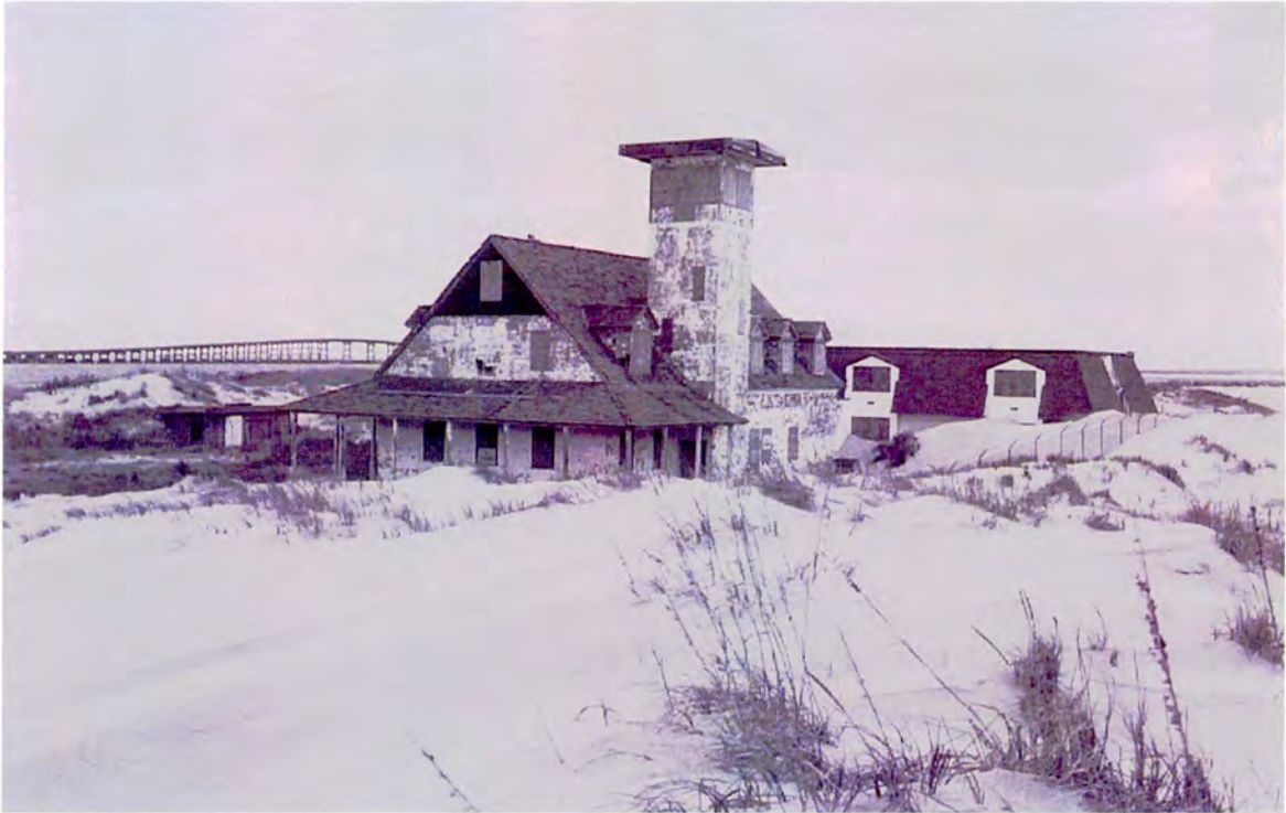
Plate 41: Oregon Inlet Station – west side and south rear elevations; 1970 addition at right and Bonner Bridge at left
