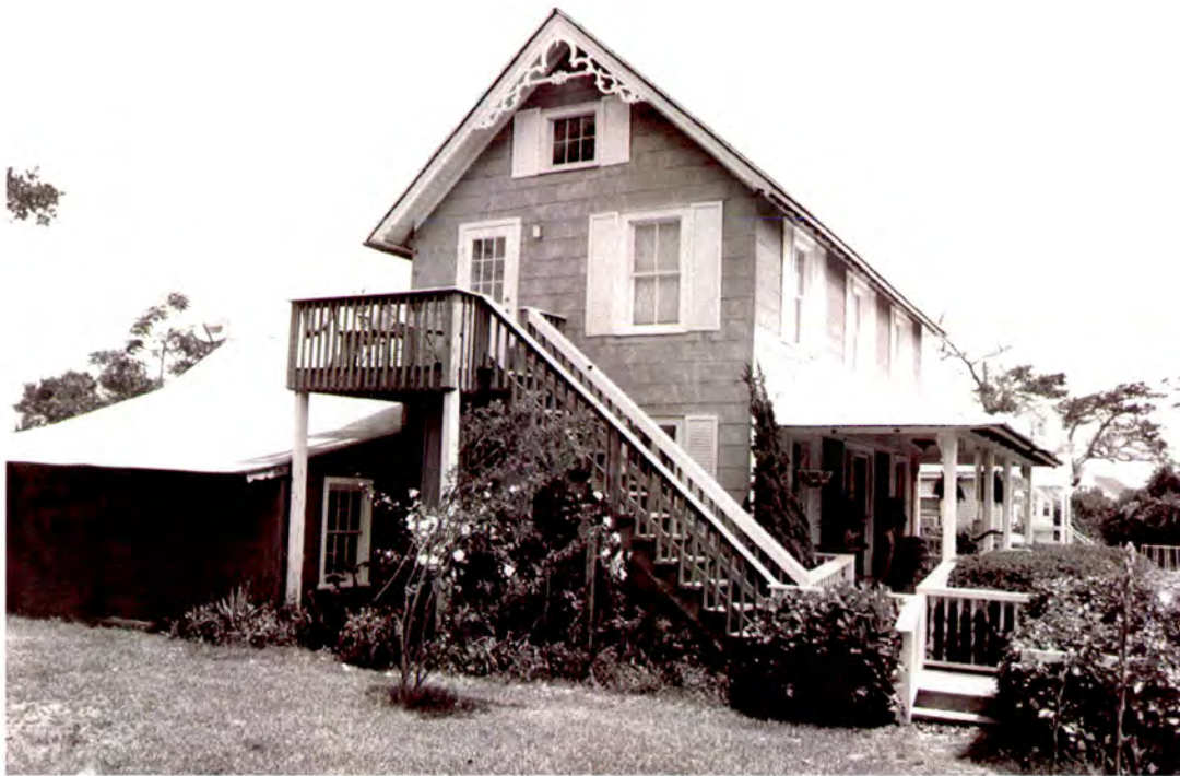
Plate 170: S. Burden and Charlotte Austin Smith House (#20) in Buxton, west side and south front elevations of house
