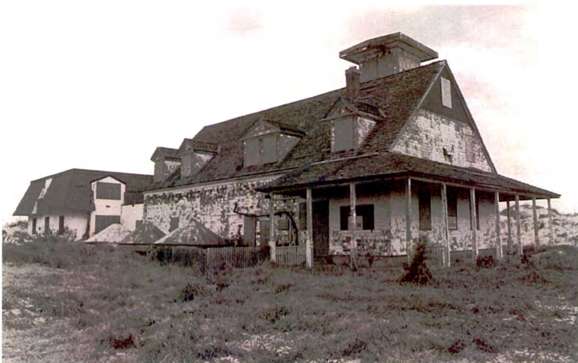
Plate 43: Oregon Inlet Station – north front and west side elevations; 1970 addition at left
