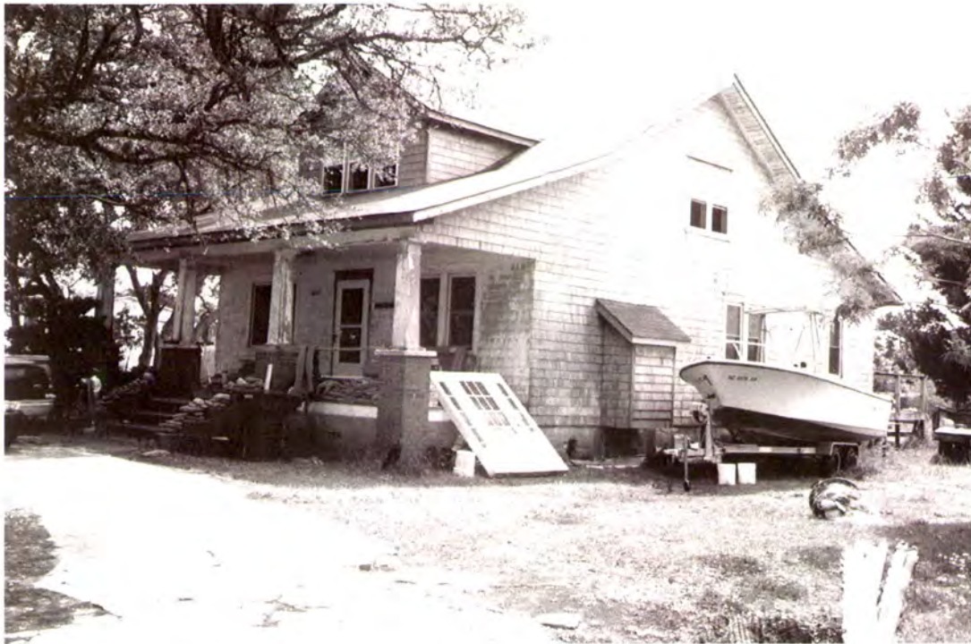
Plate 86: Alton Williams House (#39) in Avon, east front and north side elevations
