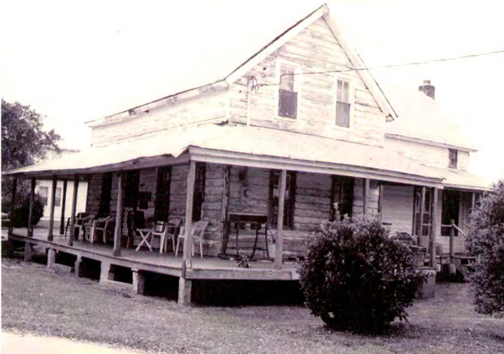
Plate 136: Henrietta Scarborough and Issac T. Meekins House (#32) – southeast front and northeast side elevations
