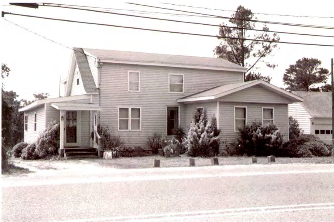
Plate 164: Former Charles P. Gray Store (#16) in Buxton, north front and east side elevations
