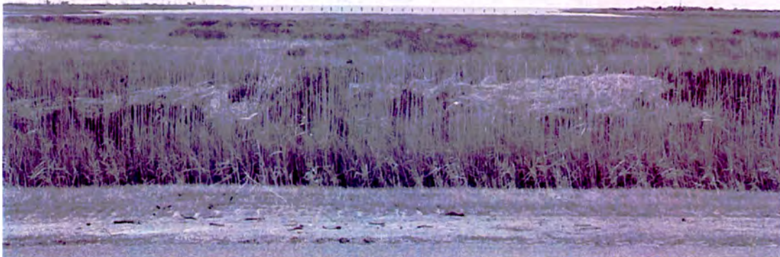
Plate 45: New Inlet Bridges - remnants of columns of southern bridge, looking west toward Pamlico Sound
