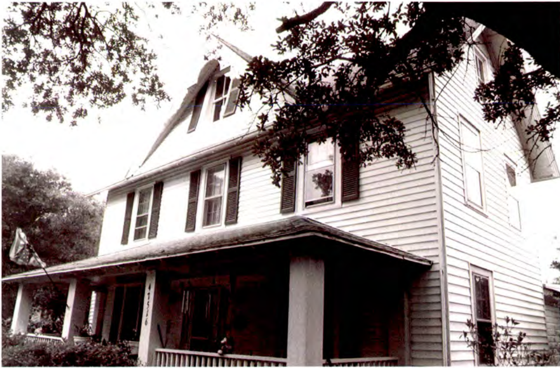
Plate 154: Urias O. and Caddie Midgett Gaskins House and Gaskins Cemetery (#8) in Buxton, south front and east side elevations of house
