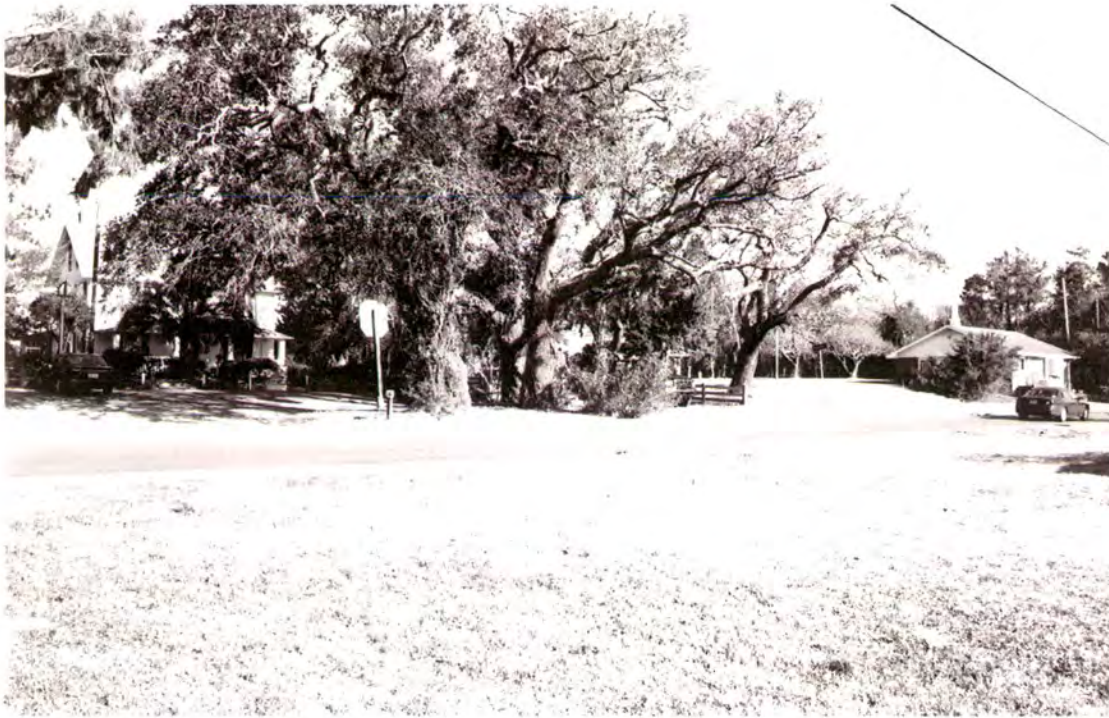
Plate 220: Buxton looking northeast toward Rocky Rollinson Road from junction with NC 12; Gaskins House (#8) at left
