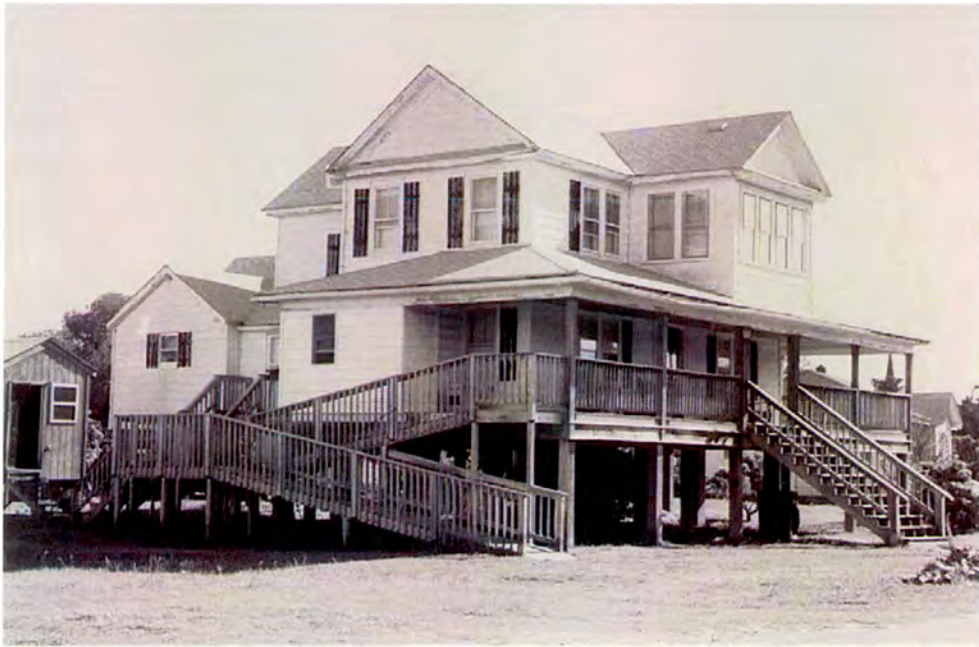
Plate 39: Avon's Hooper Family House (#45) raised on pilings within clear expanse of lawn
