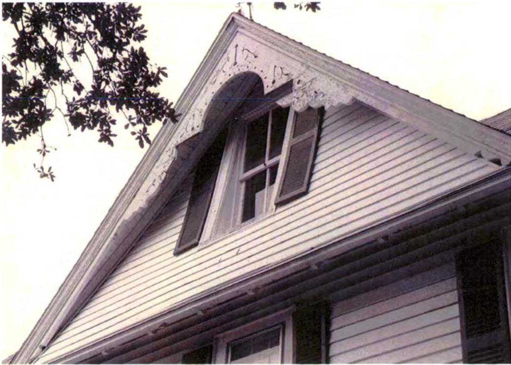
Plate 244: Urias O. and Caddie Midgett Gaskins House and Gaskins Cemetery (#8) – façade gable at south front elevation of house
