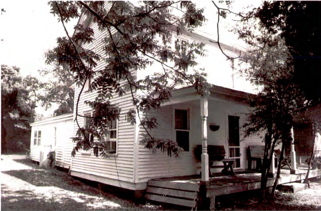
Plate 144: Thomas and Joseph Ann Gray Gray House (#41) – north side and west front elevations
