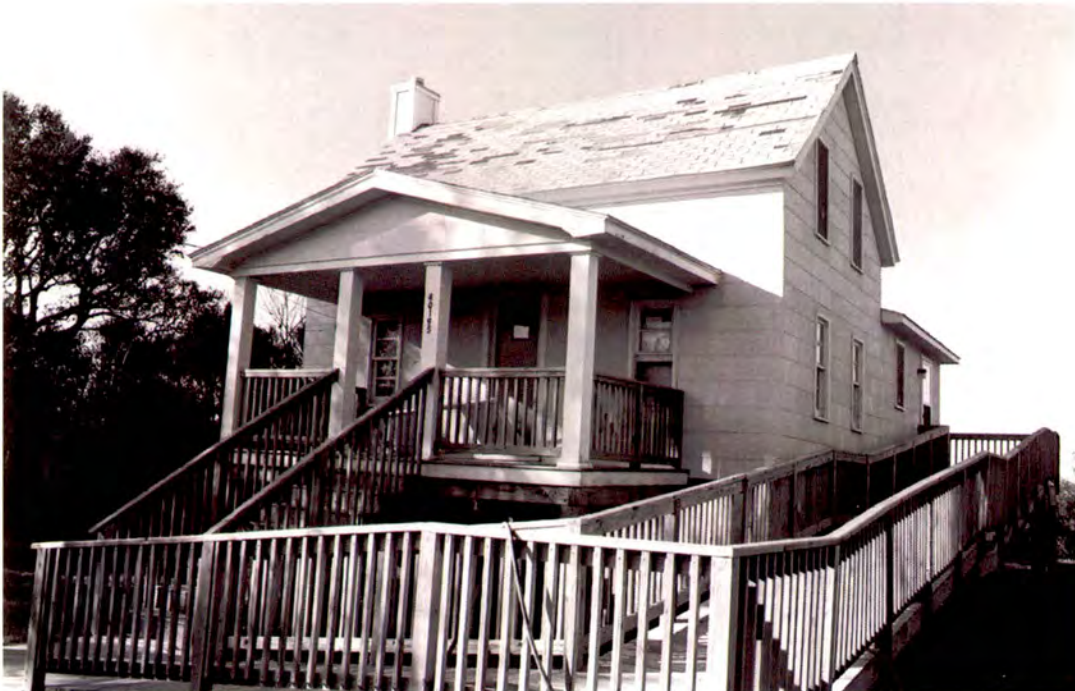
Plate 67: Thomas J. and Abelena Quidley Meekins House (#20) in Avon, south front and east side elevations
