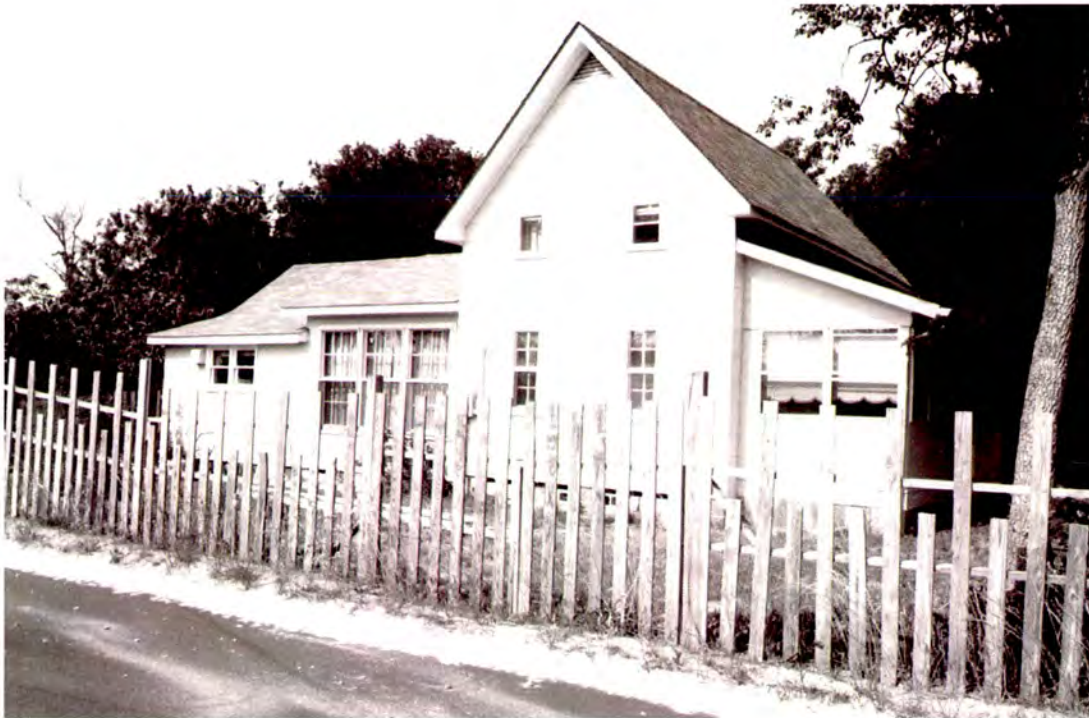
Plate 204: Farrow-Stowe-Hector House (#42) in Buxton, south front and west side elevations
