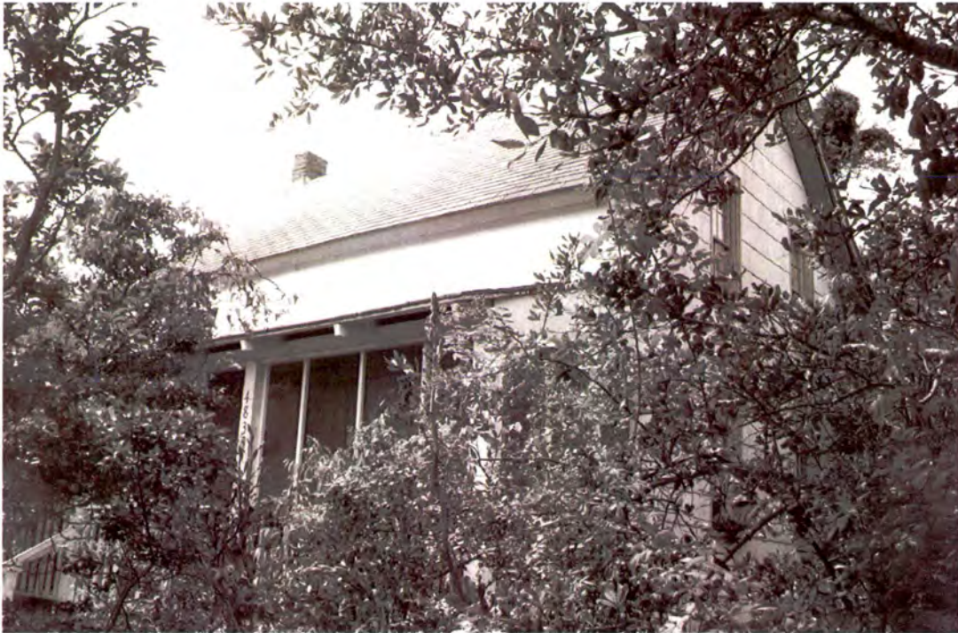
Plate 190: John A. and Brittonia Williams Gray House (#33) in Buxton, south front and east side elevations
