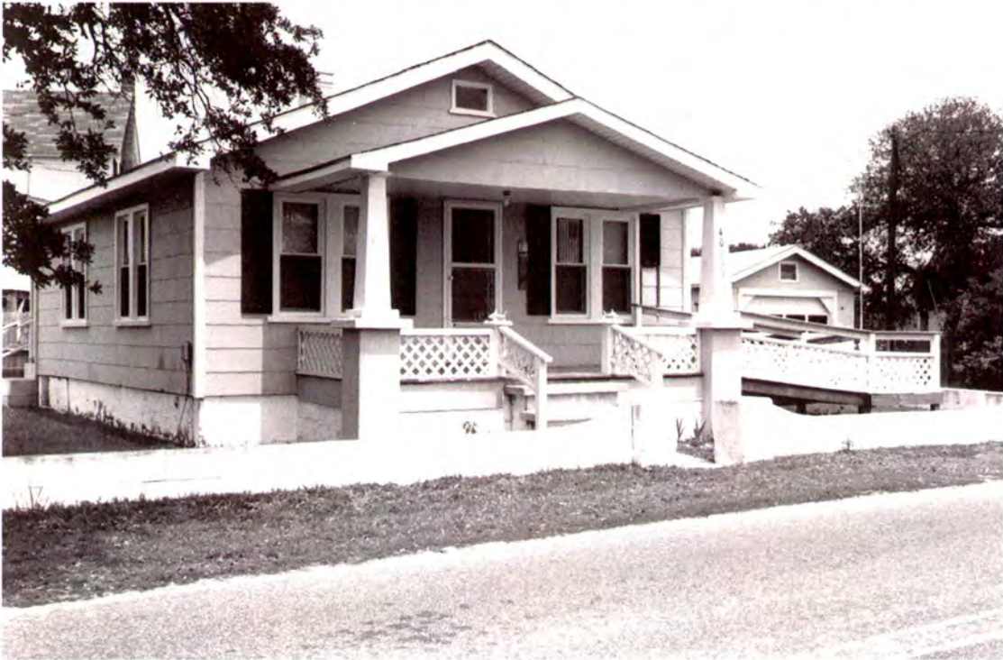
Plate 63: Virginia and Ralph Scarborough House (#16) in Avon, south front and west side elevations
