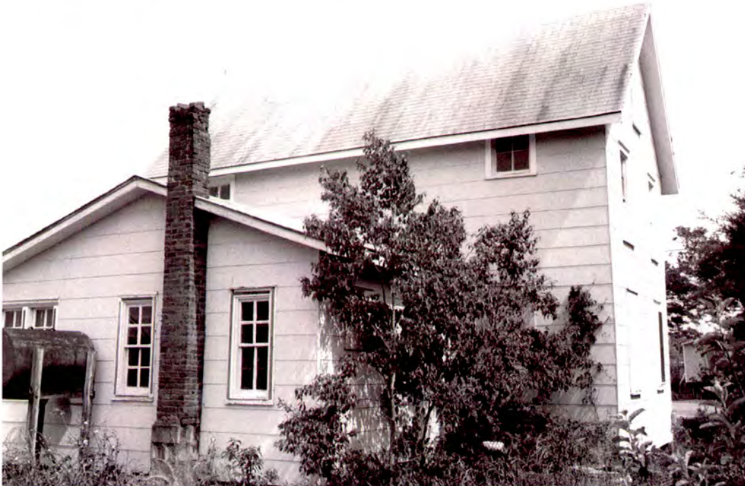
Plate 195: R. Hayes and Mary Foster Farrow House (#36) in Buxton, north rear and west side elevations
