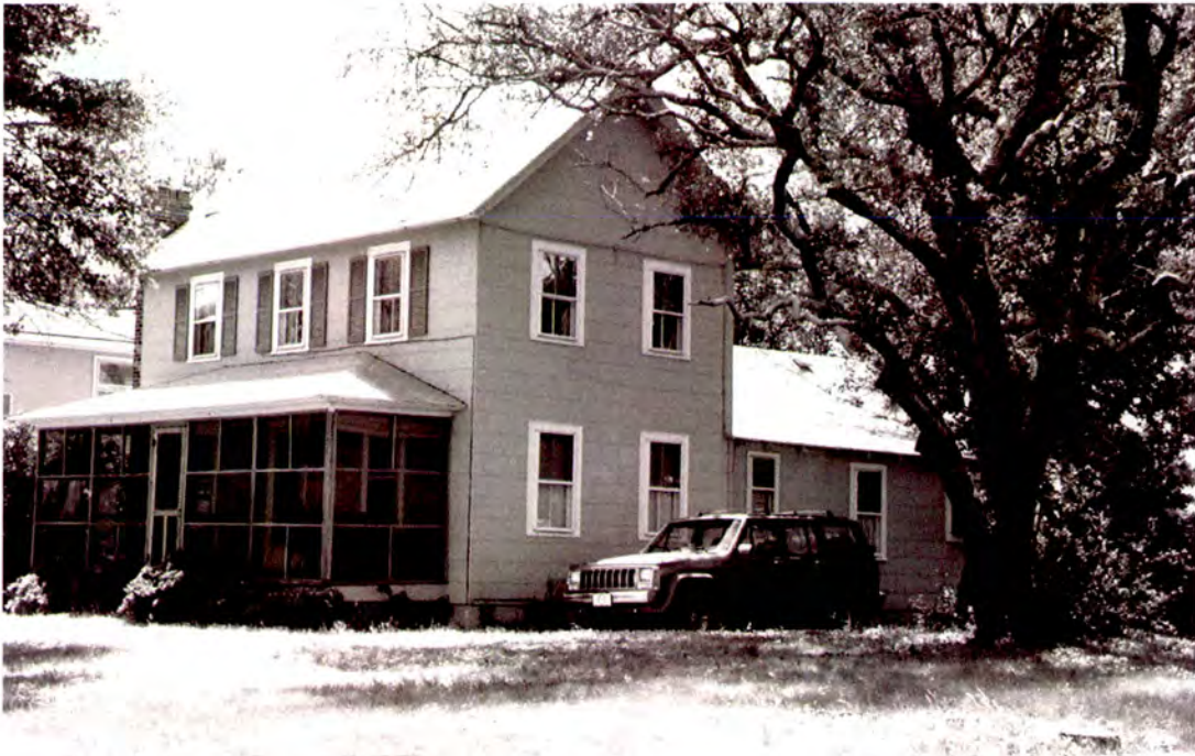
Plate 208: Simpson-Barnett House (#45) in Buxton, north front and west side elevations
