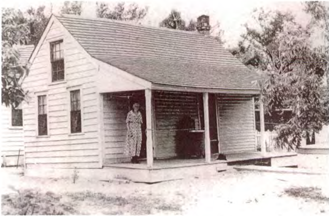
Plate 25: Story-and-a-jump Hatteras house in the early twentieth century (Courtesy of the North Carolina State Archives)
