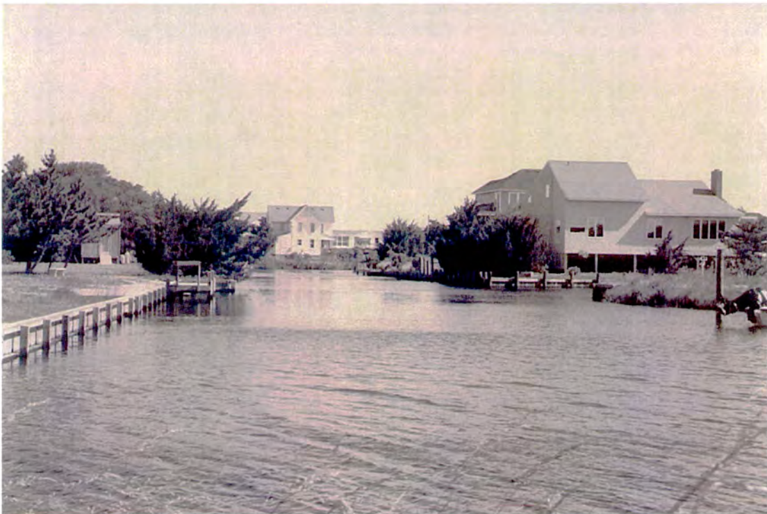
Plate 4: New houses and modern harbor on Pamlico Sound at southern edge of potential Avon Historic District, within APE of Buxton/Canadian Hole Area (R-4070C)
