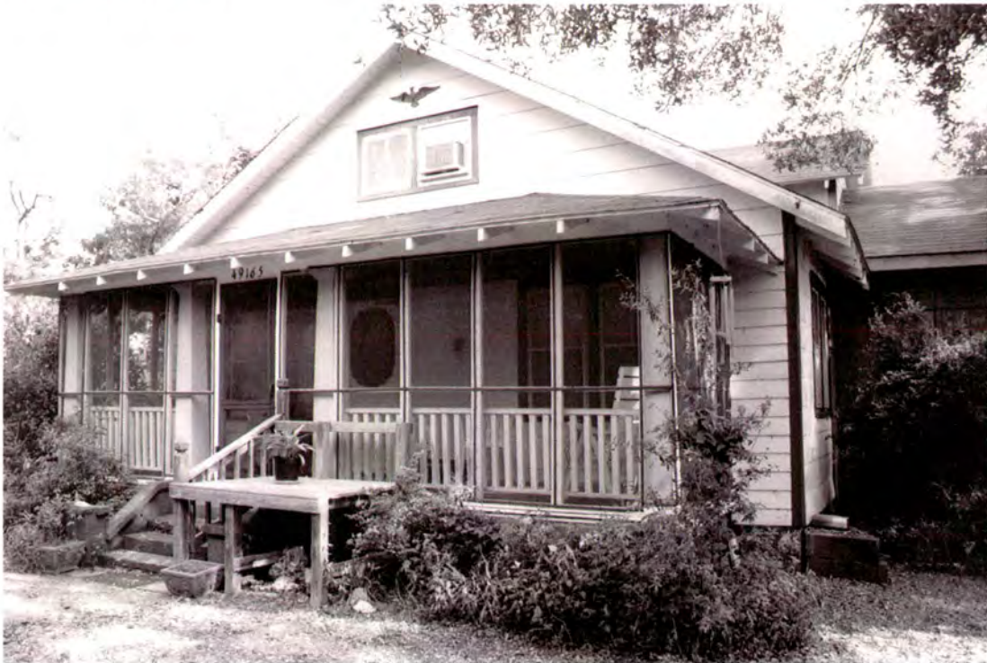
Plate 211: Burrus-Tolson House (#48) in Buxton, north front and west side elevations
