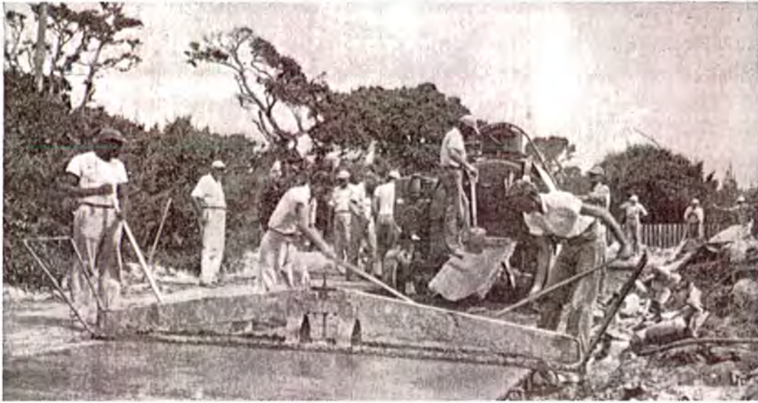
Plate 15: Paving of NC 12 on Ocracoke Island in 1950 (Source: Roadways , January/February 1951)
