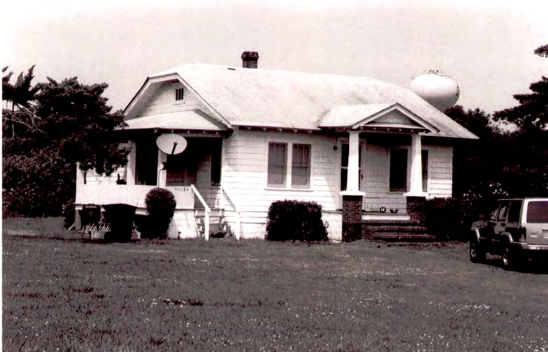
Plate 85: George and Mabel Meekins House (#38) in Avon, south front and west side elevations
