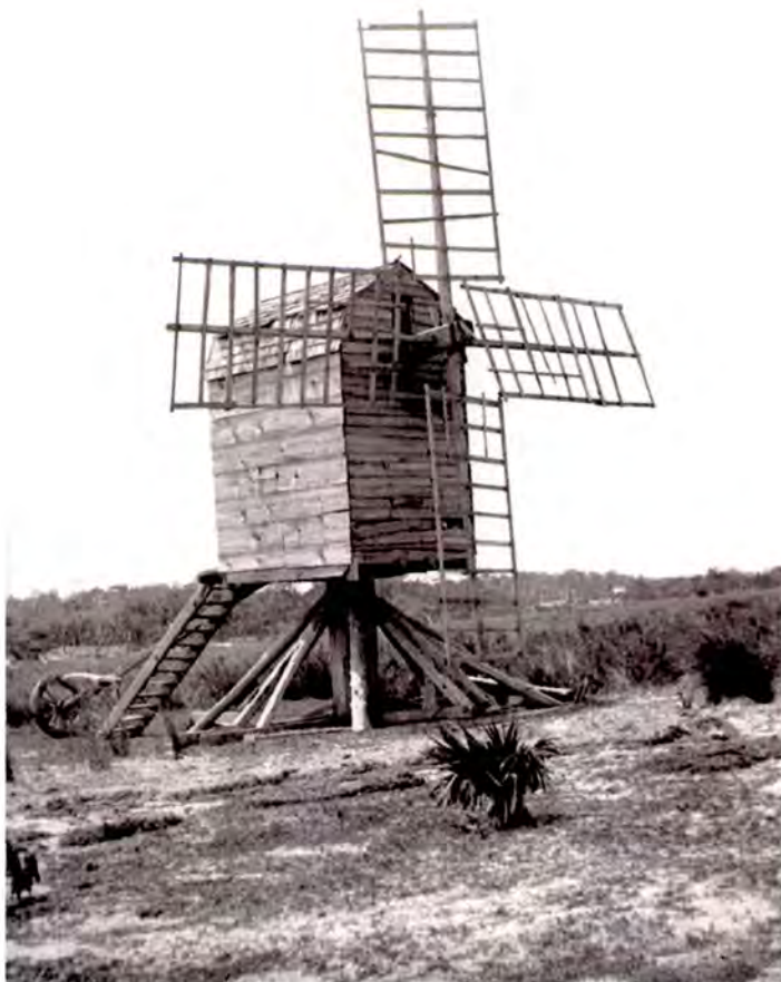
Plate 17: Captain Ben Midgett's corn-grinding windmill near Cape Hatteras at the turn of the century (Courtesy of the North Carolina State Archives)
