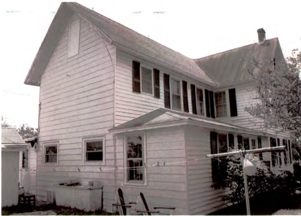
Plate 248: Urias O. and Caddie Midgett Gaskins House and Gaskins Cemetery (#8) – west side and north rear elevation of house
