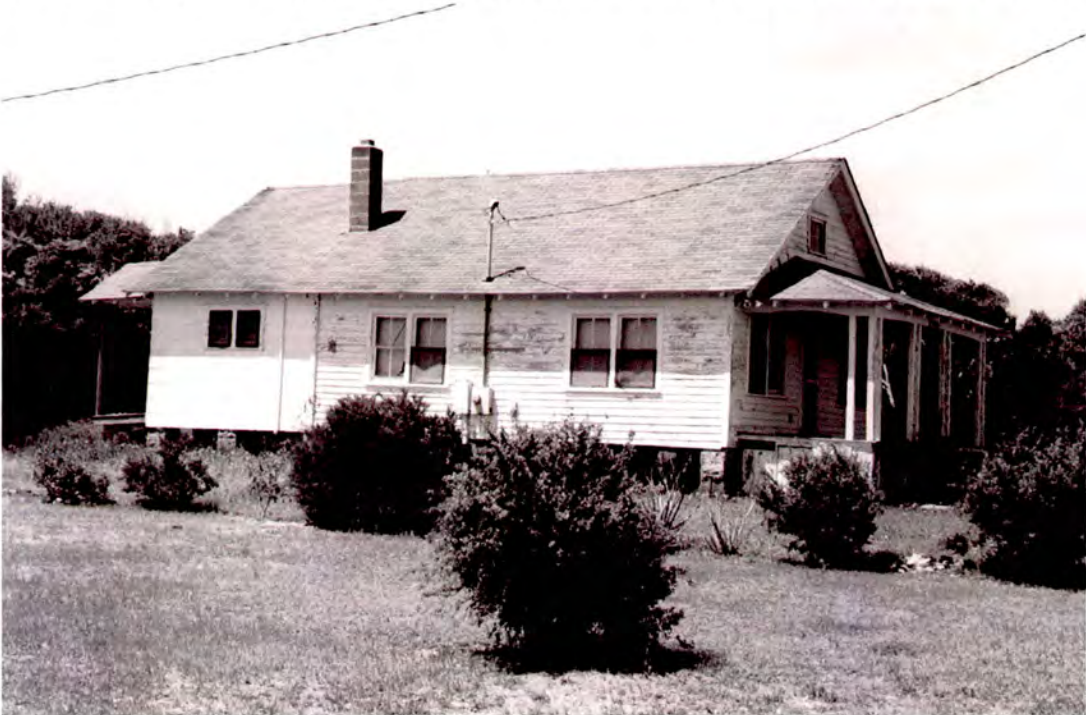
Plate 209: Whidbee-Rayle House (#46) in Buxton, east side and north front elevations
