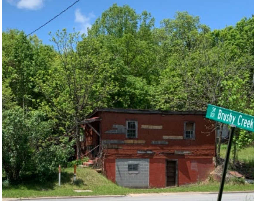
J. Myron & Ruth Greene Houston Outbuilding (NCDOT Survey May 2019)
