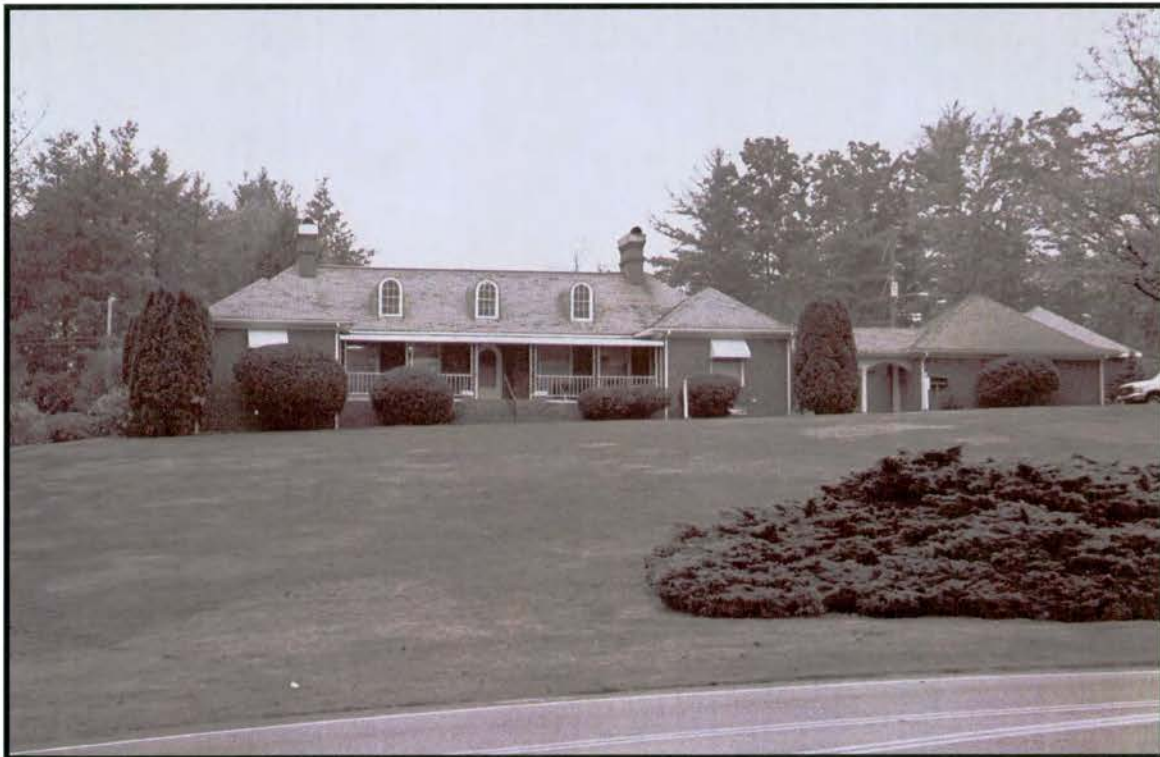
Plate 57: Carl and Mary Arrowood House – south front elevation in October 2004; note original dormers and asphalt-shingled roof
