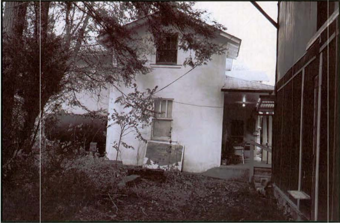
Plate 52: Sunny Brook Store – looking north at south side elevation of house and west rear elevation of store
