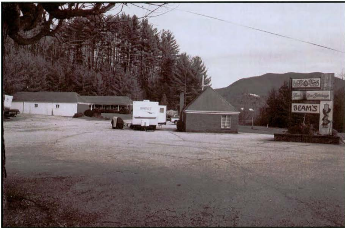
Plate 35: Beam's Motel and Restaurant – looking east from restaurant toward motel at left, office at center, and planter with sign at right
