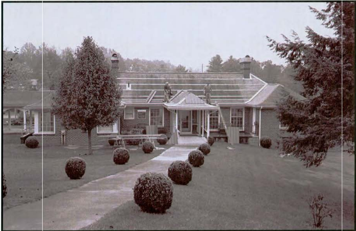
Plate 59: Carl and Mary Arrowood House –north rear elevation in November 2004; note construction of new roof and rear entryway
