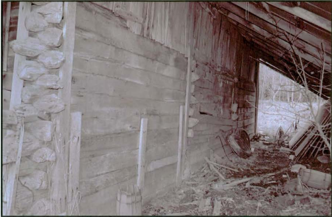
Plate 17: R.L. Hall Log Barn – east side elevation; note frame infill between projecting ends of logs at right center
