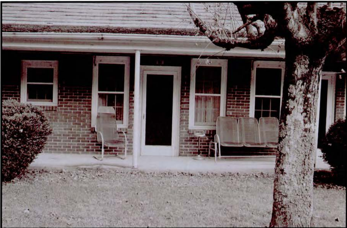
Plate 41: Beam's Motel and Restaurant – looking east toward motel unit number 13
