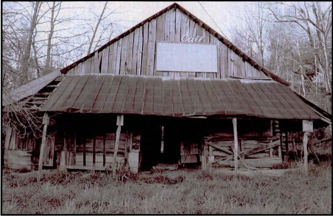
Plate 15: R.L. Hall Log Barn – south front elevation
