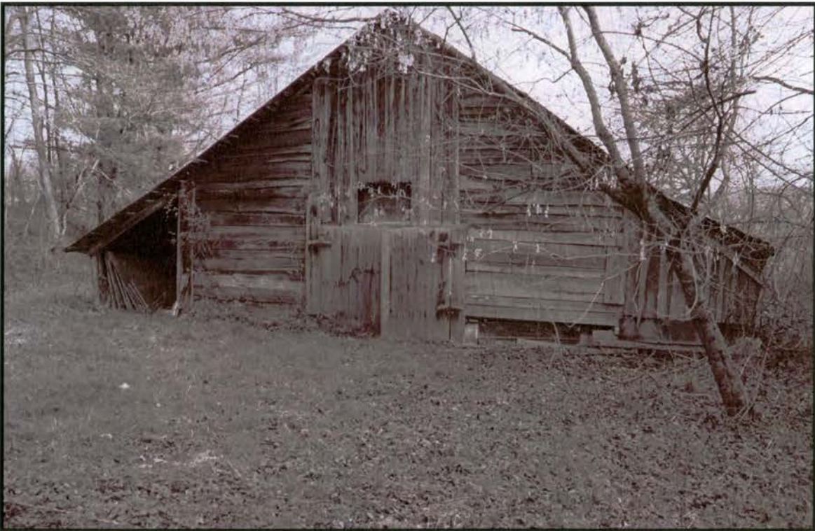
Plate 22: R.L. Hall Log Barn – west side and north rear elevations
