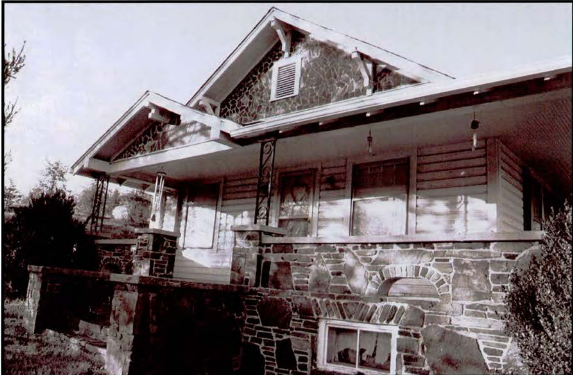
Plate 69: Homer and Golda Rutledge Grindstaff House – south front elevation; note stonework of porch and gable
