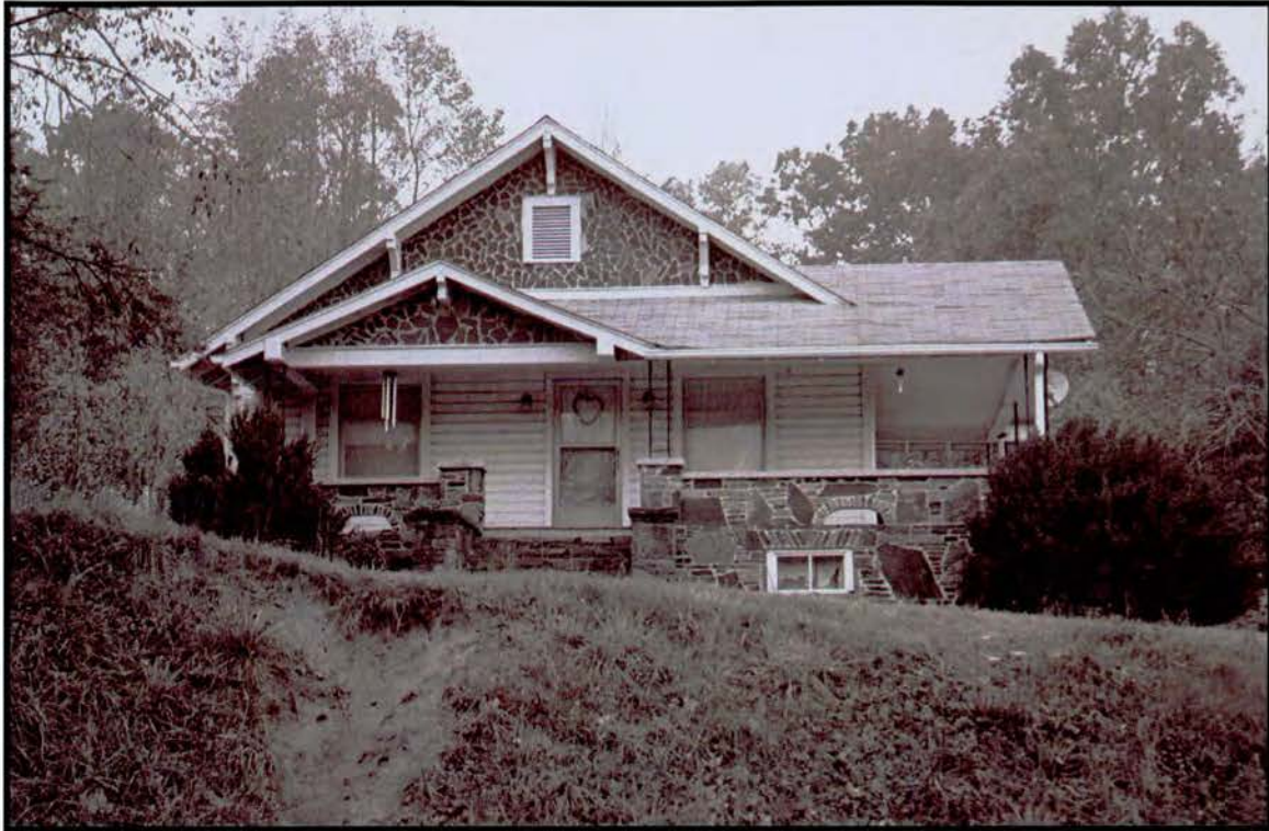
Plate 68: Homer and Golda Rutledge Grindstaff House – south front elevation
