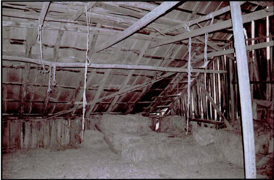
Plate 28: R.L. Hall Log Barn – hay loft
