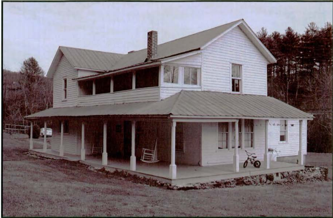
Plate 70: Sunnybrook Farmhouse – south side and west front elevations
