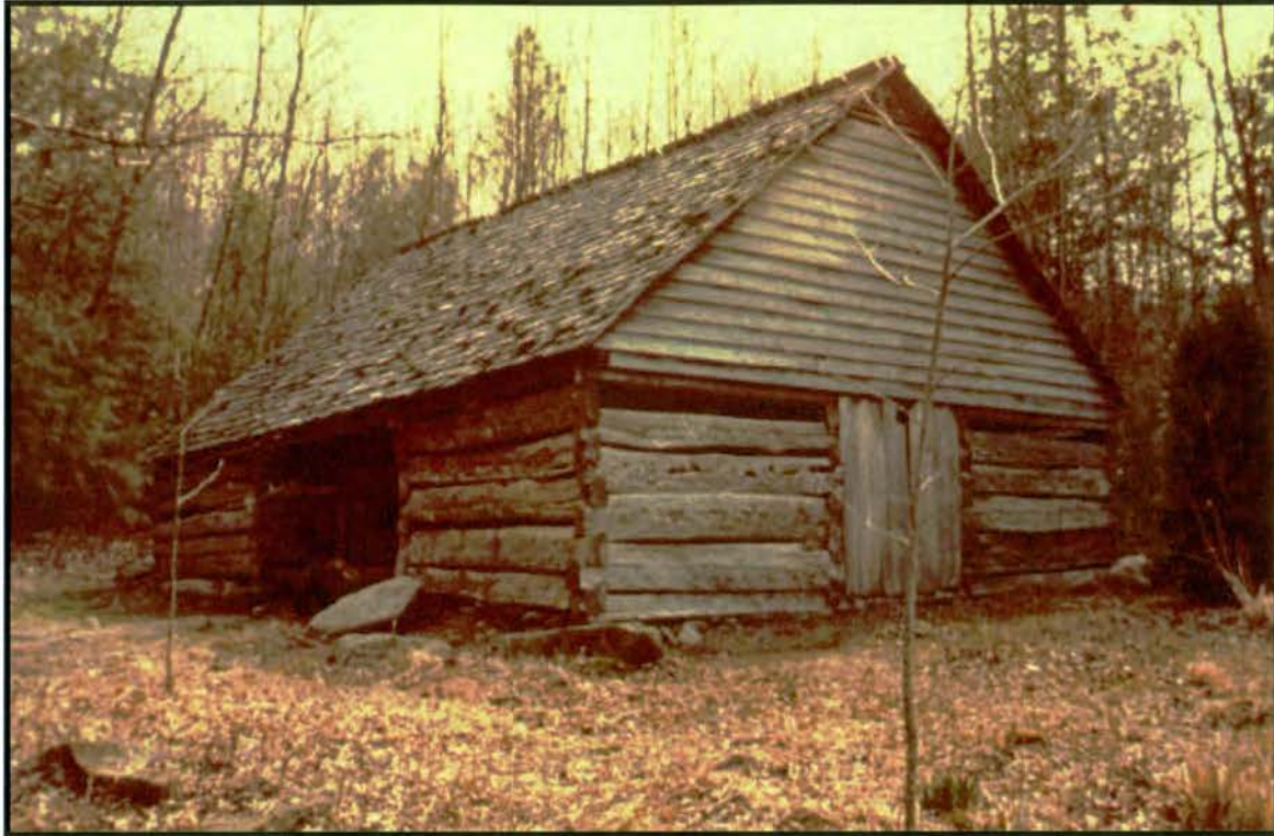
Plate 13: Tennessee example of a four-crib log barn converted to a transverse passage barn (with entry at long rather than gable end) (Source: Digital Library of Appalachia: Log Structure 58)
