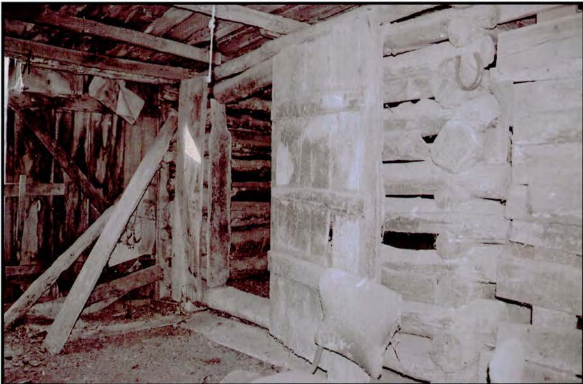
Plate 25: R.L. Hall Log Barn – transverse passage and entry to northeast log crib/stall
