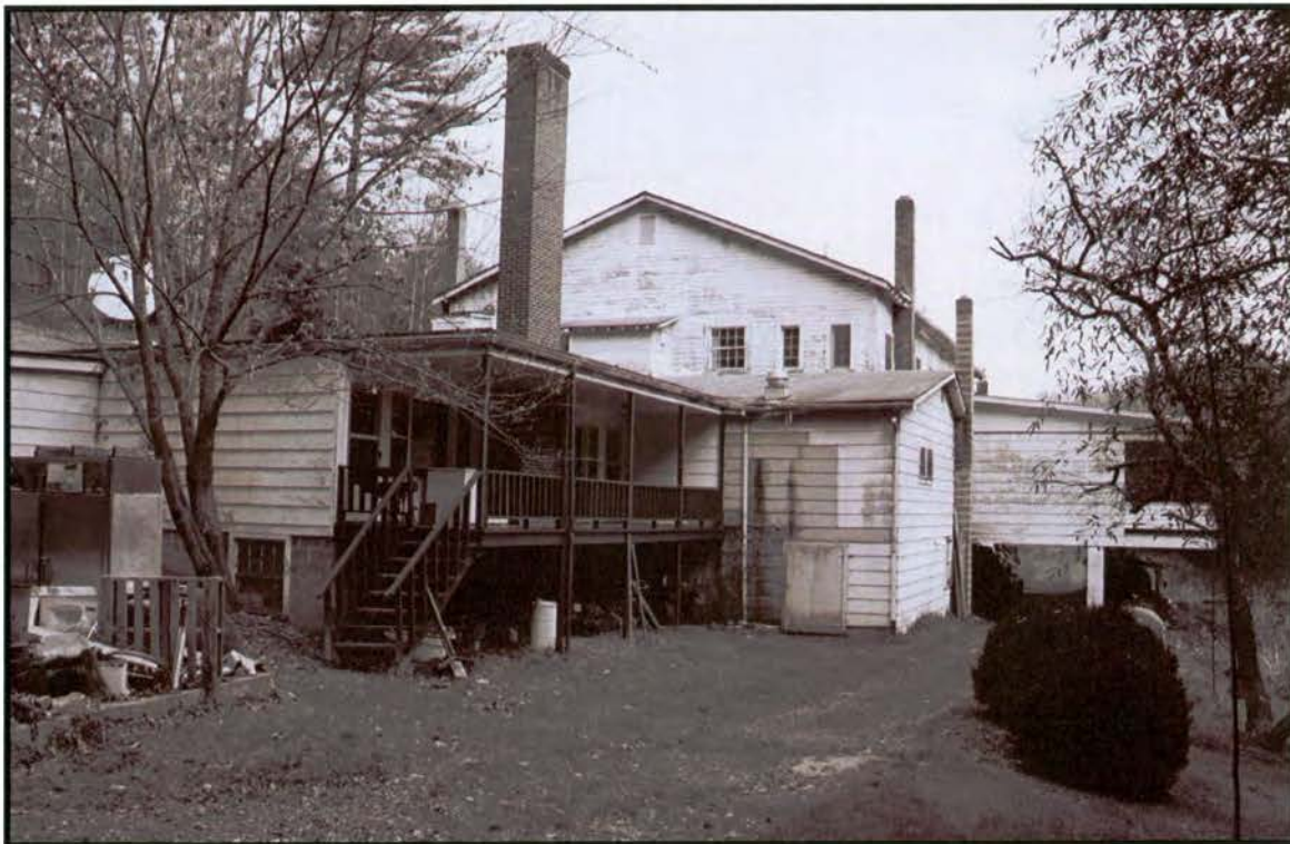
Plate 33: Beam's Motel and Restaurant – west rear and south side elevations of restaurant
