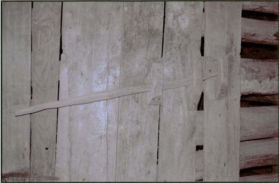
Plate 26: R.L. Hall Log Barn – detail of crib/stall door
