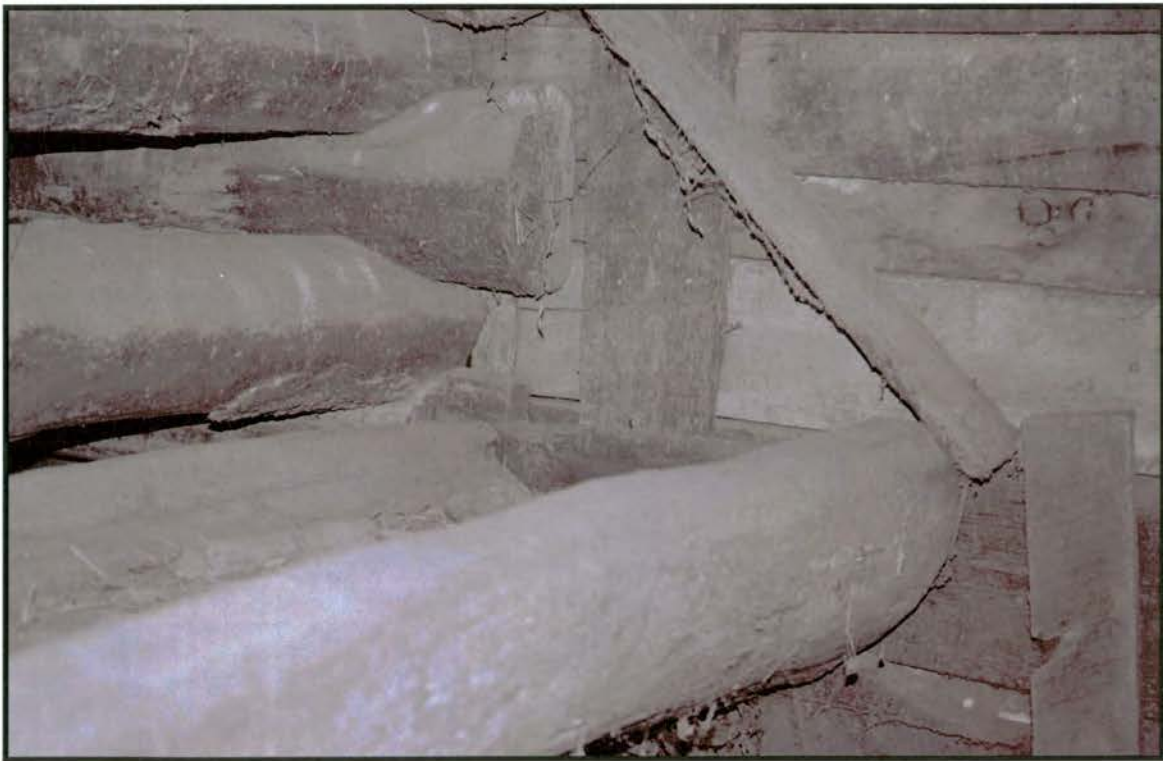
Plate 27: R.L. Hall Log Barn – detail of hollowed log trough in crib/stall
