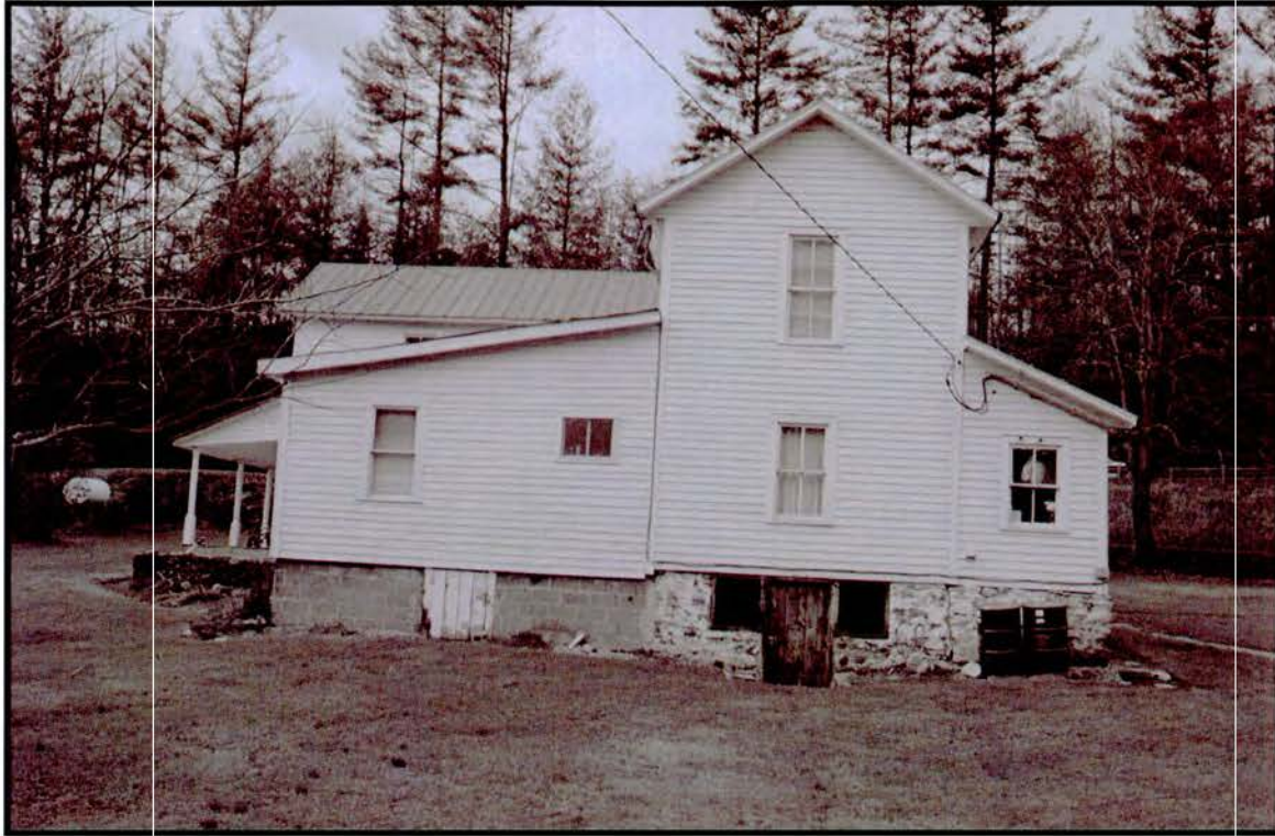
Plate 74: Sunnybrook Farmhouse – east rear elevation
