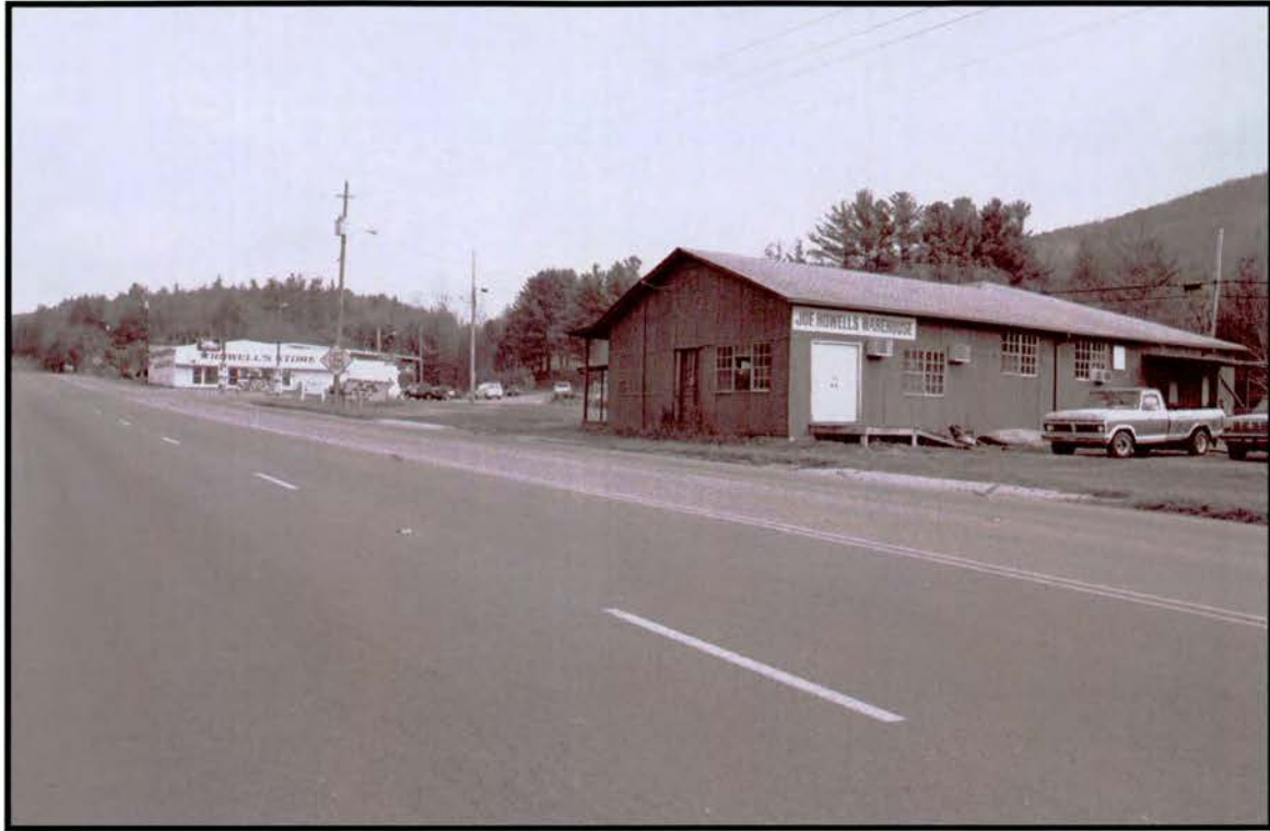
Plate 1: Looking northeast towards late twentieth-century commercial buildings at junction of US 19E and SR 1106 at northern end of APE, Avery County
