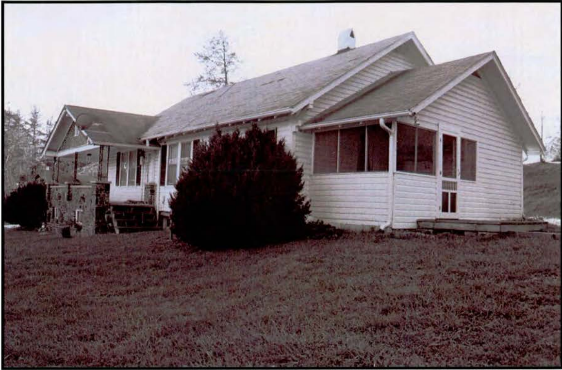
Plate 66: Homer and Golda Rutledge Grindstaff House – east side and north rear elevations
