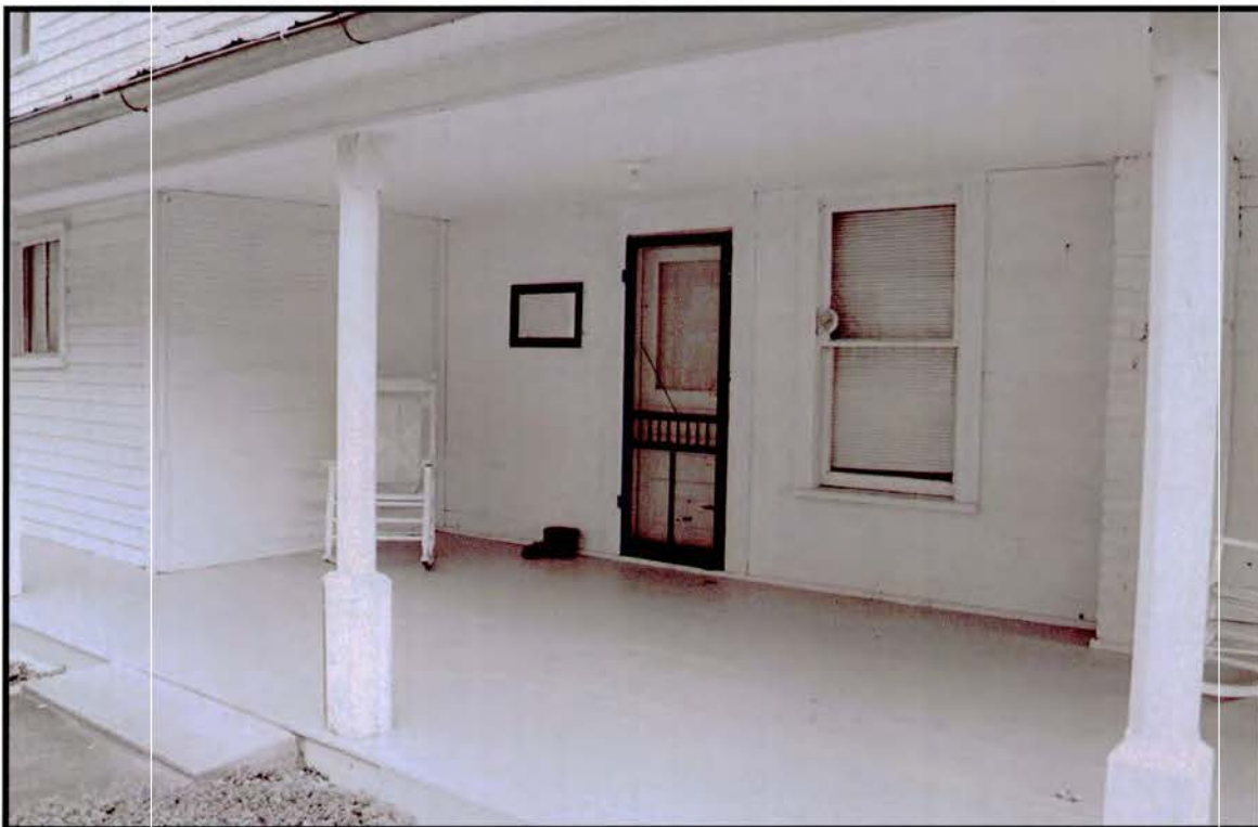
Plate 75: Sunnybrook Farmhouse – looking northeast at front porch; note German siding at left, ceiling board at left center, and flush boards at plane of entry; also note modern one-over-one sash
