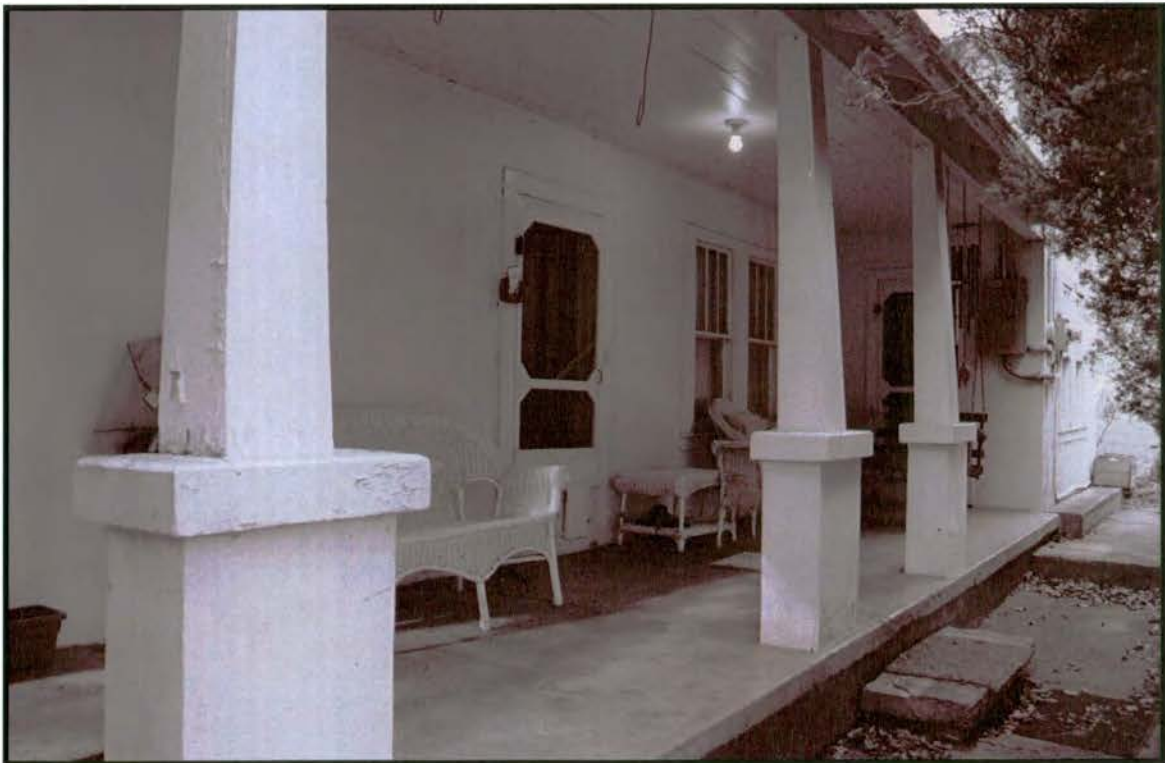
Plate 51: Sunny Brook Store – porch and east front elevation of house
