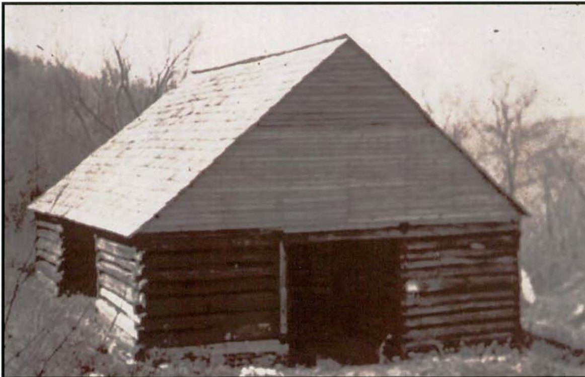
Plate 14: Tennessee example of a four-crib log barn retaining original cross passageway (Source: Digital Library of Appalachia: Log Structure 57)
