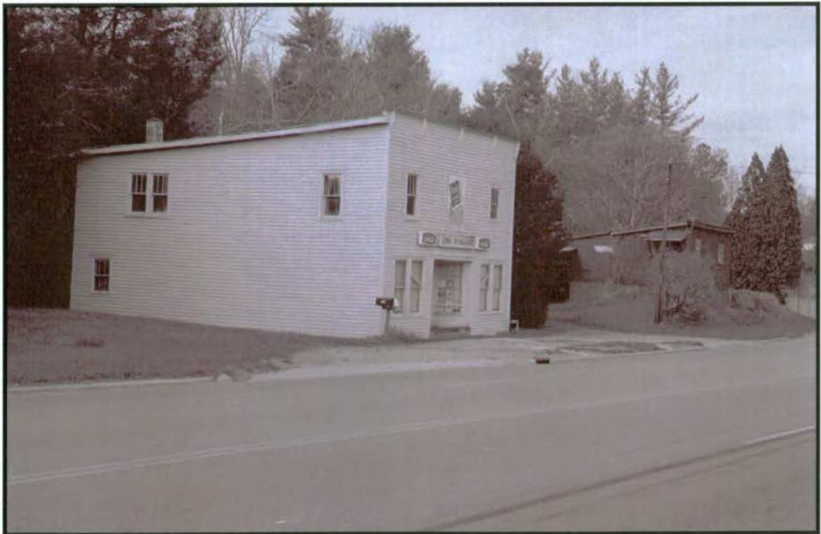
Plate 49: Sunny Brook Store – looking northwest at south side and east front elevations of store; garage/shed at right
