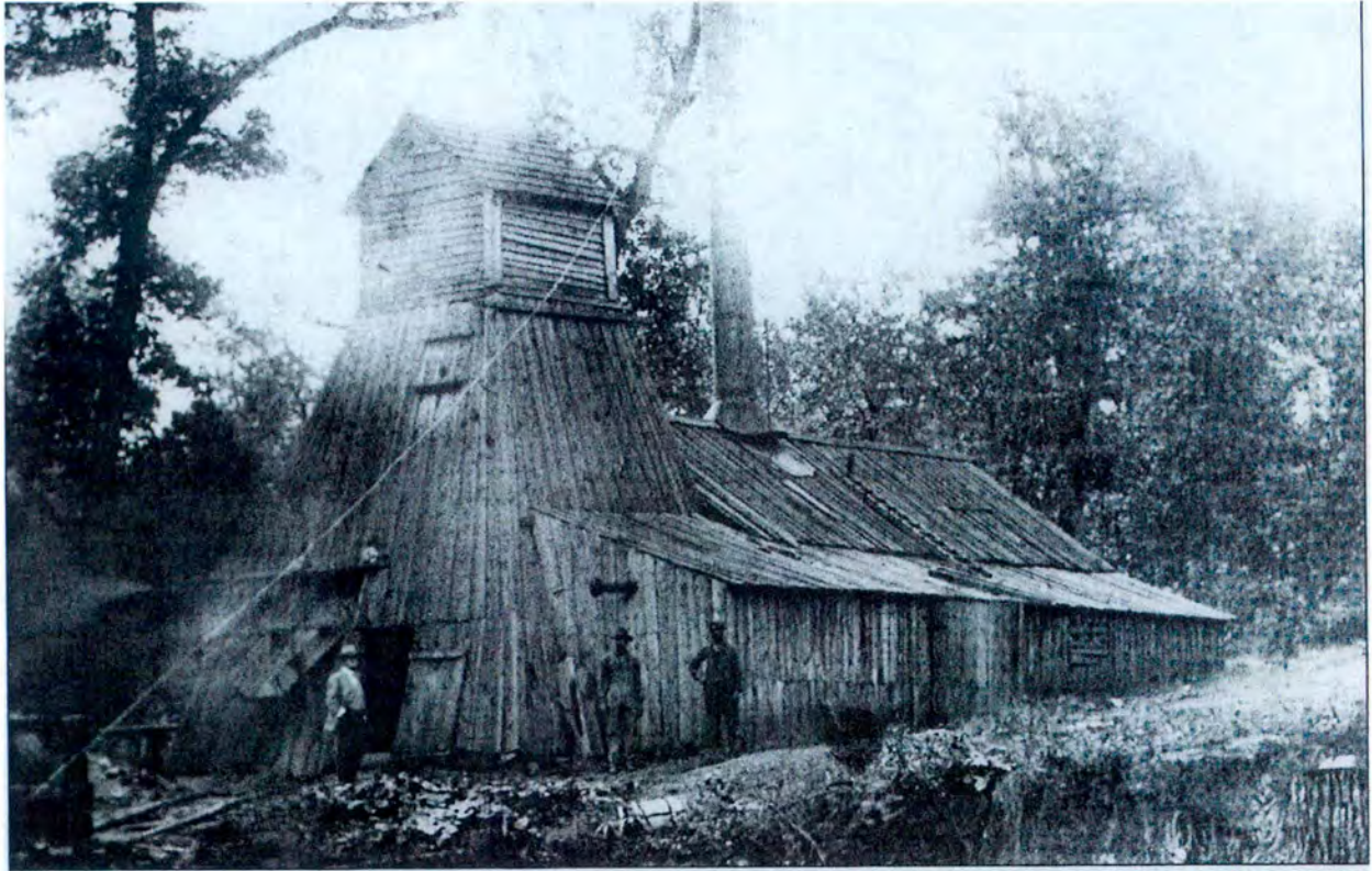
Plate 3: Headframe of the Ross Mine near Gaffney, c.1908 (Source: Lininger's "History of the Ross Mine," 1997)
