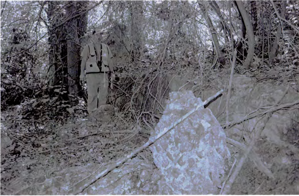
Plate 9: Concrete and brick foundation at first mill site
