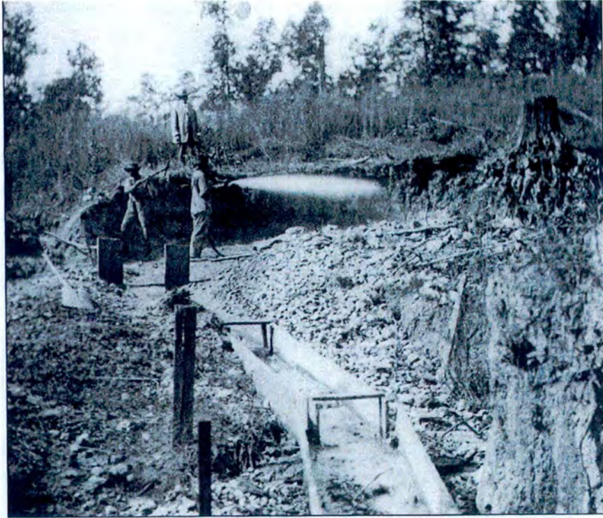
Plate 1: Placer mining and sluicing activities at the Ross Mine near Gaffney, c.1908 (Source: Lininger's "History of the Ross Mine," 1997)
