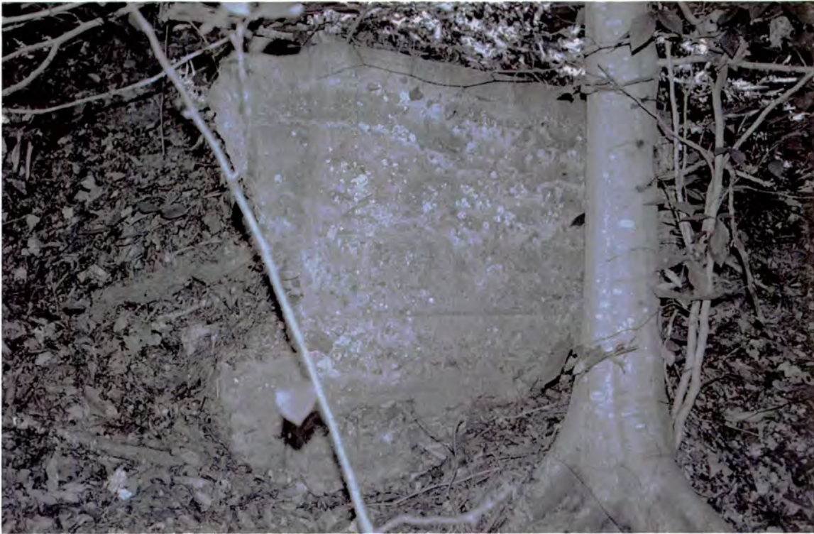
Plate 8: Concrete footing or foundation at first mill site
