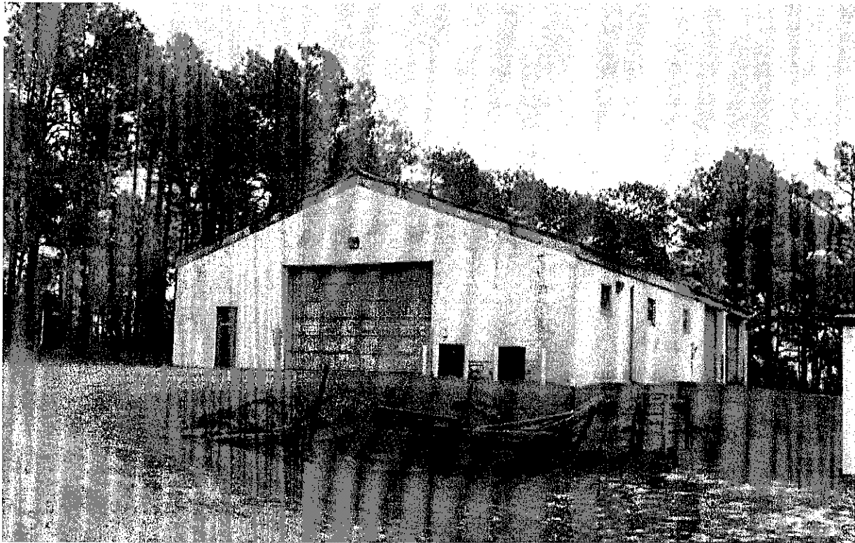
Plate 30: Southern Pines Motor Vehicle Storage Building
