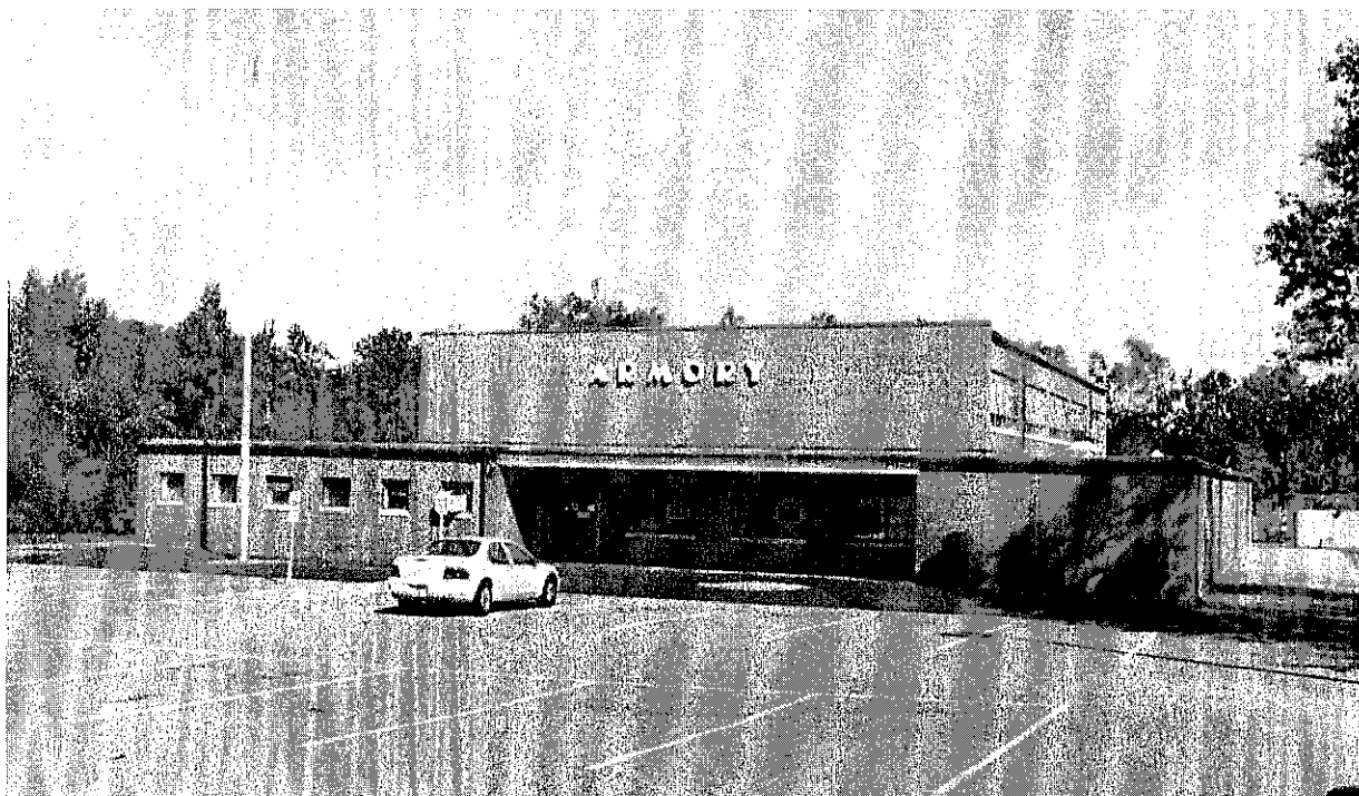
Plate 34: Thomasville National Guard Armory
