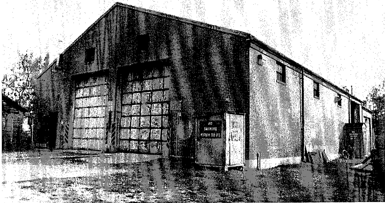
Plate 40: Youngsville Motor Vehicle Storage Building
