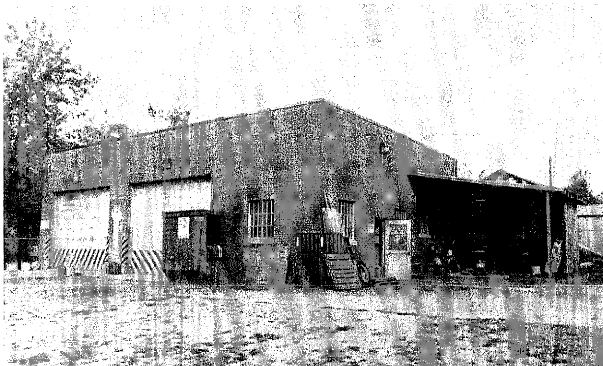
Plate 41: Youngsville Organizational Maintenance Shop
