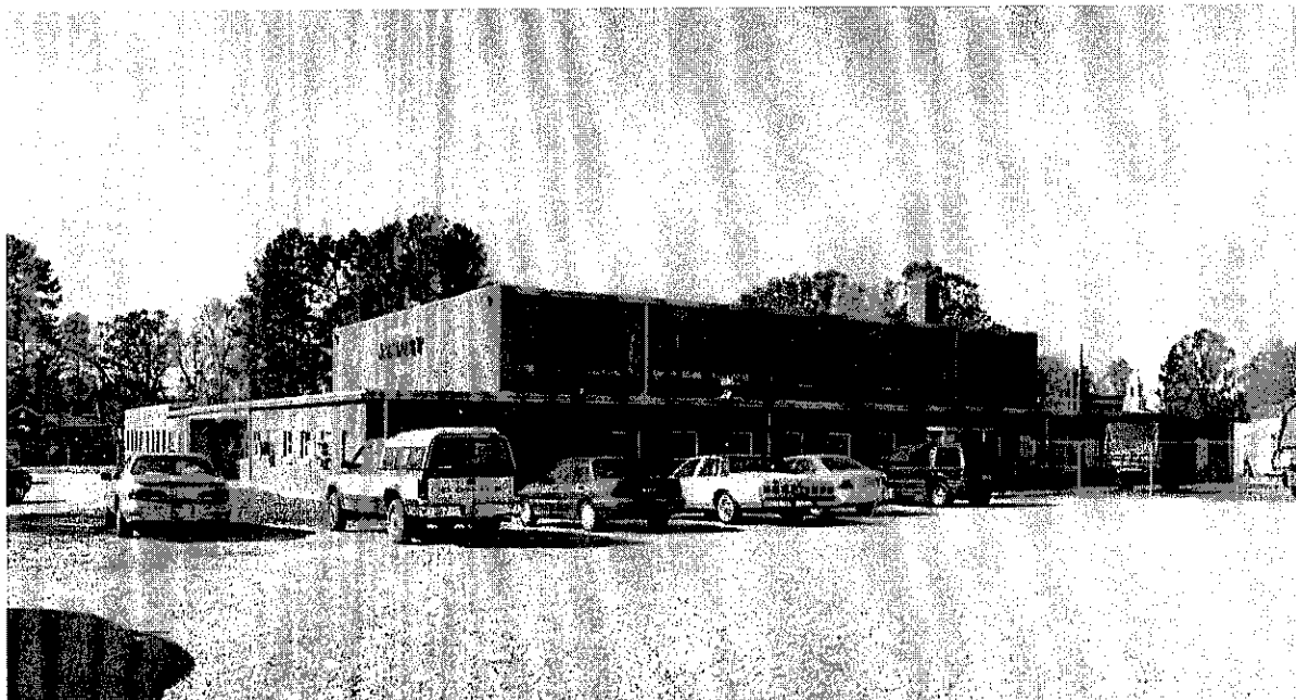
Plate 4: Ahoskie National Guard Armory
