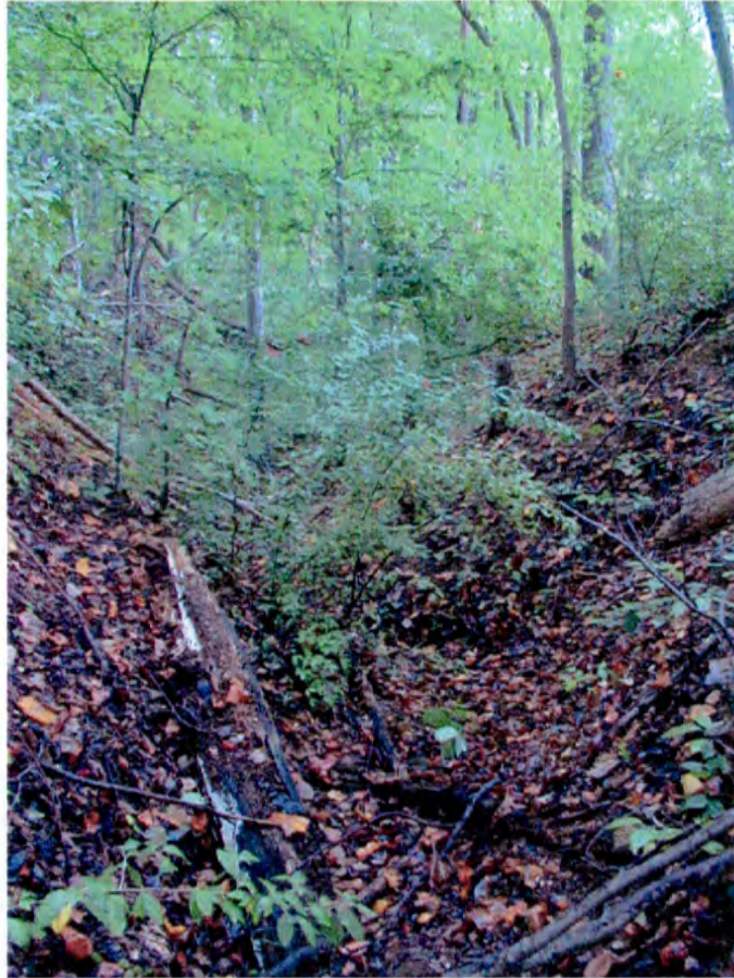
Fig. 4: Abandoned Roadbed north of Gallimore Dairy Road
