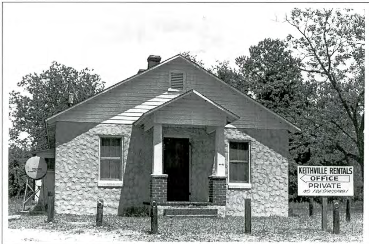
Plate 4: Keithville Rental Units, Office, Looking Southeast
