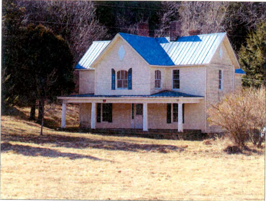
Photo 5 A. A. Woodruff House South Façade
