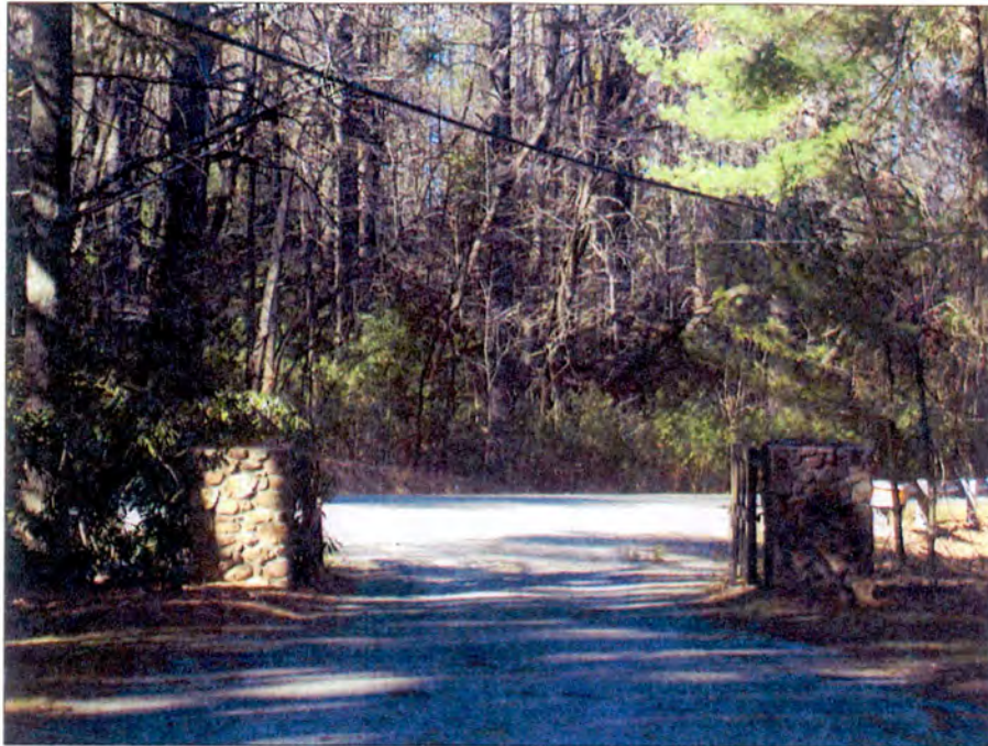
Photo 51 Hollyday Main Stone Gates
