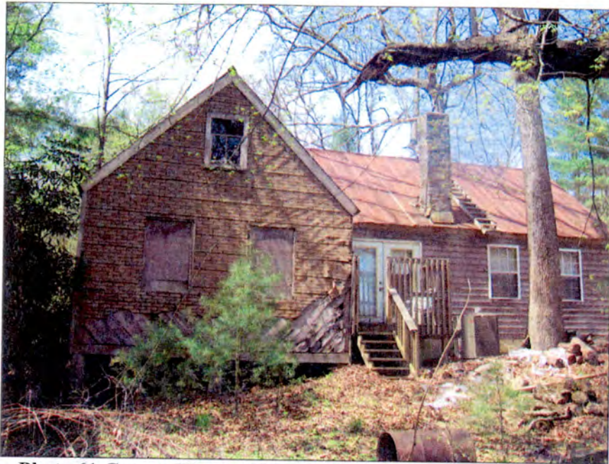
Photo 61 George Woodruff Service Station Southeast Elevation
