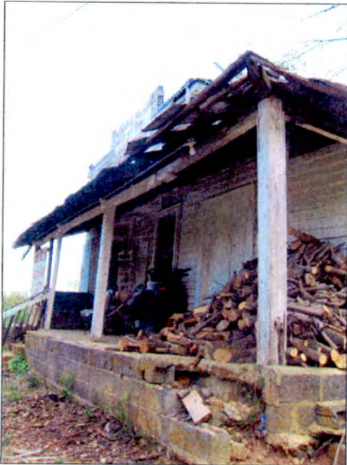
Photo 68 Old Miles Store Detail of porch foundation.
