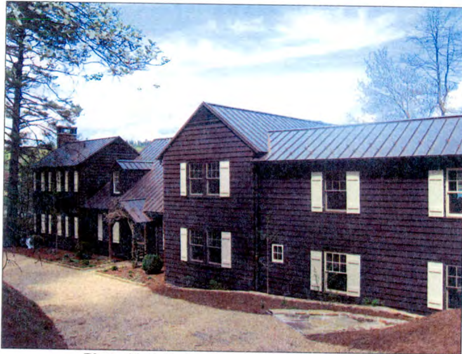
Photo 28 Hollyday Main House West Façade
