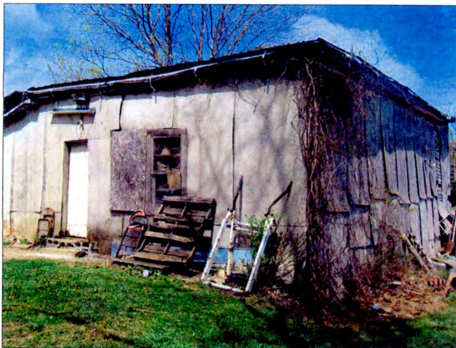
Photo 66 Old Miles Store West elevation
