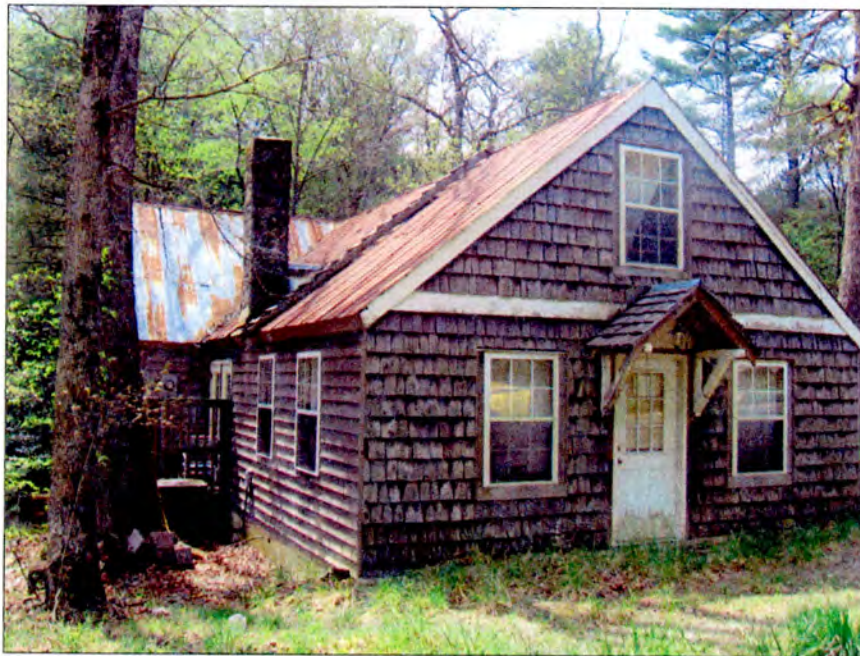
Photo 60 George Woodruff Service Station Southwest ¾ View
