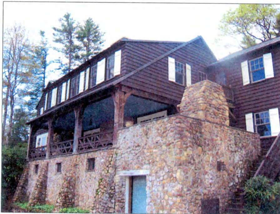
Photo 30 Hollyday Main House East elevation
