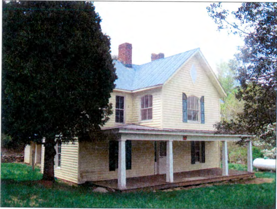
Photo 6 A. A. Woodruff House South Façade
