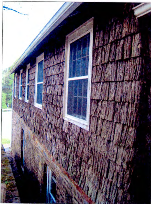
Figure 56 Inskeep's Store Detail of Bark Siding
