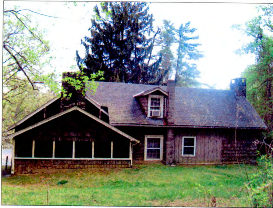
Figure 55 Inskeep's Store West elevation
