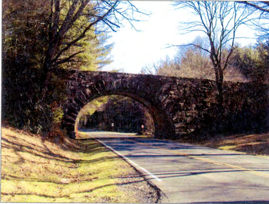
Photo 58 Stone Arch Bridge of Blue Ridge Parkway Looking South on US 21
