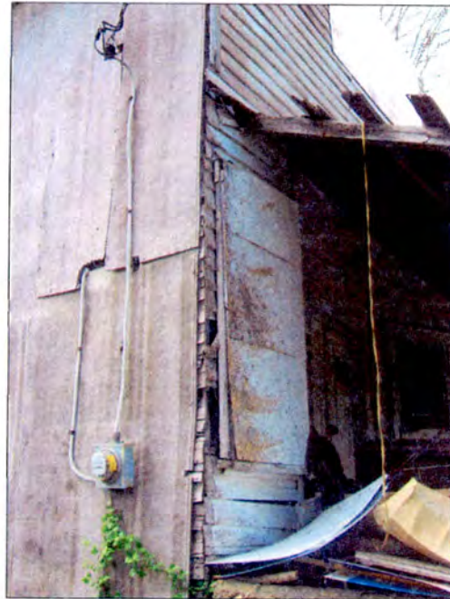
Photo 69 Old Miles Store Detail of exterior wall materials.
