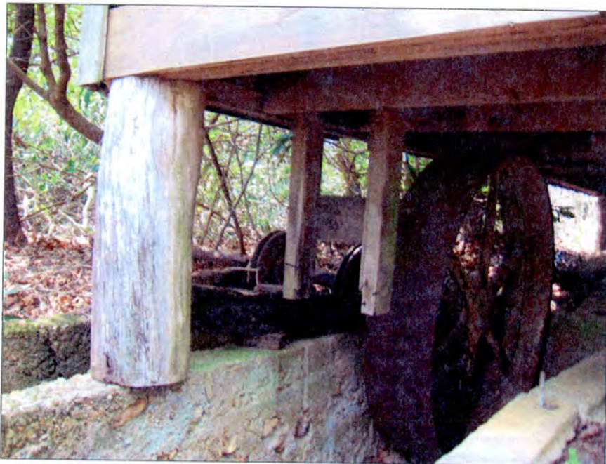
Photo 62 George Woodruff Service Station detail of water wheel
