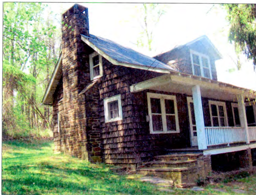
Figure 54 Inskeep's Store (Residence) Southwest \frac{3}{4} view
