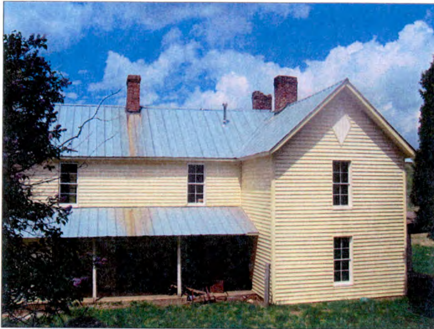
Photo 7 A. A. Woodruff House West Elevation
