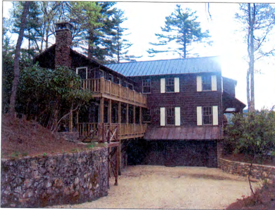
Photo 29 Hollyday Main House Southeast ¾ view
