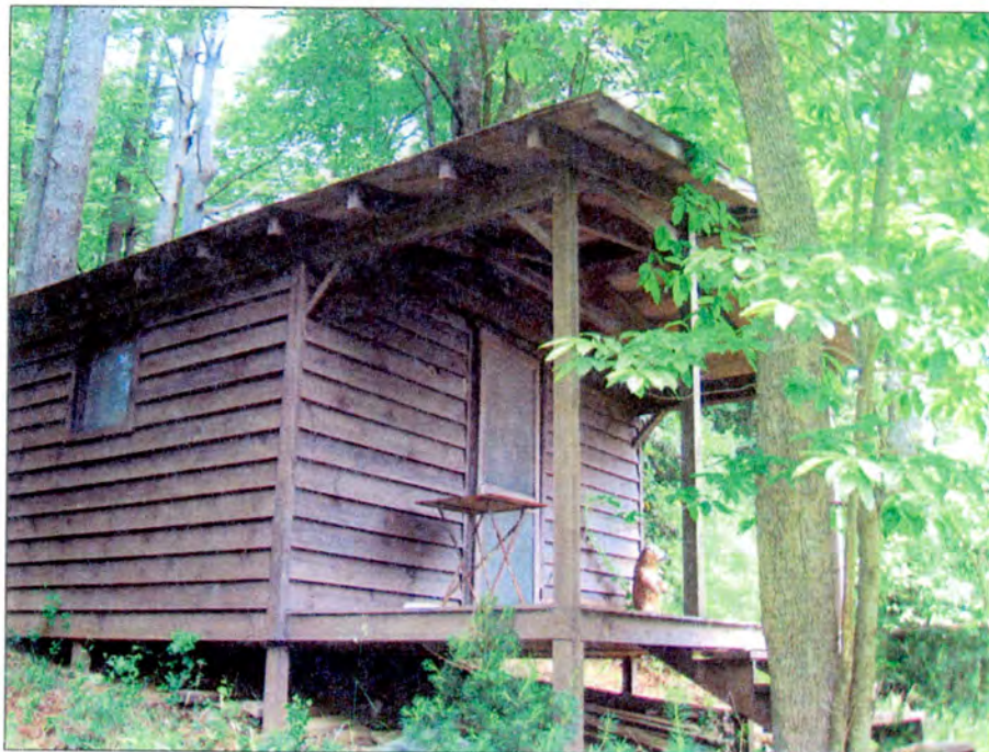
Photo 50 Hollyday Picnic House Southeast 3/4 View
