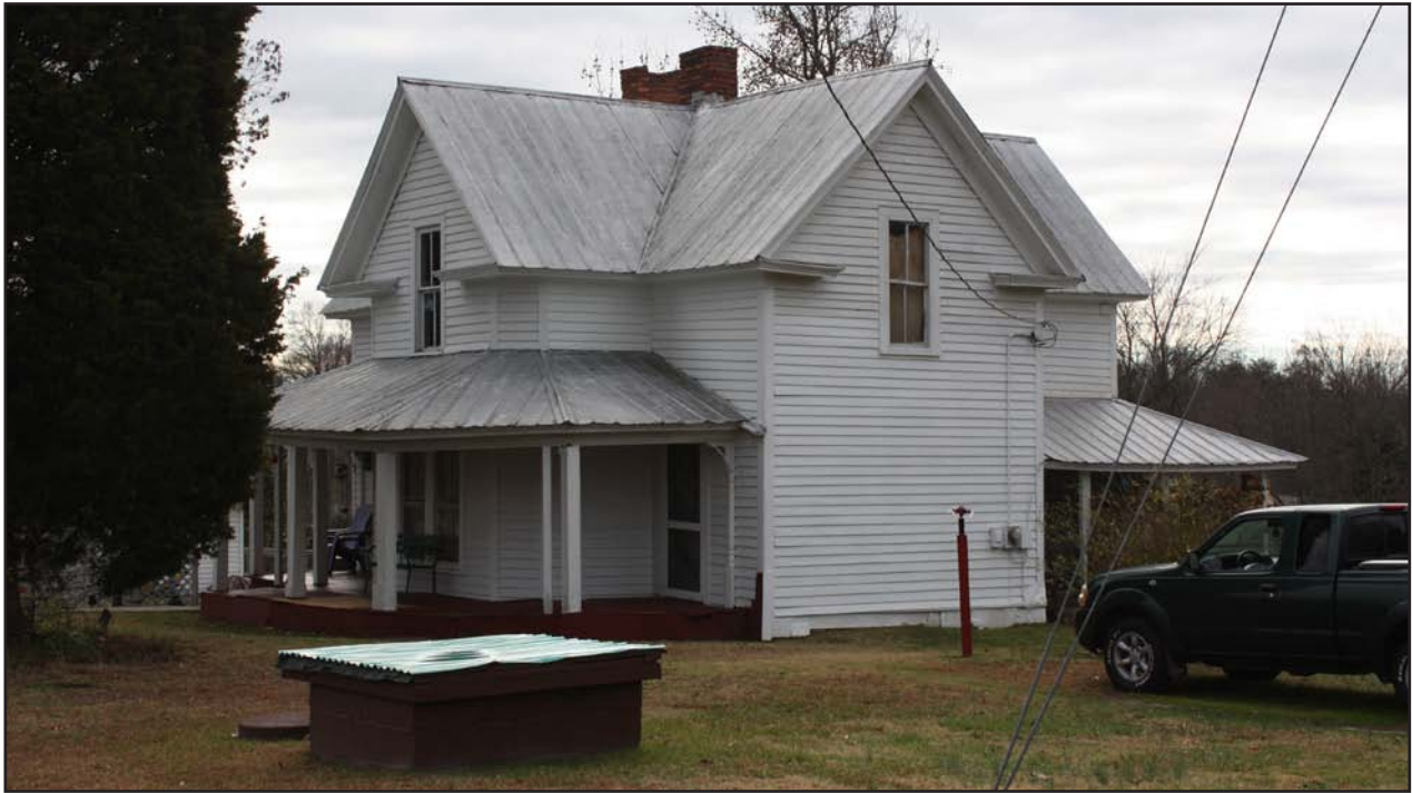
Figure 37. GF 8294 North Oblique
