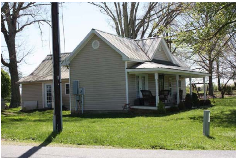
GF 8465 7725 Athens Road
