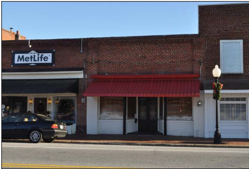
Figure 105. Powell's Drugstore Contextual Façade, Southwest Elevation
