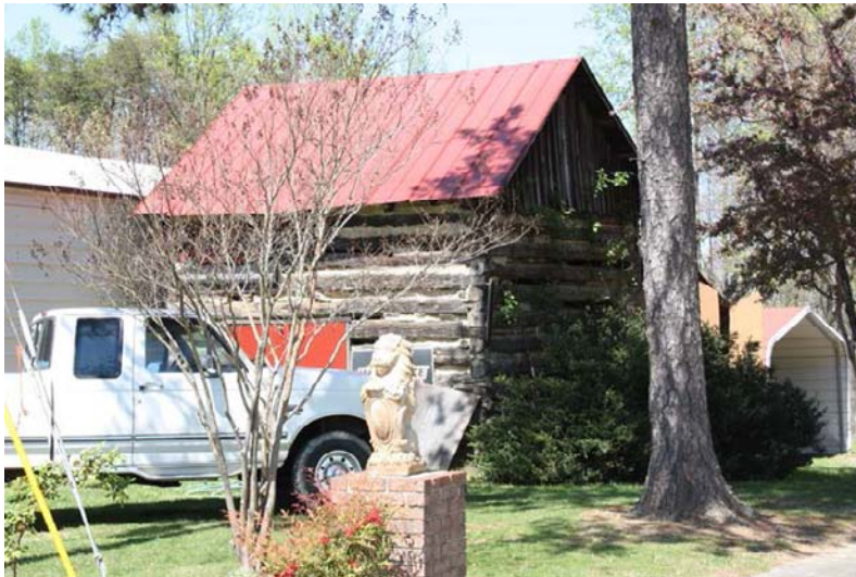
GF 8461 7984 Lester Road
