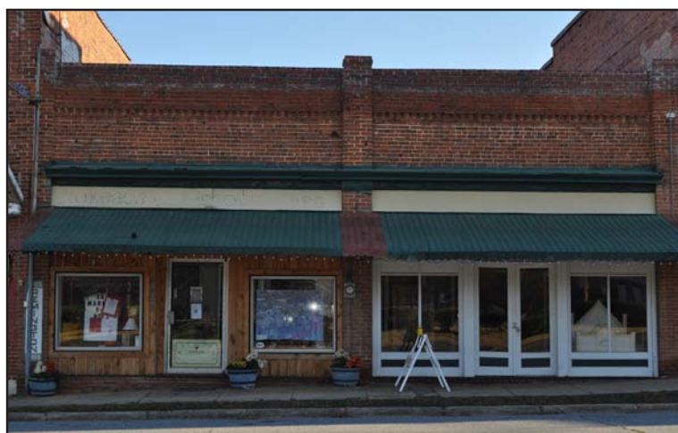
Figure 78. Tom Southard's Shoe Shop/Doreen's Beauty Shop and Raymond Angel's Barber Shop Façade, Southwest Elevation
