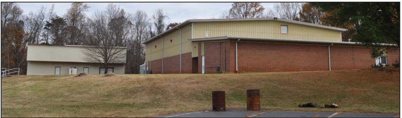
Figure 17. Edgewood Baptist Church Gymnasium (Right) and Maintenance Building (Left)
