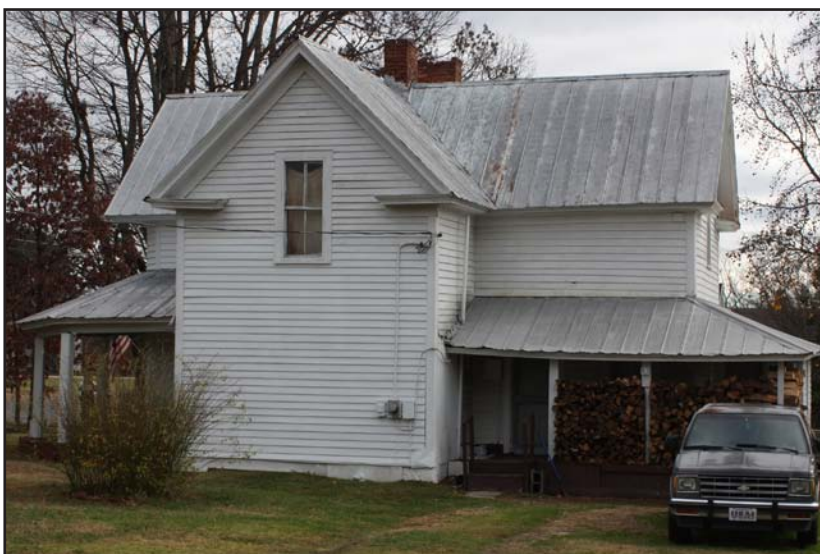
Figure 36. GF 8294 Northwest Elevation
