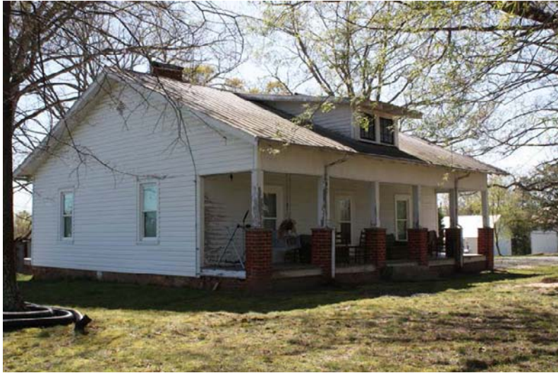
GF 8475 8415 Spotswood Road
