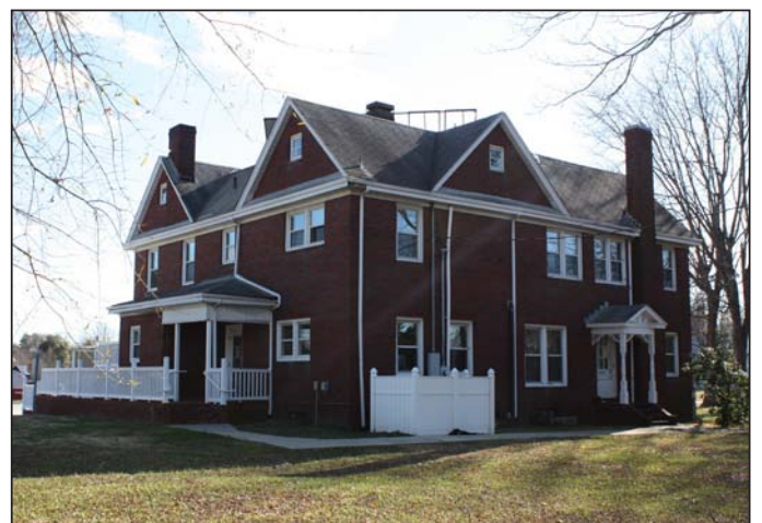
Figure 65. Taylor-Edwards House North Oblique
