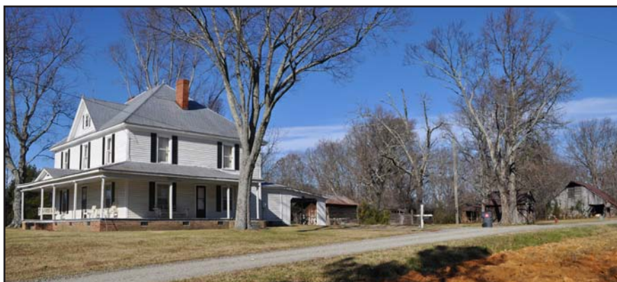
Figure 143. Left to Right, View Northwest: Wray House [A], Storage Building [E], Chicken Coop [C], Undetermined Outbuilding [G], General Storage Building [F], Large Barn [B]
