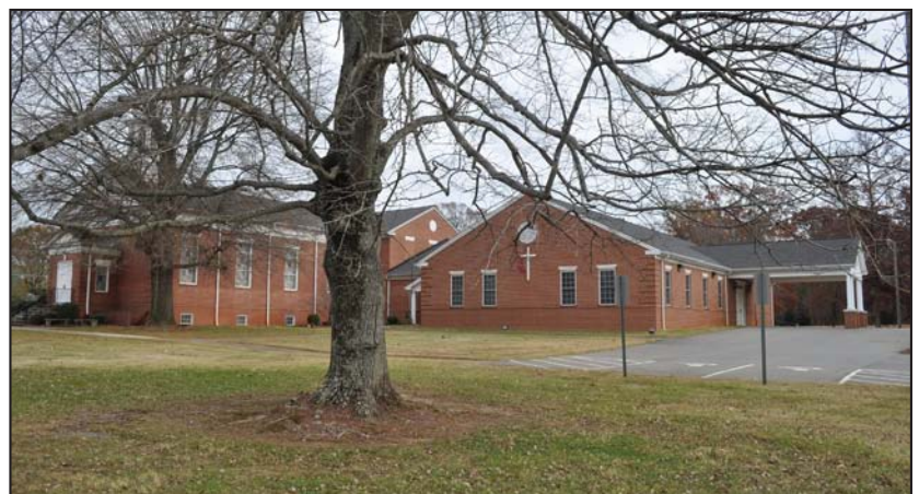
Figure 156. Crews United Methodist Church Rear Elevation: Fellowship Hall Addition (Left) and Christian Education Unit Addition (Right)
