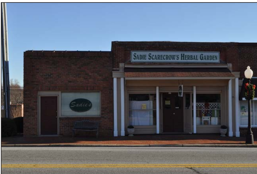
Figure 111. Car Lot Office/Fletcher Powell's Grocery Façade, Southwest Elevation
