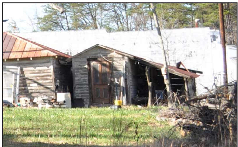
Figure 60. D.A. Jones House Shed, Southeast Elevation
