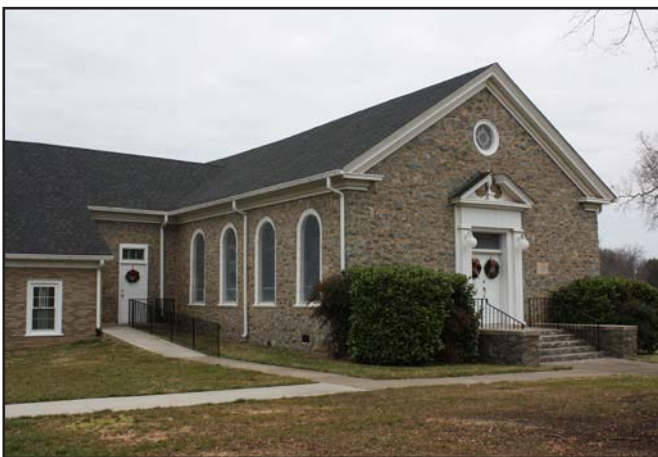
Figure 191. Flat Rock United Methodist Church Sanctuary Façade, South Elevation
