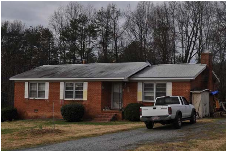
GF 8293 8504 Arapahoe Drive
