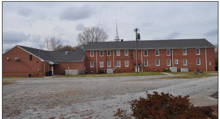
Figure 155. Crews United Methodist Church Sanctuary and Fellowship Hall Addition, West Oblique
