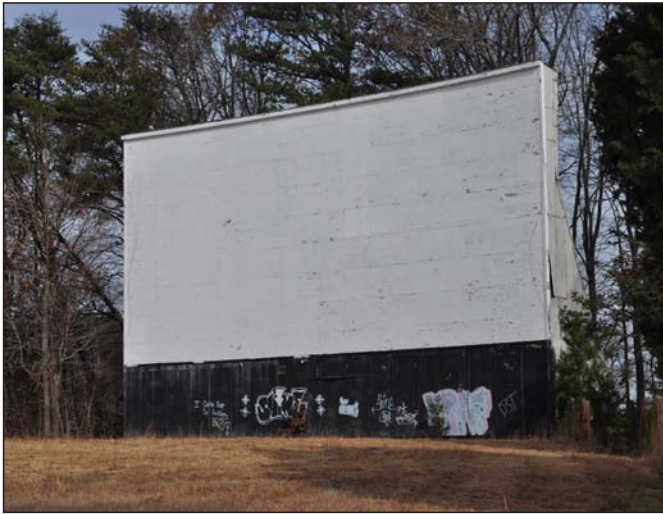
Figure 176. Screen, View East
