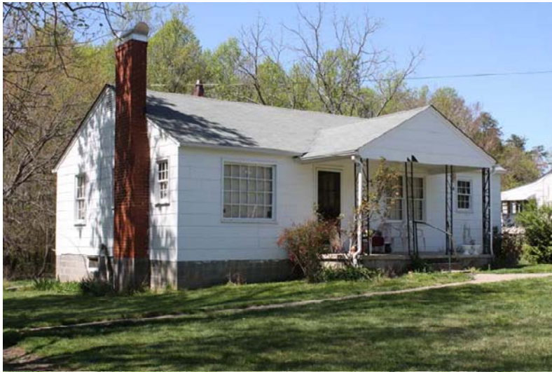
GF 8454 8018 Lester Road
