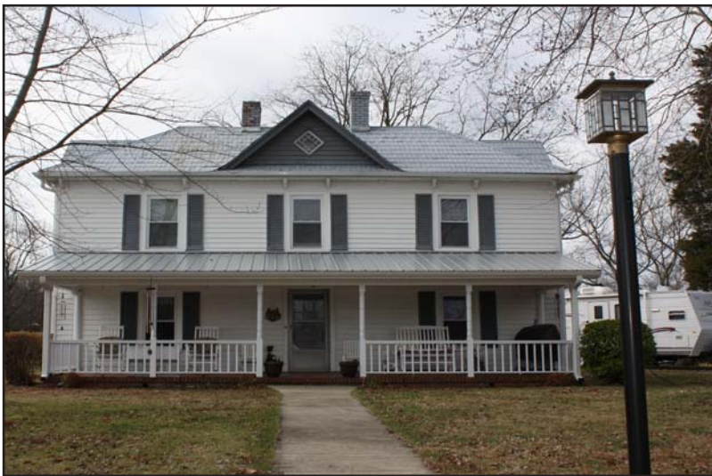
Figure 42. Vaughn House Façade, Northeast Elevation
