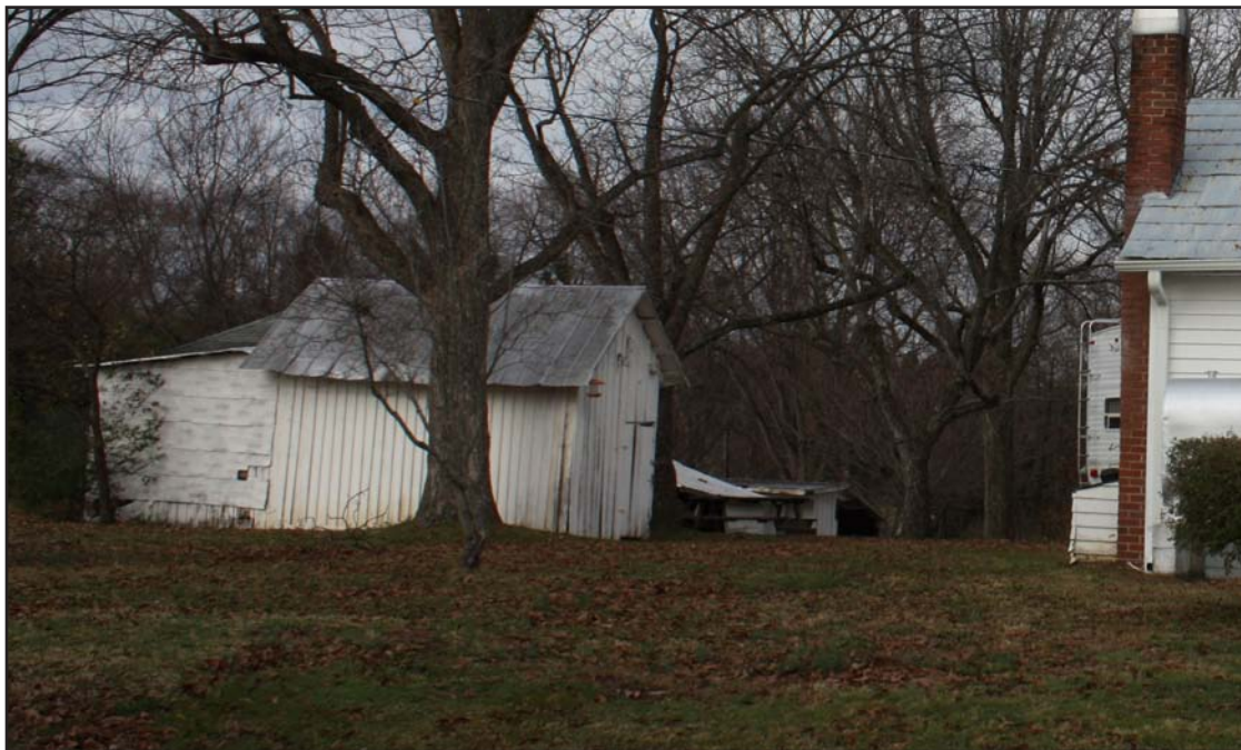
Figure 45. Vaughn House Shed, East Oblique
