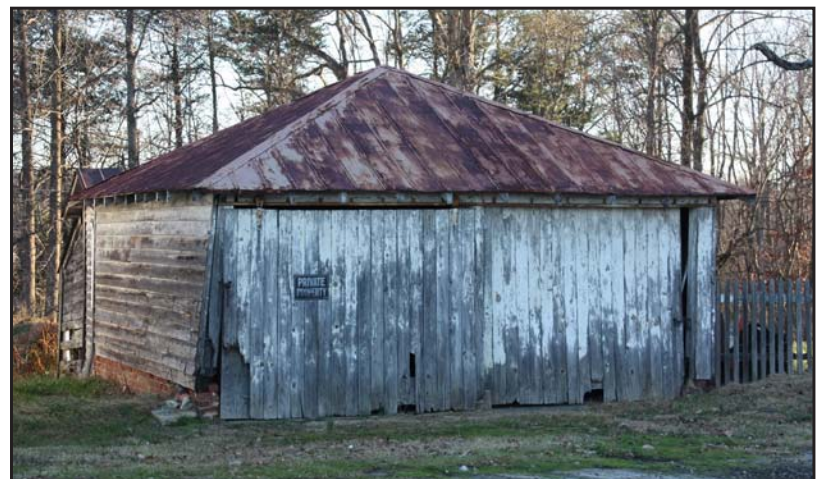
Figure 59. D.A. Jones House Garage, Southwest Elevation
