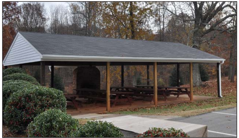
Figure 154. Crews United Methodist Church Picnic Shelter, North Oblique
