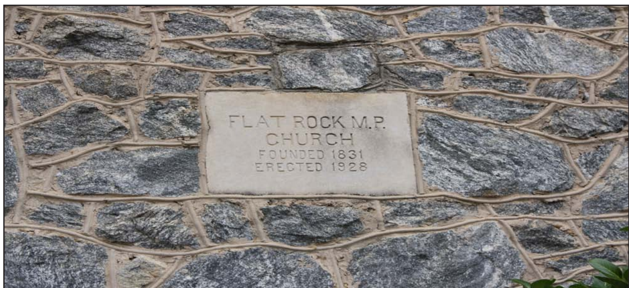
Figure 187. Cornerstone, Flat Rock United Methodist Church Sanctuary, Façade
