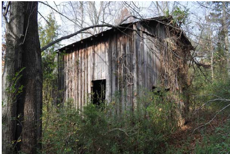
FY 4073 Between 5129 and 5153 Reidsville Road (no street address)
