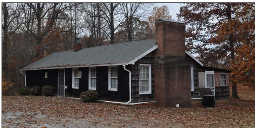
Figure 153. Crews United Methodist Church 1979 Parsonage, East Oblique
