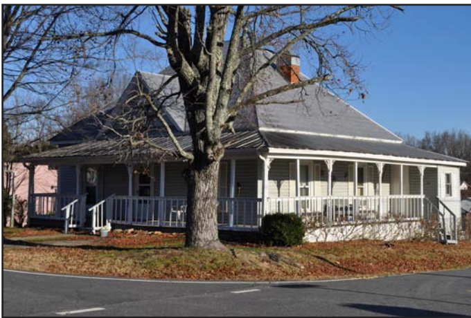
Figure 130. GF 8342 South Oblique
