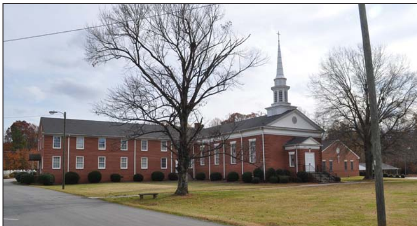
Figure 151. Crews United Methodist Church, North Oblique
