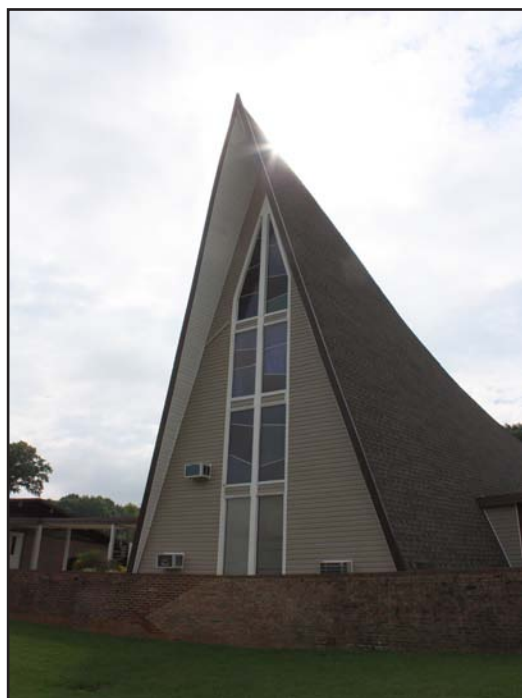
Figure 7. Edgewood Baptist Church Sanctuary Rear Elevation, West Oblique
