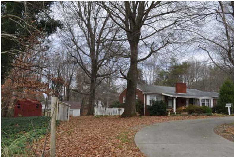
GF 8291 8508 Arapahoe Drive
