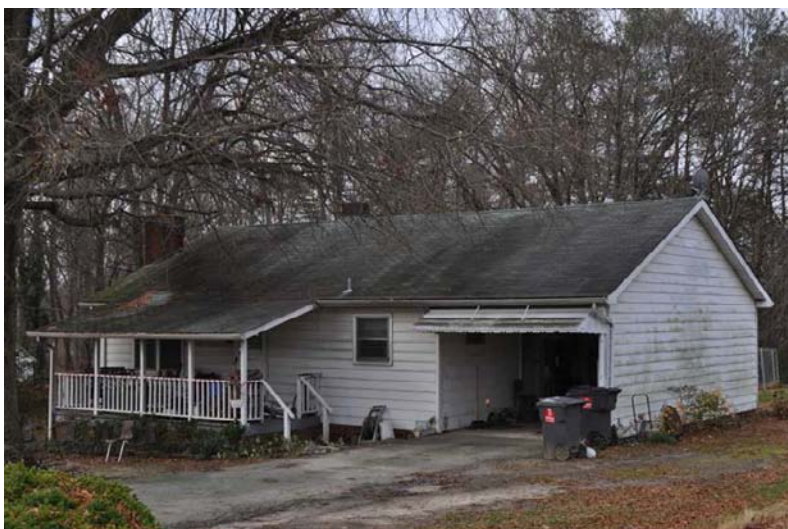
GF 8292 8506 Arapahoe Drive
