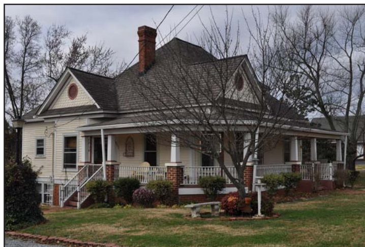
Figure 41. Stokesdale Methodist Church Parsonage East Oblique
