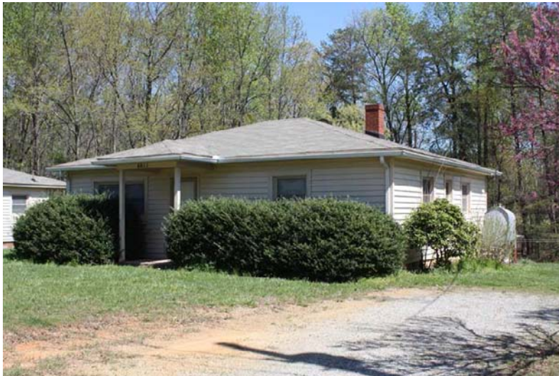
GF 8458 8011 Lester Road
