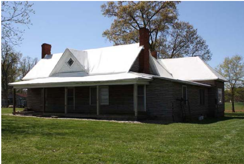
GF 8467 8013 Treeline Road
