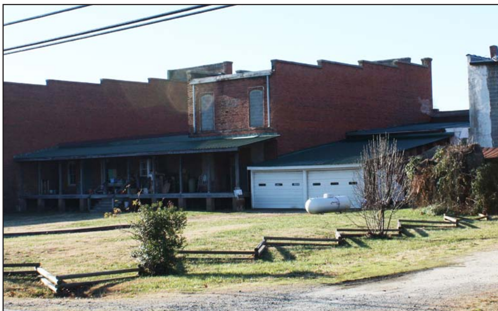
Figure 84. Preston's Grocery North Oblique
