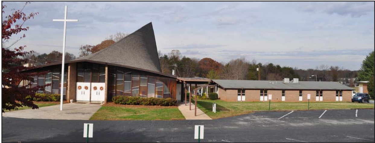
Figure 12. Edgewood Baptist Church Sanctuary and North Education Building, Southwest Elevation
