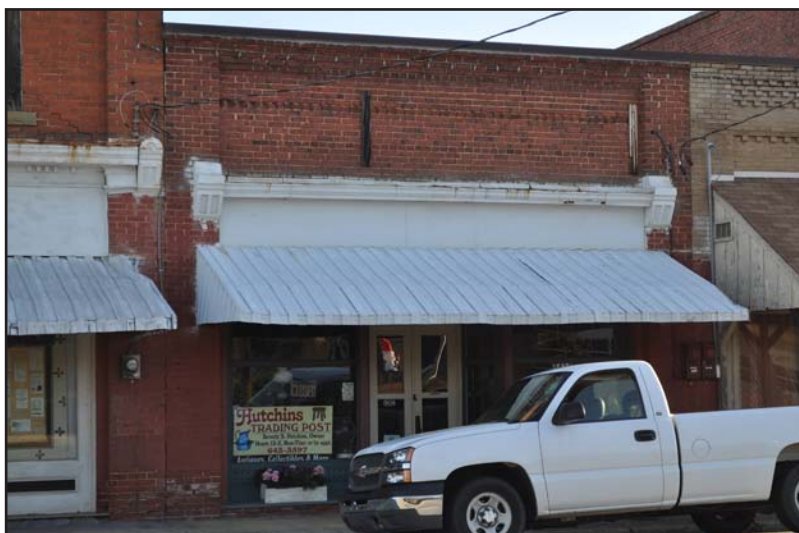
Figure 86. United States Post Office #2 Façade, Southwest Elevation
