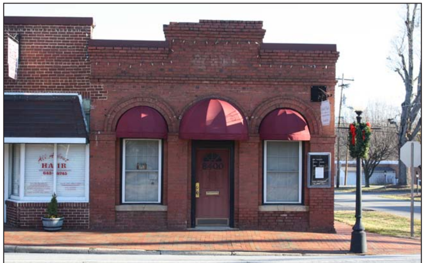
Figure 120. Stokesdale Commercial Bank Façade, Southwest Elevation
