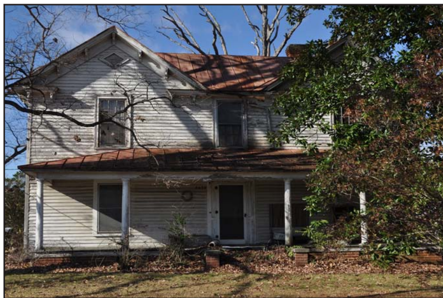
Figure 56. D.A. Jones House Façade, Southeast Elevation
