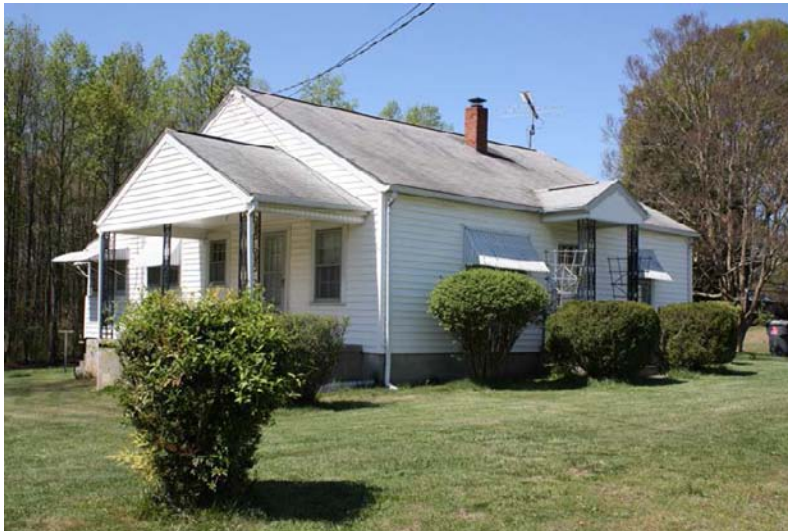
GF 8455 8016 Lester Road
