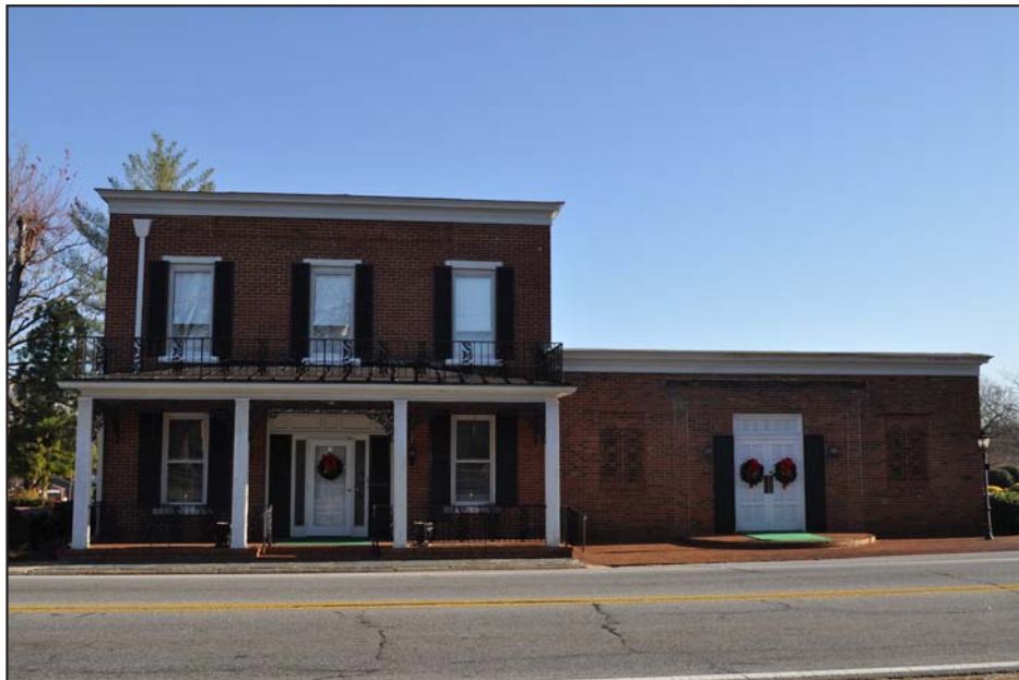
Figure 127. Stokesdale Hotel Façade, Southwest Elevation
