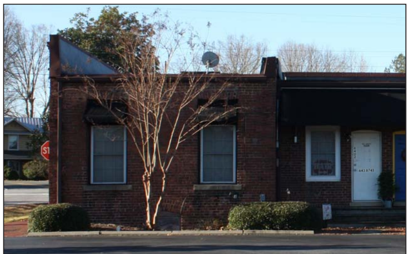
Figure 121. Stokesdale Commercial Bank Northeast Elevation
