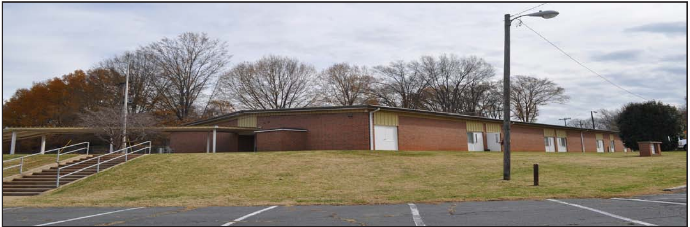
Figure 16. Edgewood Baptist Church School Building, West Oblique Gymnasium [G]
