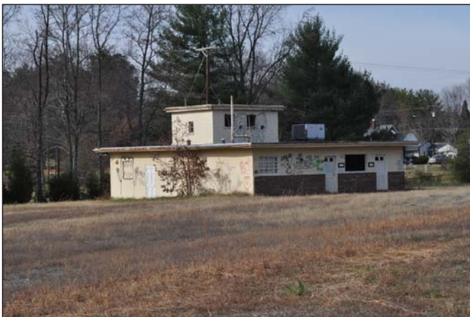
Figure 177. Bel Air Drive-In Theater Concession Stand/Restroom Building, Southeast Oblique
