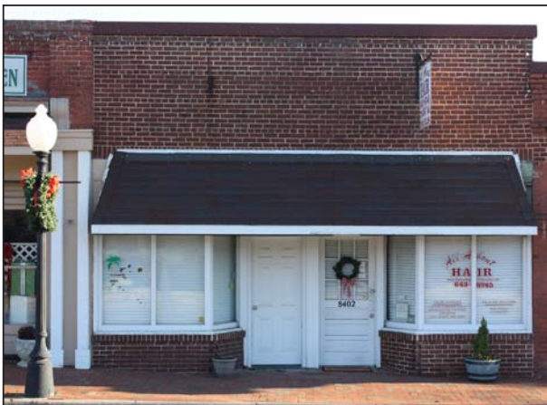
Figure 115. Hot Dog Stand/Lawyer's Office Façade, Southwest Elevation
