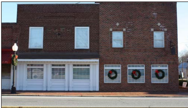
Figure 108. United States Post Office #3 Former Façade, Southwest Elevation
