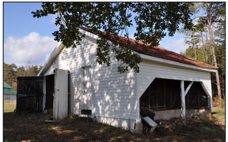
Figure 169. Lowery-Martin House Equipment Barn, South Oblique
