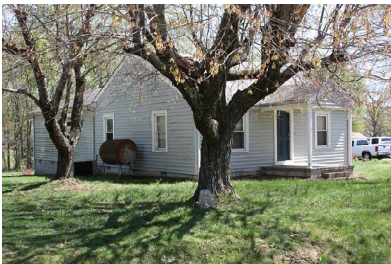
GF 8456 8015 Lester Road
