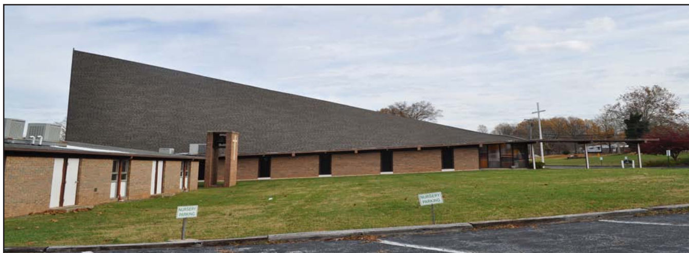
Figure 6. Edgewood Baptist Church Sanctuary Parabolic Roof, Southwest Elevation
