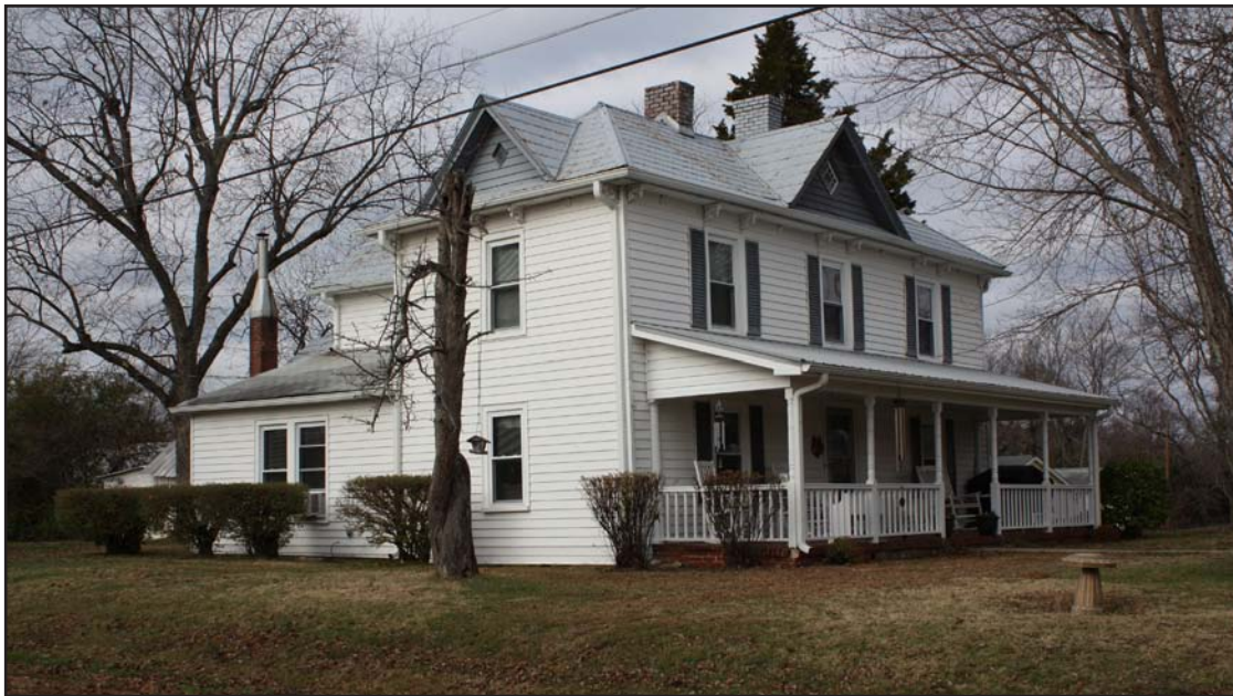
Figure 44. Vaughn House East Oblique
