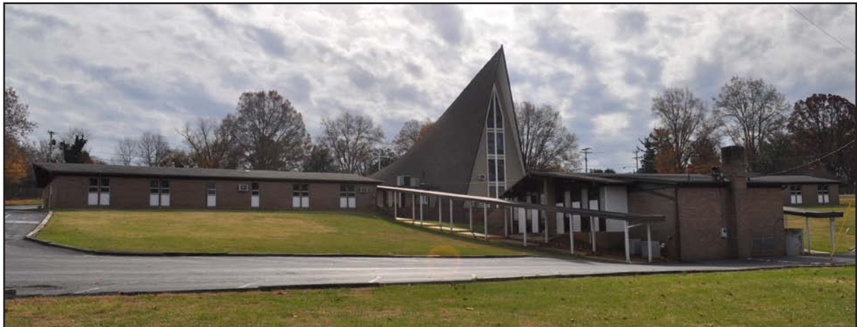
Figure 13. Edgewood Baptist Church North Education Building, Sanctuary, and Fellowship Hall, North Oblique
