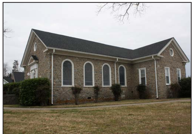
Figure 192. Flat Rock United Methodist Church Sanctuary, Southeast Oblique
