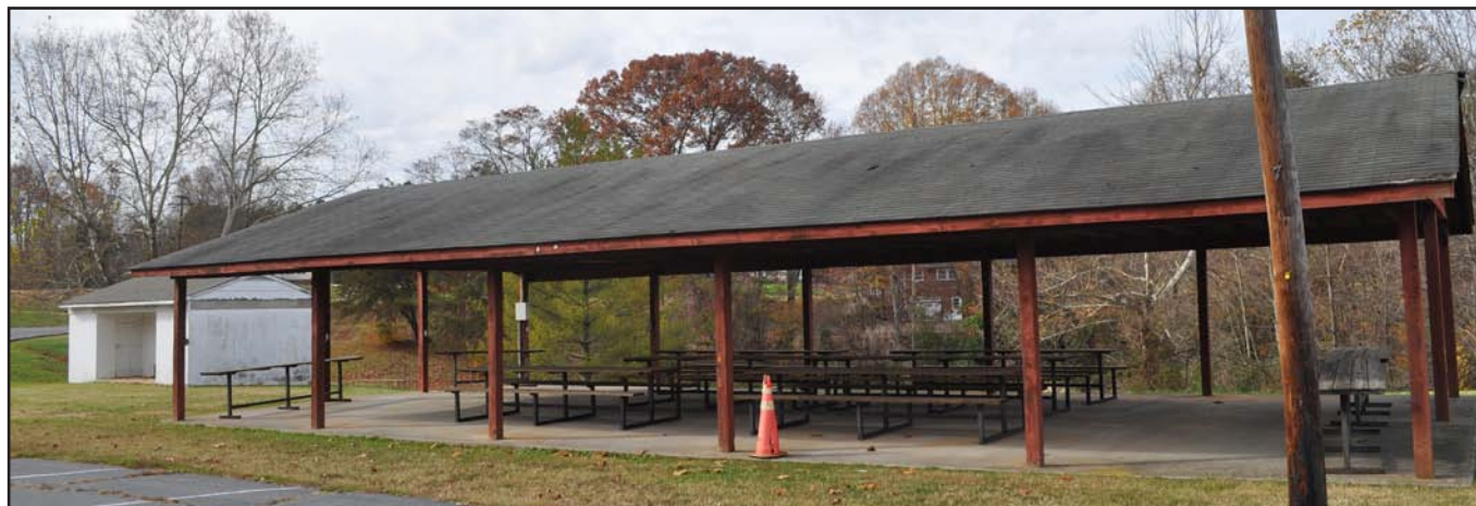
Figure 18. Edgewood Baptist Church Picnic Shelter (Right) and Comfort Station (Left)
