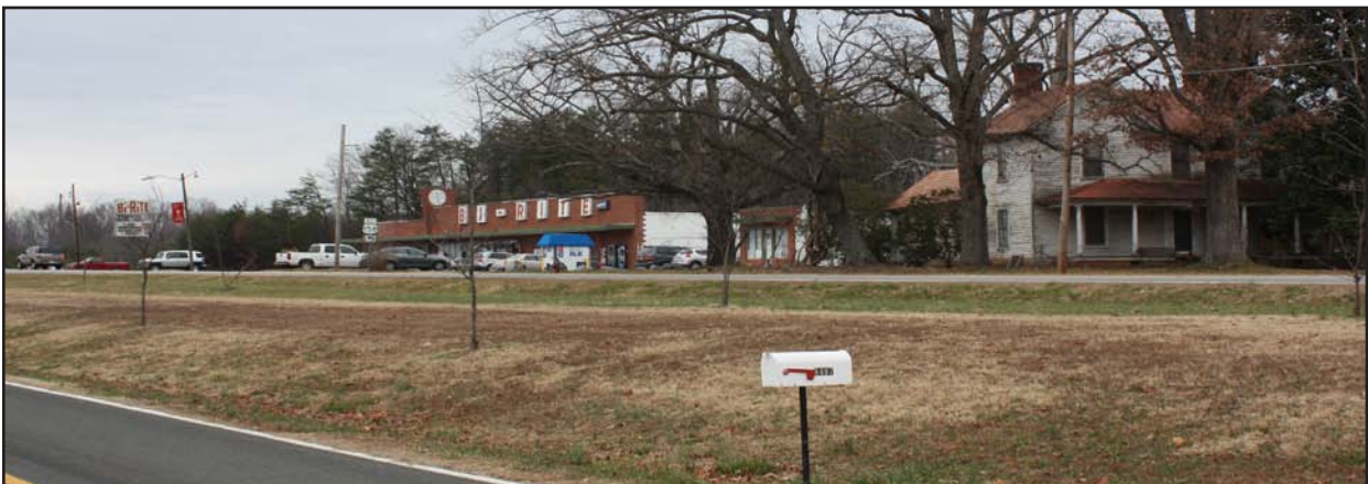
Figure 34. Northern Boundary at Bi-Rite Supermarket (GF 8327, Left) with D.A. Jones House (GF 1702, Right), View North
