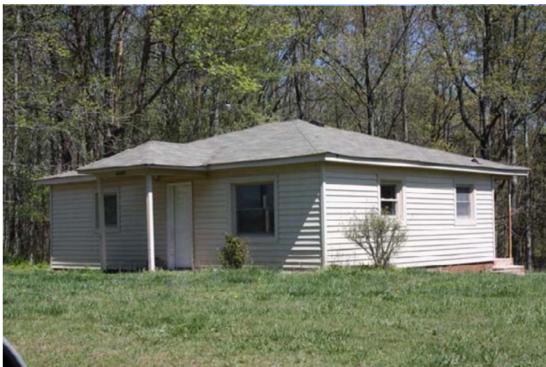
GF 8459 8010 Lester Road
