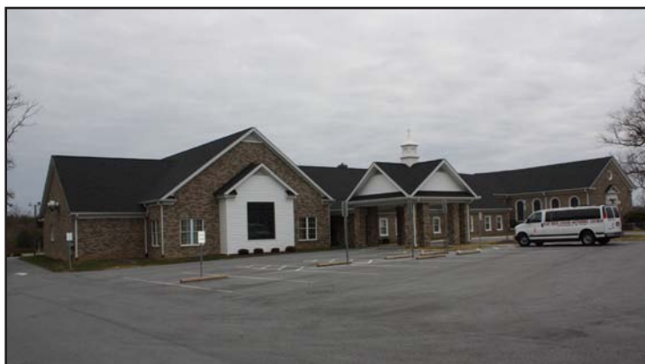
Figure 193. Flat Rock United Methodist Church Sanctuary Façade, South Elevation
