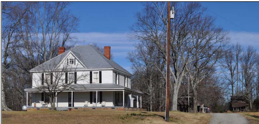
Figure 142. Wray House and Outbuildings, View North
