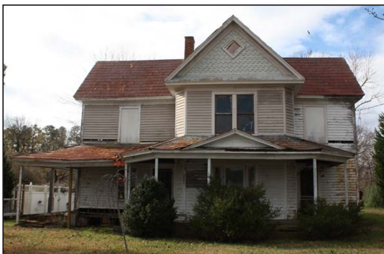
Figure 49. Knight House #2 Façade, Northeast Elevation
