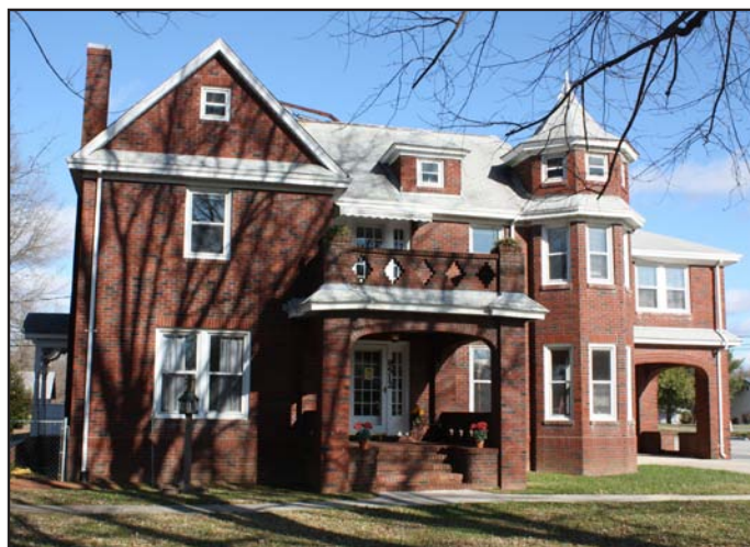
Figure 62. Taylor-Edwards House Façade, Southwest Elevation
