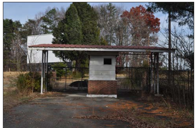
Figure 180. Bel Air Drive-In Theater Ticket Booth, View Southeast
