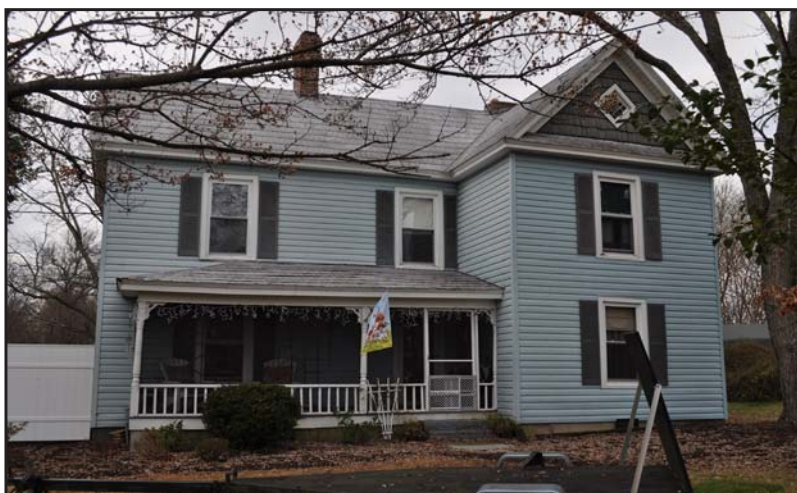
Figure 46. Knight House #1 Façade, Northeast Elevation
