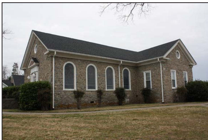
Figure 195. Flat Rock United Methodist Church Sanctuary, Southeast Oblique
