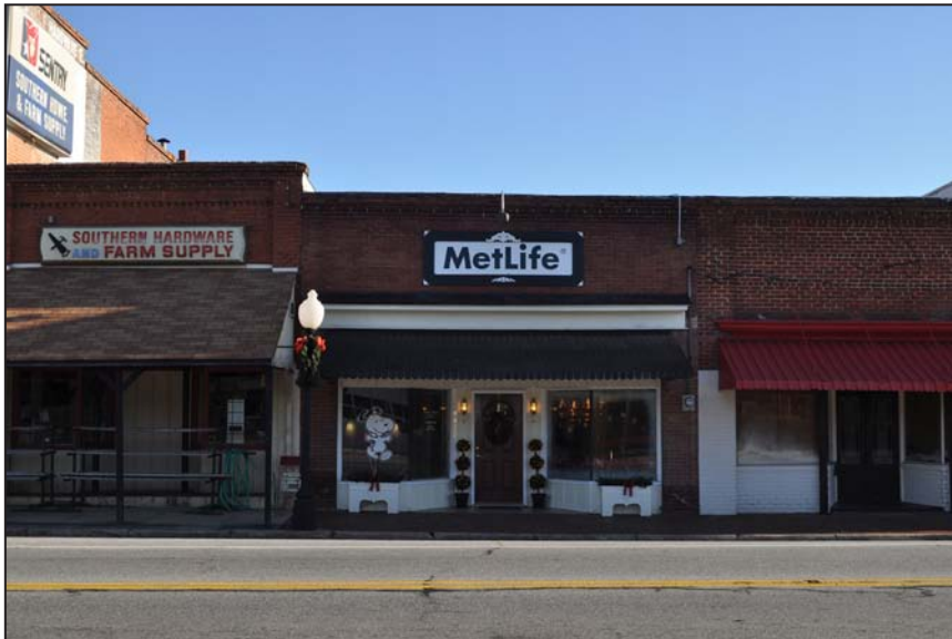
Figure 103. Western Auto Contextual Façade, Southwest Elevation
